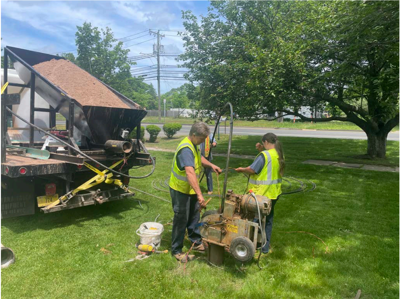
Picture 11: Grela placing sand into the well located on the 272 Main Street, Durham, property as part of well decommissioning activities. View to the east.
