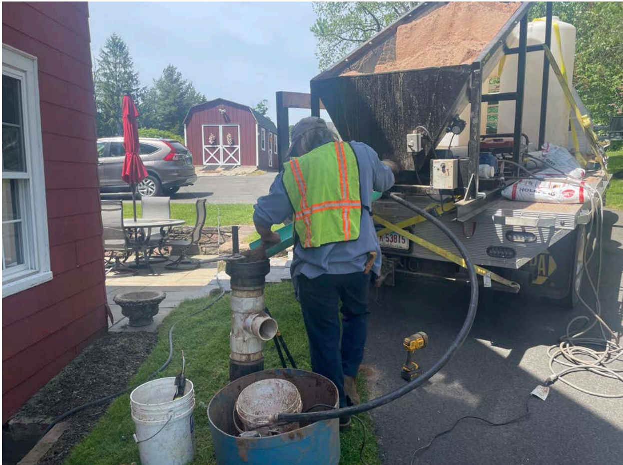
Picture 8: Grela placing sand into the well located on the north side of the 186 Main Street, Durham, property as part of well decommissioning activities. View to the west.
