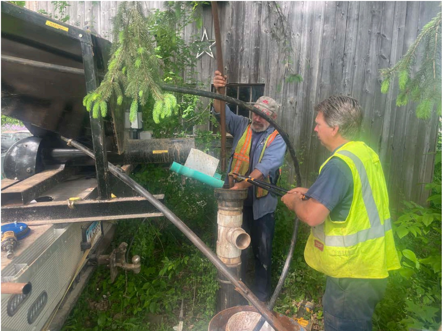
Picture 6: Grela placing sand into the well located at the 208 Main Street, Durham, property as part of well decommissioning activities. View to the southwest.
