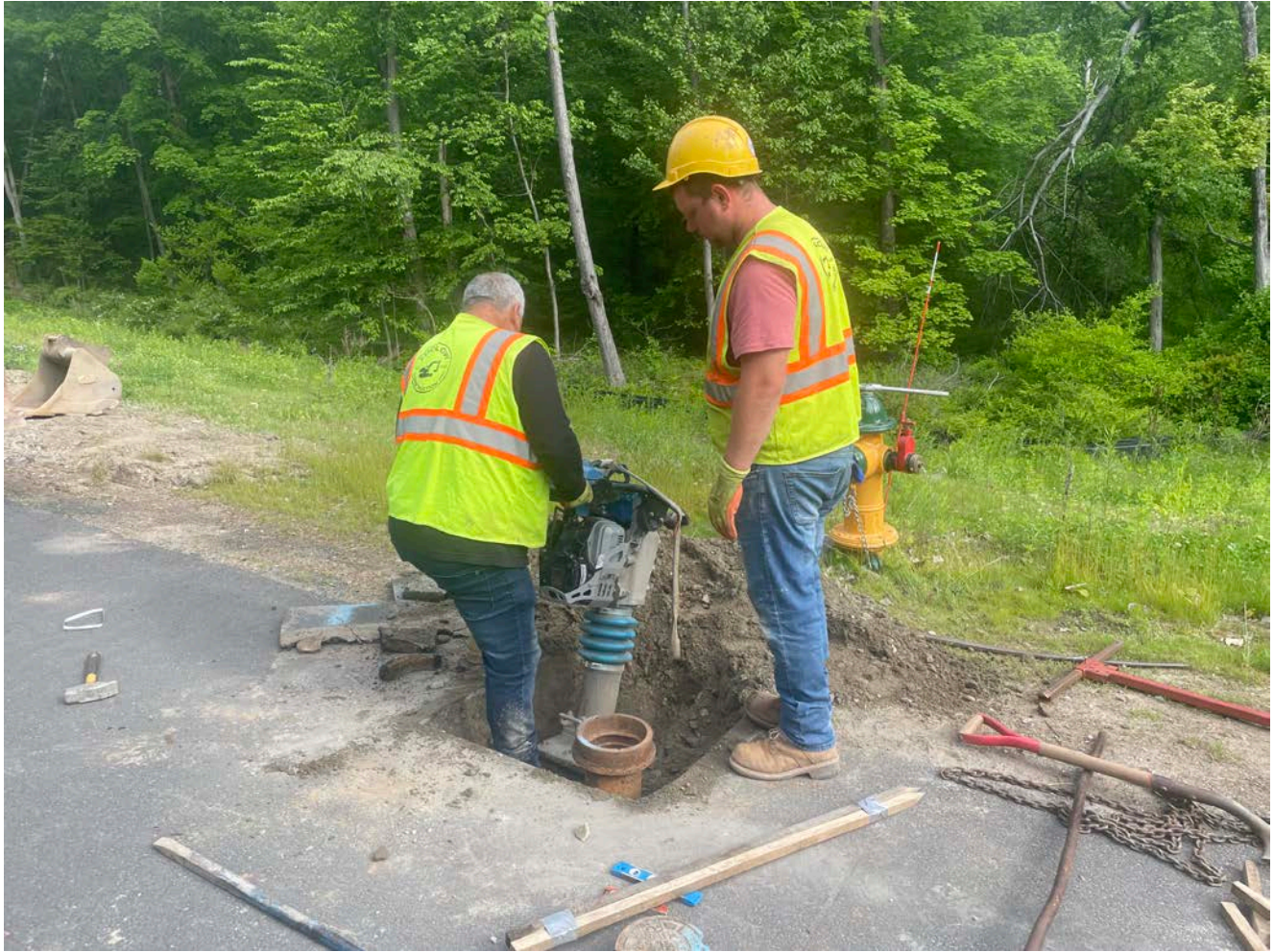
Picture 2: Ludlow compacting soil around the roadbox located at Station ~14+70 after Ludlow raised it by several inches ahead of an upcoming paving event. View to the north.
