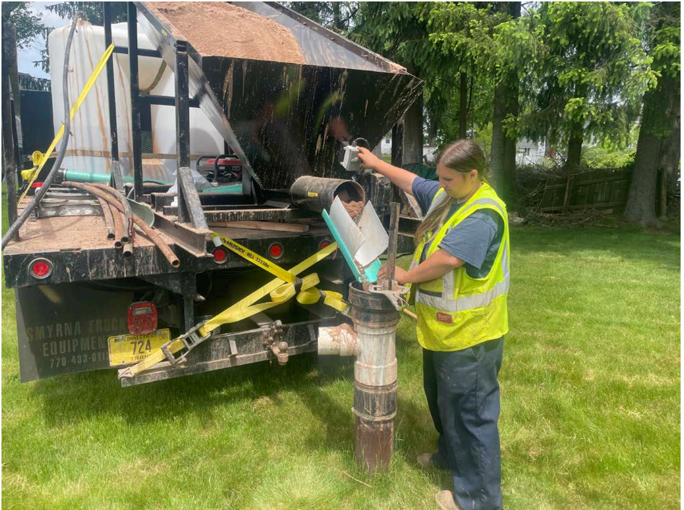
Picture 9: Grela placing sand into the well located on the 176 Main Street, Durham, property as part of well decommissioning activities. View to the northwest.
