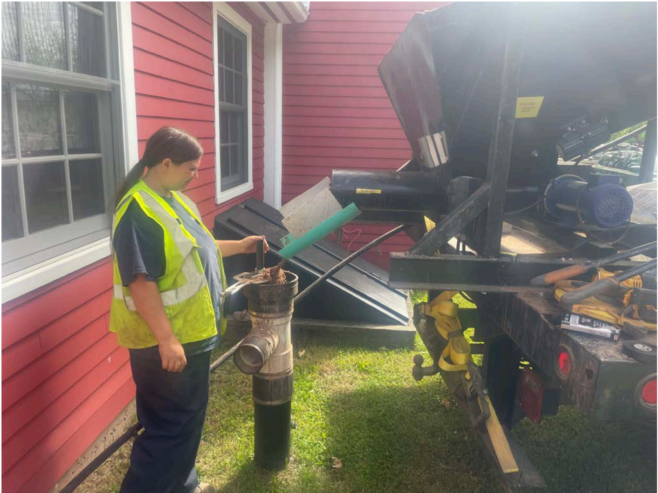
Picture 5: Grela placing sand into the well located on the south side of the 216 Main Street, Durham, residence as part of well decommissioning activities. View to the east.
