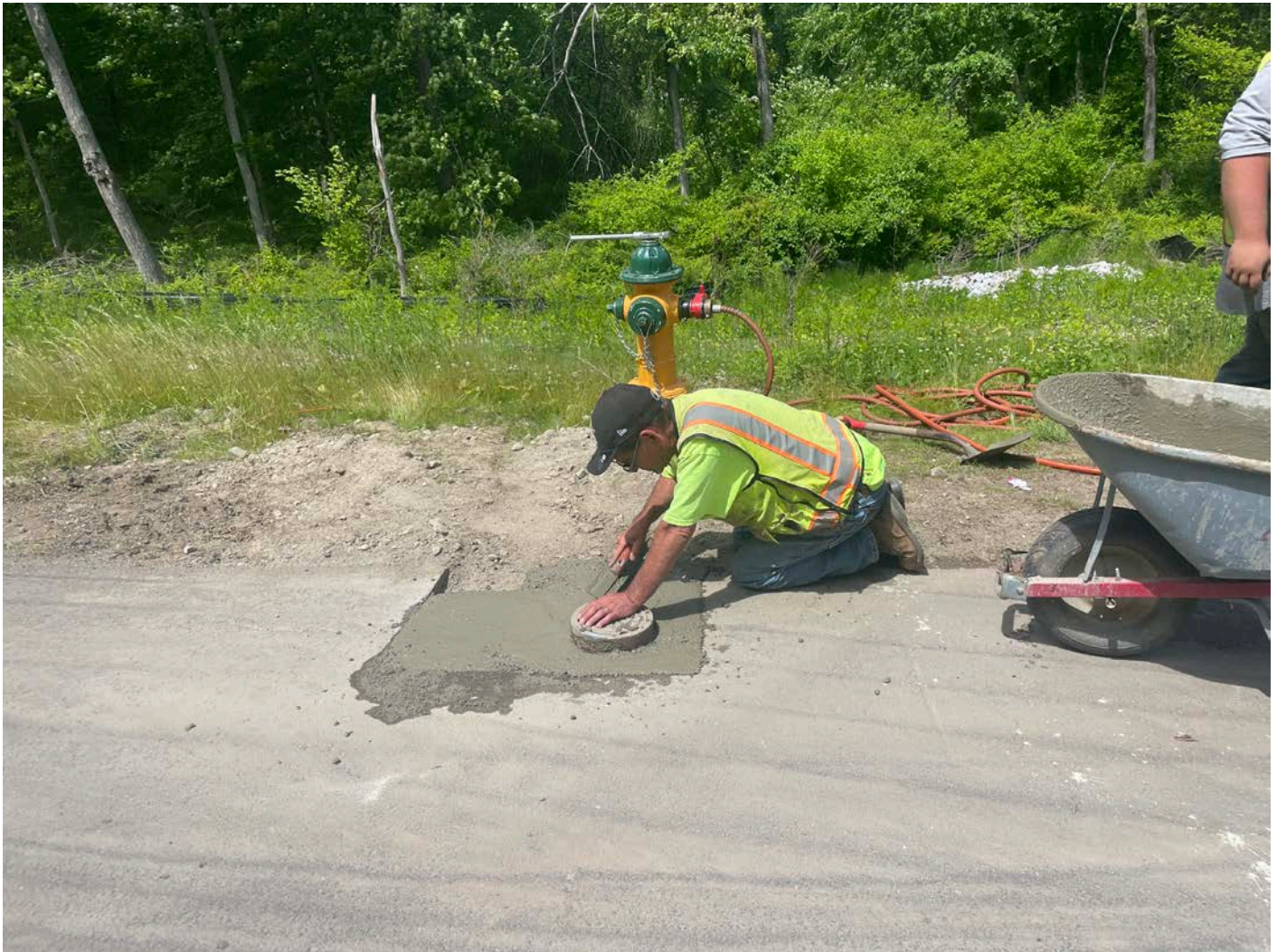
Picture 12: Ludlow placing concrete around the roadbox located at Station ~14+70 on the Shared Access Driveway in Middletown. View to the north.
