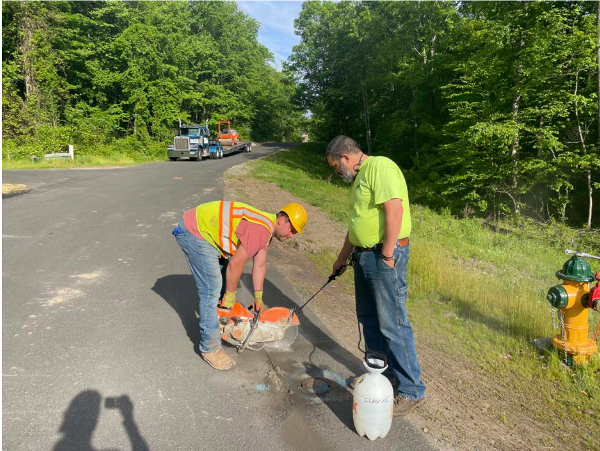
Picture 1: Ludlow saw-cutting pavement around a roadbox located at Station ~14+70 on the north side of the Shared Access Driveway as they prepare to raise it ahead of an upcoming paving event. View to the west.
