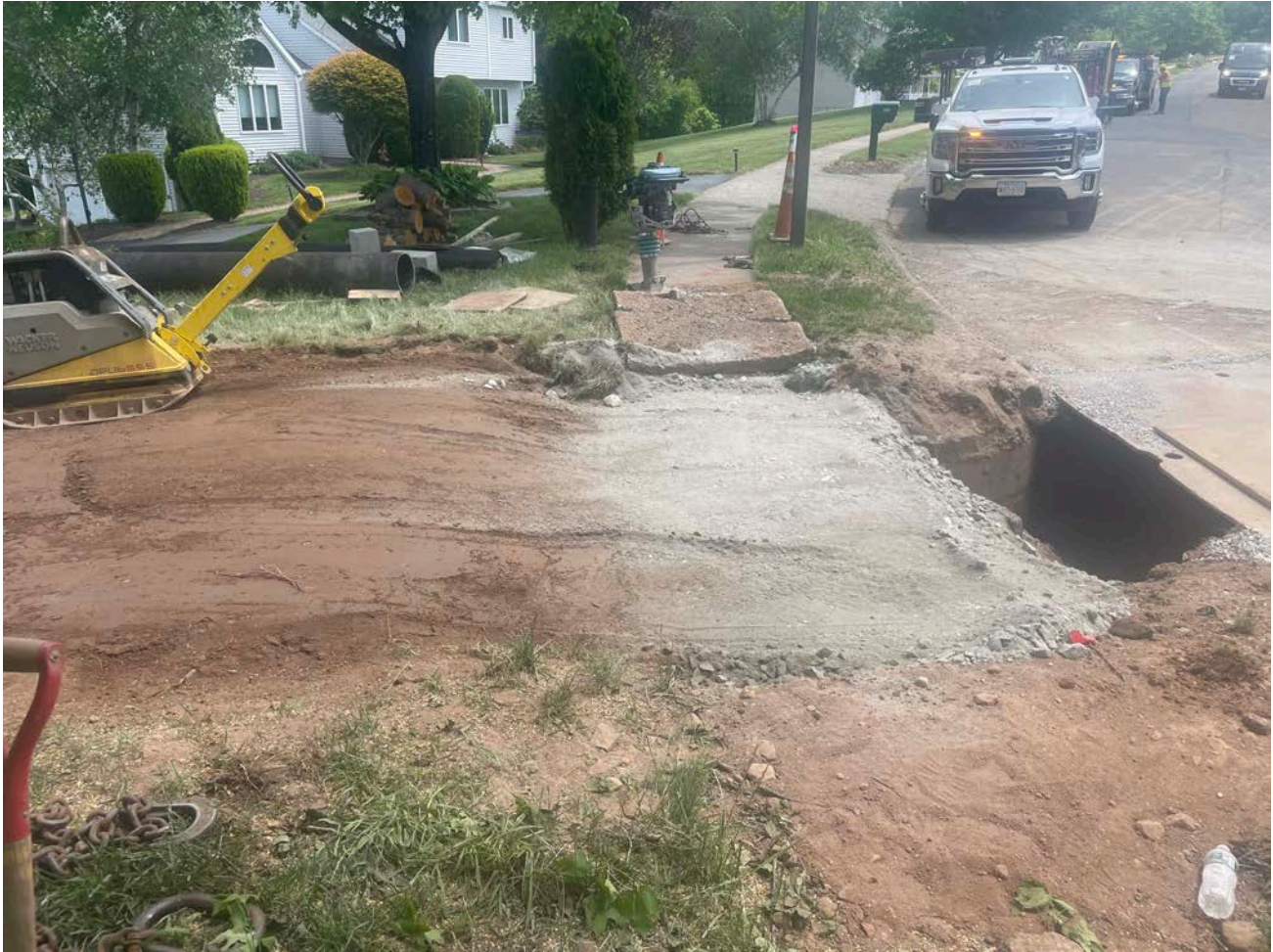
Picture 10: Station 40+41 where Ludlow has partially backfilled the excavation they made to tie in the 12" water line coming in from Round Hill Road to the 16" DIP waterline that Ludlow installed on Talcott Ridge Drive. View to the west.
