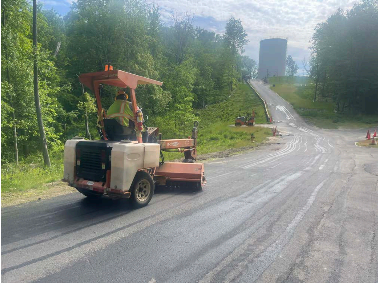
Picture 4: Ludlow using a Broce Broom to clean the Shared Access Driveway in Middletown. View to the east.
