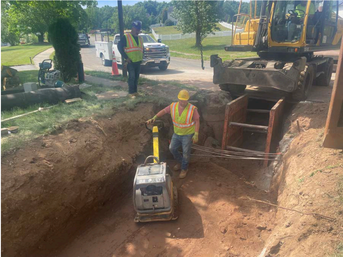
Picture 7: Ludlow compacting fill that is being placed in 1' lifts over the 12" DIP they installed at Station 40+41 on Talcott Ridge Drive, Middletown. View to the southeast.
