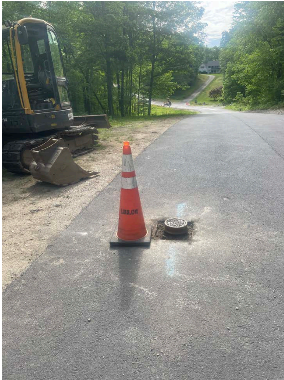
Picture 3: Roadbox located at Station 17+91 on the north side of the Shared Access Driveway that Ludlow raised ahead of an upcoming paving event. View to the east.
