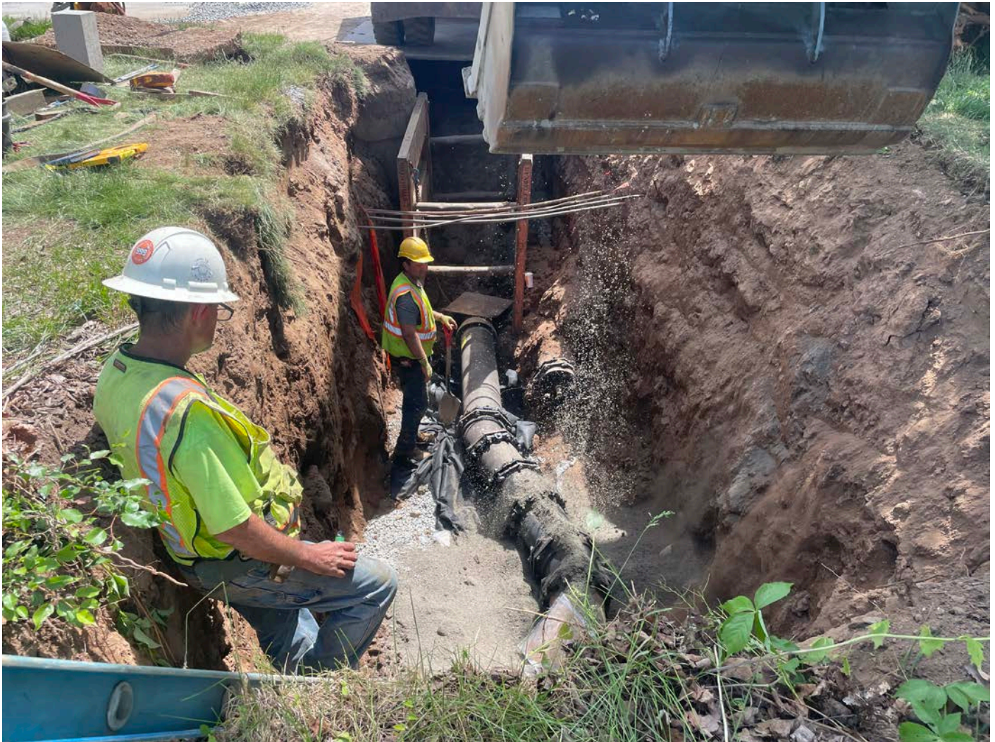
Picture 12: Ludlow placing sand over the 12" DIP they installed while connecting the 12" DIP water line coming in from Round Hill Road to the 16" DIP on Talcott Ridge Drive in Middletown at Station 40+41. View to the south.
