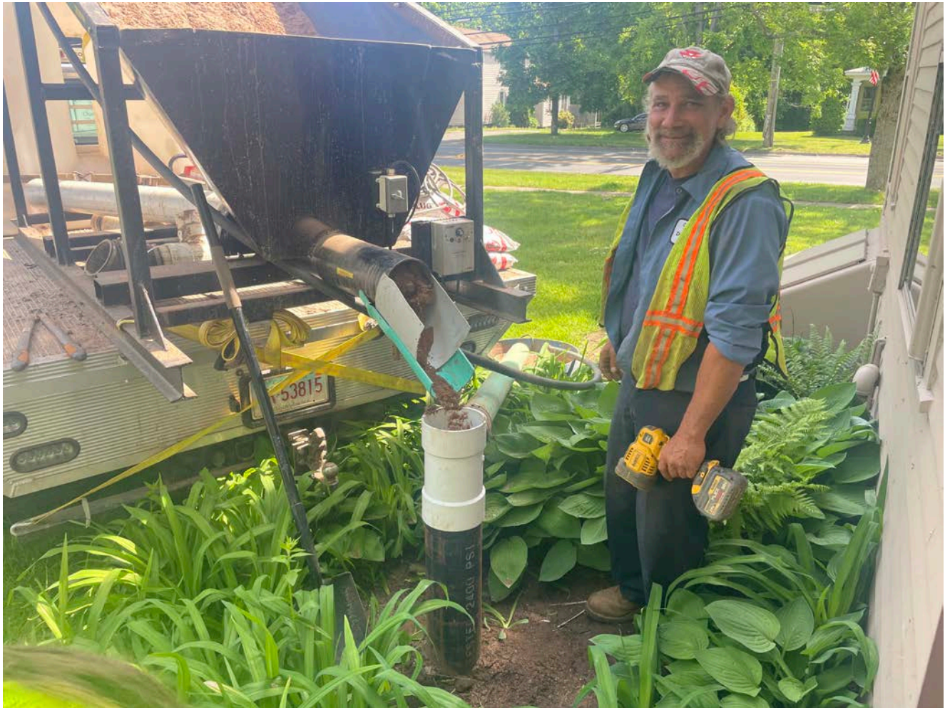
Picture 2: Grela placing sand into the well located on the north side of the 228 Main Street, Durham, building as part of well decommissioning activities. View to the east.
