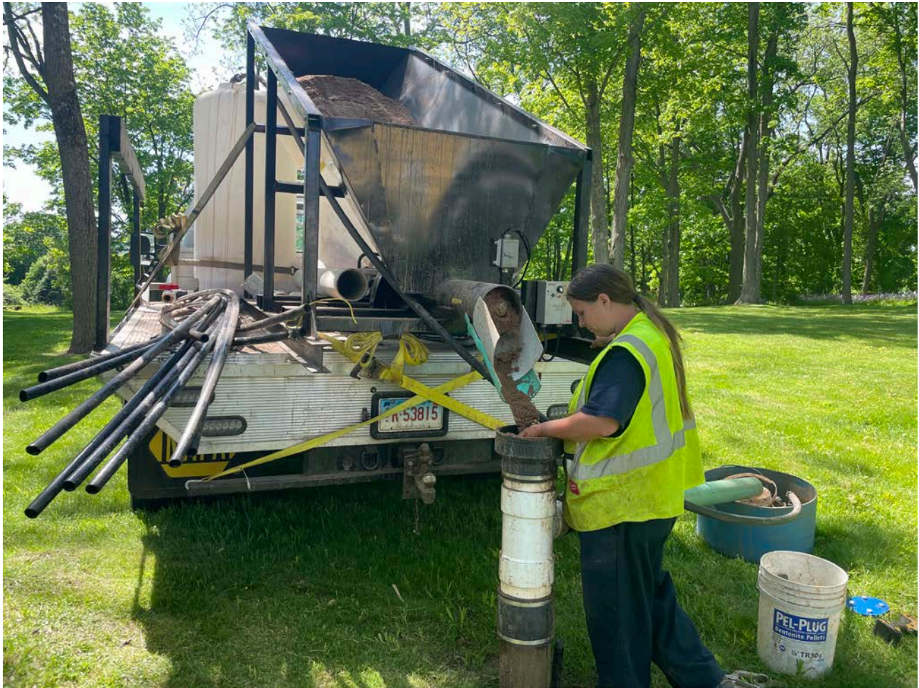
Picture 5: Grela placing sand into the well located on the west side of the 202 Main Street, Durham, property as part of well decommissioning activities. View to the east.
