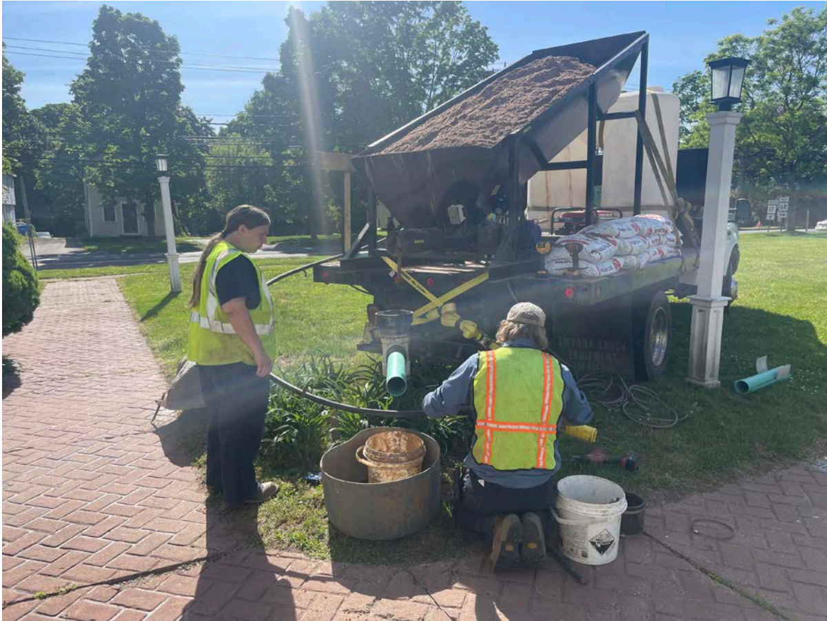
Picture 1: Grela setting up to decommission the well located on the south side of the 236 Main Street, Durham, building. View to the east.
