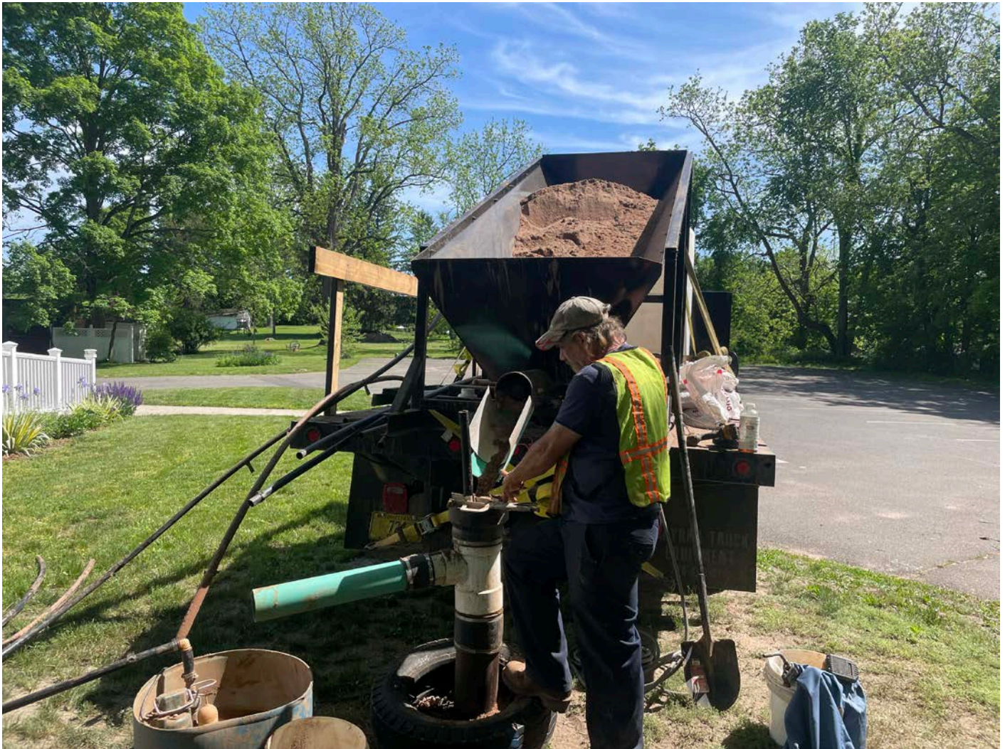
Picture 6: Grela placing sand into the well located on the west side of the 196 Main Street, Durham, building as part of well decommissioning activities. View to the south.
