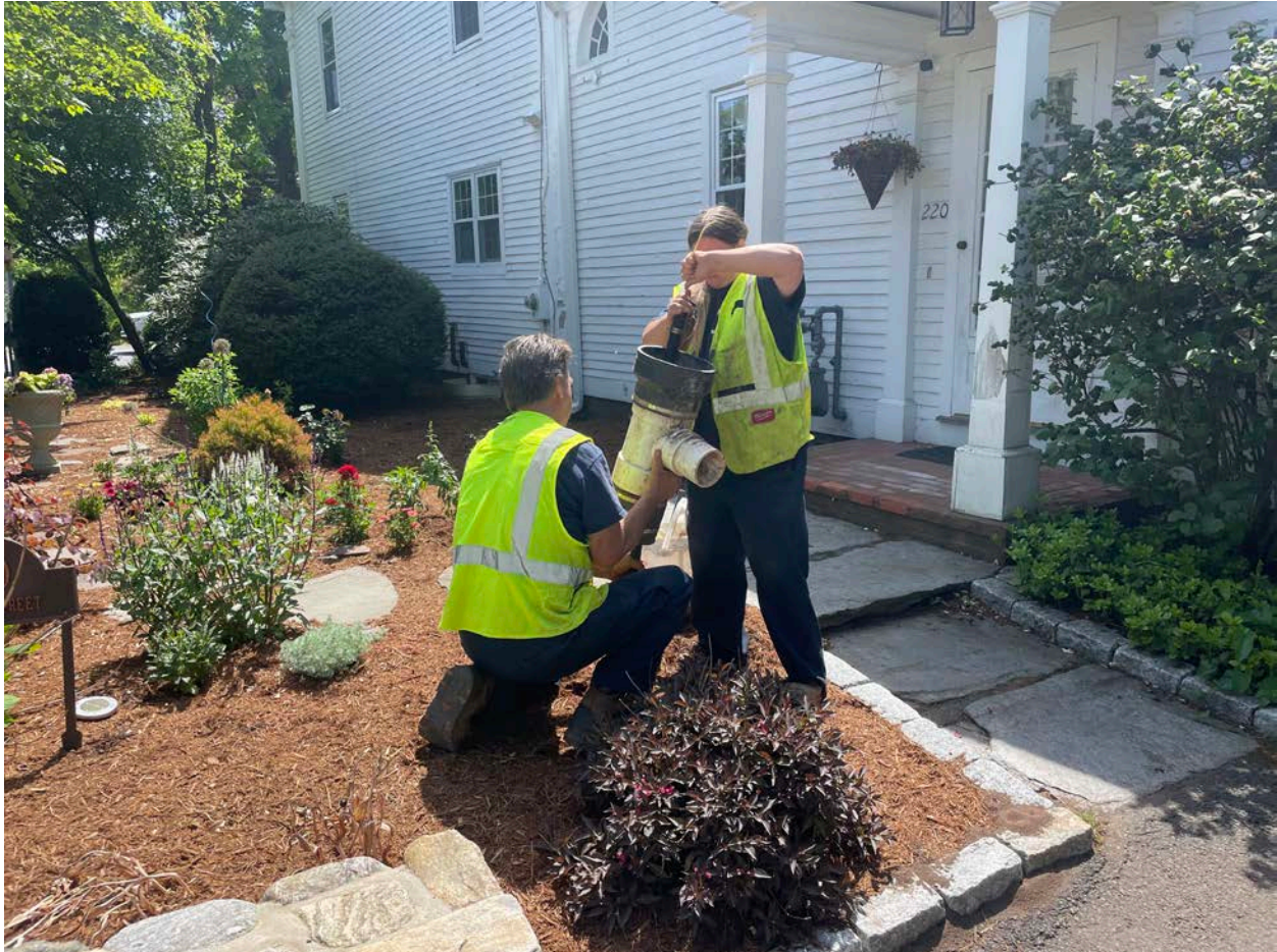
Picture 3: Grela setting up to decommission the well located on the north side of the 220 Main Street, Durham, building. View to the southeast.
