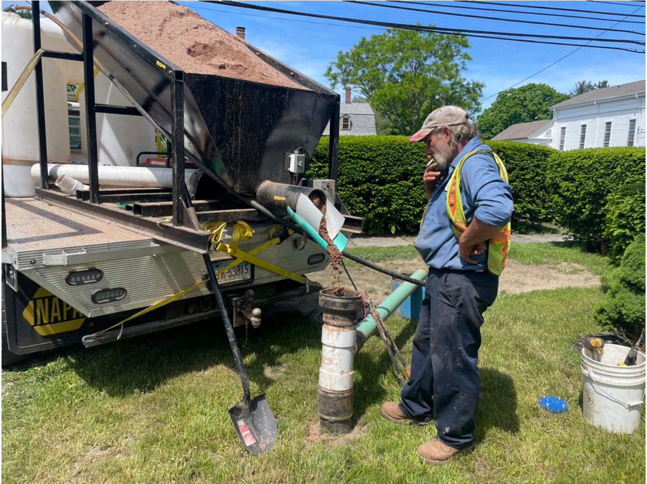
Picture 4: Grela placing sand into the well located on the south side of the 227 Main Street, Durham, building as part of well decommissioning activities. View to the west.
