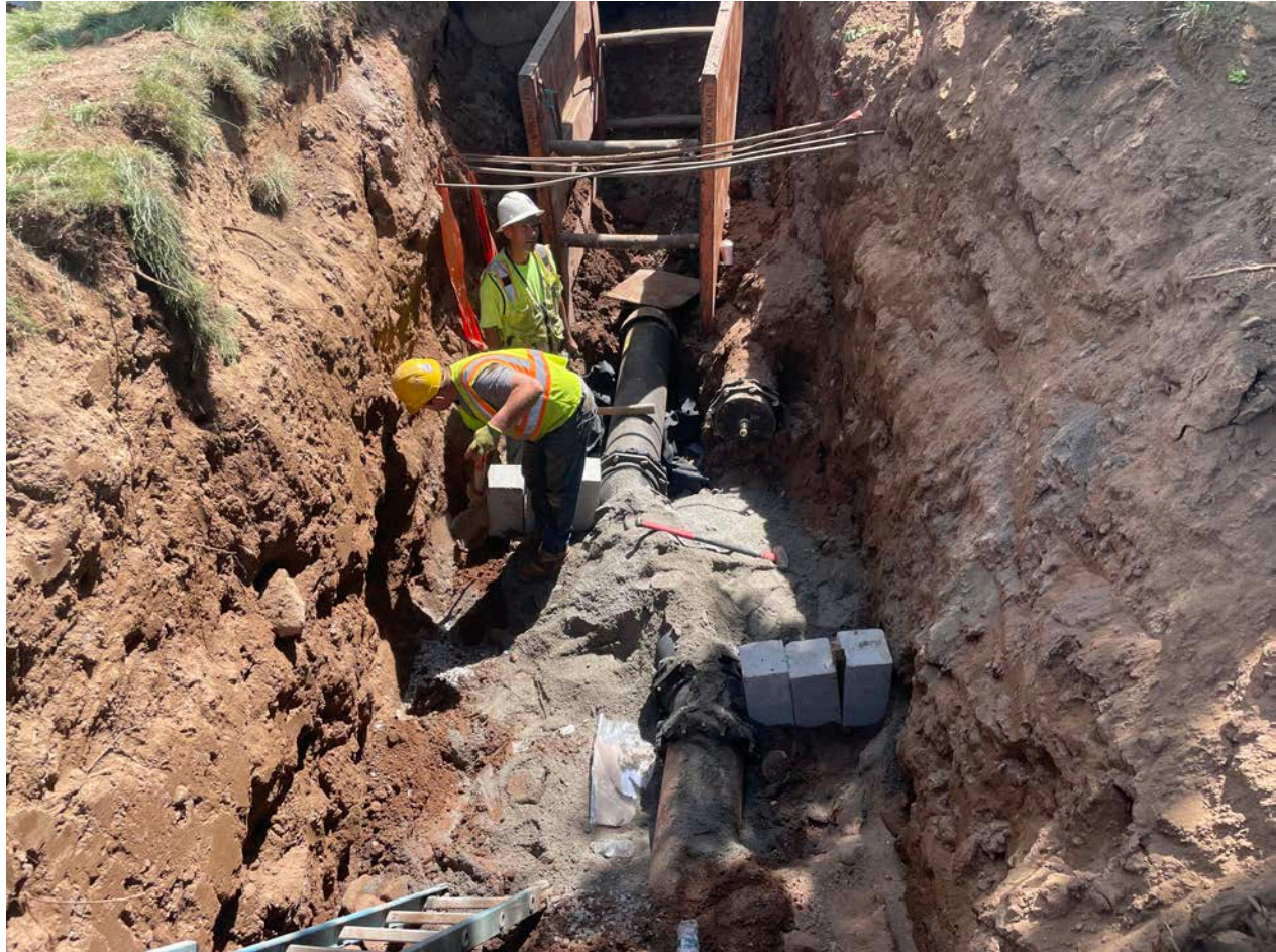
Picture 13: Ludlow placing thrust blocks on the bends in the 12" DIP they installed while connecting the 12" DIP water line coming in from Round Hill Road to the 16" DIP on Talcott Ridge Drive in Middletown at Station 40+41. View to the south.
