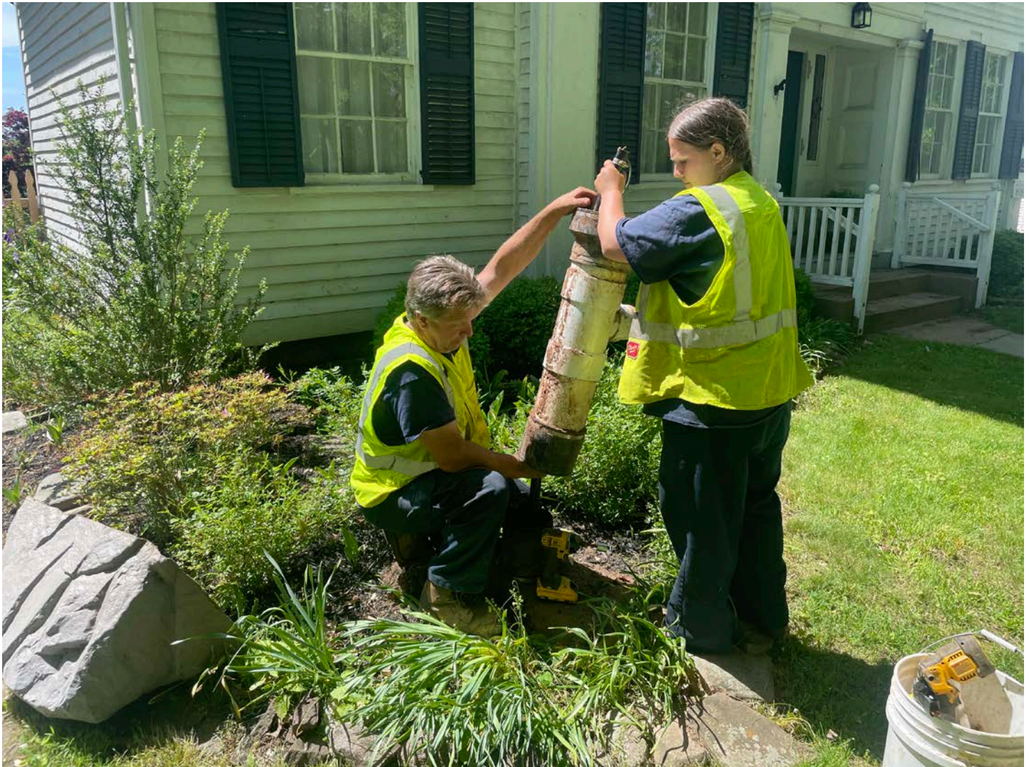
Picture 10: Grela placing sand into the well located on the east side of the 246 Main Street, Durham residence as part of well decommissioning activities. View to the north.
