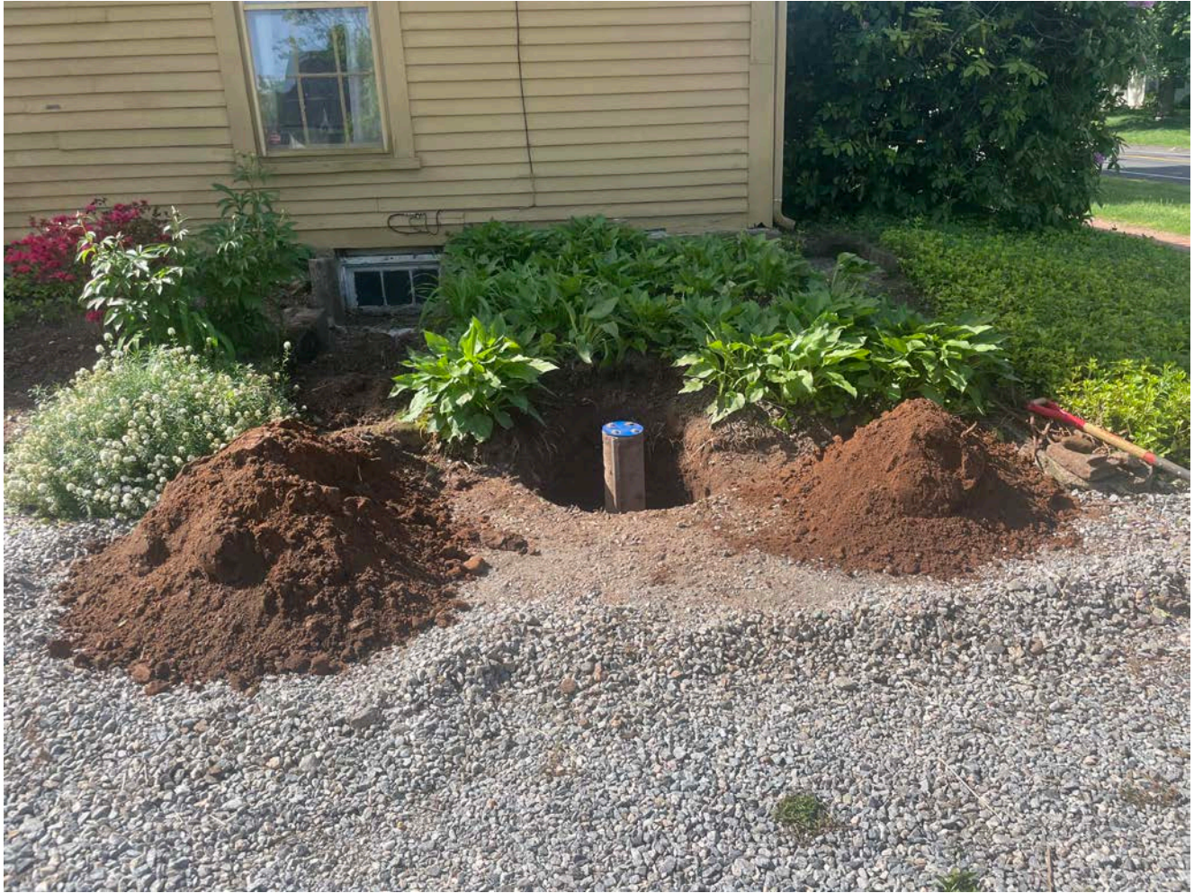
Picture 2: The well located on the north side of the 257 Main Street, Durham, residence that Ludlow has excavated around to allow Grela to cut the well casing 2' below surface grade. View to the south.
