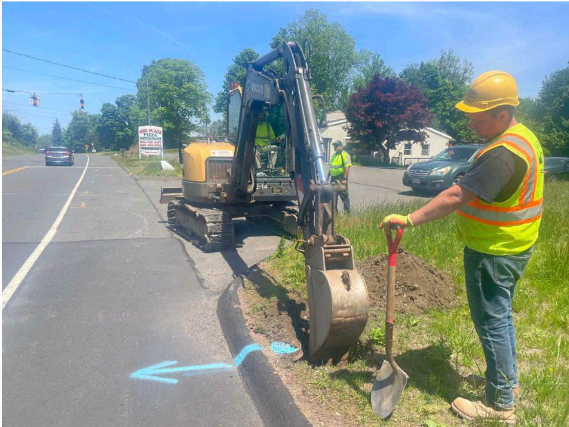
Picture 8: Ludlow excavating around the road box located at Station 750+59 on S. Main Street, Durham as they work to center it over the valve stem to an 8" M.J. gate valve. View to the north.
