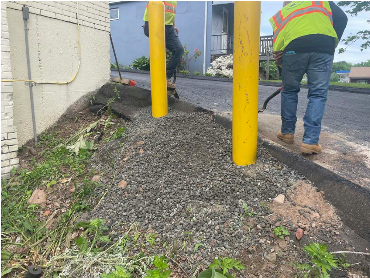
Picture 1: Ludlow placing ¾” stone over the spot where Grela removed the well for the 325 Main Street, Durham, building. View to the northwest.
