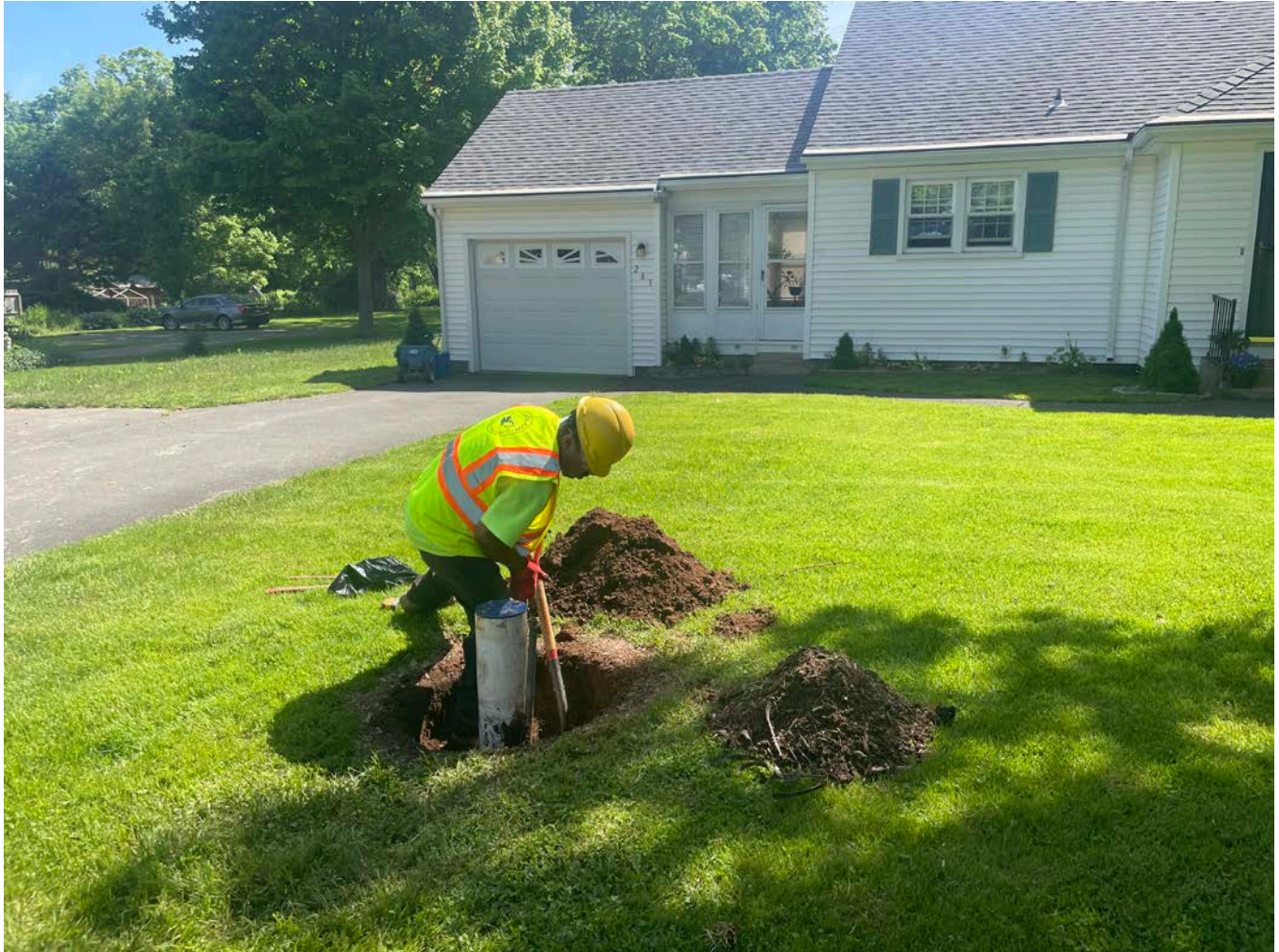
Picture 4: Ludlow hand-excavating around the 6" PVC casing of the well located on the west side of the 261 Main Street, Durham residence. This is being done to provide Grela room to cut the casing 2' below surface grade as part of well decommissioning activities. View to the northeast.
