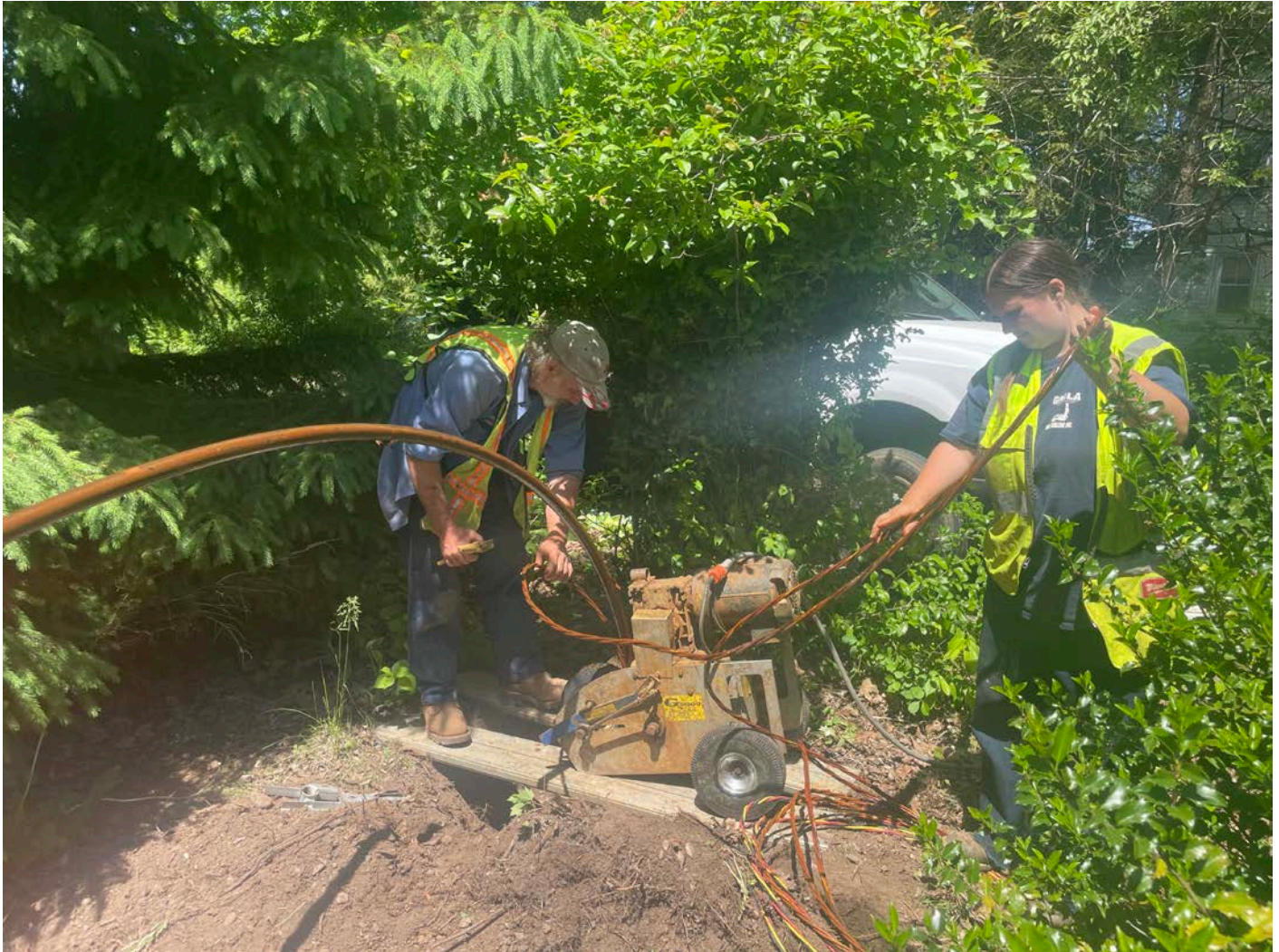
Picture 6: Grela pulling the pump from the well located on the north side of the 308 Main Street, Durham residence as part of well decommissioning activities. View to the northwest.
