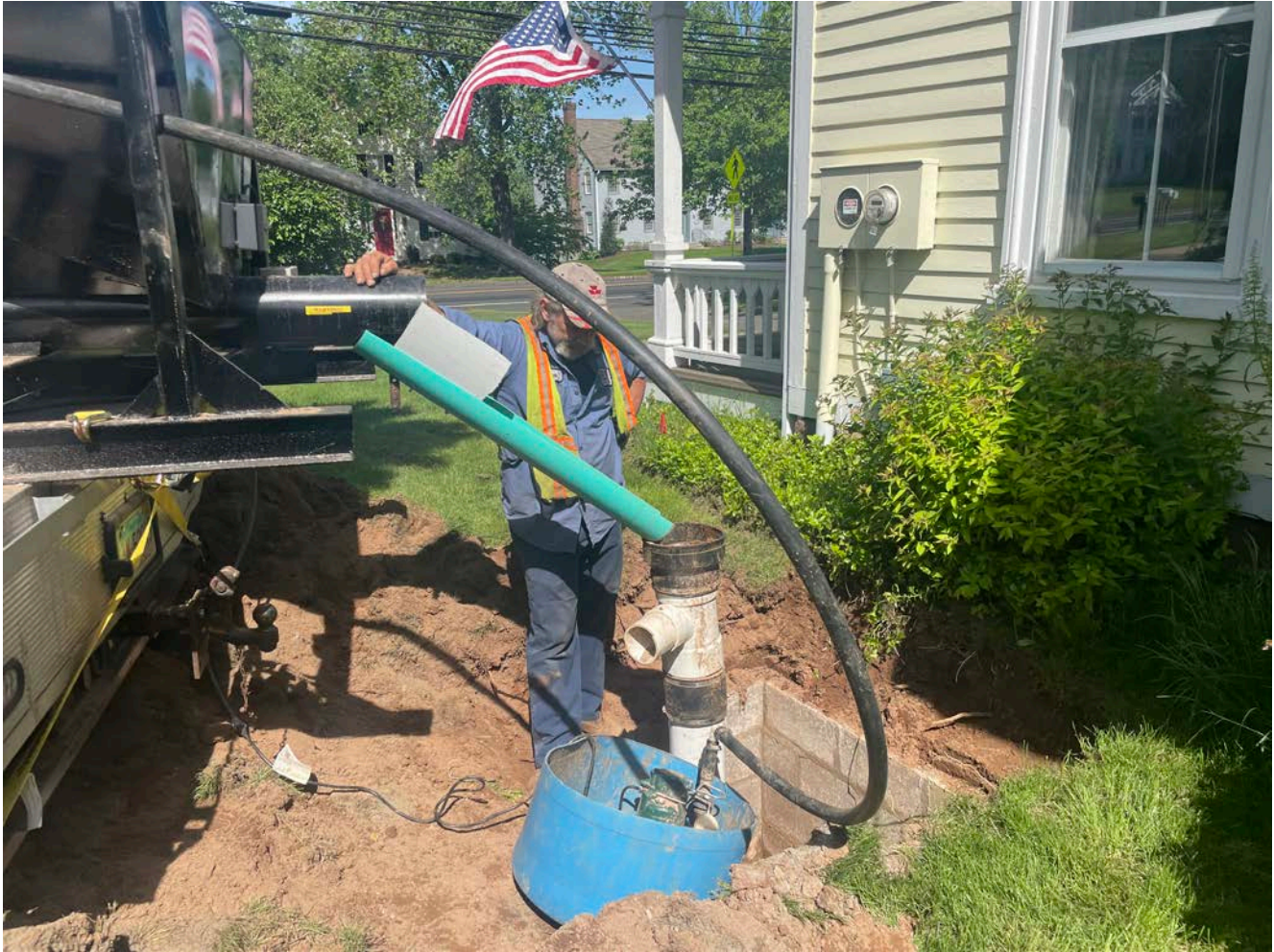
Picture 5: Grela placing sand into the well located on the south side of the 265 Main Street, Durham residence as part of well decommissioning activities. View to the northwest.
