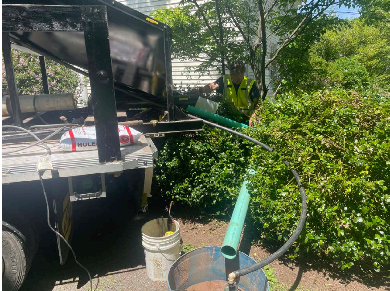
Picture 7: Grela placing sand into the well located on the east side of the 261 Main Street, Durham property as part of well decommissioning activities. View to the northwest.
