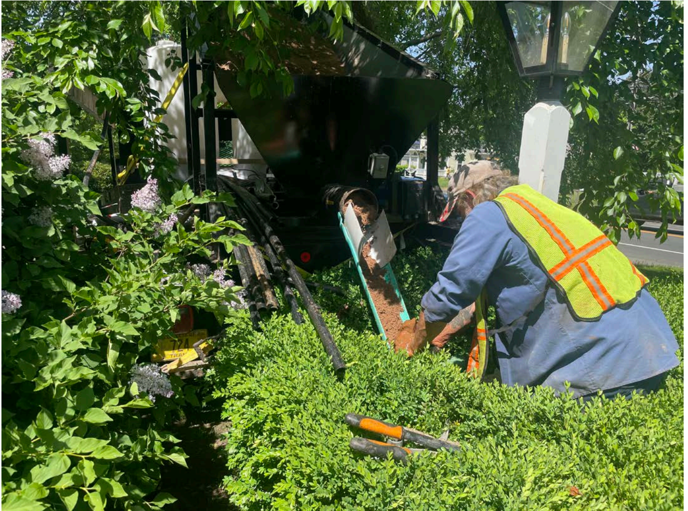
Picture 9: Grela placing sand into the well located on the east side of the 256 Main Street, Durham, residence as part of well decommissioning activities. View to the northeast.
