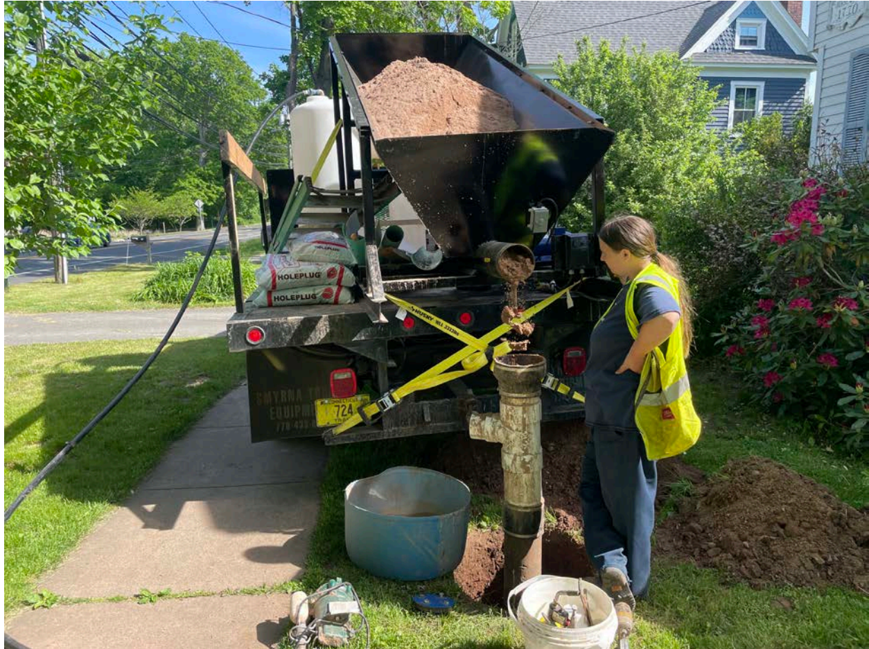
Picture 3: Grela placing sand into the well located on the west side of the 267 Main Street, Durham residence as they work to finish well decommissioning activities on this property. View to the north.
