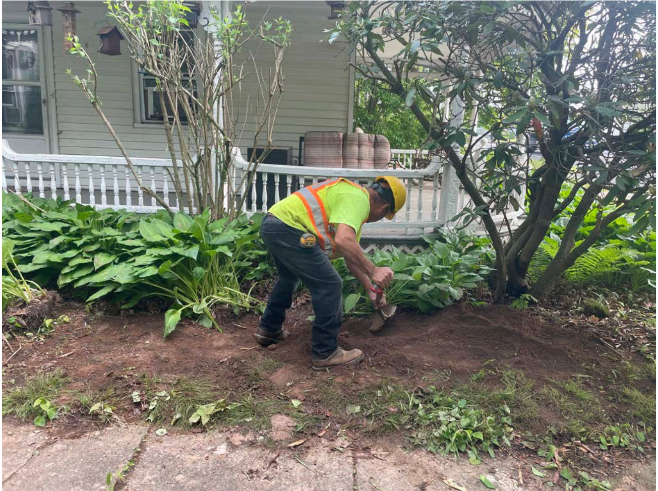
Picture 2: Ludlow backfilling the former location of the well at the 312 Main Street property that Grela decommissioned yesterday. View to the north.
