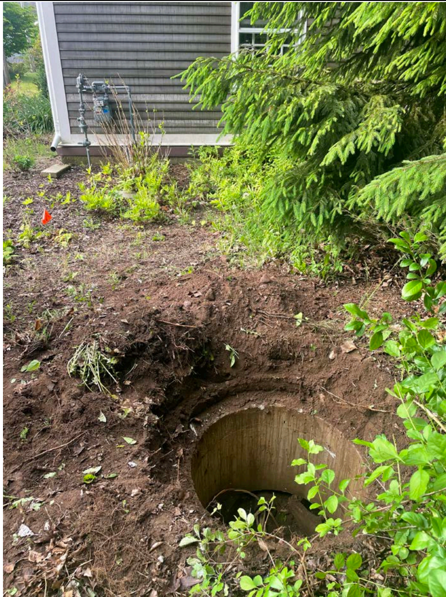
Picture 1: Well tile that Ludlow daylighted on the north side of the 308 Main Street residence to assist Grela in decommissioning the well located inside of it. View to the south.
