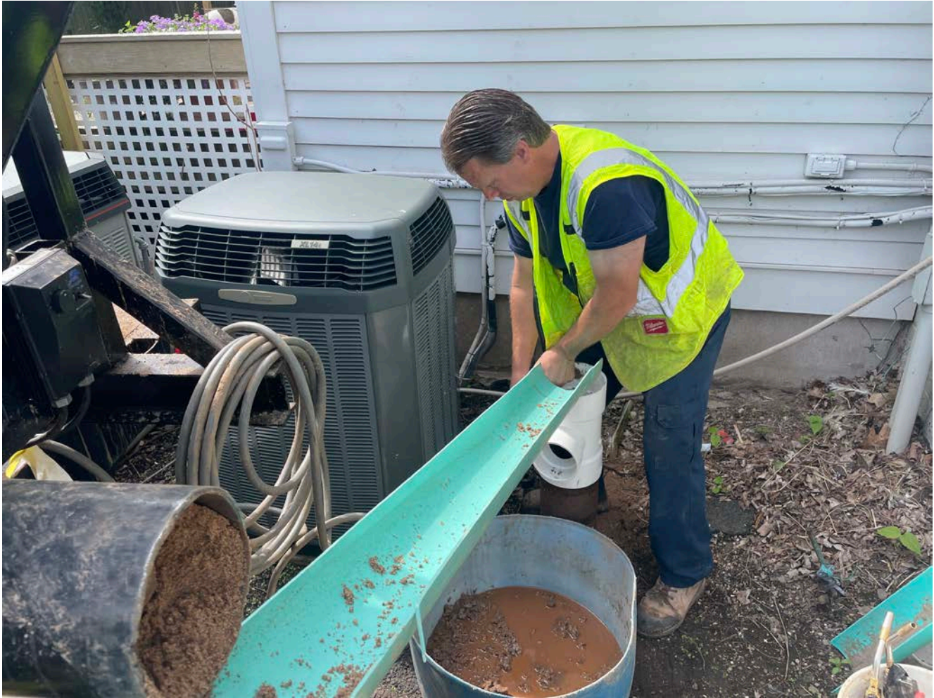
Picture 5: Grela placing sand into the well located on the north side of the 253 Main Street, Durham residence as part of well decommissioning activities. View to the south.
