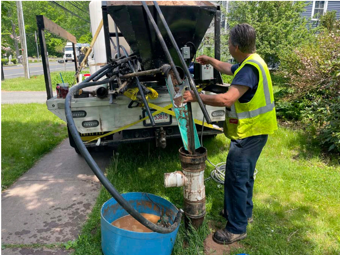
Picture 8: Grela placing sand into the well located on the west side of the 267 Main Street, Durham property as part of well decommissioning activities. View to the north.
