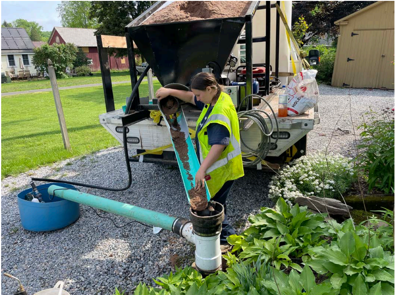
Picture 4: Grela placing sand into the well located on the north side of the 257 Main Street, Durham residence as part of well decommissioning activities. View to the northeast.
