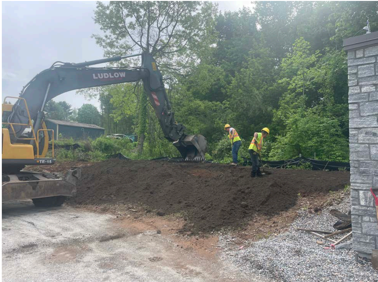
Picture 3: Ludlow placing and grading loam on the north side of the Water Meter Building located at Station 124+80 on S. Main Street, Middletown. View to the northeast.
