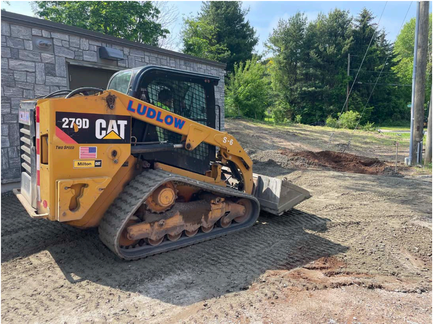
Picture 6: Ludlow grading fill on the driveway footprint located on the west side of the Water Meter Building located at Station 124+80 on S. Main Street in Middletown. View to the southeast.
