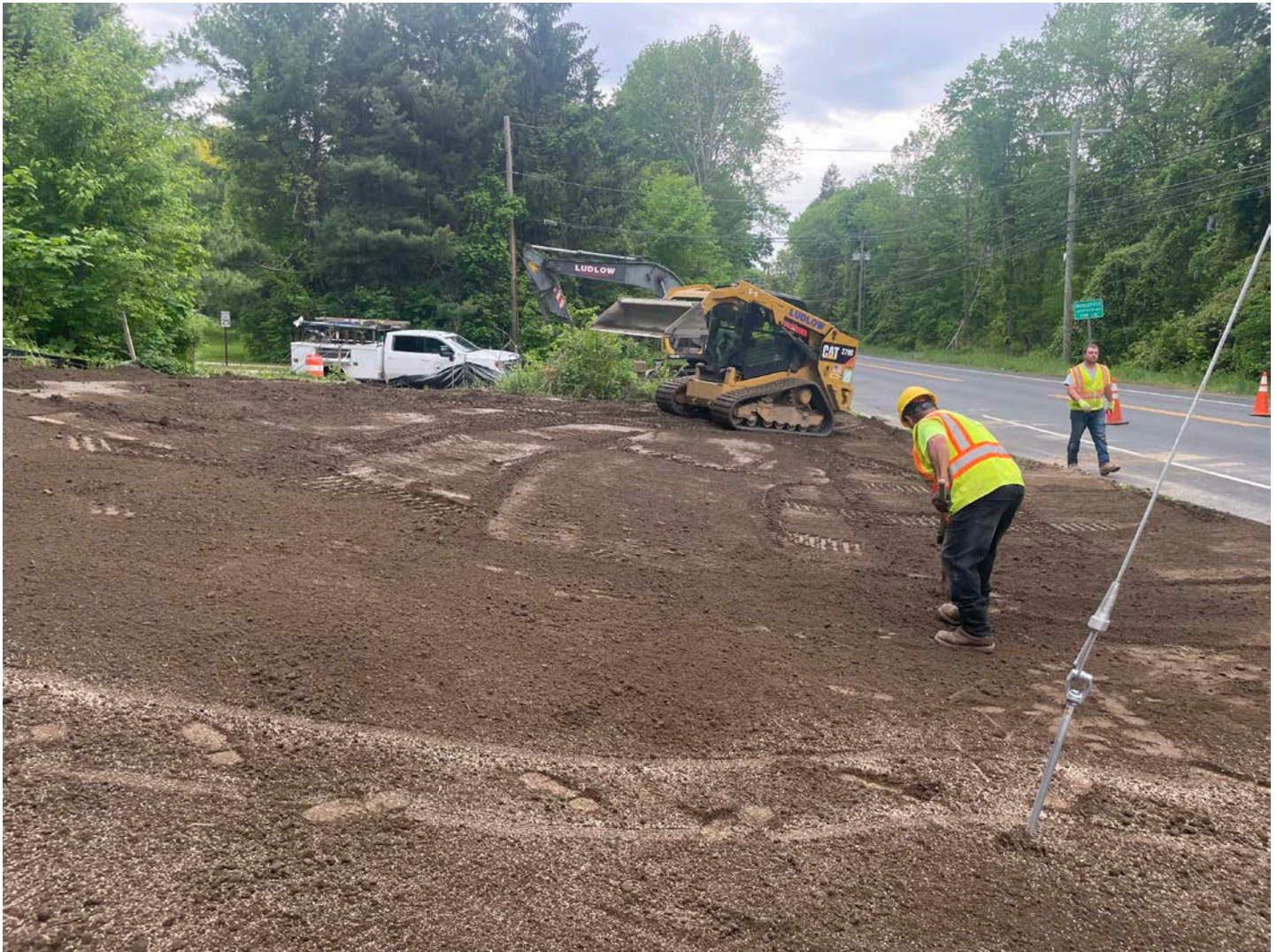
Picture 10: Ludlow raking and seeding the slope located on the south side of the Water Meter Building located at Station 124+80 on S. Main Street in Middletown. View to the south.
