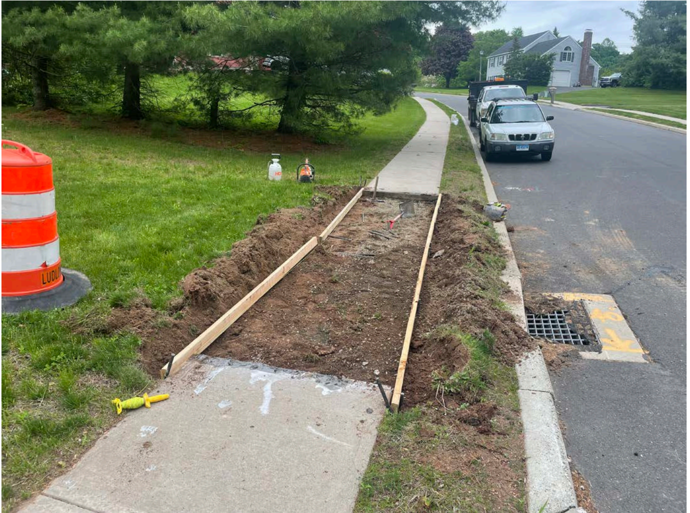
Picture 9: Section of sidewalk on the north side of Acorn Drive, Middletown at Station 125+92, where Ludlow has removed damaged panels of concrete and have built a form to pour new panels. View to the east.
