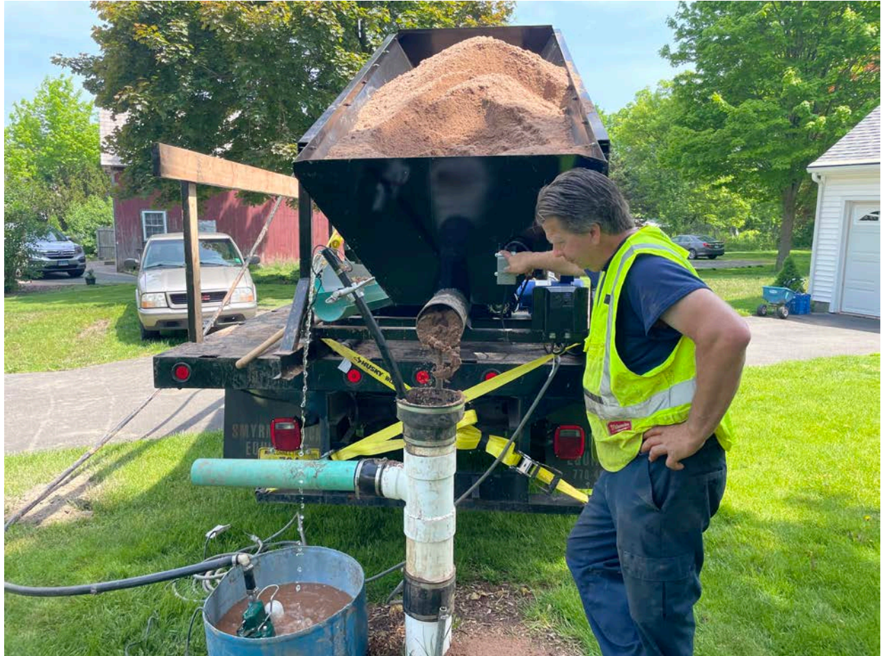
Picture 7: Grela placing sand into the well located on the west side of the 261 Main Street, Durham property as part of well decommissioning activities. View to the northeast.
