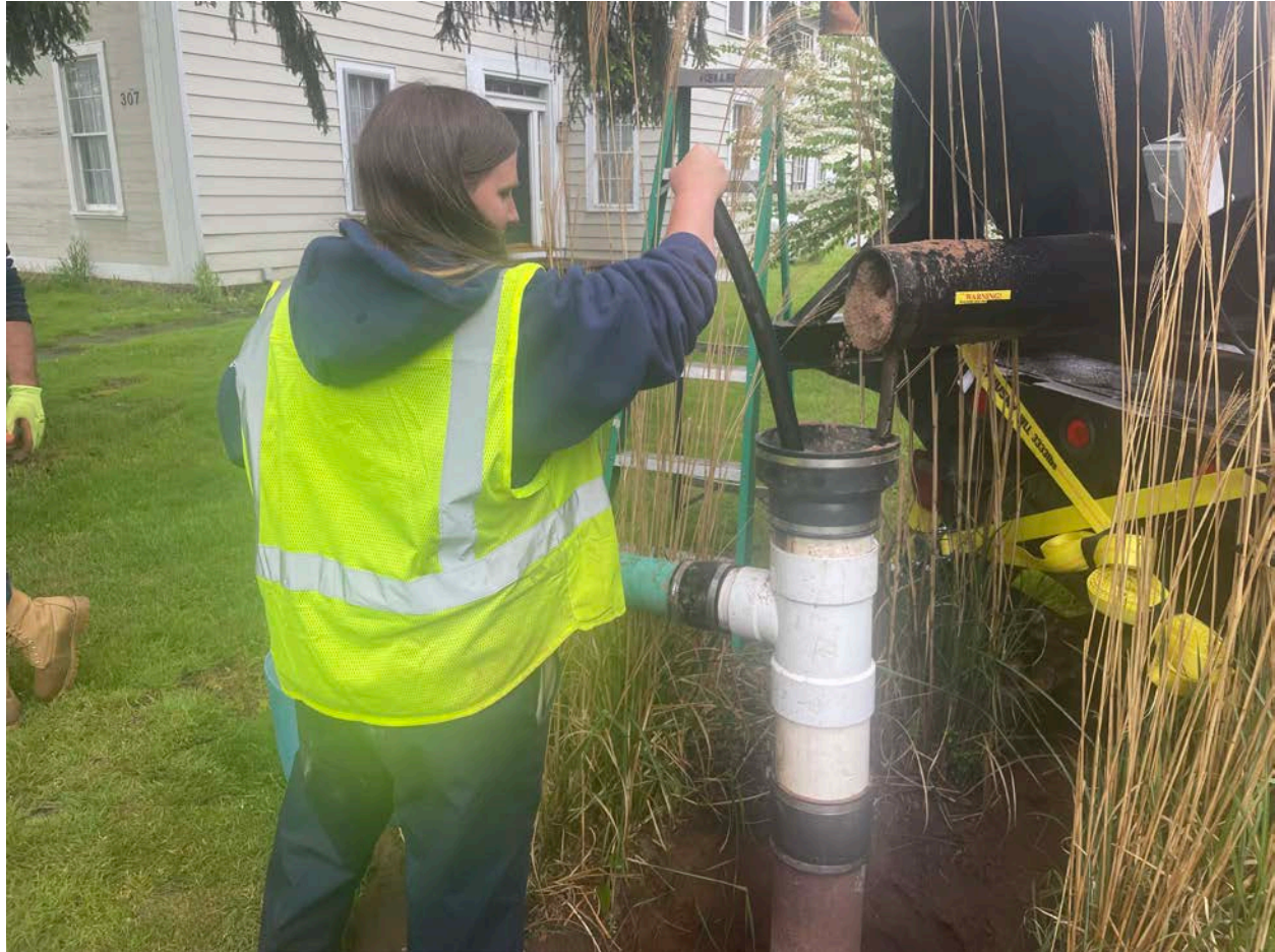
Picture 3: Grela placing sand into the well located on the southwest corner of the 307 Main Street, Durham property as part of well decommissioning activities. View to the northeast.
