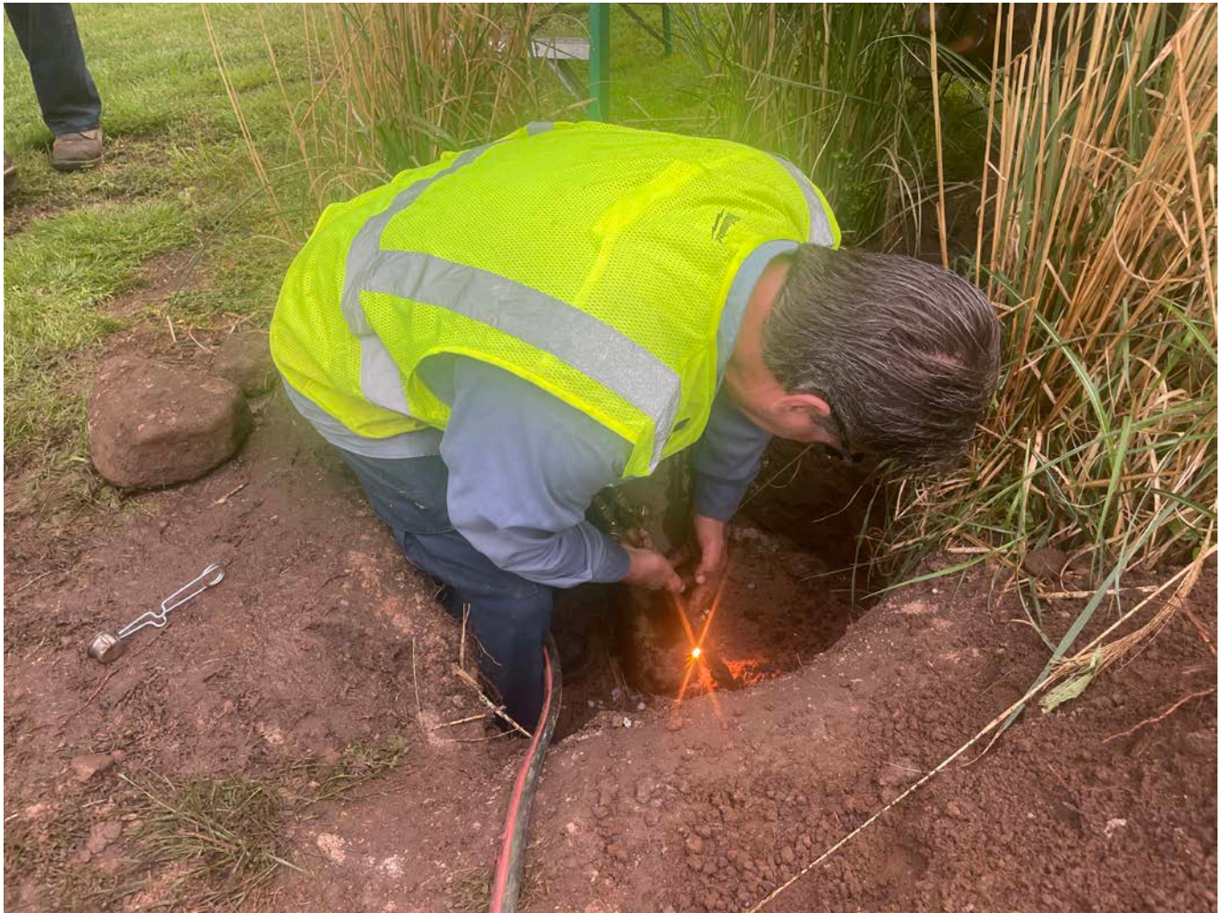
Picture 4: Grela using a torch to cut the steel casing of the well located on the 307 Main Street, Durham property as part of well decommissioning activities. View to the northeast.
