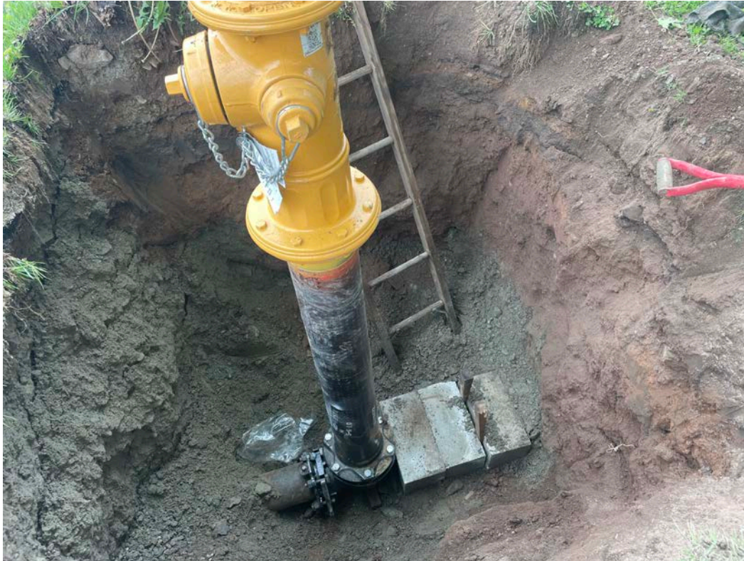
Picture 10: Three cinder blocks that Ludlow placed as thrust blocks on the west side of the hydrant stem at Station 174+91. View to the south.
