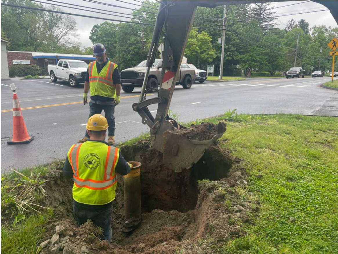
Picture 8: Ludlow excavating around the stem of a damaged hydrant located at Station 174+91 that they are in the process of replacing. View to the southeast.
