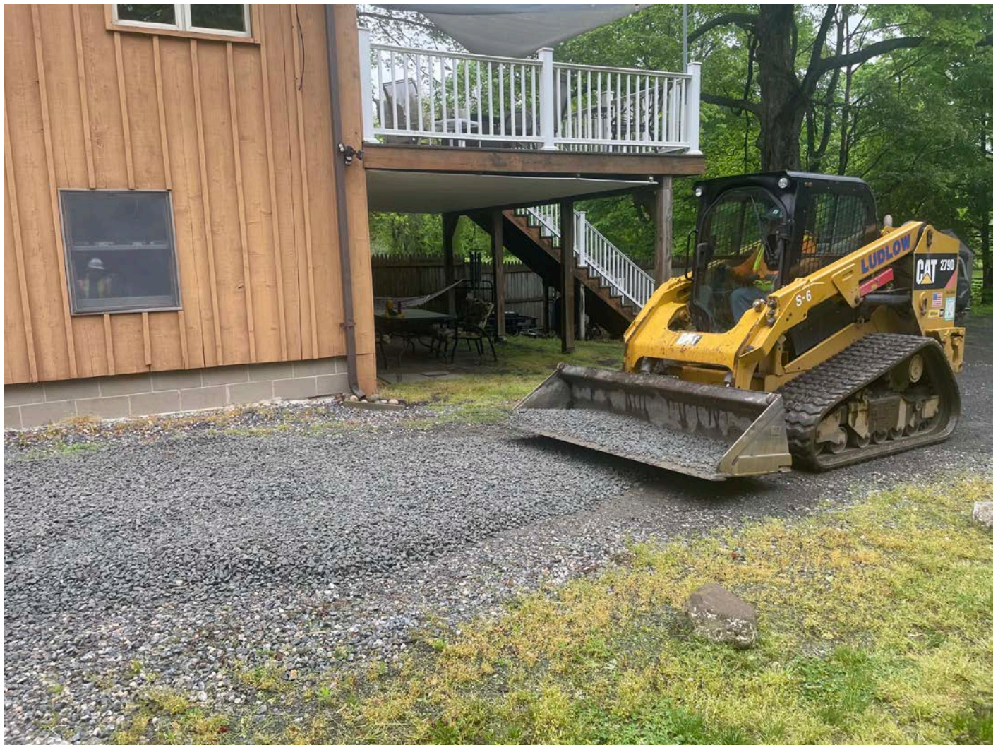
Picture 6: Ludlow grading \frac{3}{4} " gravel they placed on the south side of the 305 Main Street, Durham, residence as they work to restore the driveway. View to the northeast.
