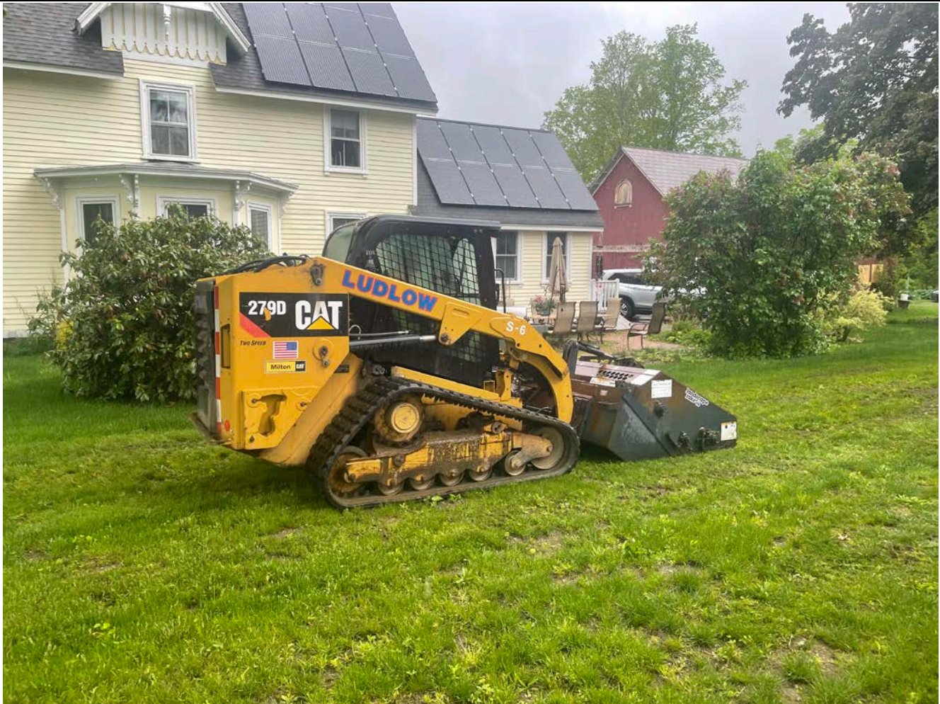
Picture 1: Ludlow using a CAT 279D to run a Harley Rake across the portion of the lawn at the 261 Main Street property where they plan to perform lawn restoration activities in Durham. View to the northeast.
