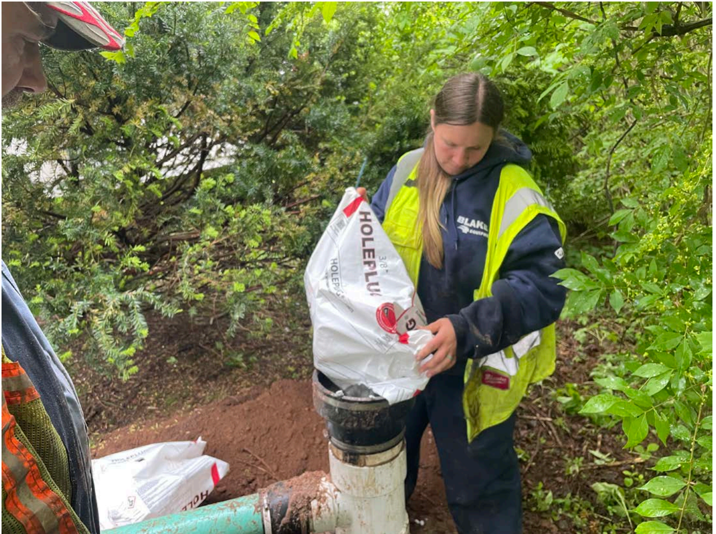
Picture 13: Grela placing bentonite chips into the well located on the north side of the 316 Main Street residence as part of well decommissioning activities. View to the west.
