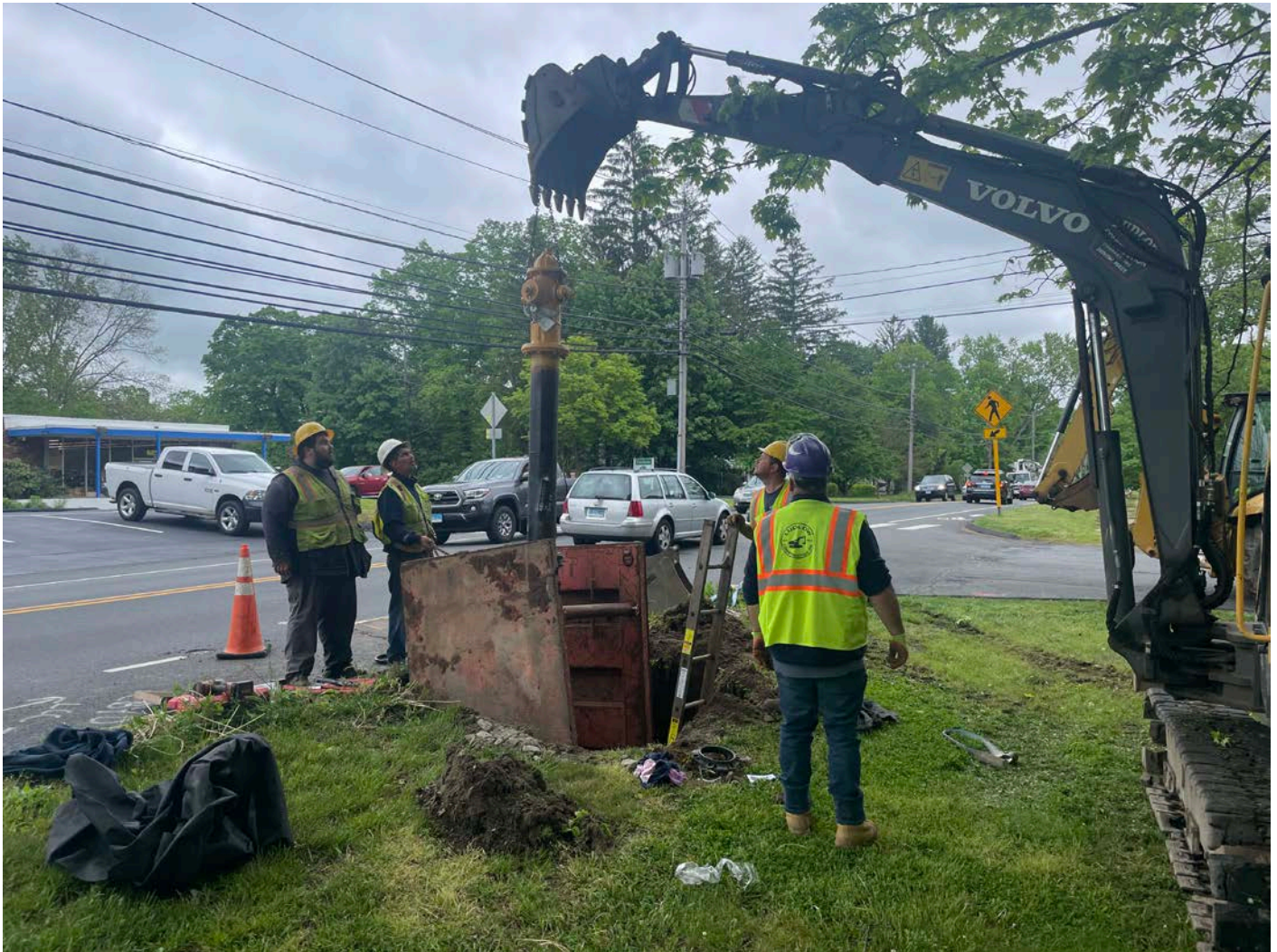
Picture 9: Ludlow placing a new hydrant at Station 174+91. View to the southeast.
