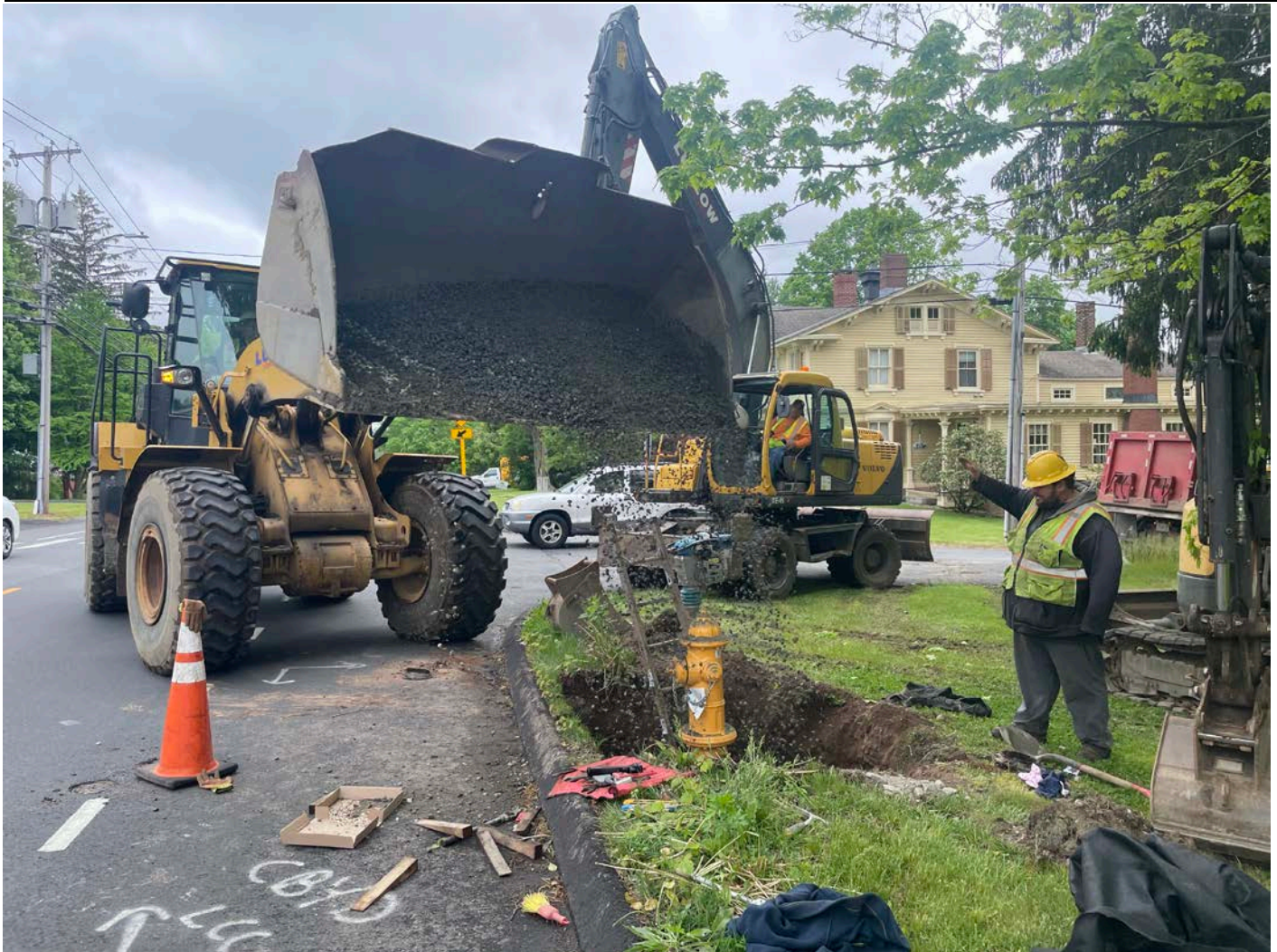
Picture 11: Ludlow backfilling around the new hydrant they installed at Station 174+91. View to the south.
