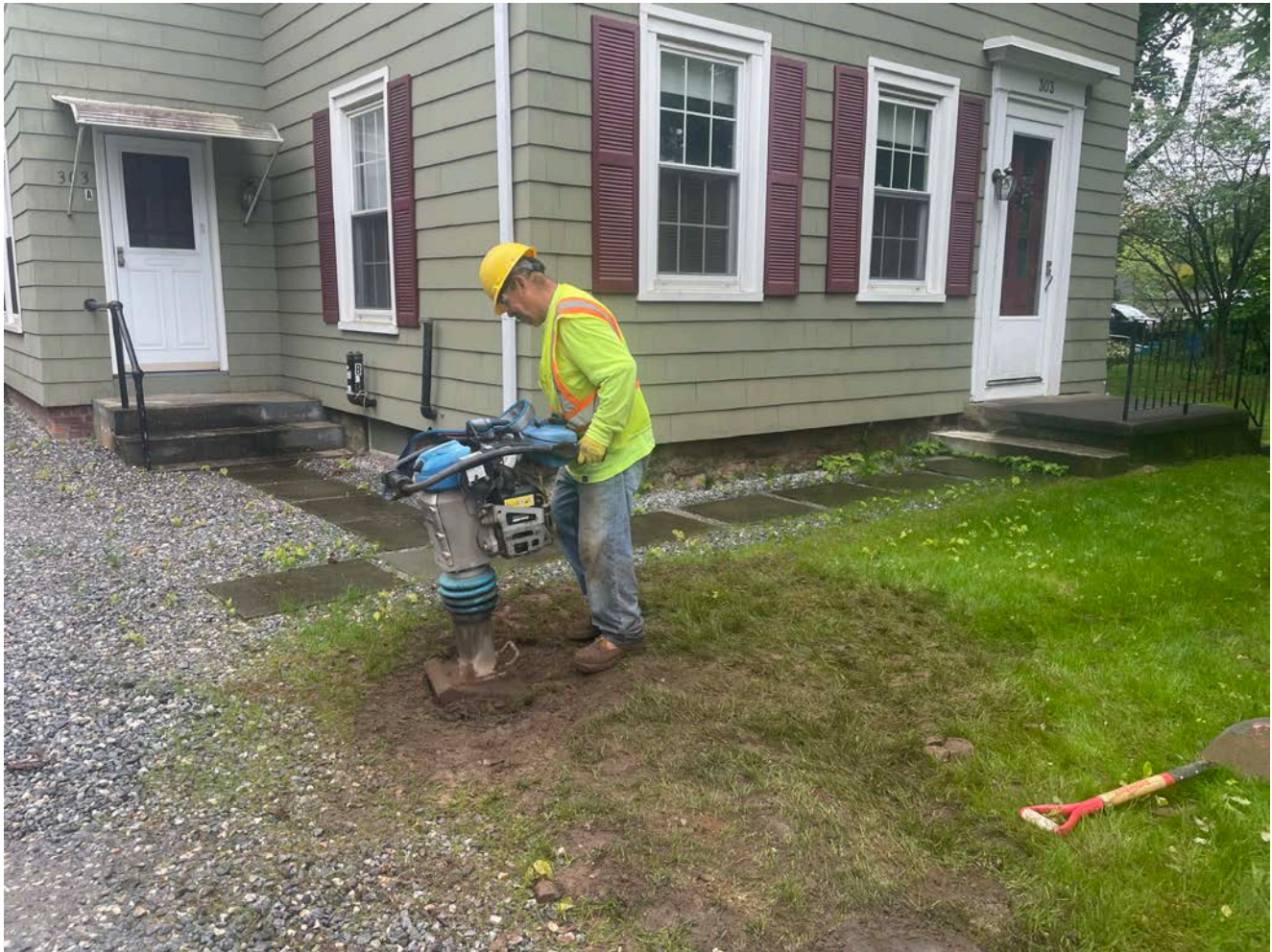
Picture 2: Ludlow compacting fill where the backfilled the location of the well for the 305 Main Street residence that Grela decommissioned yesterday. View to the southeast.
