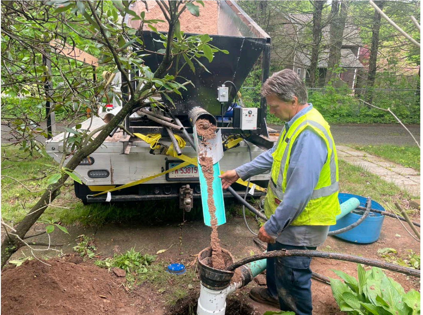
Picture 12: Grela placing sand into the well located on the north side of the 312 Main Street residence as part of well decommissioning activities. View to the south.
