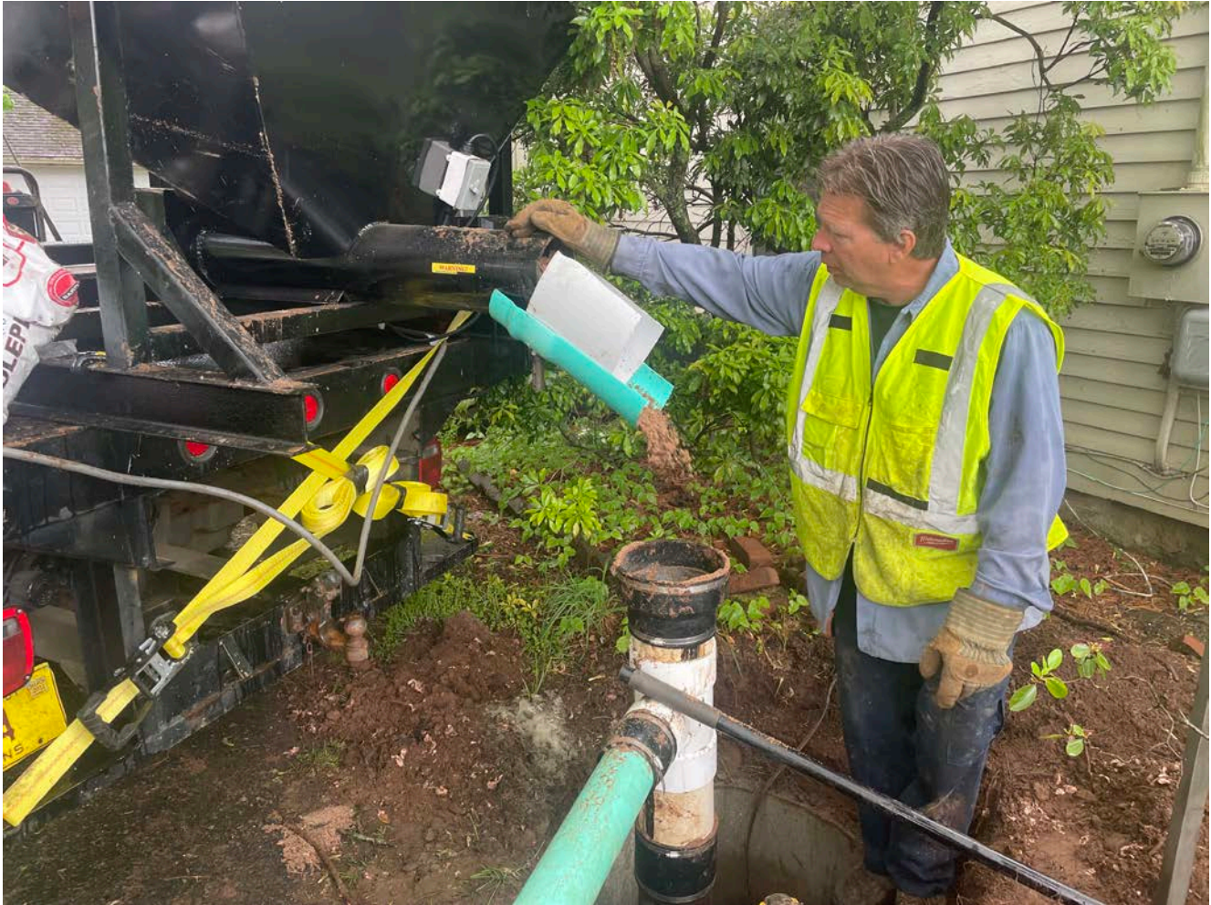
Picture 5: Grela placing sand into the well located on the northwest corner of the 297 Main Street residence as they work to decommission the well. View to the southeast.
