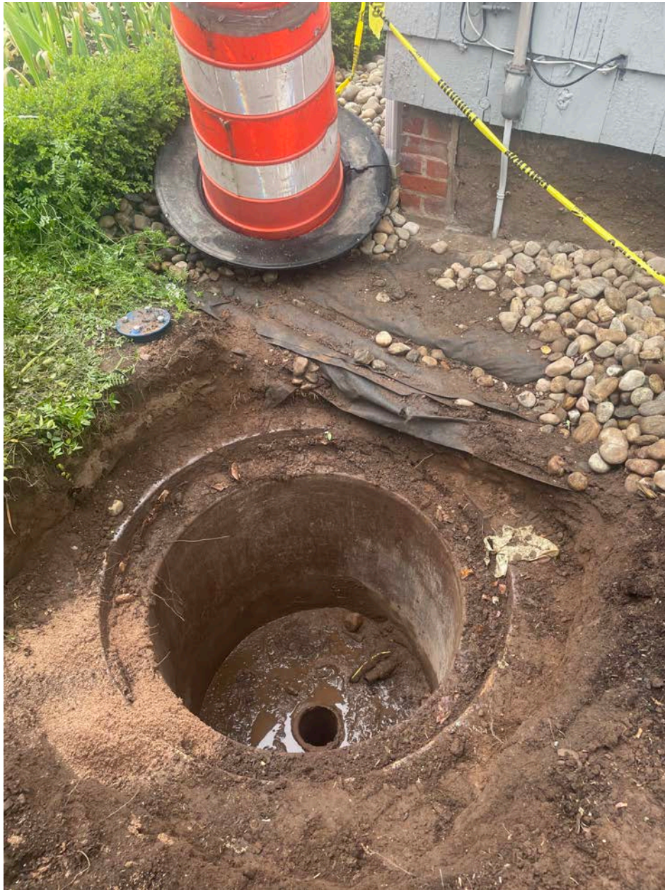
Picture 7: View of the well located on the southwest corner of the 297 Main Street property that Grela is in the process of decommissioning. View to the northwest.
