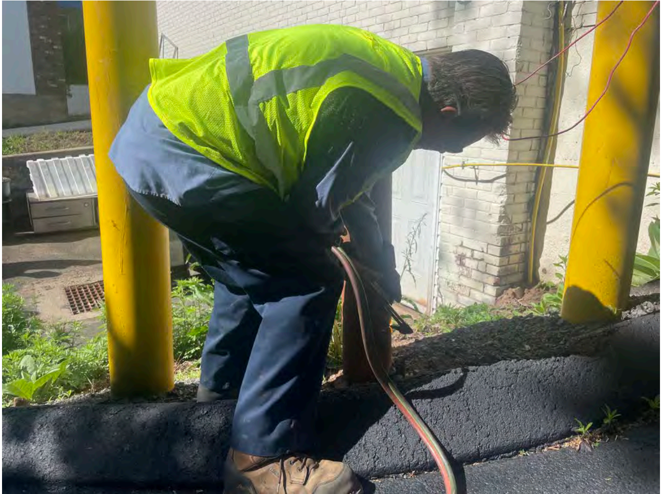
Picture 7: Grela using a torch to cut the 6" steel riser for the well located at the 325 Main Street property. Grela will return to cut the casing 2' below surface grade once Ludlow has removed the top two feet of soil from around the casing. View to the southwest.
