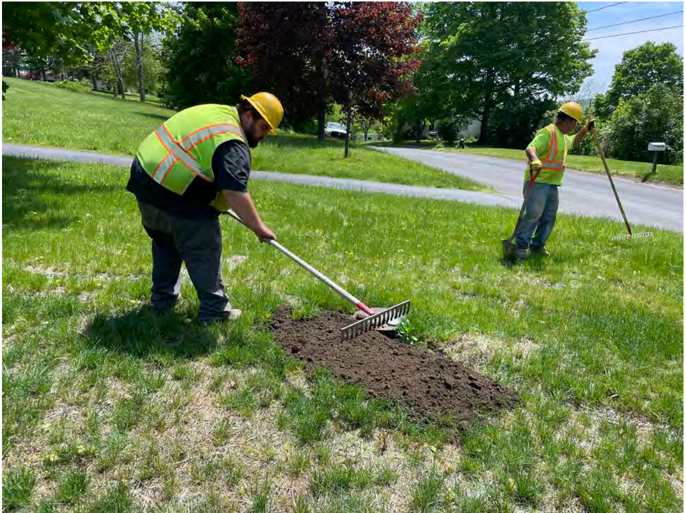
Picture 4: Ludlow placing loam and grass seed as they restore a portion of the lawn at the 119 Maple Avenue property that was disturbed last year during the installation of a copper water service line. View to the south.
