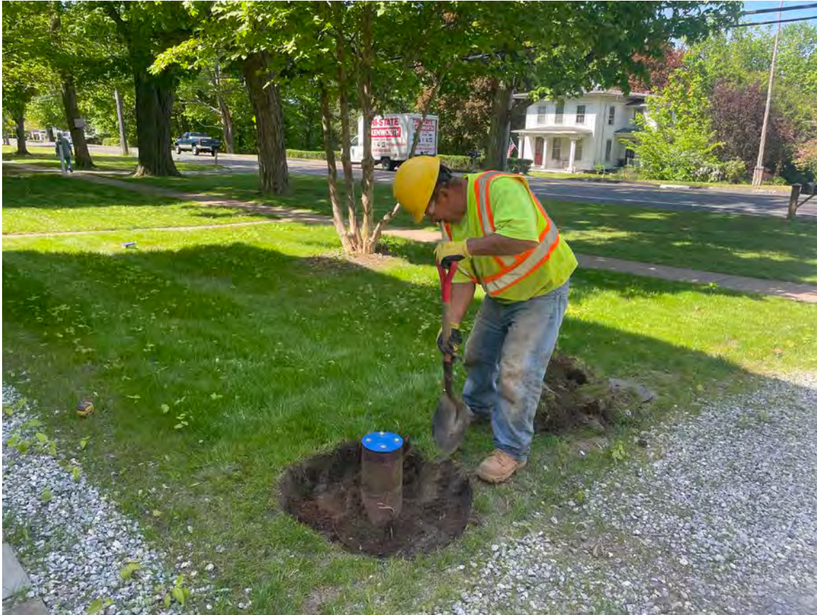
Picture 8: Ludlow hand-excavating around the casing of the well that services the 305 Main Street, Durham, residence. Ludlow is removing soil to 2' below surface grade. View to the southwest.
