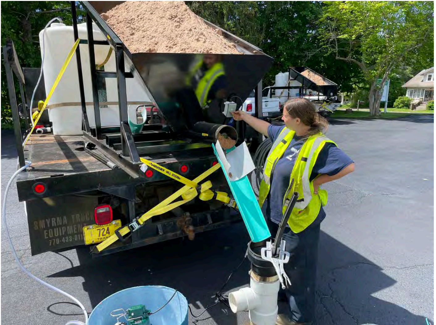
Picture 9: Ludlow placing sand into the well located on the south side of the 321 Main Street, Durham, building as part of well decommissioning activities. View to the southwest.
