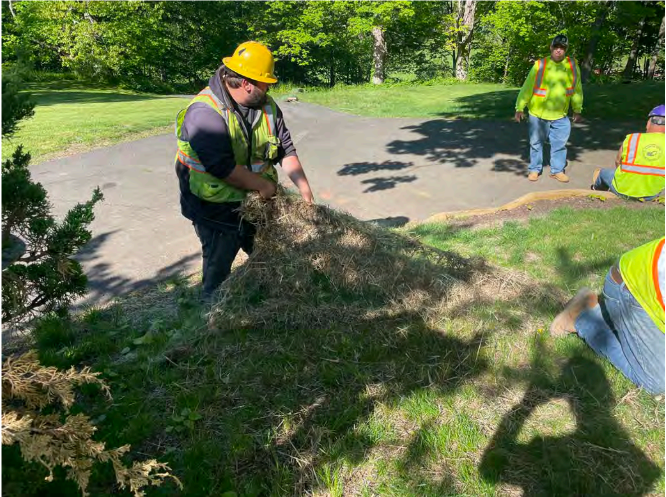
Picture 1: Ludlow removing erosion control blankets from the 95R Maple Avenue property in Durham. View to the west.
