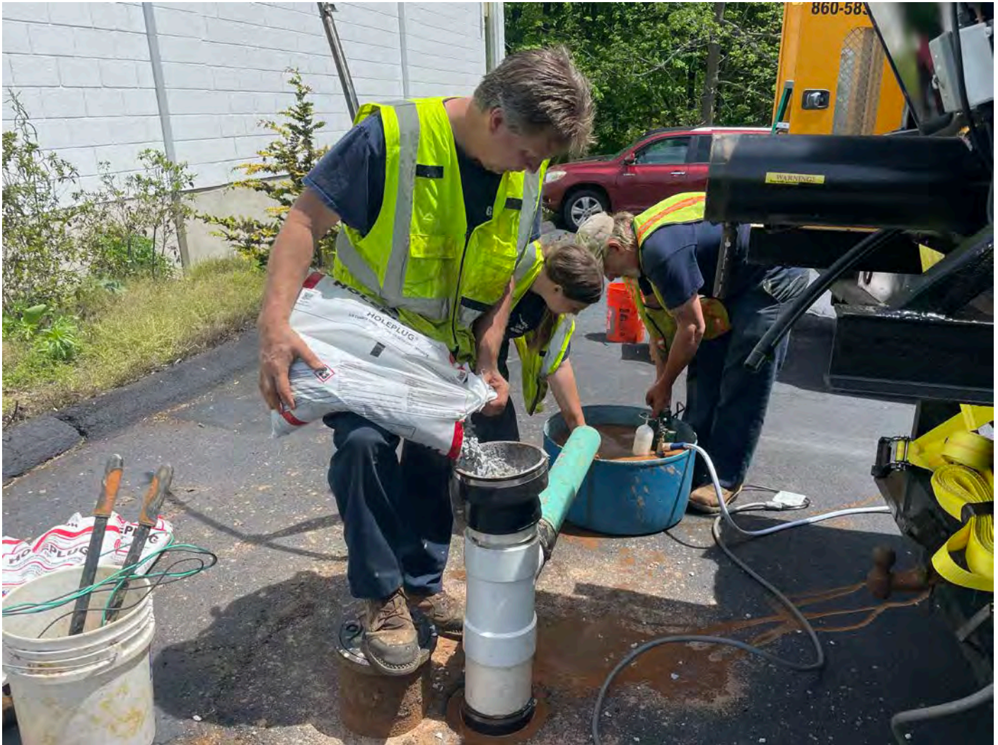
Picture 11: Ludlow placing bentonite chips into the well located on the south side of the 321 Main Street, Durham, building as part of well decommissioning activities. View to the east.
