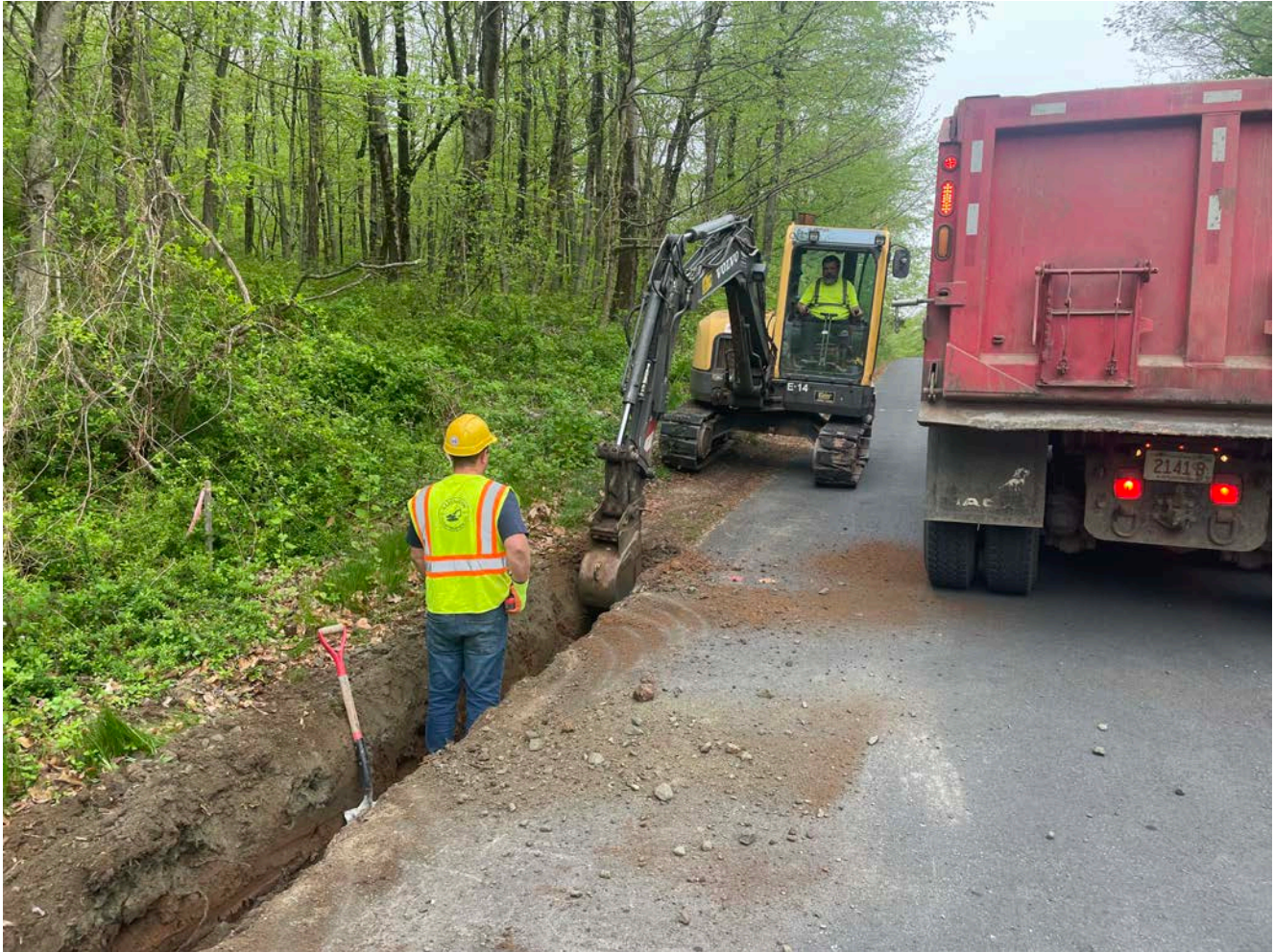
Picture 1: Ludlow excavating soil along the south edge of the Shared Access Driveway in Middletown where they are constructing a drain comprised of \frac{3}{4} " stone and 4" black, plastic, corrugated drain line. View to the southwest.
