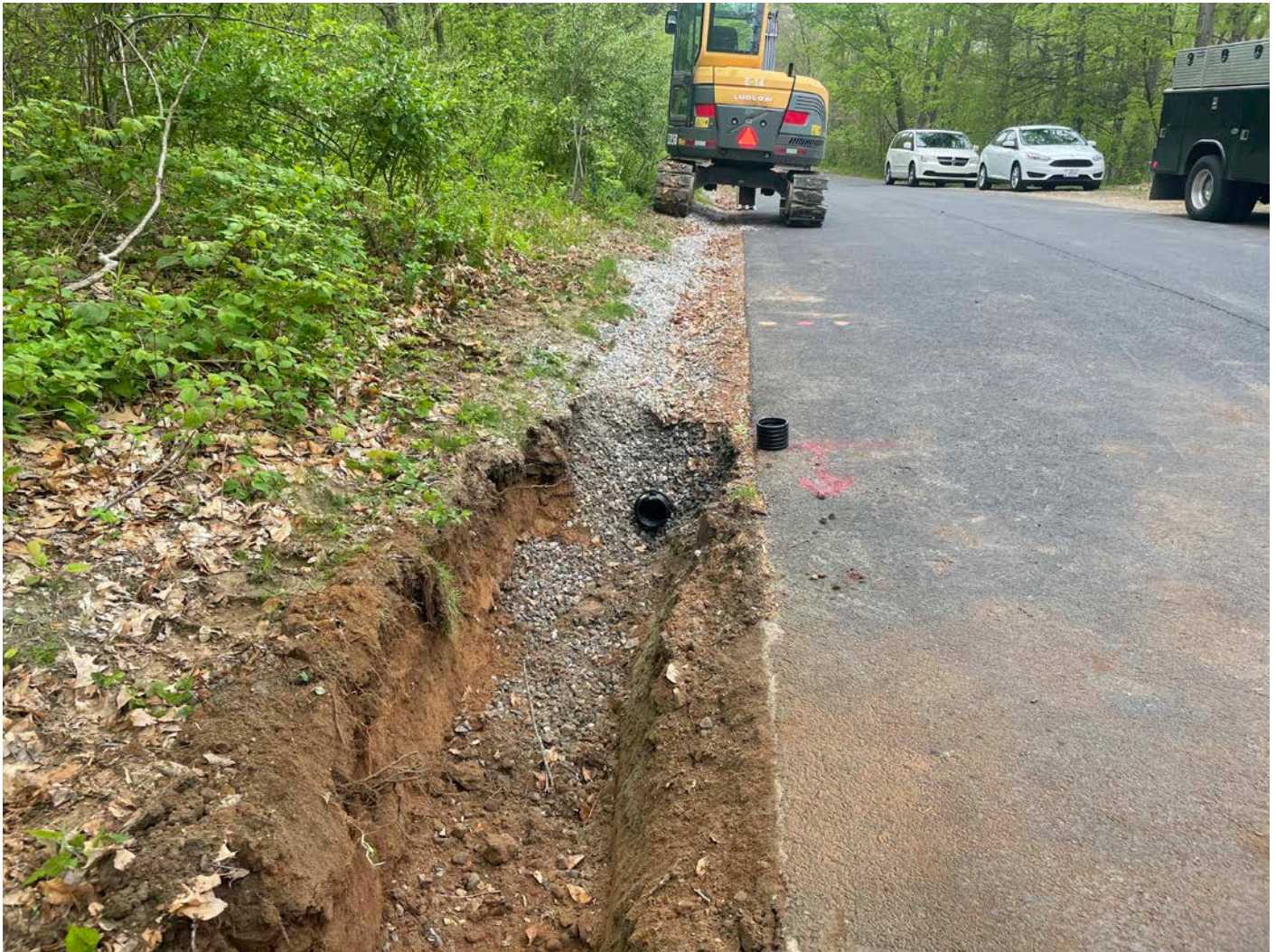
Picture 6: Previously installed 4" drain line at Station 17+90 that Ludlow daylighted in order to tie into it with the 4" drain line they are installing today. View to the west.
