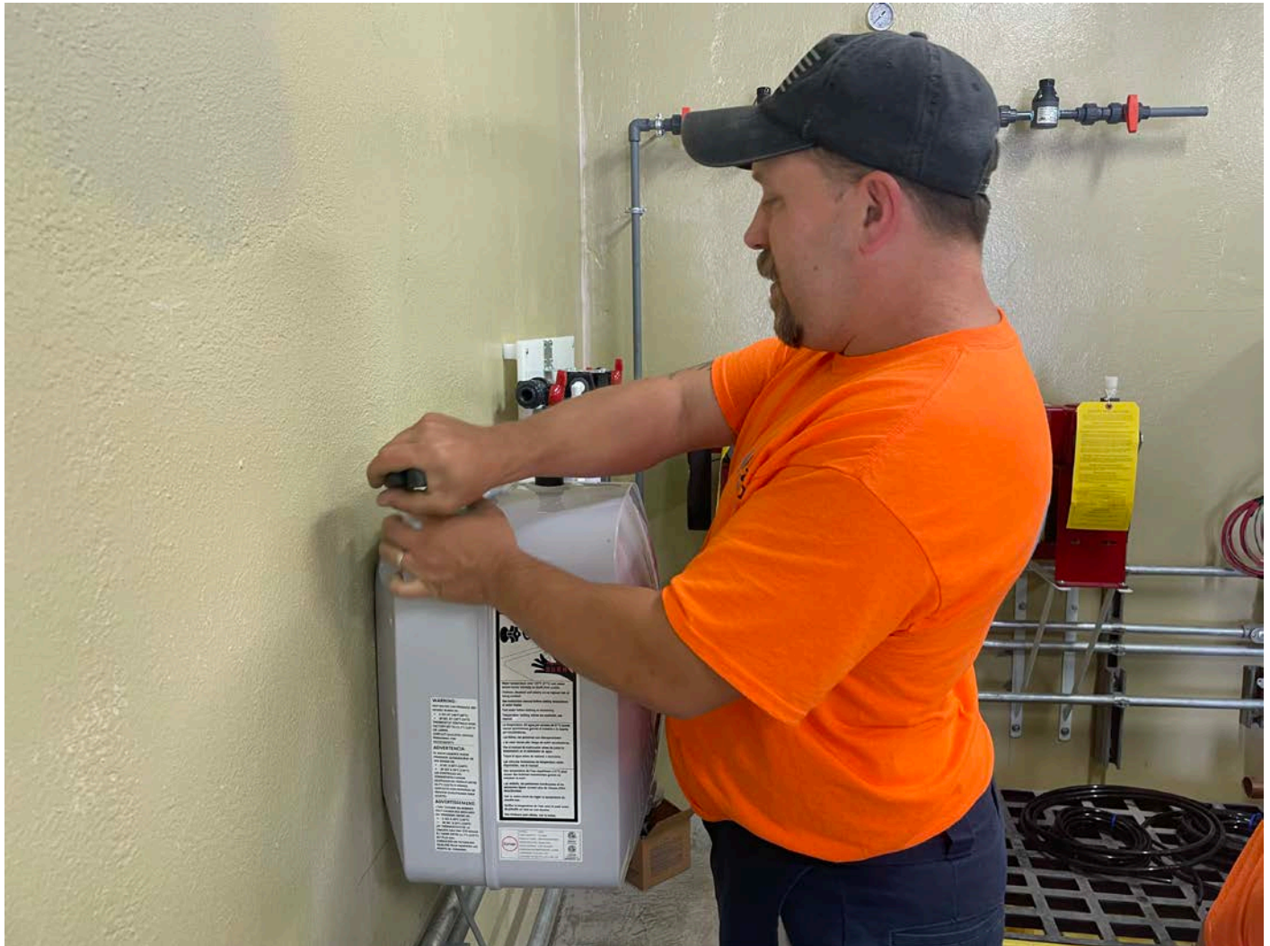
Picture 9: Fazzino Plumbing working on the chlorination system that is being installed at the southeast corner of the Long Hill Pump Station in Middletown.
