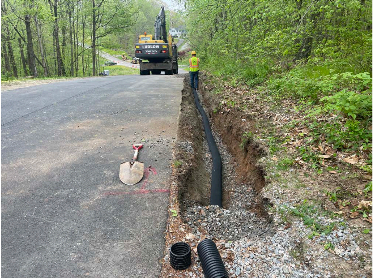
Picture 7: Station 17+90, looking east after Ludlow tied the 4" drain line they installed today into the 4" drain line that was previously installed between Stations 17+90 and 18+15 on the south side of the Shared Access Driveway.
