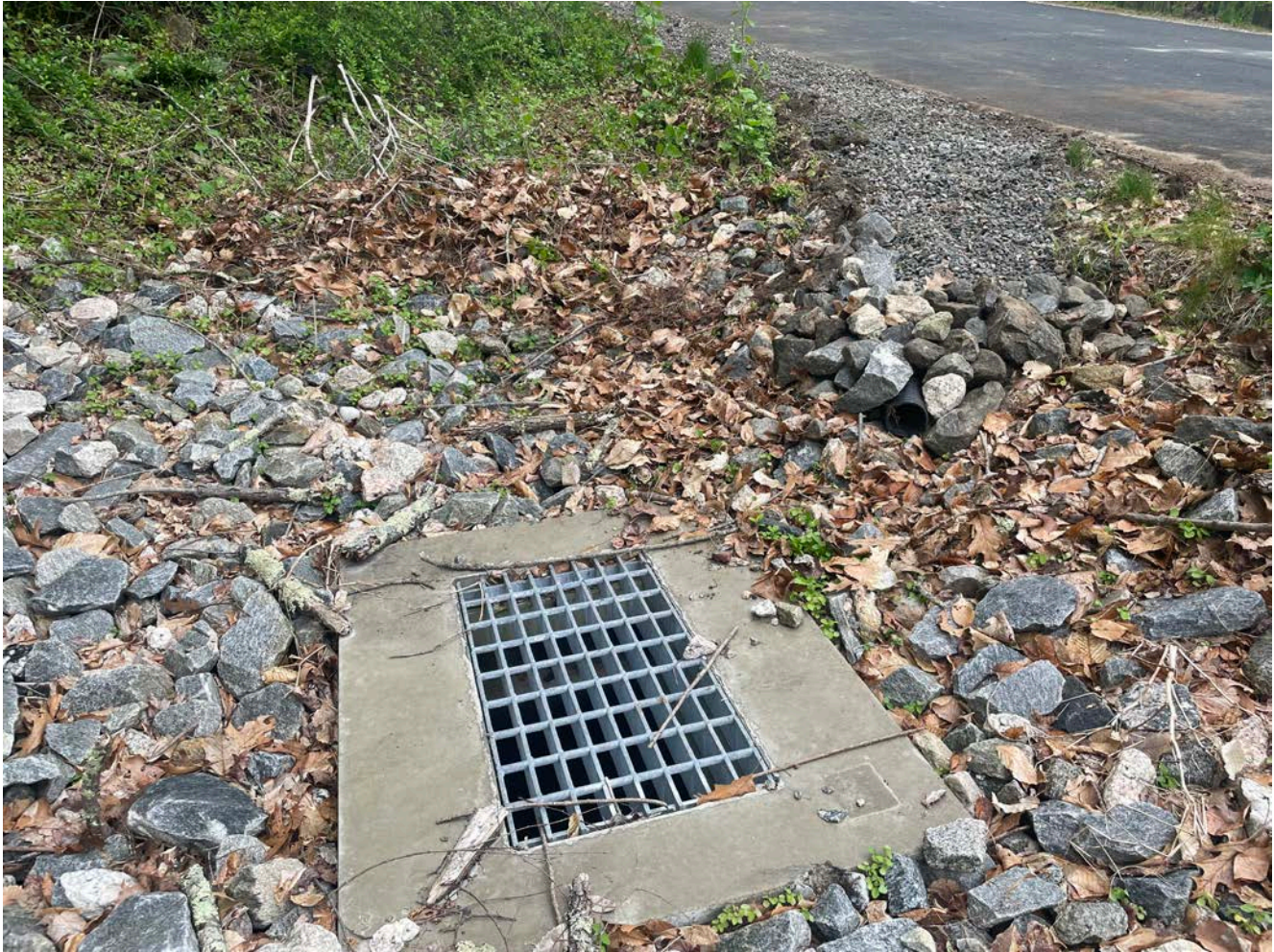
Picture 5: Finished drain line installation at Station 15+90, looking northwest.
