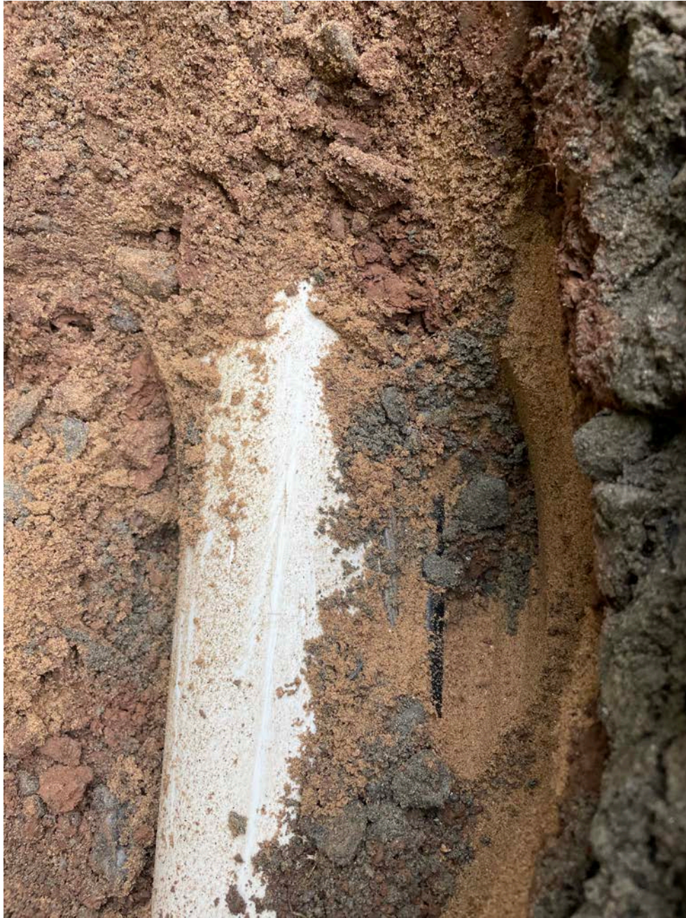
Picture 8: White 4" PVC conduit and several other unshielded utilities located on the right-hand side of the PVC that Ludlow daylighted while hand-excavating on the south edge of the Shared Access Driveway.
