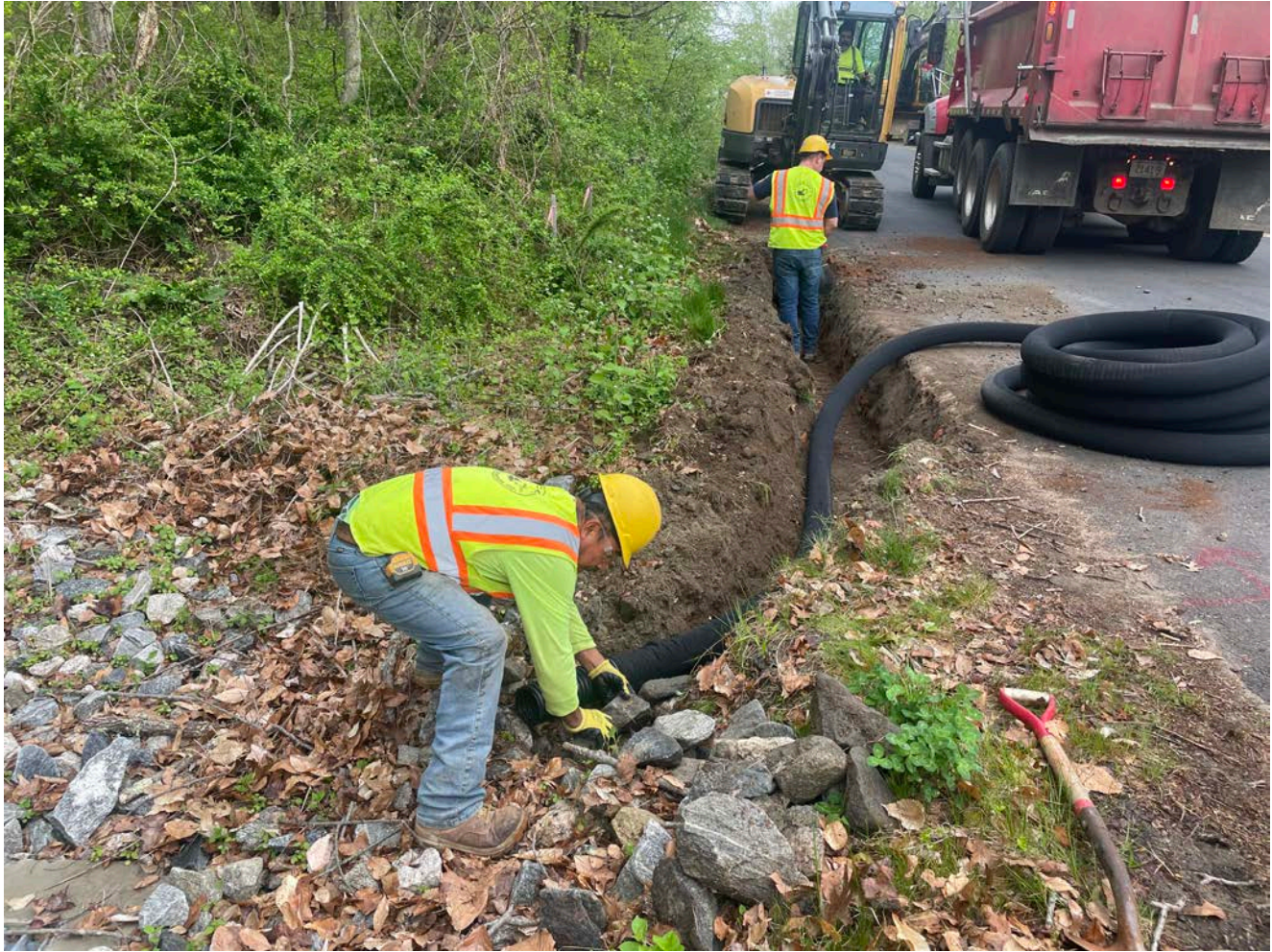
Picture 2: Ludlow installing a 4" black, plastic, corrugated drain line at Station 15+90. View to the west.
