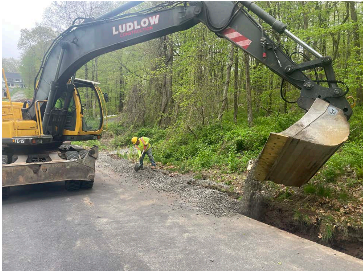
Picture 3: Ludlow placing \frac{3}{4} " stone over 4" black, plastic, corrugated drain line along the south edge of the Shared Access Driveway in Middletown. View to the southeast.
