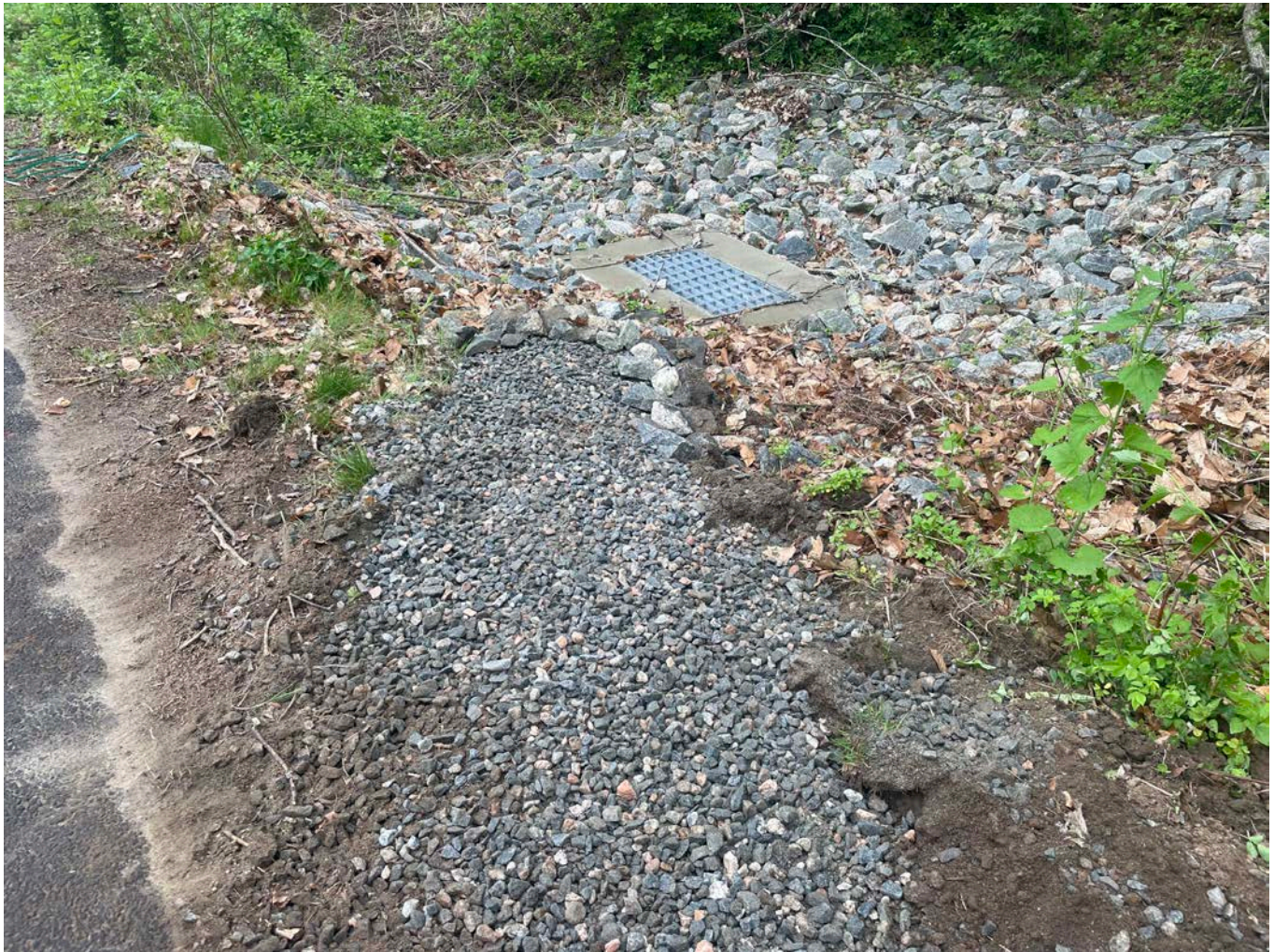
Picture 4: Finished drain line installation at Station 15+90, looking southeast towards the plunge bowl.
