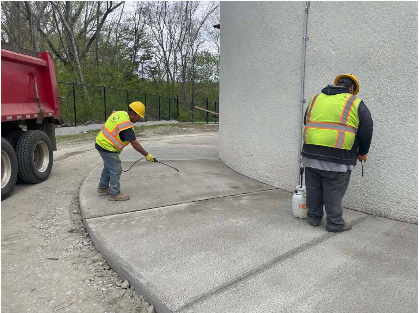
Picture 6: Ludlow applying Cure Shield X sealant on the concrete that was placed yesterday around the perimeter of the water tank located east of the Shared Access Driveway in Middletown.
