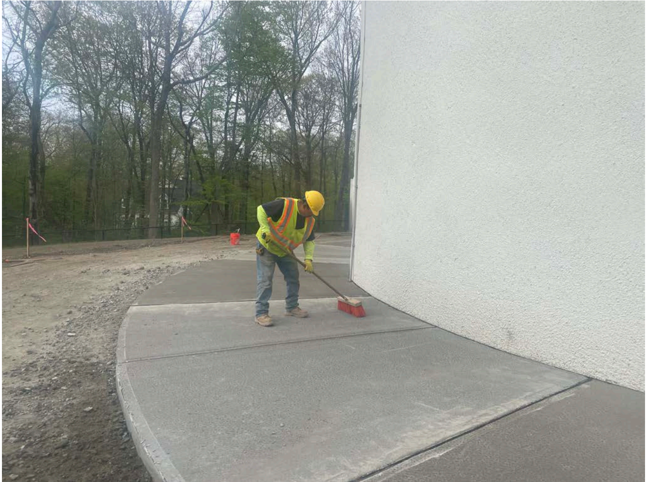
Picture 2: Ludlow sweeping the concrete sidewalk they constructed around the perimeter of the water tank located east of the Shared Access Driveway in Middletown. View to the southwest.
