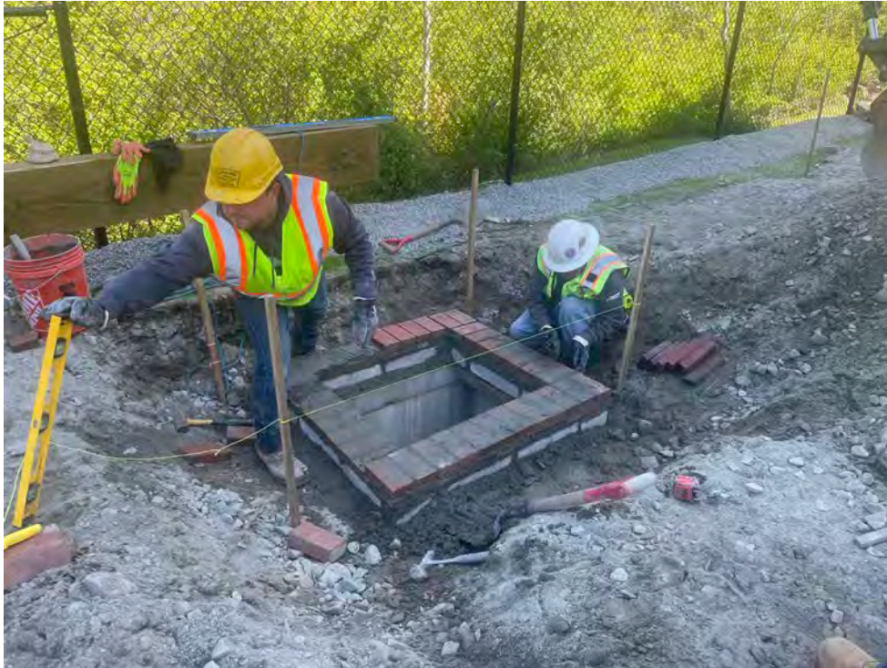
Picture 4: Ludlow using bricks, cinder blocks, and mortar to raise the elevation of the catch basin located on the north side of the Shared Access Driveway at Station 10+40. View to the northeast.
