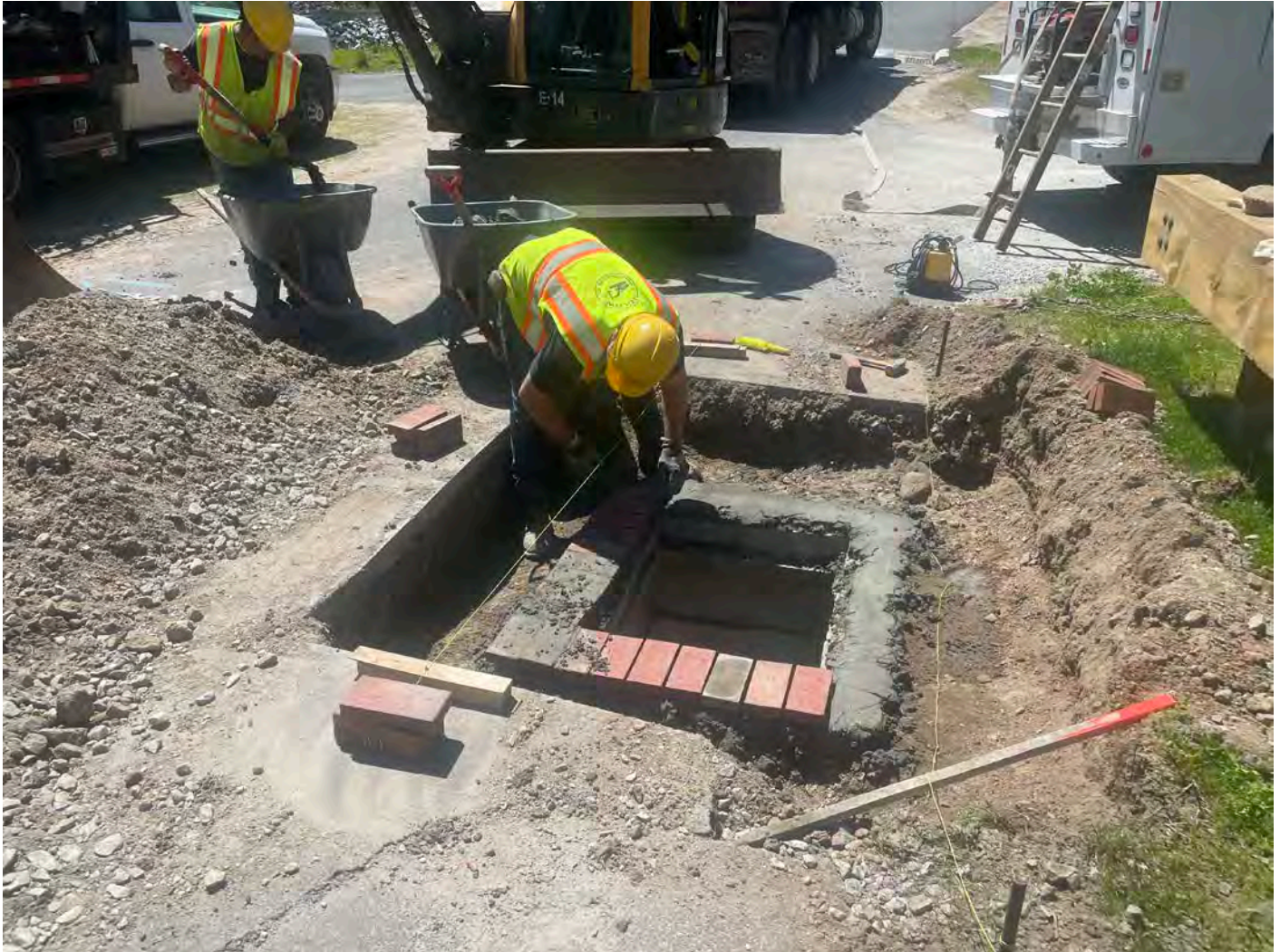
Picture 10: Ludlow placing mortar and bricks to raise the elevation of the catch basin located at Station 13+70 on the Shared Access Driveway in Middletown. View to the west.
