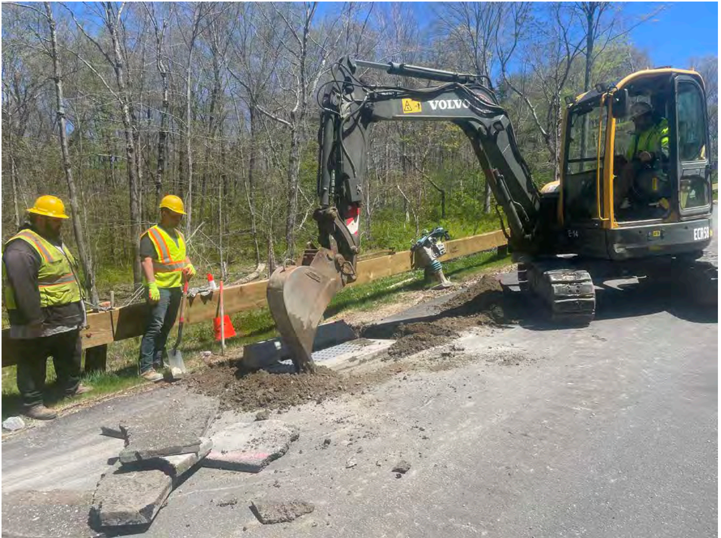
Picture 6: Ludlow excavating around the catch basin located at Station 13+00 on the north side of the Shared Access Driveway in Middletown. View to the northeast.
