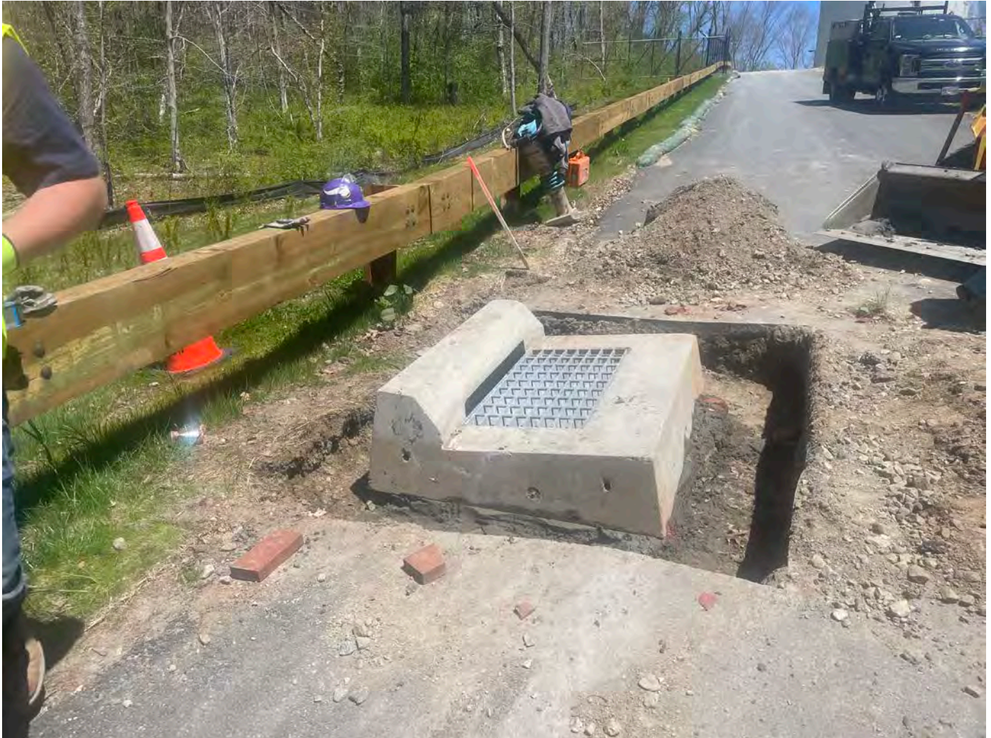
Picture 8: The catch basin located at Station 13+00 on the Shared Access Driveway after Ludlow raised its elevation by 1.75". View to the east.
