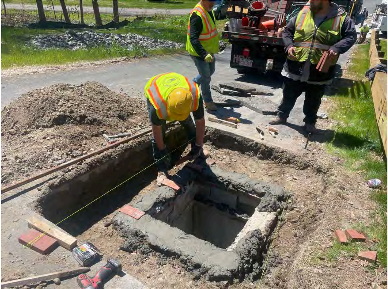
Picture 7: Ludlow placing mortar and bricks to raise the elevation of the catch basin located at Station 13+00 on the Shared Access Driveway in Middletown. View to the west.
