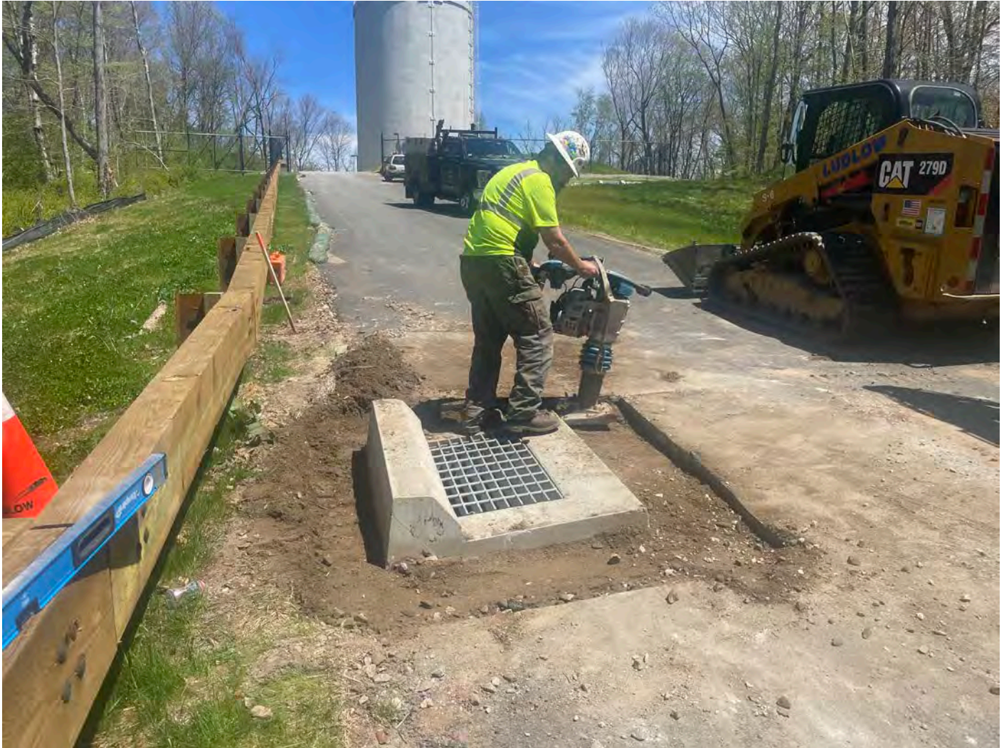
Picture 9: Ludlow using a jumping jack to compact the backfill that was placed around the catch basin located at Station 13+00 on the Shared Access Driveway in Middletown. Ludlow raised the catch basin 1.75". View to the east.
