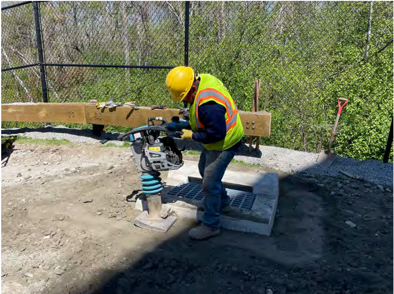
Picture 5: Ludlow compacting the backfill that was placed around the catch basin located at Station 10+40 after it was raised up 8". View to the north.
