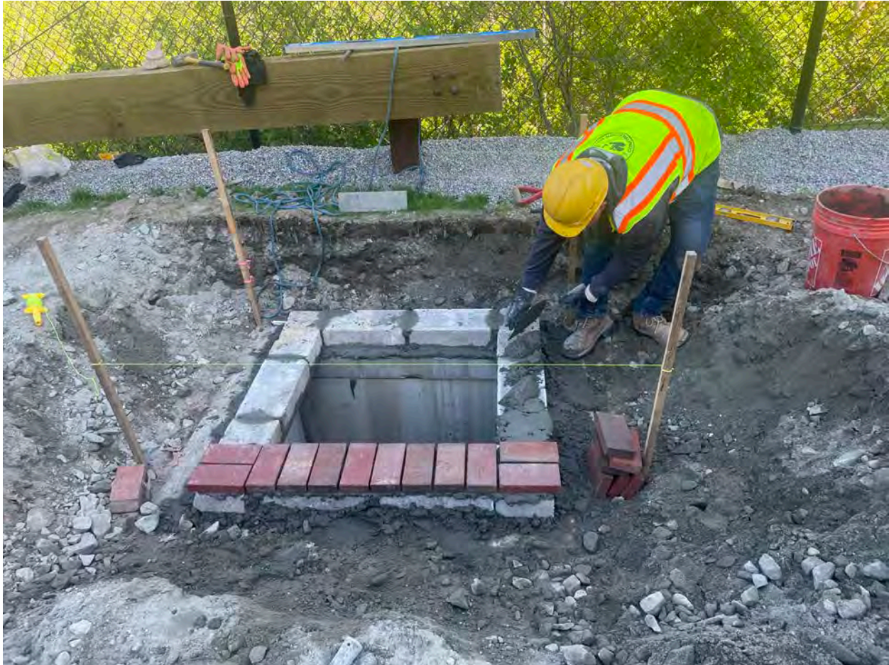
Picture 3: Ludlow using bricks, cinder blocks, and mortar to raise the elevation of the catch basin located on the north side of the Shared Access Driveway at Station 10+40. View to the north.
