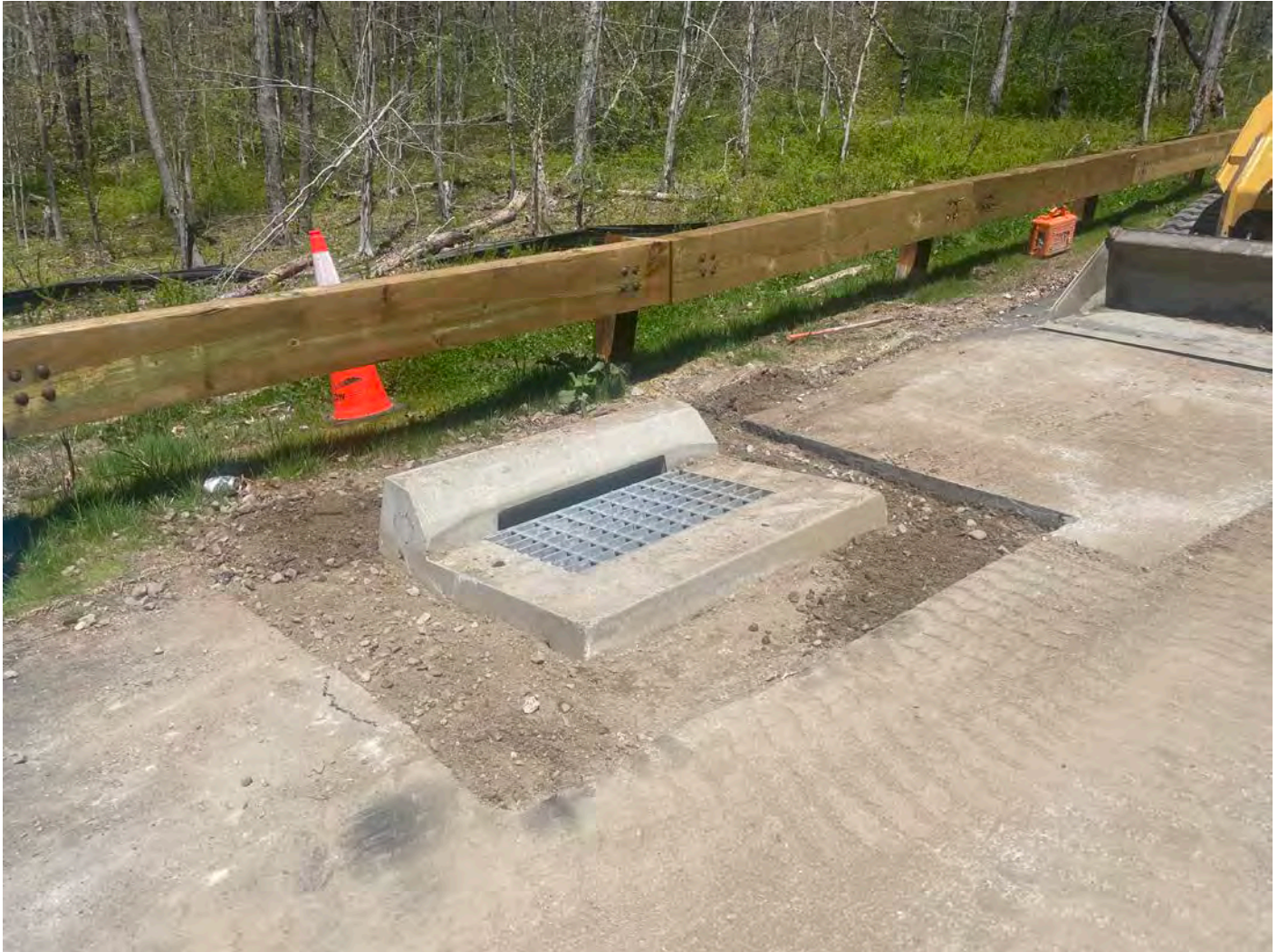
Picture 12: View of a catch basin located at Station 13+70 after Ludlow raised it by 1.75" and compacted the backfill that was placed around it. View to the northeast.
