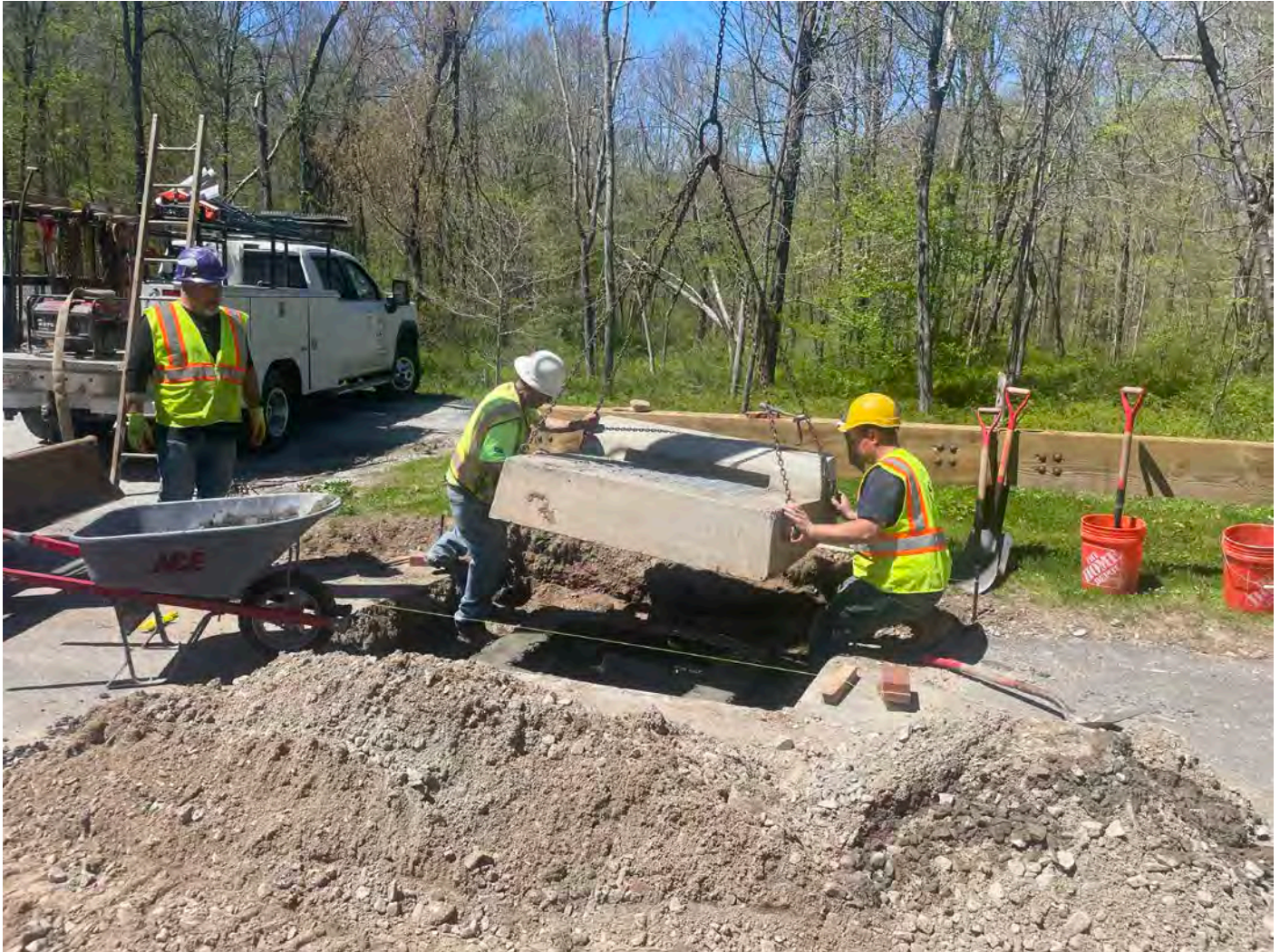
Picture 11: Ludlow placing the catch basin located at Station 13+70 back into place after Ludlow raised it by 1.75". View to the north.
