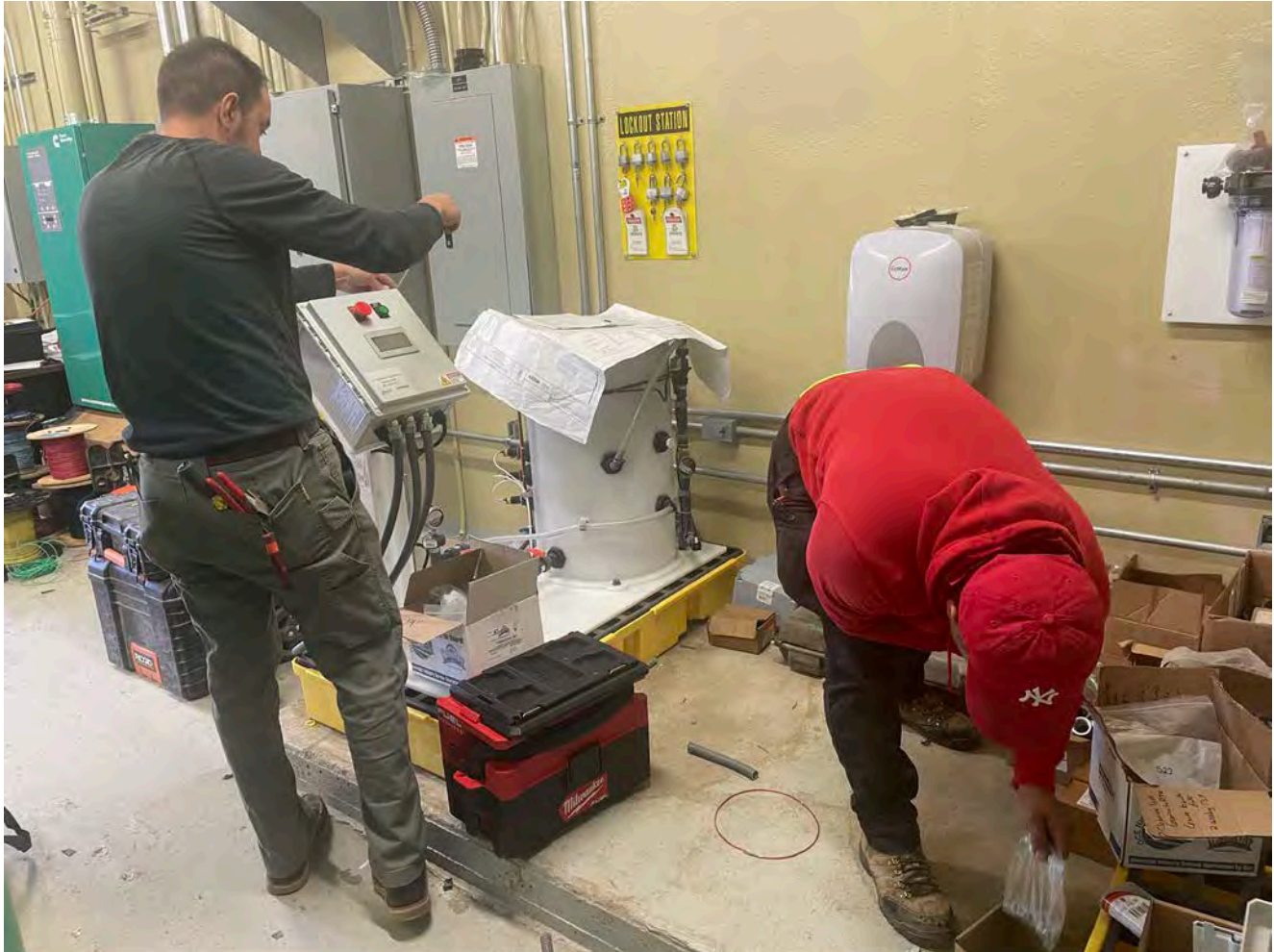
Picture 2: A&R Electrical continuing the installation of wiring at the Long Hill pump station in Middletown that is associated with the new chlorination system. View to the northeast.
