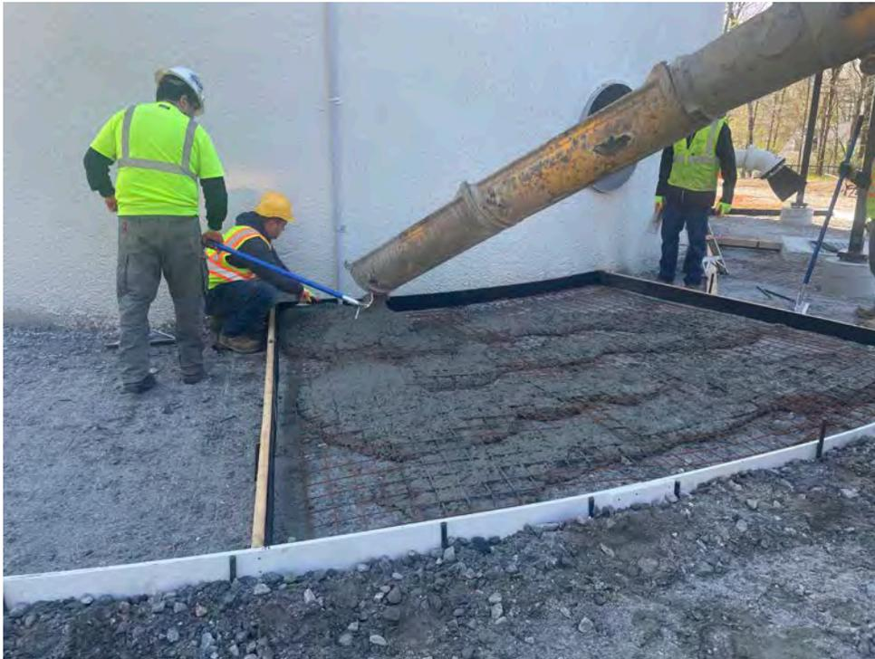
**Picture 4: Ludlow and Farmington Ready-Mix placing concrete in one of the sidewalk form panels on the west side of the water tank located east of the Shared Access Driveway in Middletown. Note the sheet of 4"x4" steel mesh located between 2 lifts of the 4000 PSI mix they are pouring. View to the east.**
