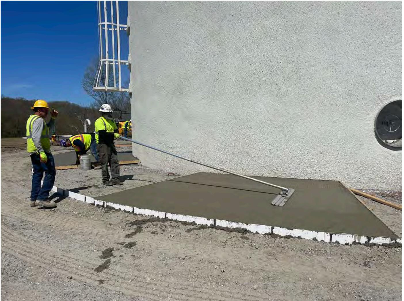
**Picture 8: Ludlow using a bull float to smooth the top of the 4000 PSI mix that was just poured on the southeast side of the water tank. View to the west.**
