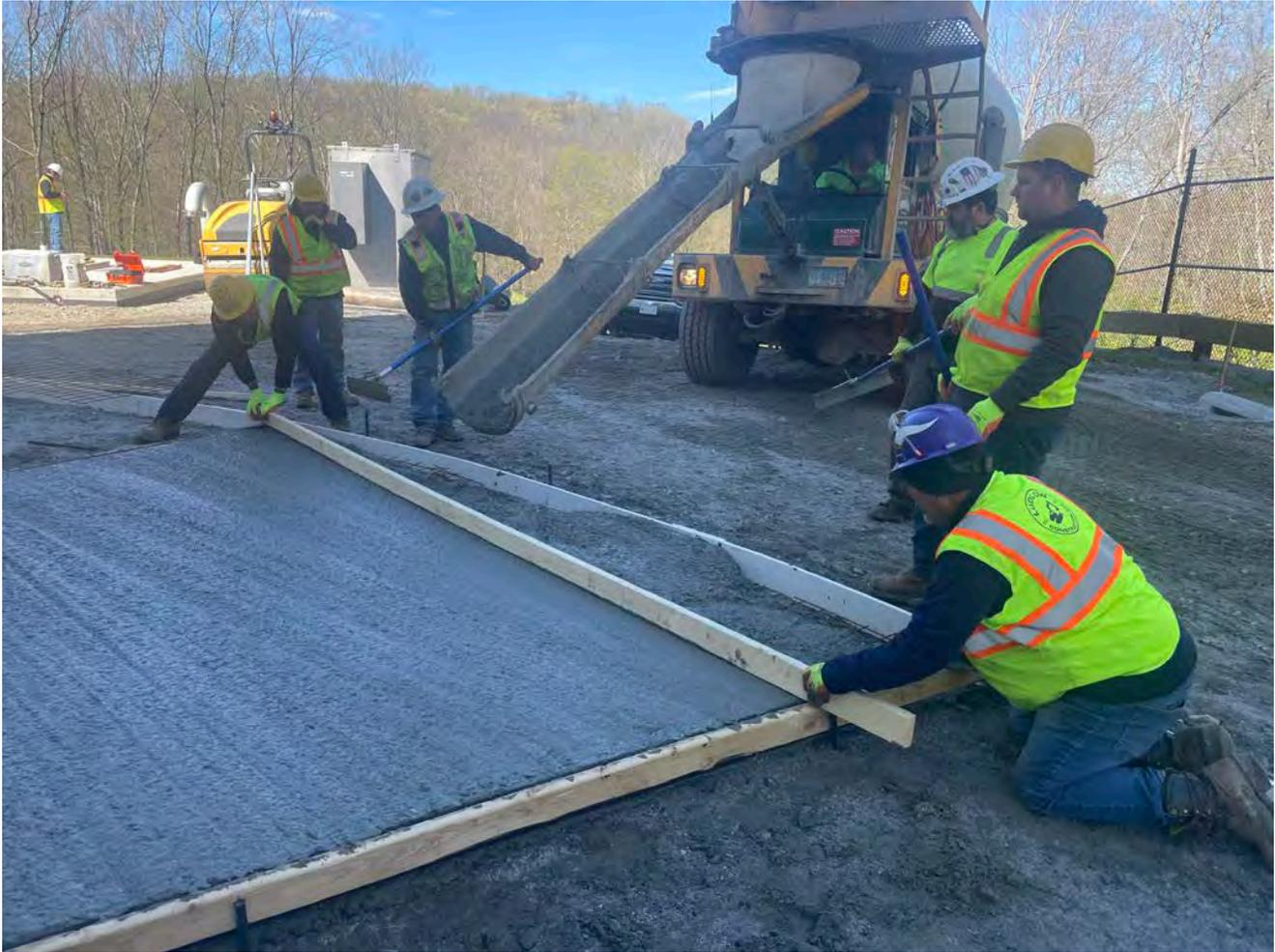
Picture 5: Ludlow using a 2"x4" to level the top of the concrete they are pouring as part of sidewalk installation activities on the west side of the water tank. View to the west.
