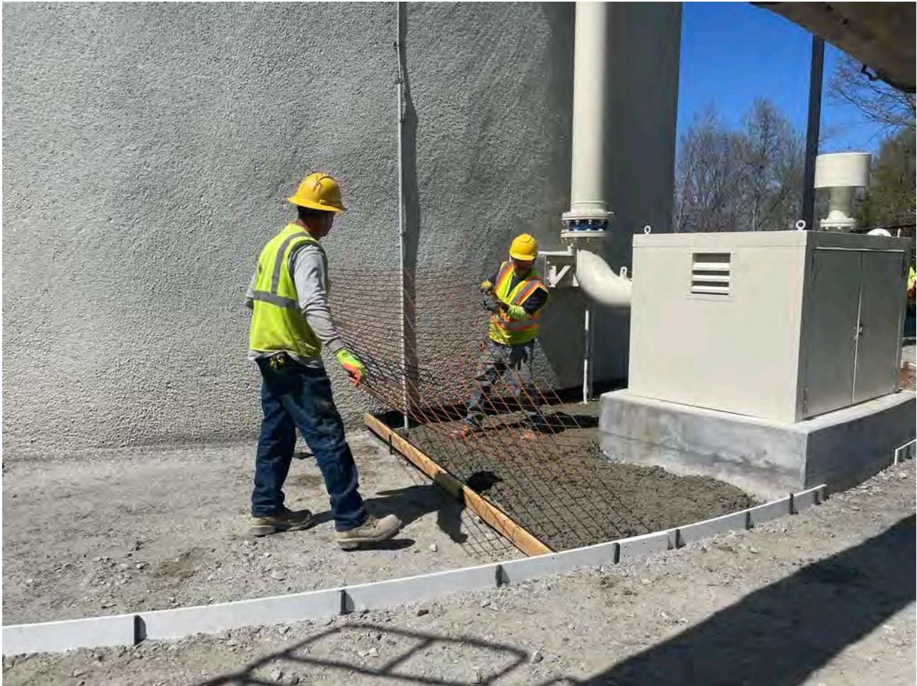
Picture 7: Ludlow placing 4"x4" steel screen in the panel that surrounds the base of the blower located on the northeast side of the water tank. View to the northwest.
