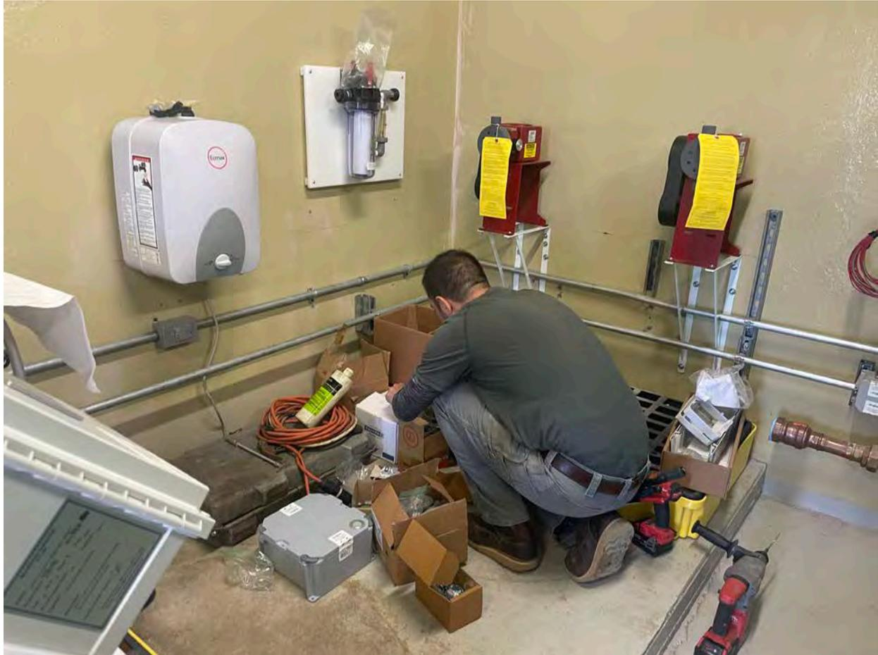
Picture 3: A&R Electrical continuing the installation of wiring at the Long Hill pump station in Middletown that is associated with the new chlorination system. View to the southeast.
