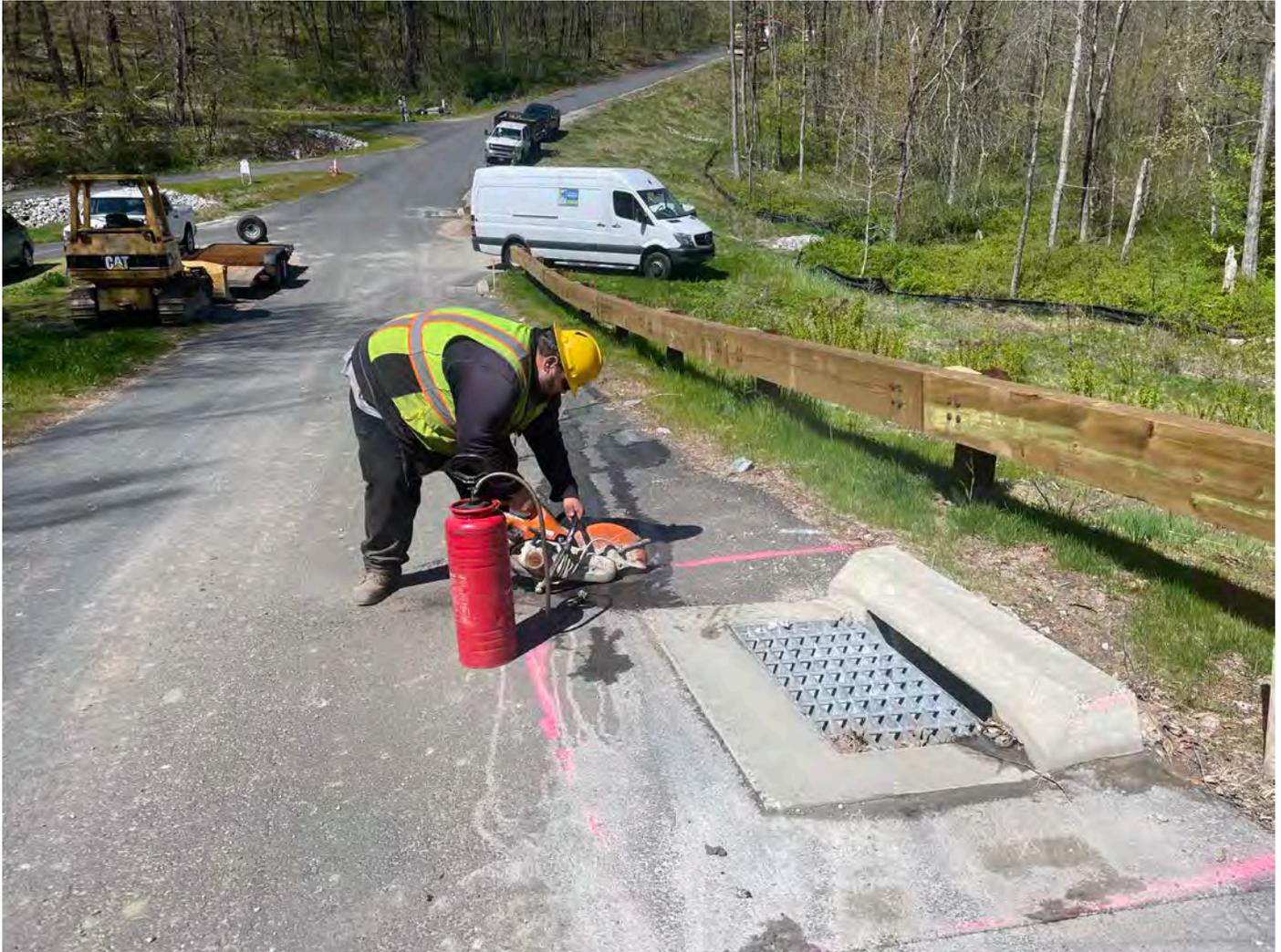
Picture 9: Ludlow saw cutting pavement around the catch basin located at Station 13+00 on the Shared Access Road in Middletown. The catch basin is scheduled to be raised 1.75". View to the west.
