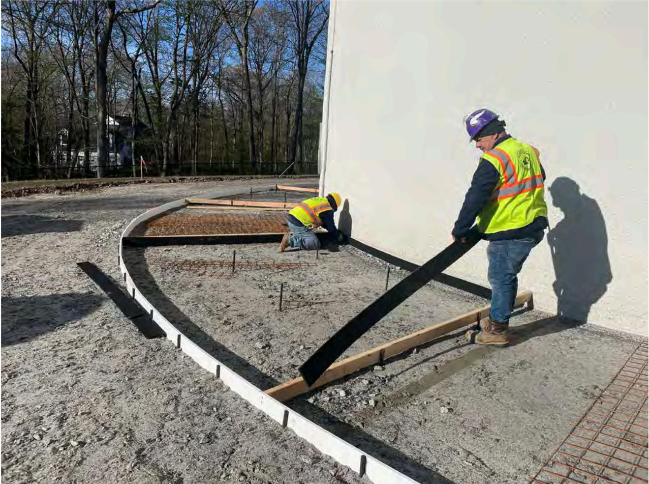
**Picture 1: Ludlow placing expansion joints on the concrete form they built for the construction of the concrete sidewalk they are installing around the base of the water tank located east of the Shared Access Driveway in Middletown.**
