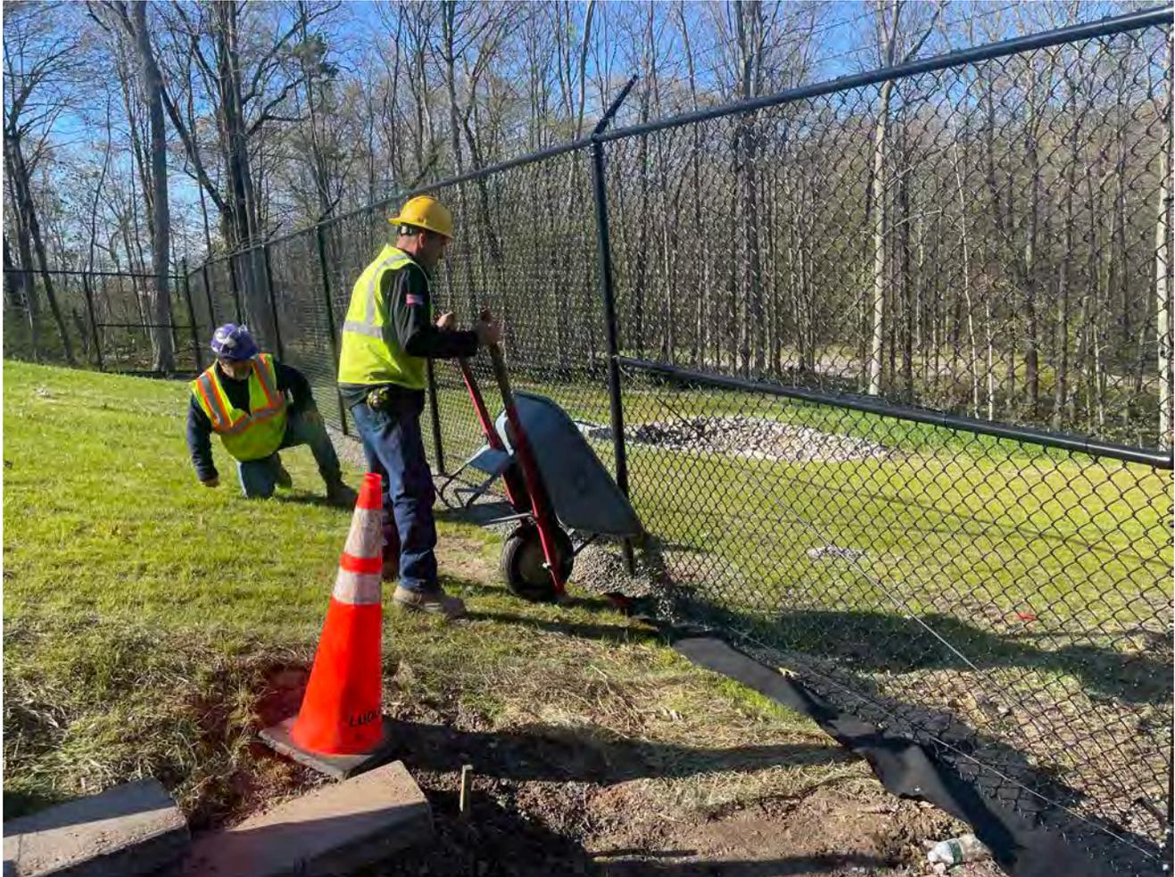
Picture 2: Ludlow placing 3/8" stone over black geofabric at the toe of the chain link fence located west of the water tank located east of the Shared Access Driveway in Middletown. View to the south.
