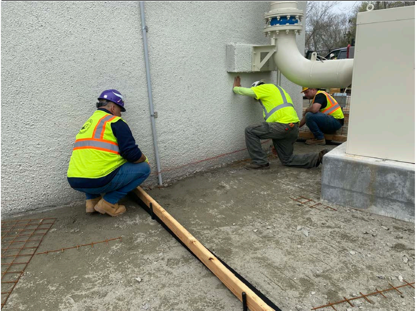
Picture 4: Ludlow chalks the perimeter of the tank for a reference of depth when pouring the concrete.
