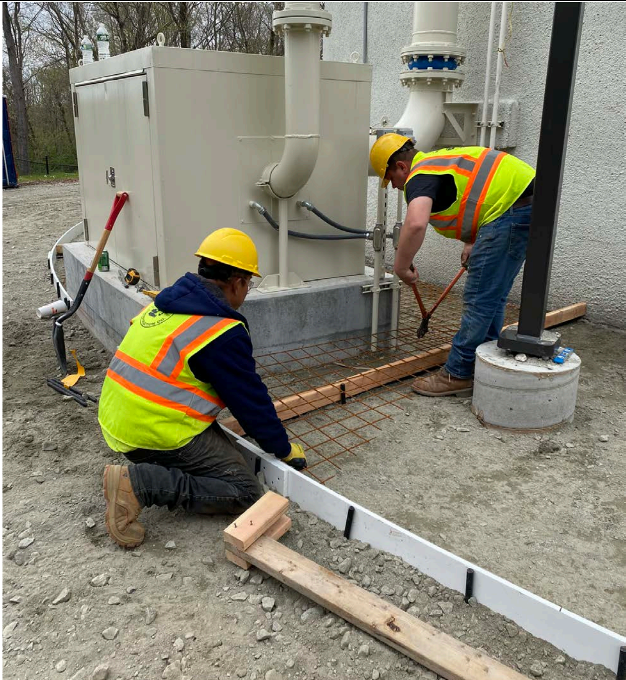
Picture 2: Ludlow cuts the wire mesh sheets to fit within in each 15' section.
