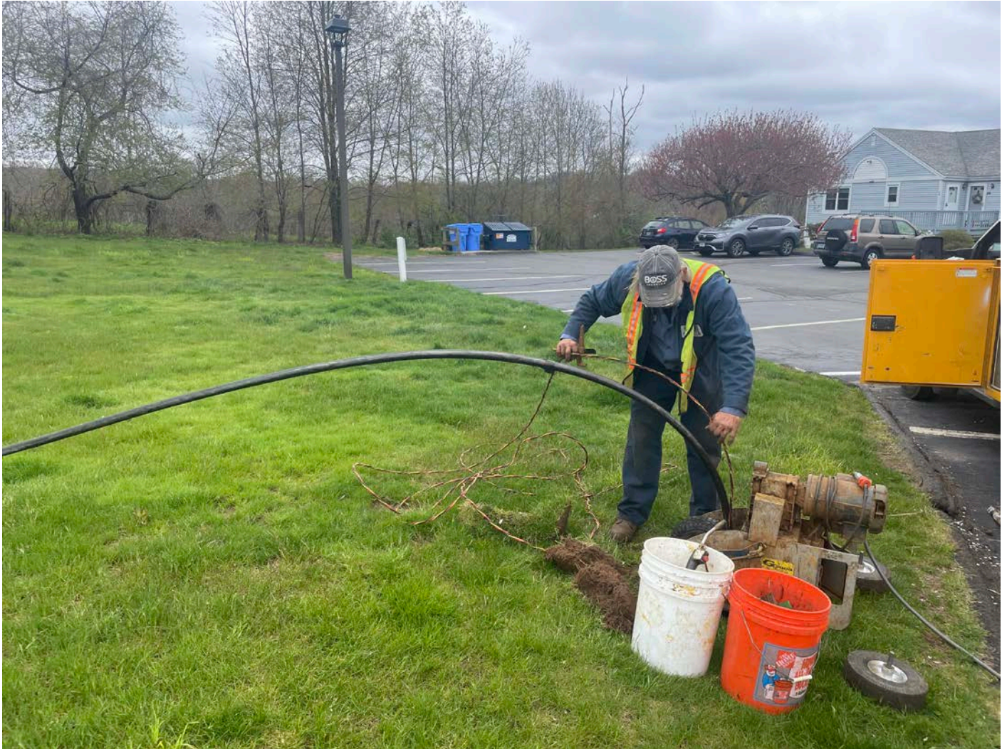
Picture 8: Grela removing the pump from the third of three wells located at the condominium complex on Mill Pond Lane in Durham. View to the northeast.
