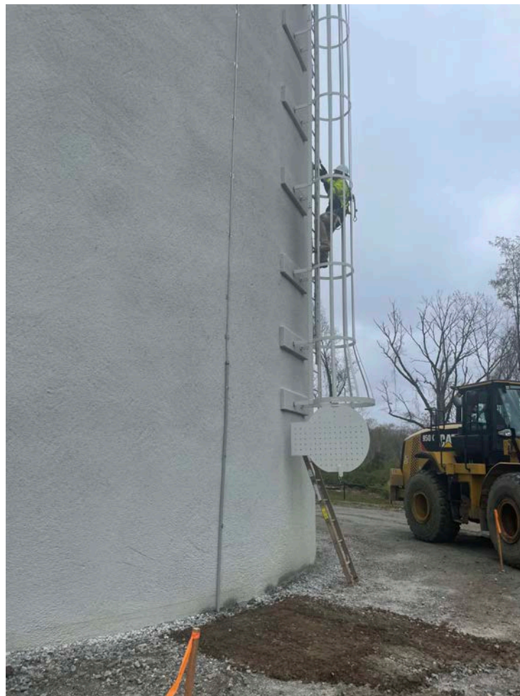
Picture 4: DN Tanks ascending the water tank located to the east of the Shared Access Driveway in Middletown to collect a water level from the tank as part of their leak test activities. View to the east.
