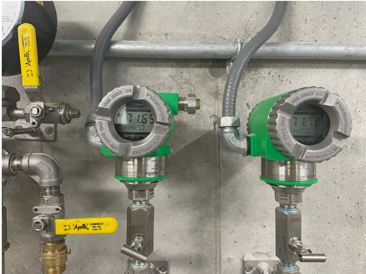
Picture 3: Water tank level gauges in the altitude vault (water tank is currently full). View to the south.
