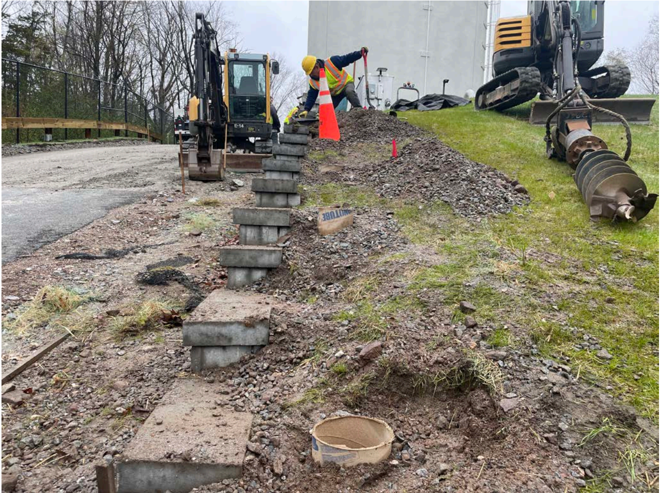
Picture 1: Ludlow working on the installation of Sonotubes on the south side of the retaining wall located between Stations 10+65 and 11+35 on the Shared Access Driveway in Middletown. View to the east.
