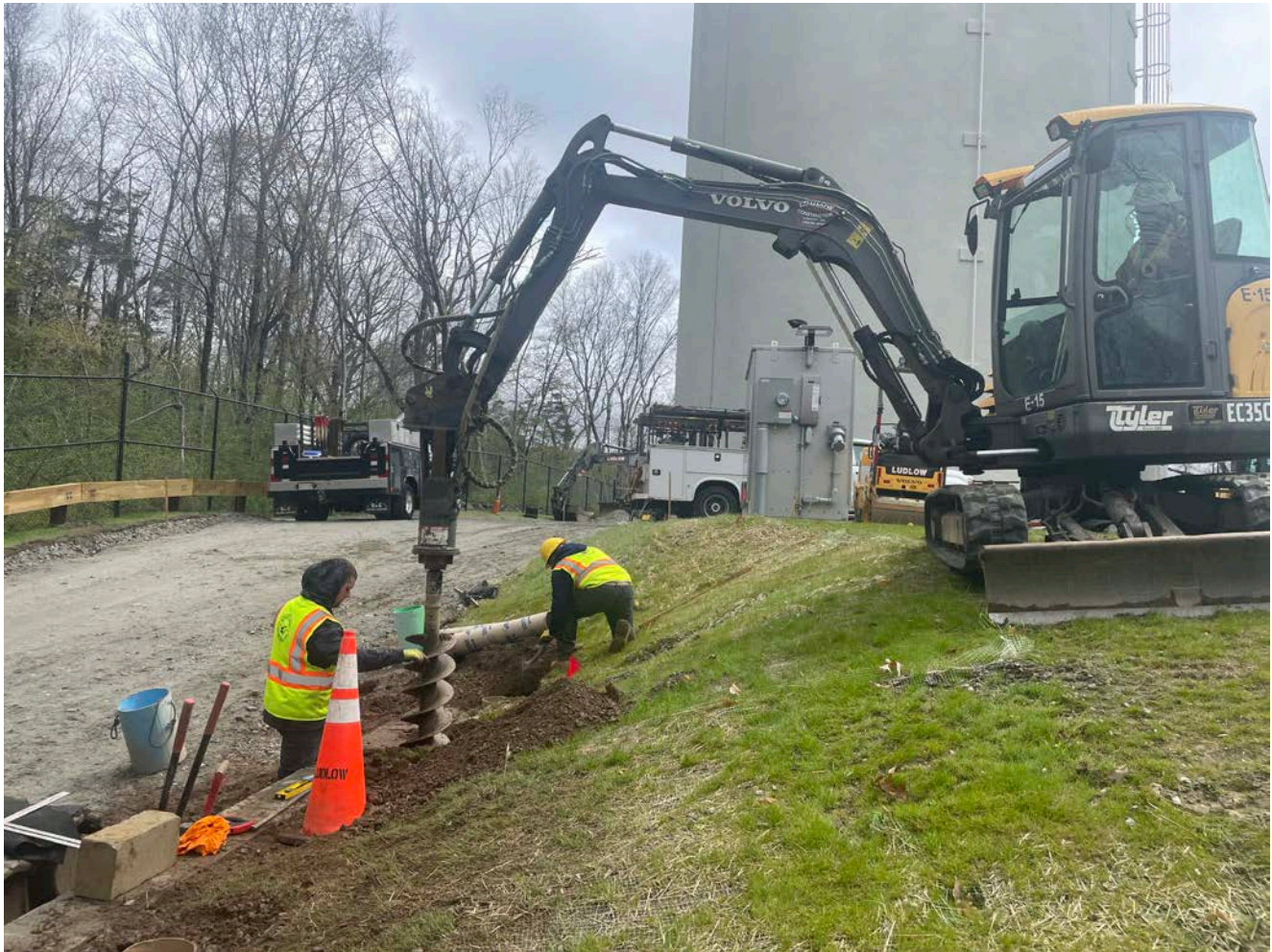
Picture 2: Ludlow auguring a hole on the south side of the retaining wall located between Stations 10+65 and 11+35 on the Shared Access Driveway in Middletown for the installation of a Sonotube. View to the east.
