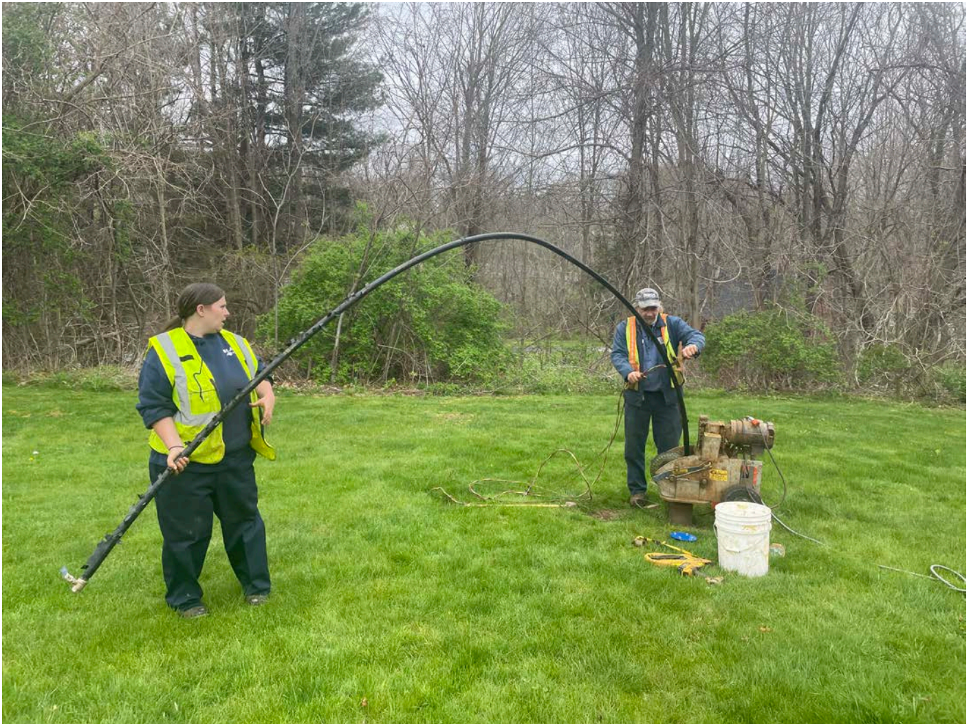
Picture 6: Grela removing the pump from the first of three wells located at the condominium complex on Mill Pond Lane in Durham. View to the southwest.
