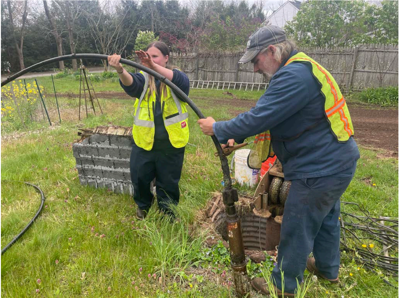
Picture 5: Grela removing the pump from the well located on the north side of the 230 Maple Avenue, Durham, property. View to the southwest.
