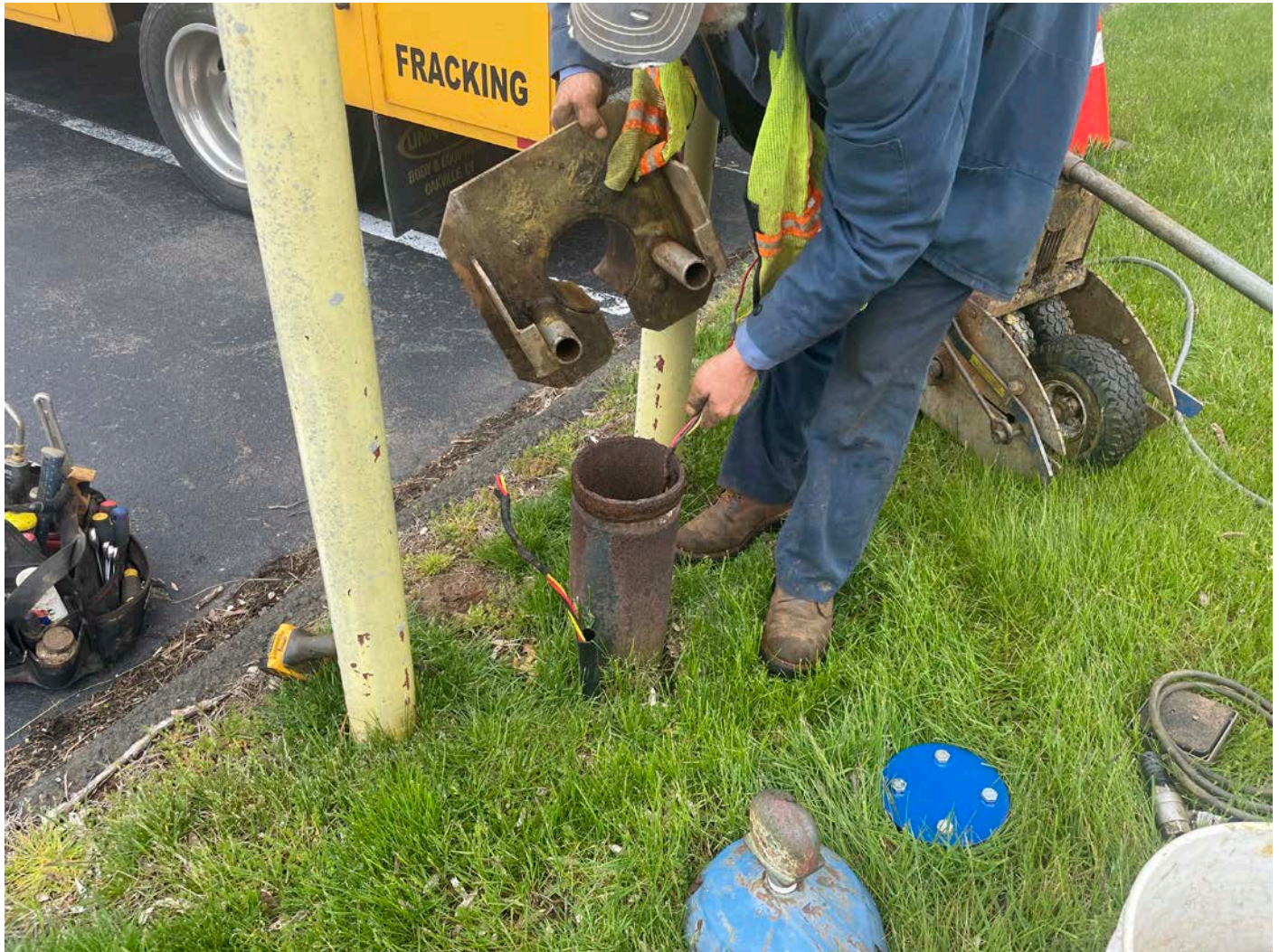
Picture 7: Grela setting up the pump puller on the second of three wells located at the condominium complex on Mill Pond Lane in Durham. View to the southwest.
