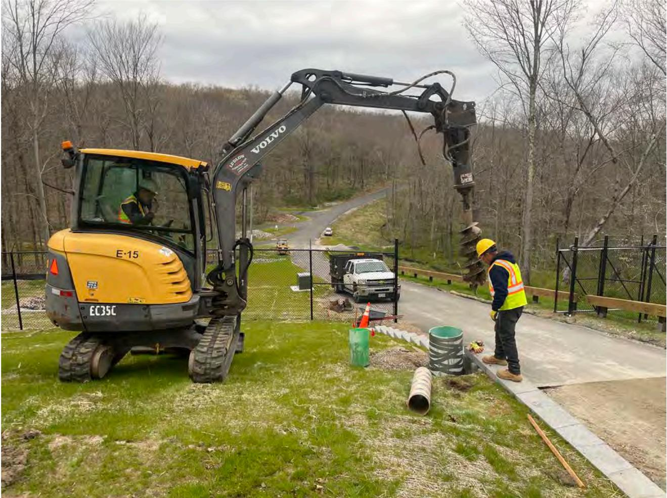
**Picture 1: Ludlow auguring a hole for the placement of a 4' section of 8" diameter Sonotube on the south side of the retaining wall located between Stations 10+65 and 11+35 on the Shared Access Driveway in Middletown. View to the west.**
