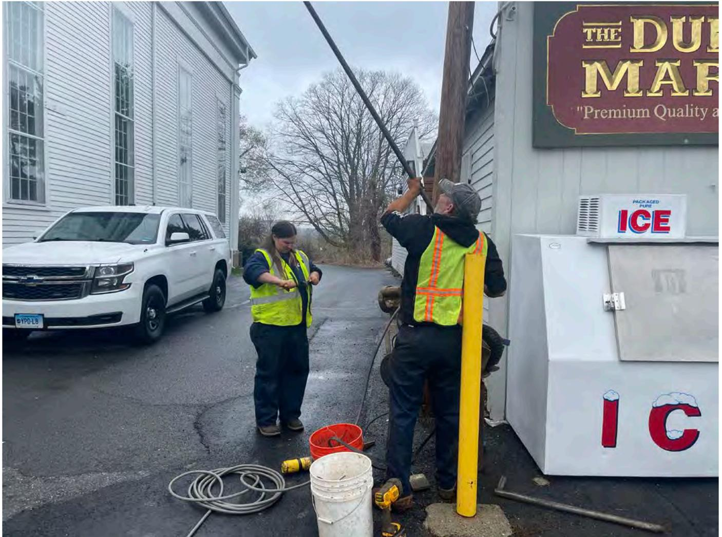
Picture 8: Grela removing the pump from the well located on the north side of the 238 Main Street, Durham, property. View to the west.
