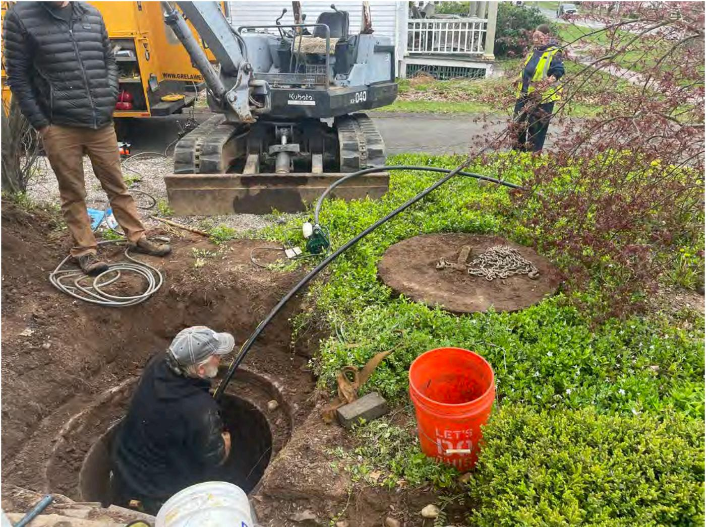
Picture 9: Grela removing the pump from the well located at 293 Main Street, Durham, property. View to the south.
