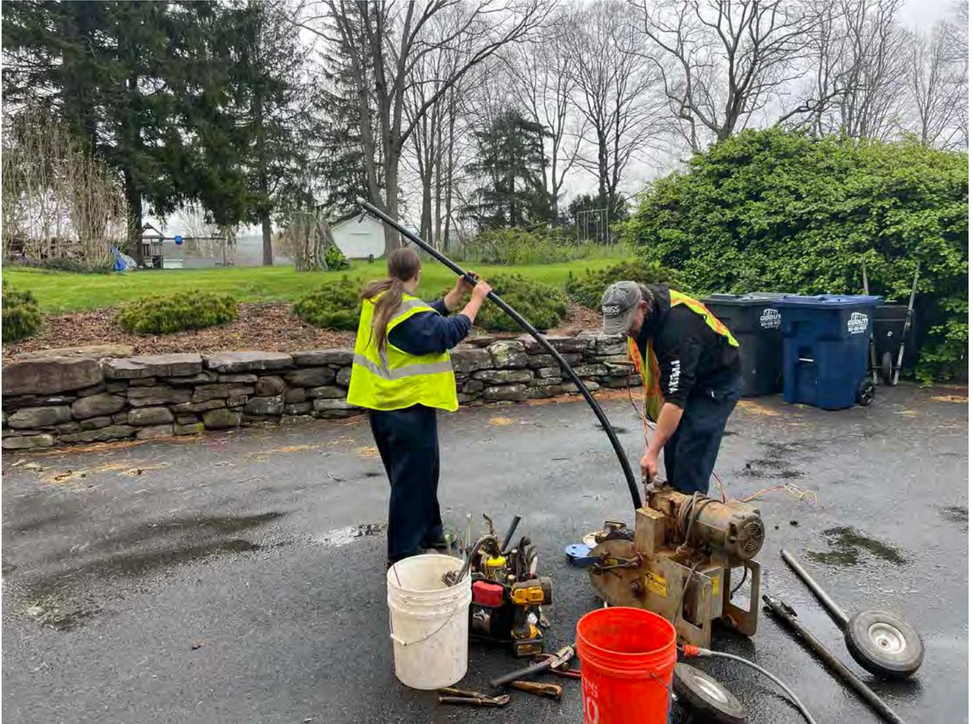
**Picture 7: Grela removing the pump from the well located on the north side of the 97R Maple Avenue, Durham, property. View to the southeast.**
