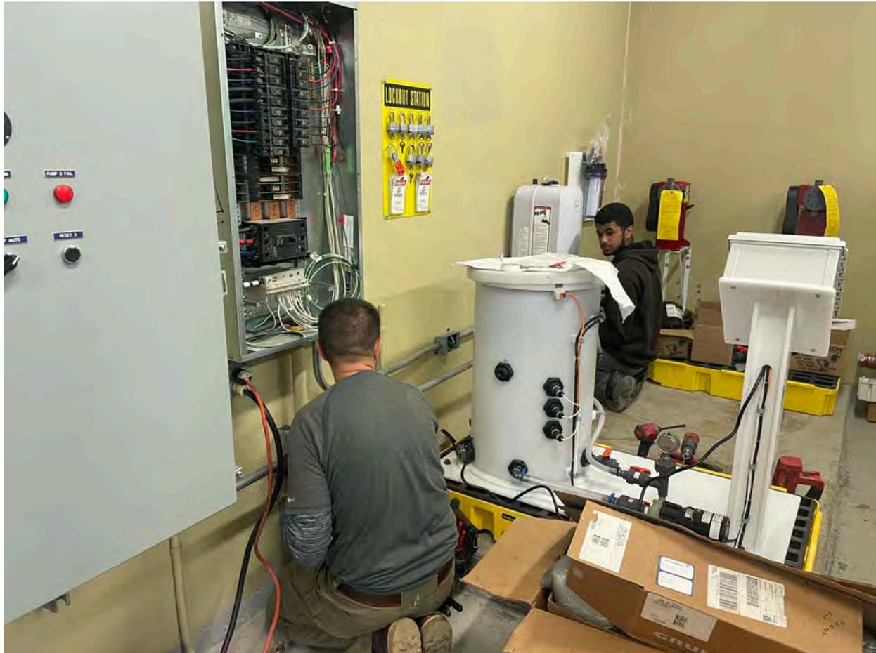
Picture 3: A&R Electrical installing electrical line conduits as part of the chlorination system being installed at the Long Hill pump station located on Long Hill Road in Middletown. View to the southeast.
