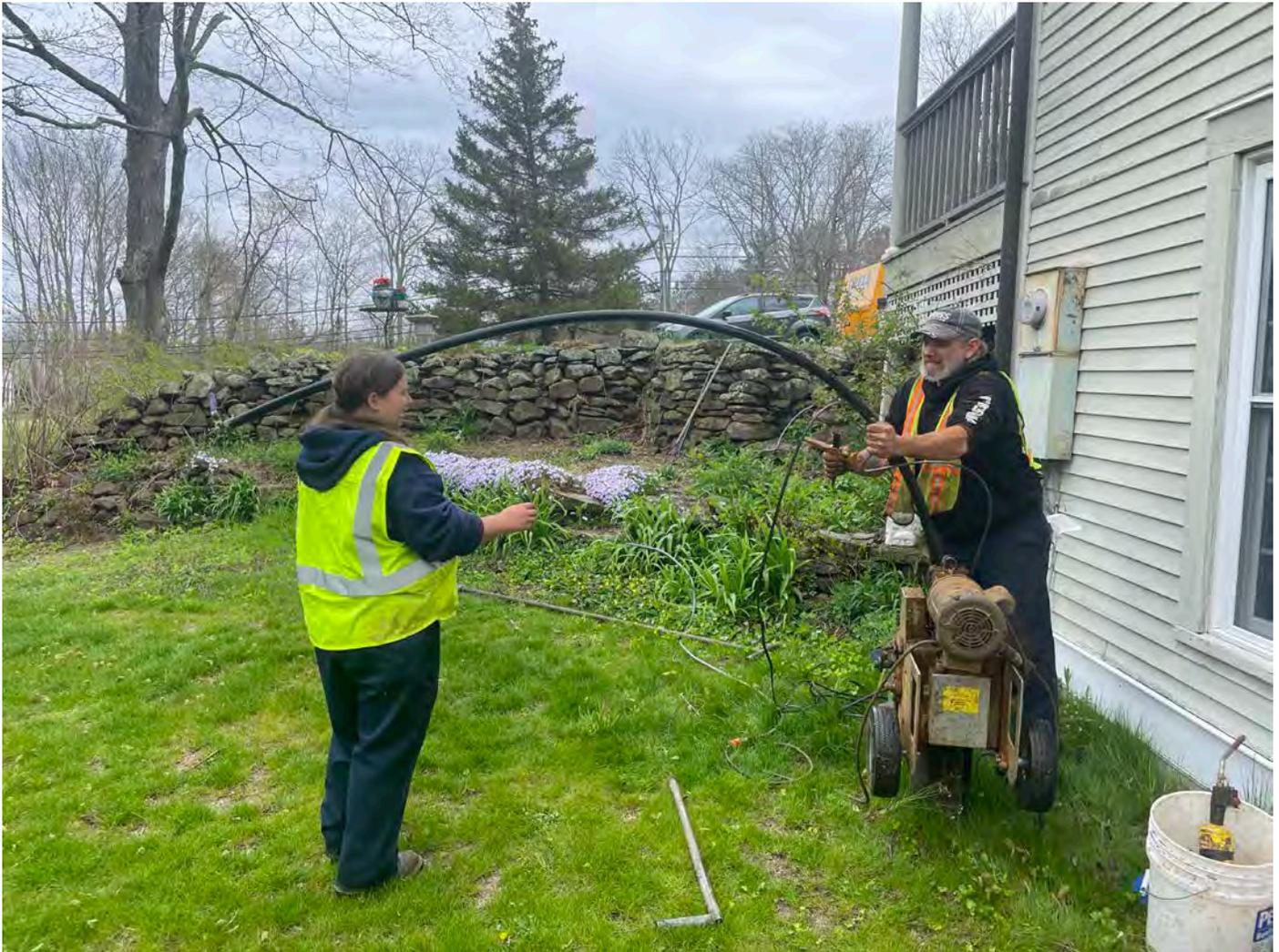
**Picture 6: Grela removing the pump from the well located on the north side of the 22 Wallingford Road, Durham, property. View to the north.**
