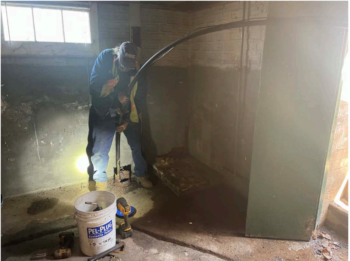
Picture 9: Grela removing the pump from the well located inside the basement of the 175 Maple Avenue, Durham, property. View to the northeast.
