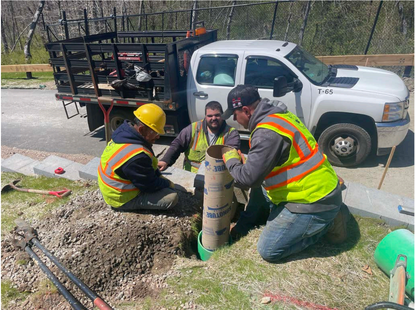
Picture 5: Ludlow installing a 4' section of 8" diameter Sonotube on the south side of the retaining wall located between Stations 10+65 and 11+35 on the Shared Access Driveway in Middletown. View to the northwest.
