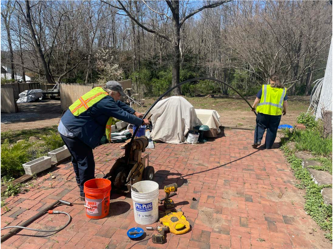
Picture 11: Grela removing the pump from the well located on the south side of the 244 Maple Avenue, Durham, property. View to the west.
