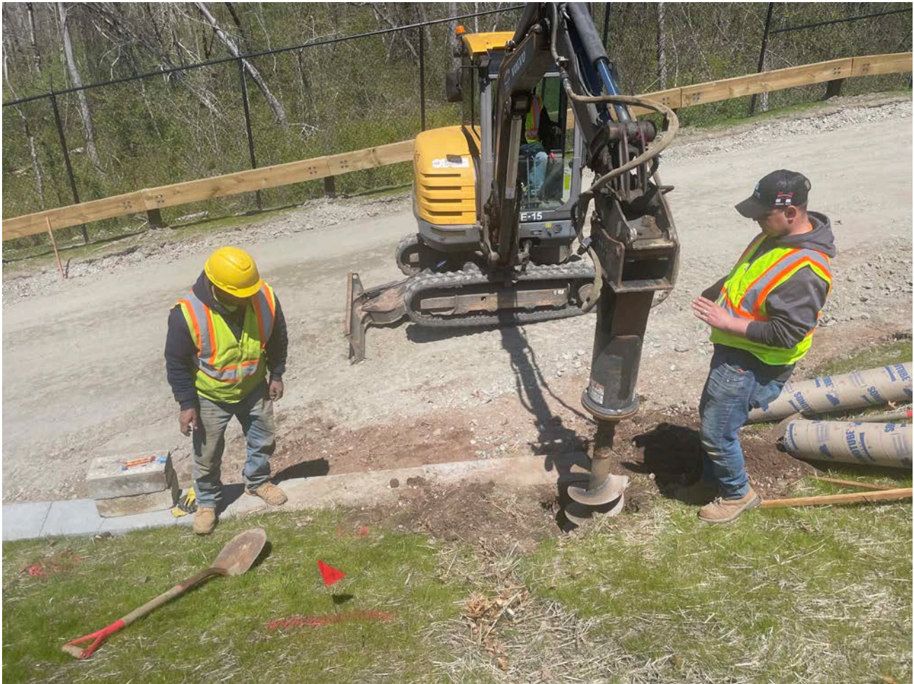
Picture 4: Ludlow auguring a hole for the placement of a 4' section of 8" diameter Sonotube on the south side of the retaining wall located between Stations 10+65 and 11+35 on the Shared Access Driveway in Middletown. View to the north.
