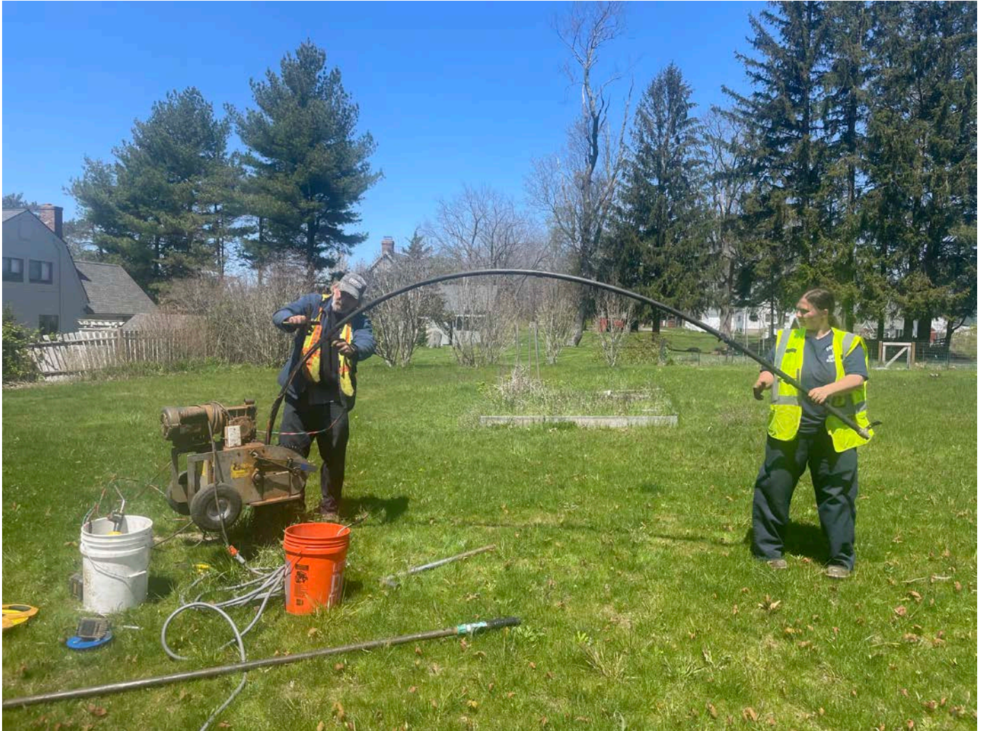
Picture 7: Grela removing the pump from the well located on the north side of the 95R Maple Avenue, Durham, property. View to the north.
