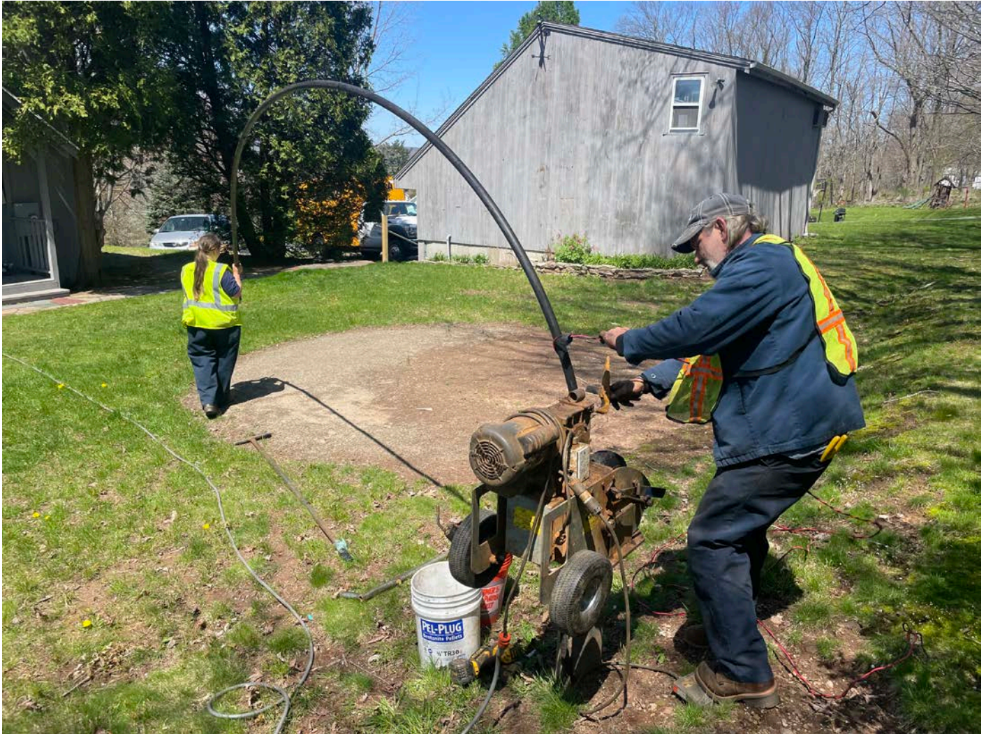
Picture 8: Grela removing the pump from the well located on the north side of the 119 Maple Avenue, Durham, property. View to the northwest.
