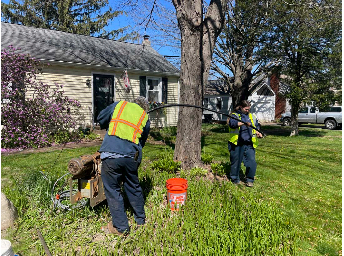
Picture 9: Grela removing the pump from the well located on the east side of the 184 Maple Avenue, Durham, property. View to the northwest.
