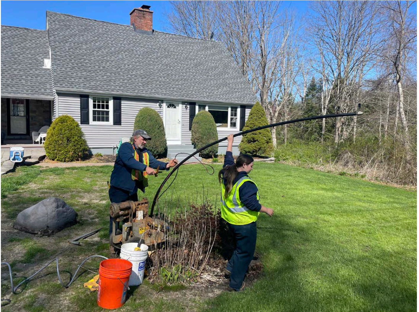
Picture 10: Grela removing the pump from the well located on the east of the 206 Maple Avenue, Durham, property. View to the northwest.
