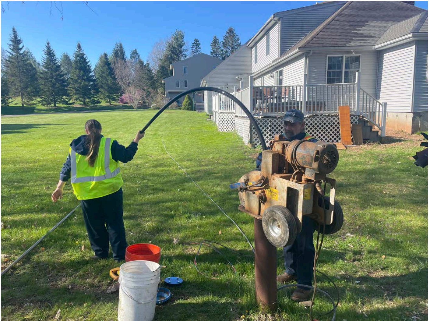
Picture 6: Grela removing the pump from the well located on the north side of the 10 Johns Way, Durham, property. View to the south.
