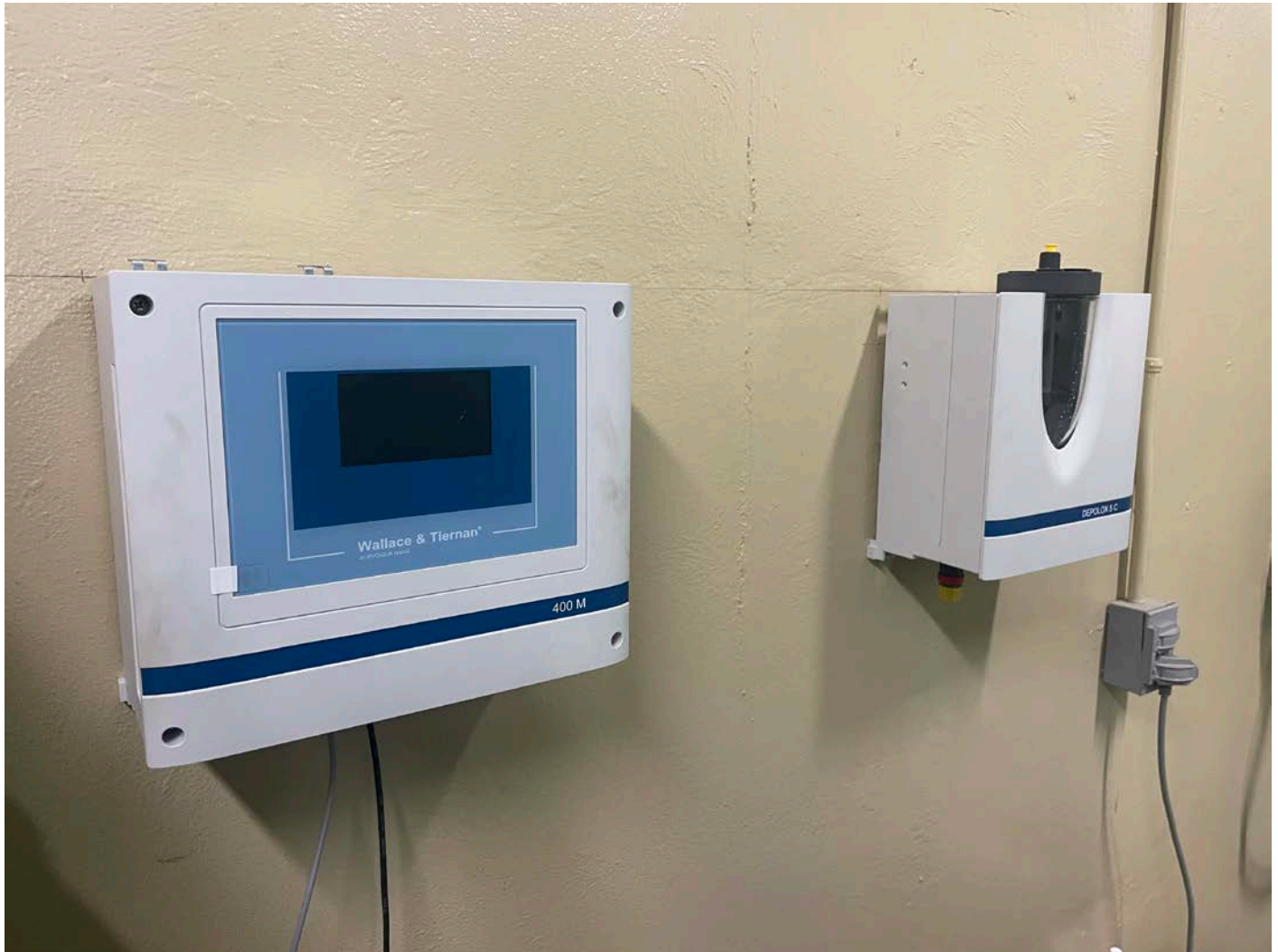
Picture 2: Chlorine monitor (Wallace & Tiernan 400M) and analyzer (Depolox 5 C) that Ludlow installed on the south wall of the Long Hill pump station. View to the southwest.
