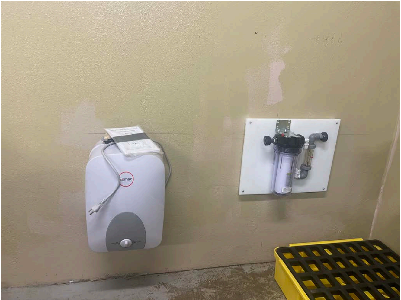
Picture 5: Water heater and filter that Ludlow installed on the east wall of the Long Hill pump station. View to the southeast.
