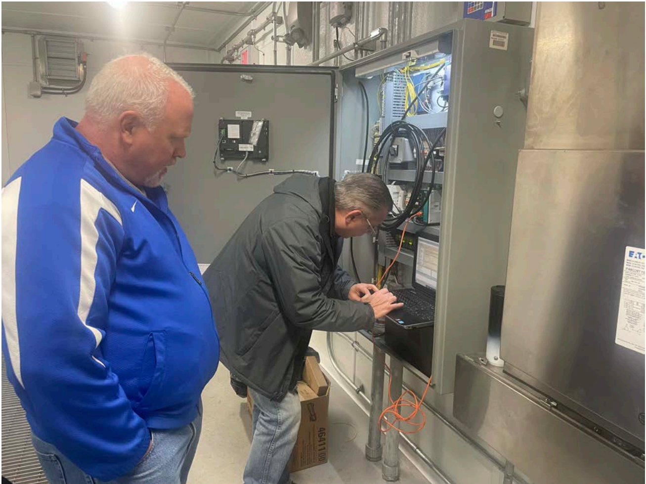
Picture 4: Knapp Engineering working on the communication system at the booster station located on S. Main Street in Middletown. View to the northwest.
