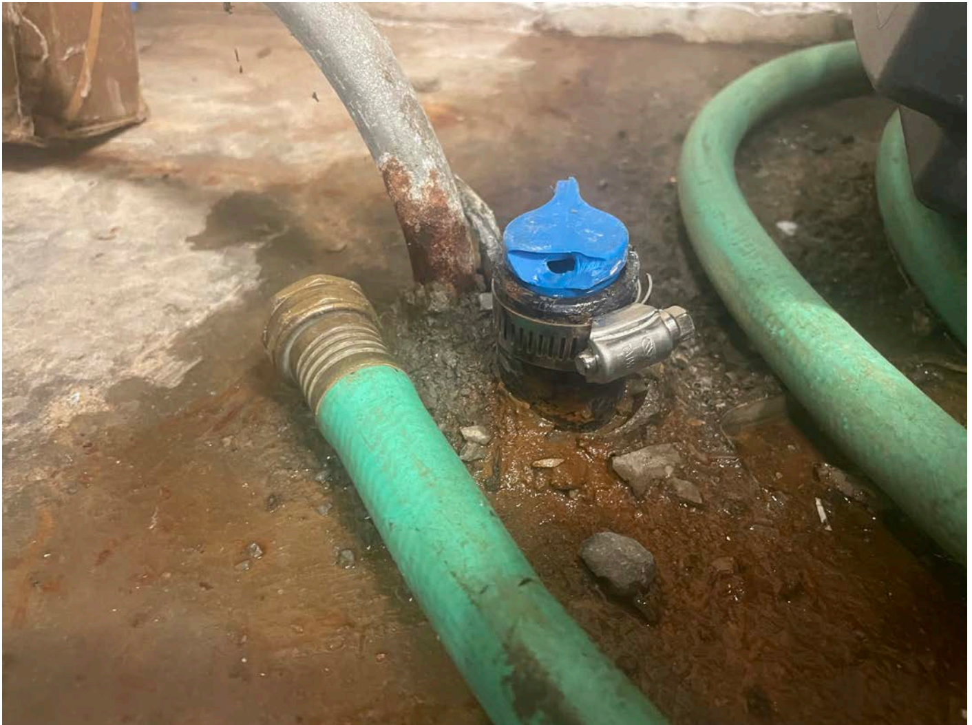
Picture 6: Damaged cap located on top of the black plastic well line on the basement floor of the 212R Maple Avenue residence. View to the southwest.
