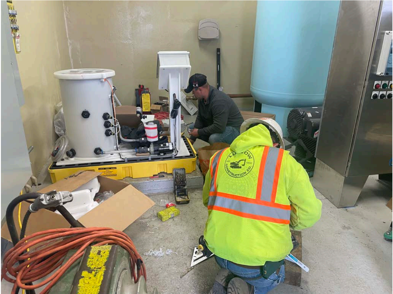
Picture 1: Ludlow continuing work on the installation of a chlorination system at the Long Hill pump station located on Long Hill Road in Middletown. View to the south.
