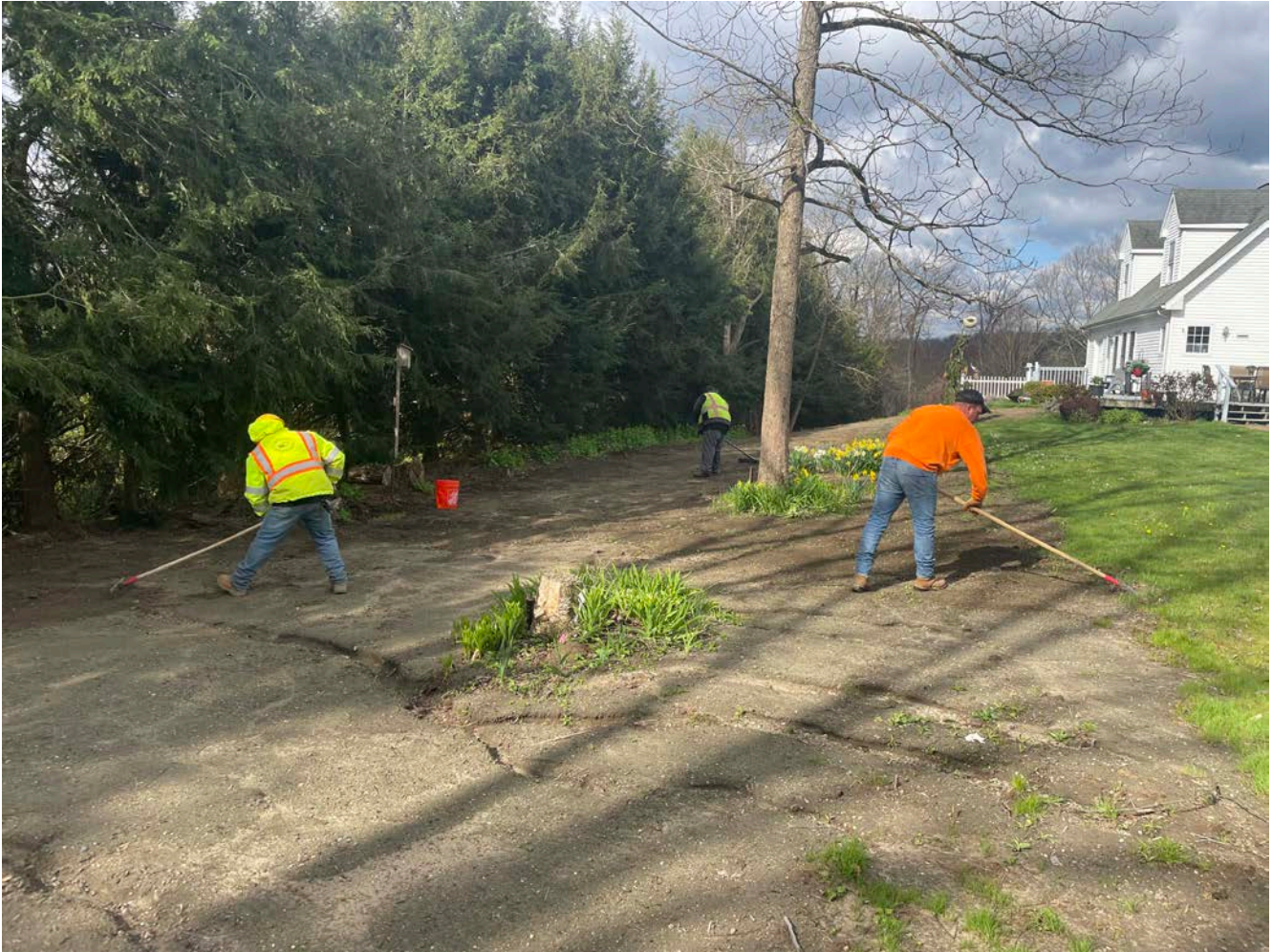
Picture 9: Ludlow performing restoration activities on the areas of the 228R Maple Avenue property that were disturbed last year during the installation of a copper water service line. View to the west.
