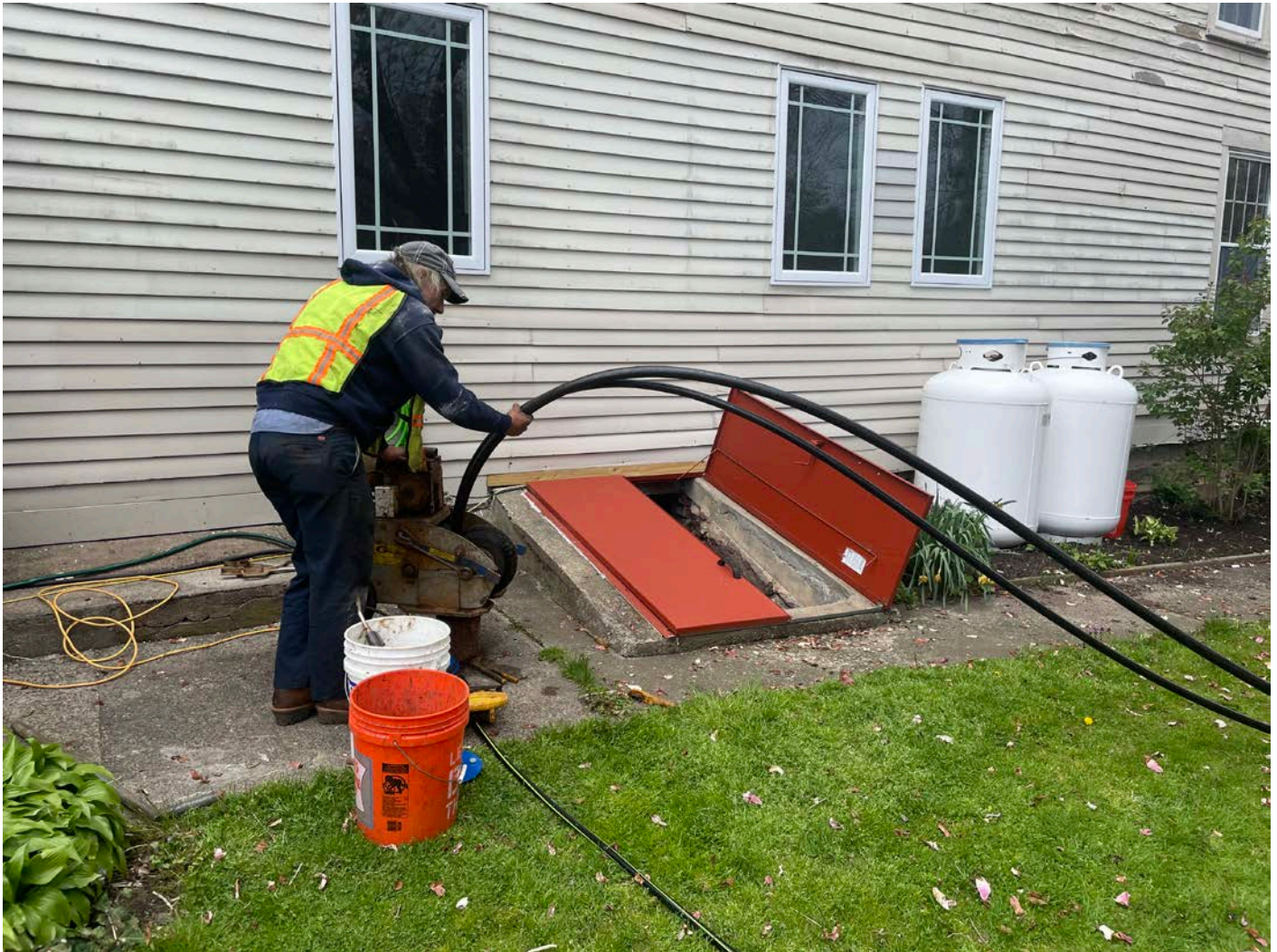
Picture 6: Grela pulling the pump from the well located at the 168 Main Street, Durham, residence. View to the northeast.
