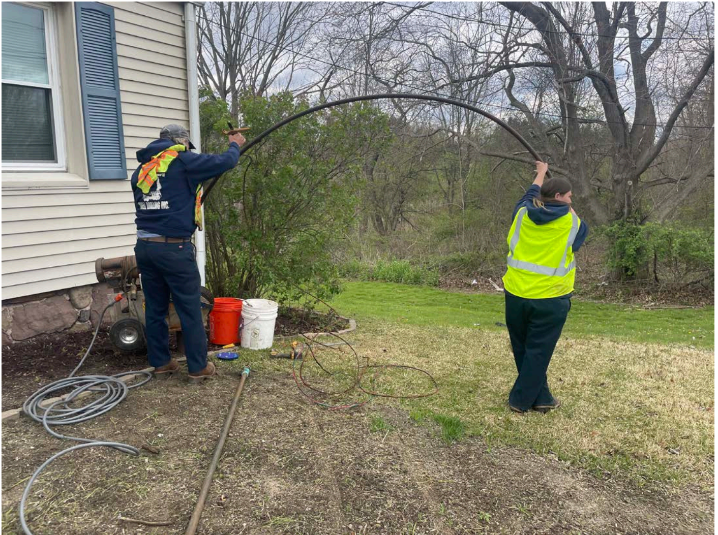
Picture 7: Grela pulling the pump from the well located at the 235 Maple Avenue, Durham, property. View to the southeast.
