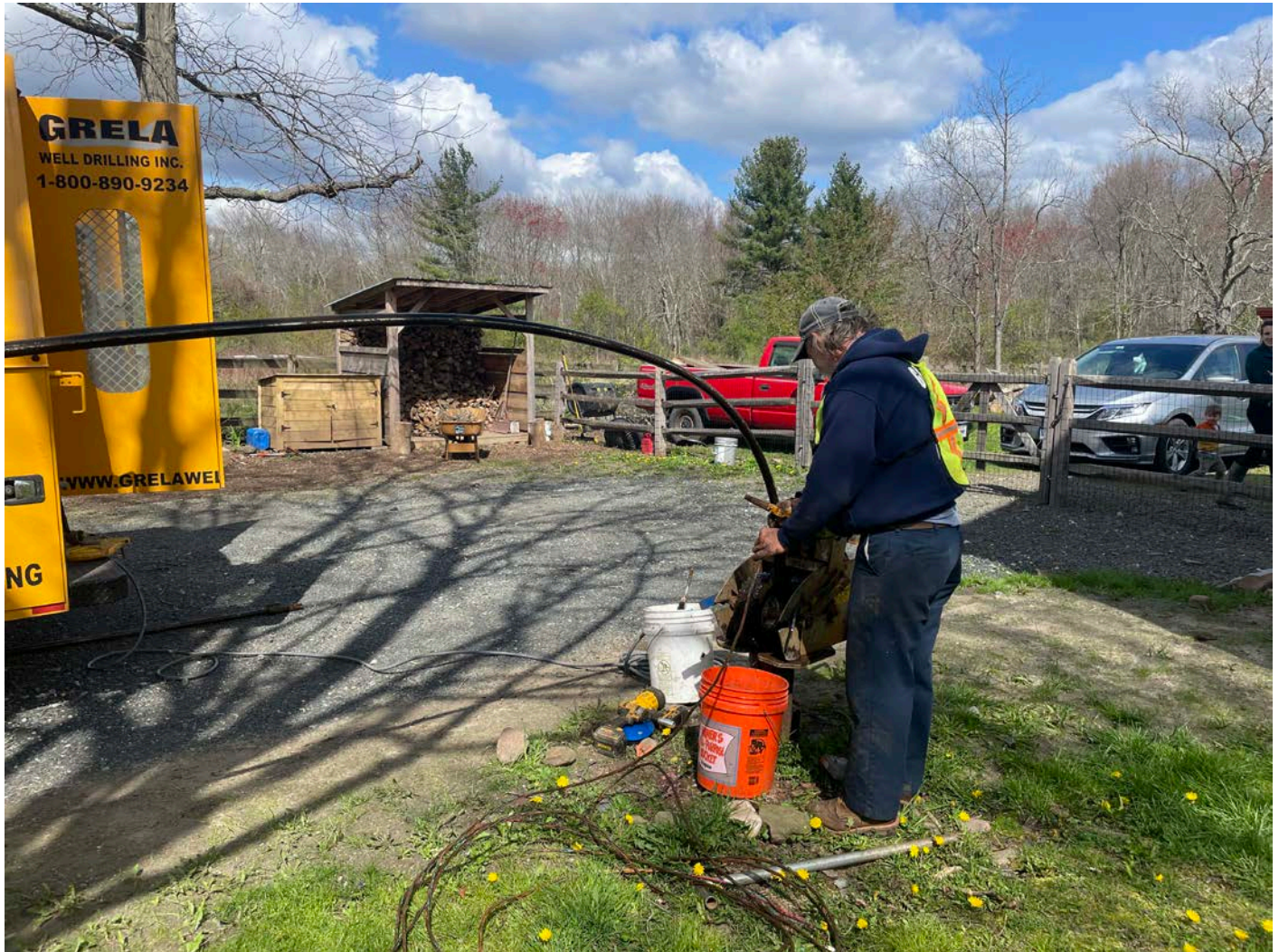
Picture 2: Grela pulling the pump from the well located at the 78 Maiden Lane, Durham, property. View to the northwest.
