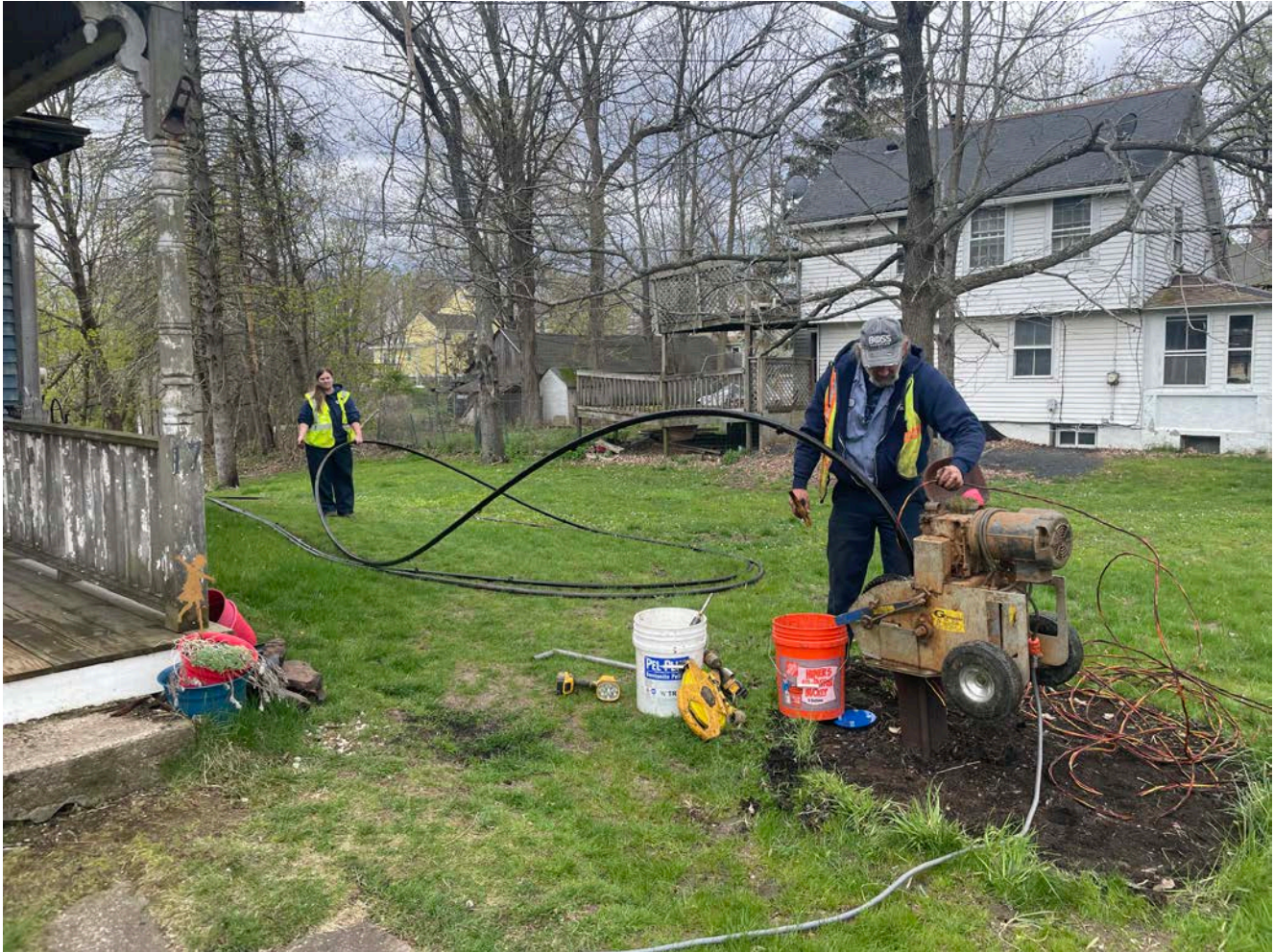
Picture 1: Grela pulling the pump from the well located at the 17 Maiden Lane, Durham, property. View to the southeast.
