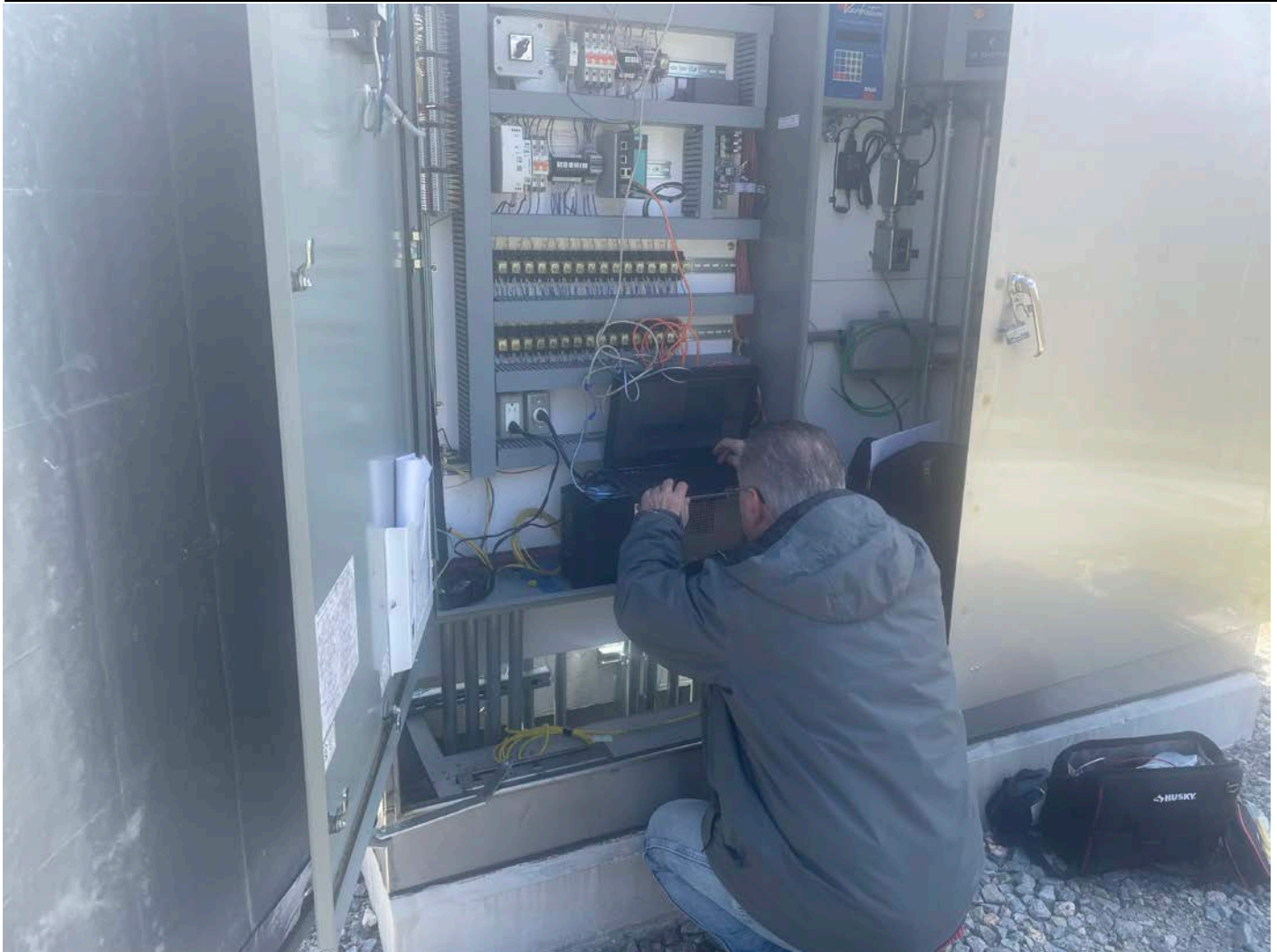
Picture 10: Knapp Engineering working on setting up relays inside of the electrical enclosure located on the west side of the water tank located east of the Shared Access Driveway in Middletown. View to the south.
