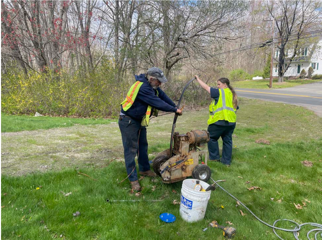
Picture 3: Grela pulling the pump from the well located at the 105 Maiden Lane, Durham, property. View to the northwest.
