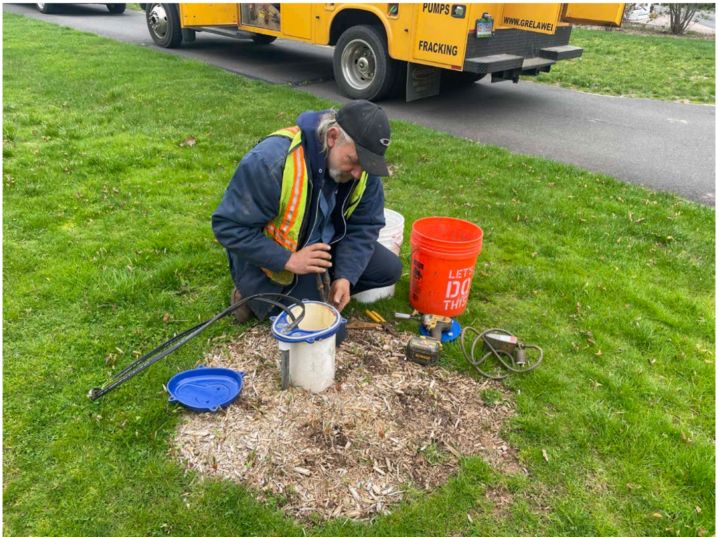
Picture 6: Grela pulling the pump from the well located at the 261 Main Street, Durham, residence. View to the northwest.
