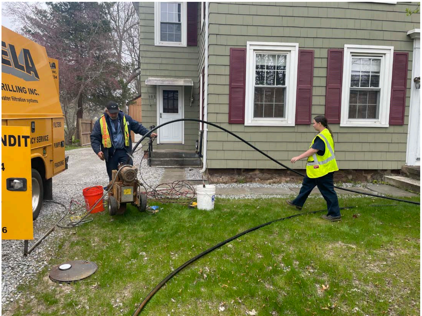
Picture 7: Grela pulling the pump from the well located at the 303 Main Street, Durham, property. View to the east.
