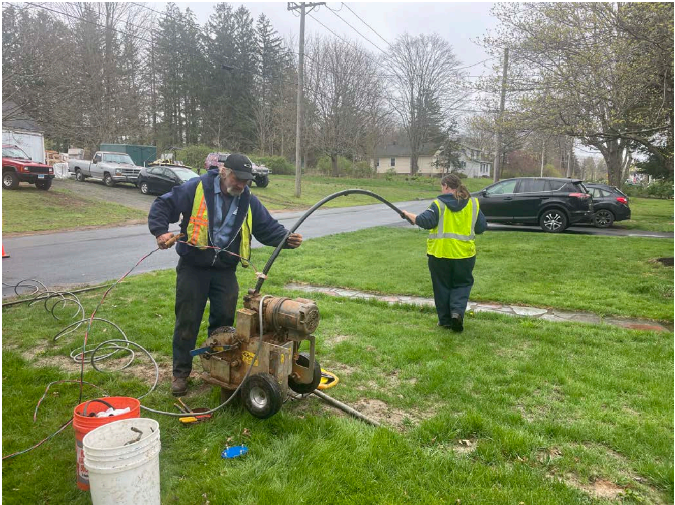
Picture 5: Grela having just pulled the pump from the well located at the 188 Maple Avenue, Durham, property. View to the southeast.
