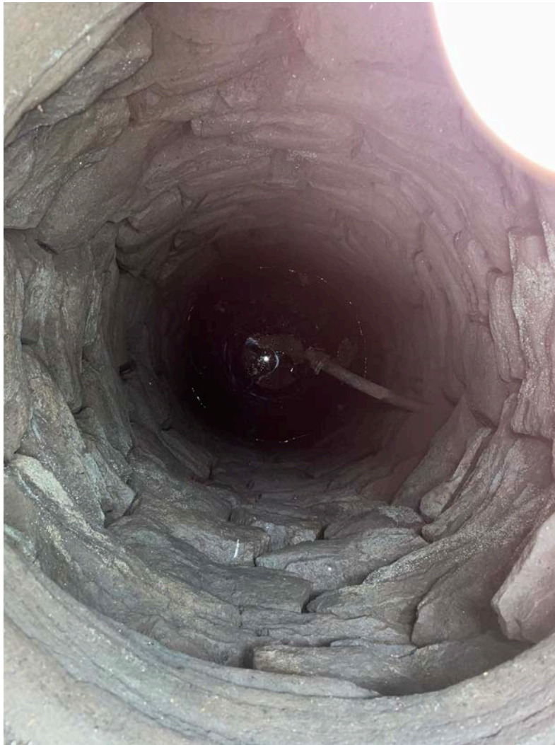
Picture 4: Inside of the dug well where the well at the 119 Main Street, Durham, property is located. Grela was unable to remove the pump from this well today due to logistical issues.
