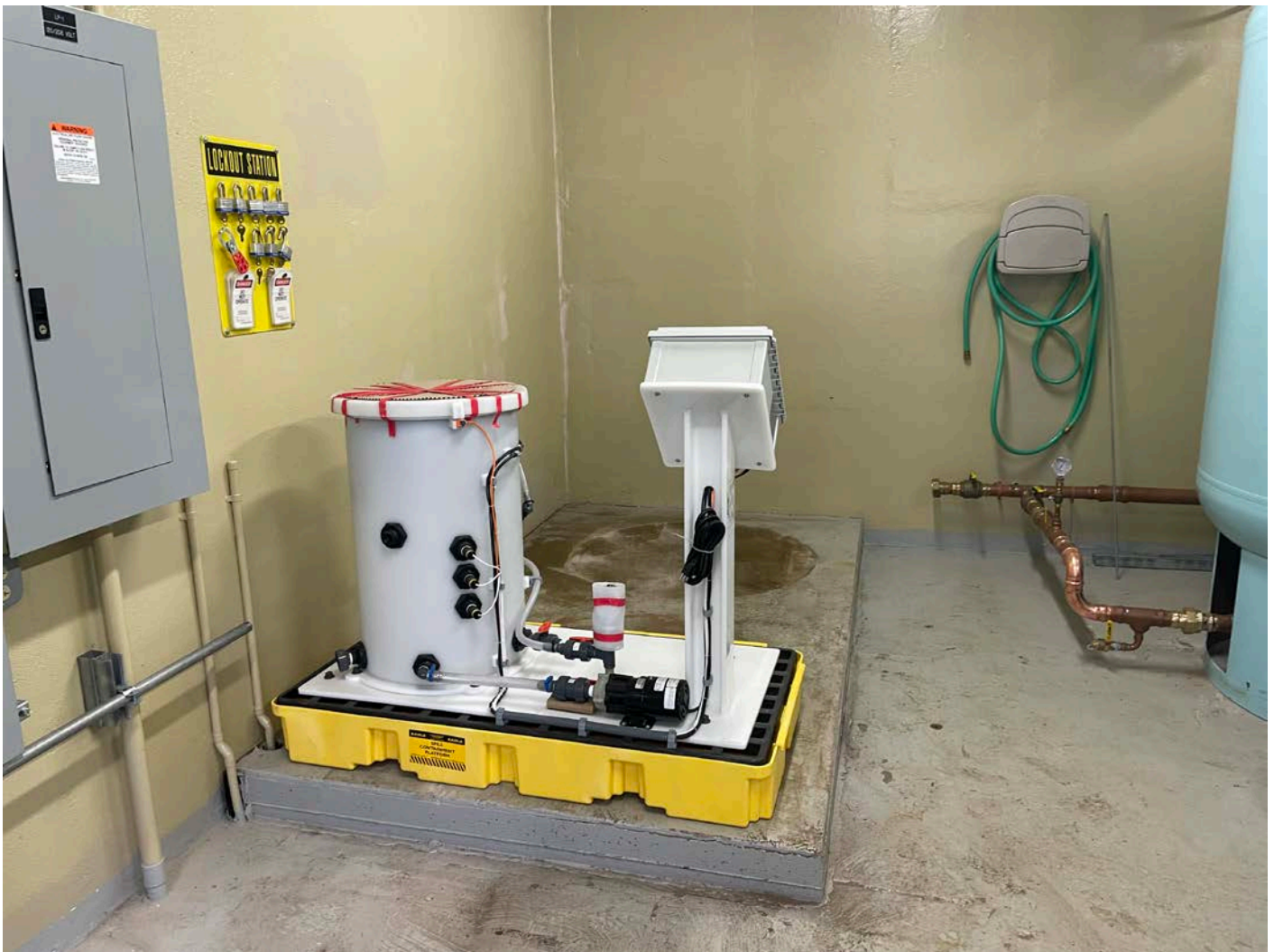
Picture 10: Chlorination station that Ludlow has placed on the concrete pad located at the southeast corner of the Long Hill pump station. View to the south.
