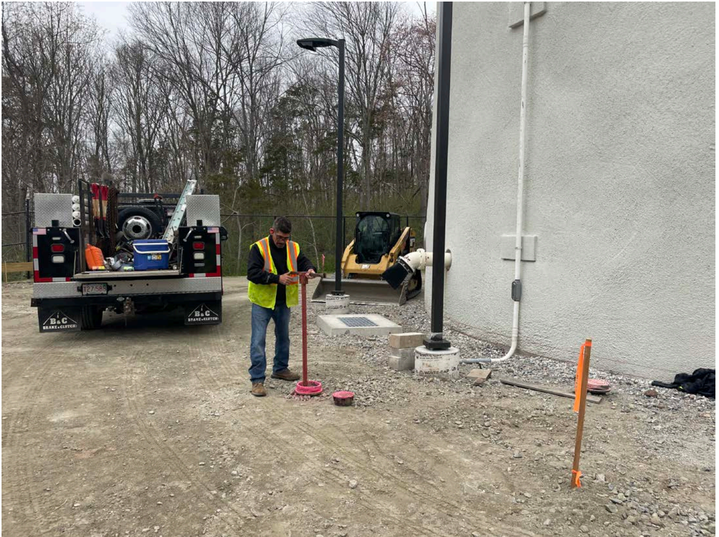
Picture 11: Ludlow opening a valve in order to fill the water tank located east of the Shared Access Driveway in Middletown. View to the north.
