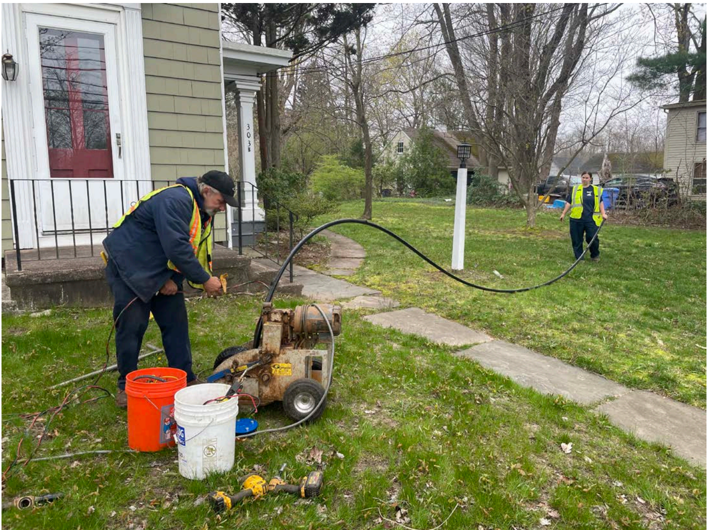
Picture 8: Grela pulling the pump from the well located at the 305B Main Street, Durham, property. View to the southeast.
