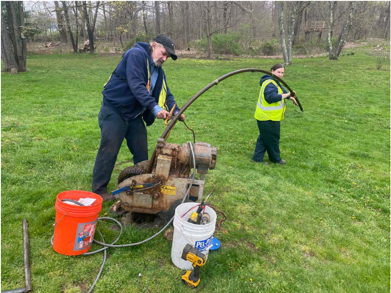
Picture 1: Grela pulling the pump from the well located at the 93R Maiden Lane, Durham, residence. View to the west.
