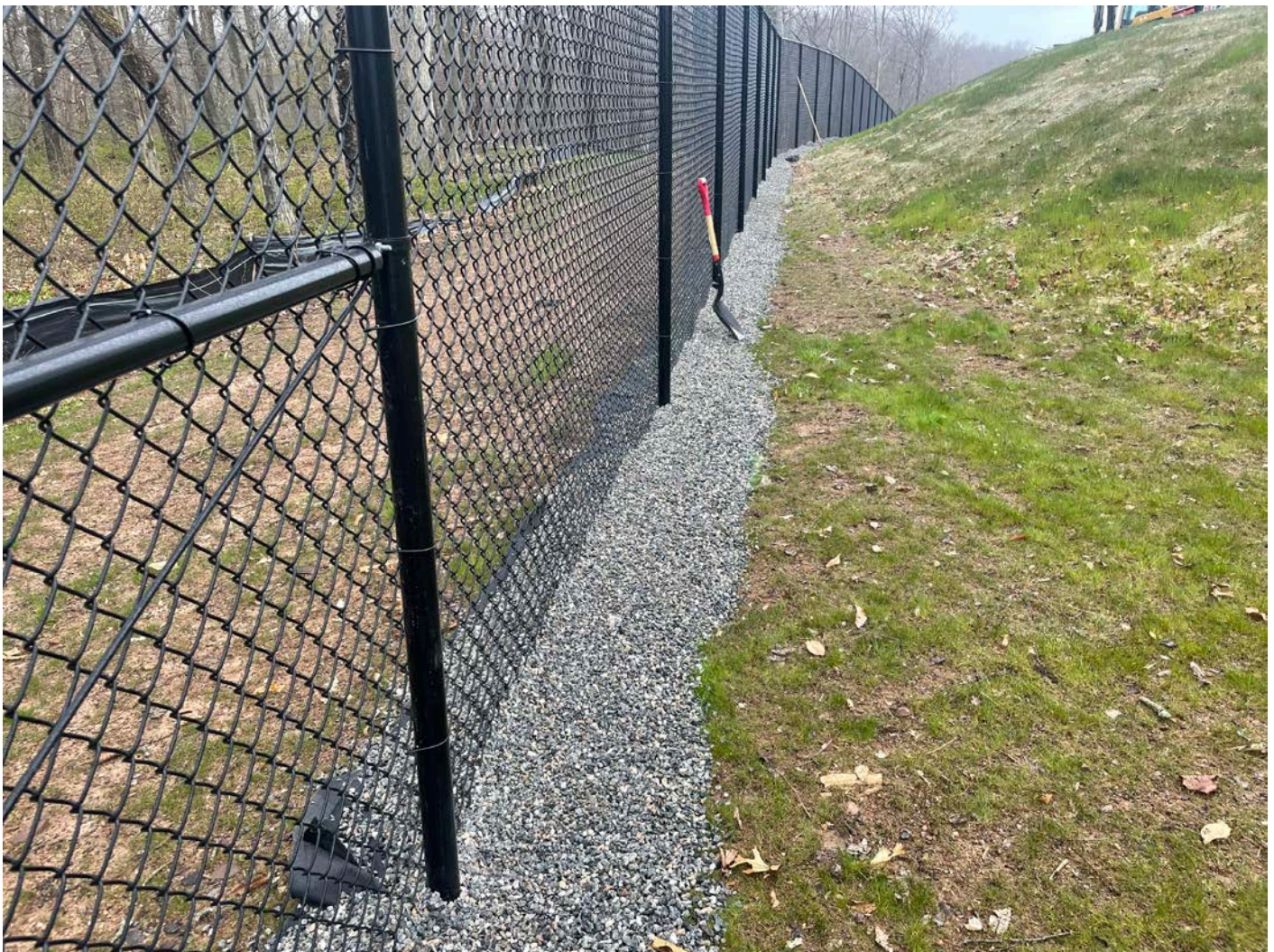
Picture 14: 3/8" stone that Ludlow placed over black geofabric along the bottom of the fence located south of the water tank located east of the Shared Access Driveway in Middletown. View to the west.
