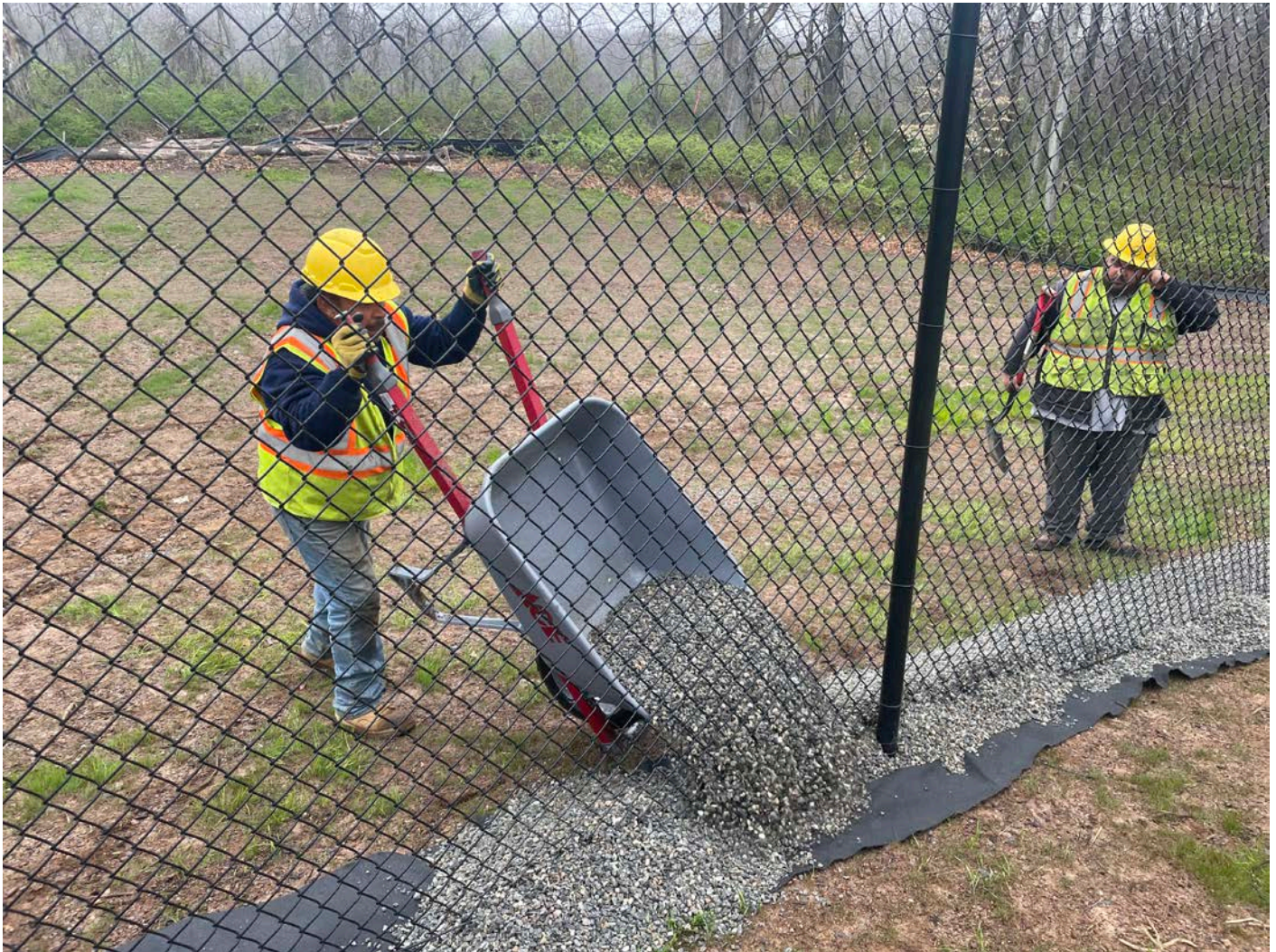
Picture 12: Ludlow placing 3/8" stone over black geofabric along the east side of the fence that surrounds the water tank located east of the Shared Access Driveway in Middletown. View to the southeast.
