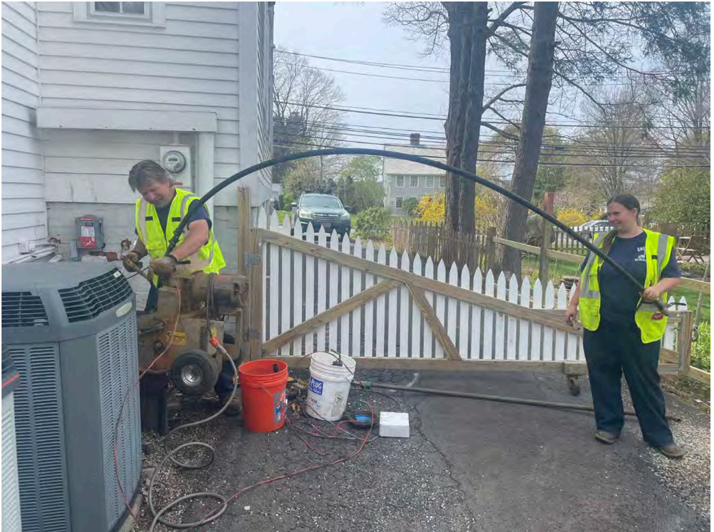
Picture 8: Grela pulling the pump from the well located at the 253 Main Street, Durham, property. View to the west.
