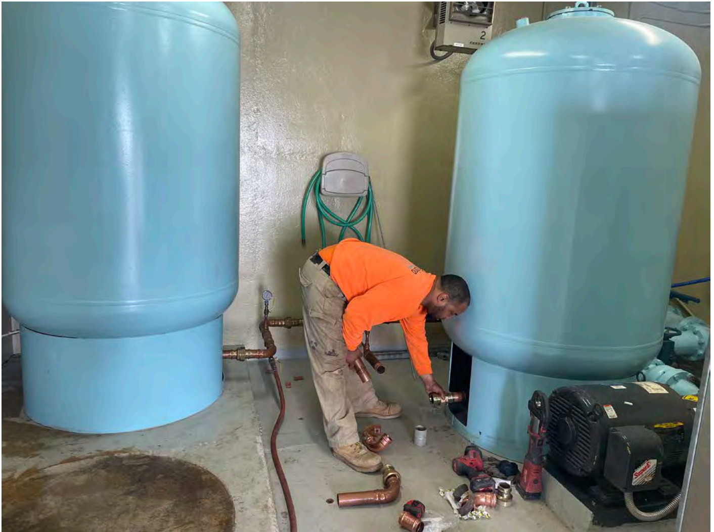
Picture 11: Fazzino working on connecting copper pipe to one of the expansion tanks that Ludlow moved inside of the Long Hill pump station this morning. View to the south.
