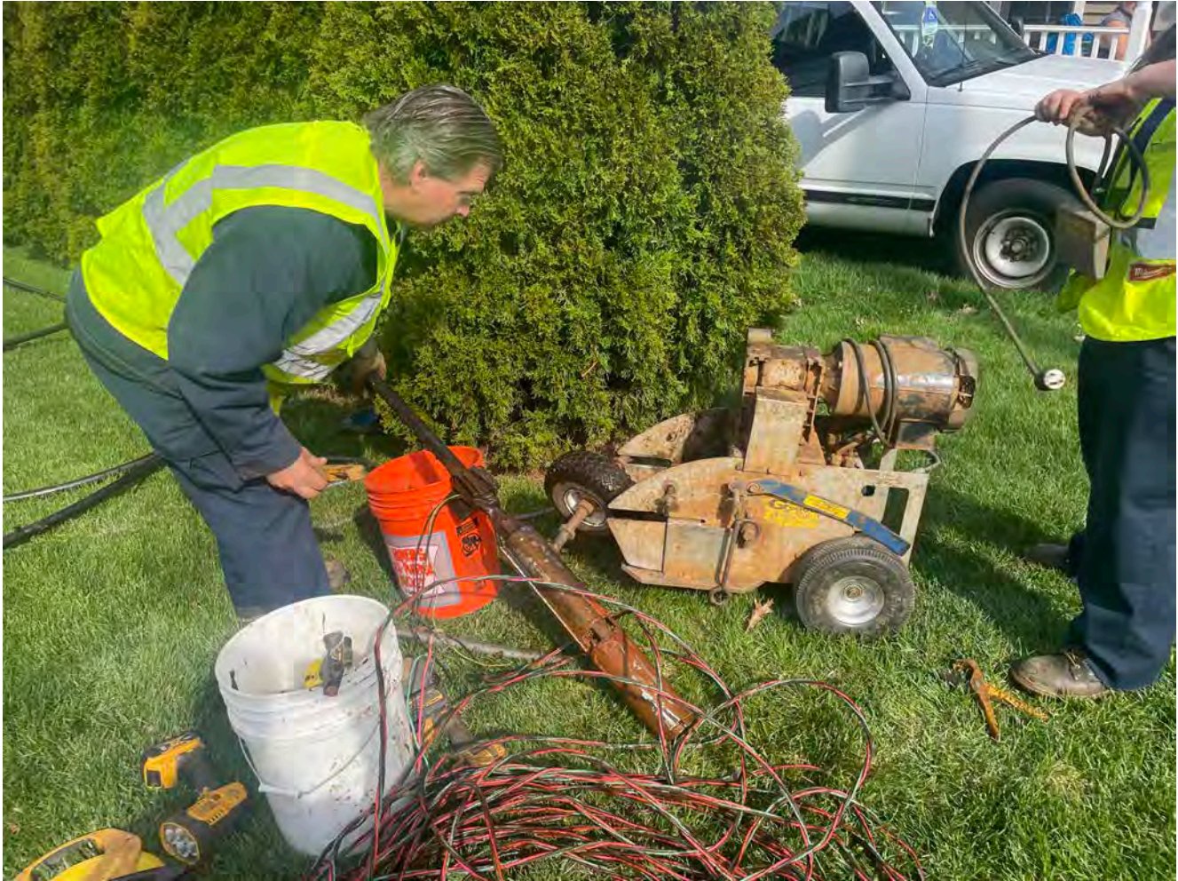
Picture 5: Grela having just pulled the pump from the well located at the 166 Maple Avenue, Durham, property. View to the northwest.
