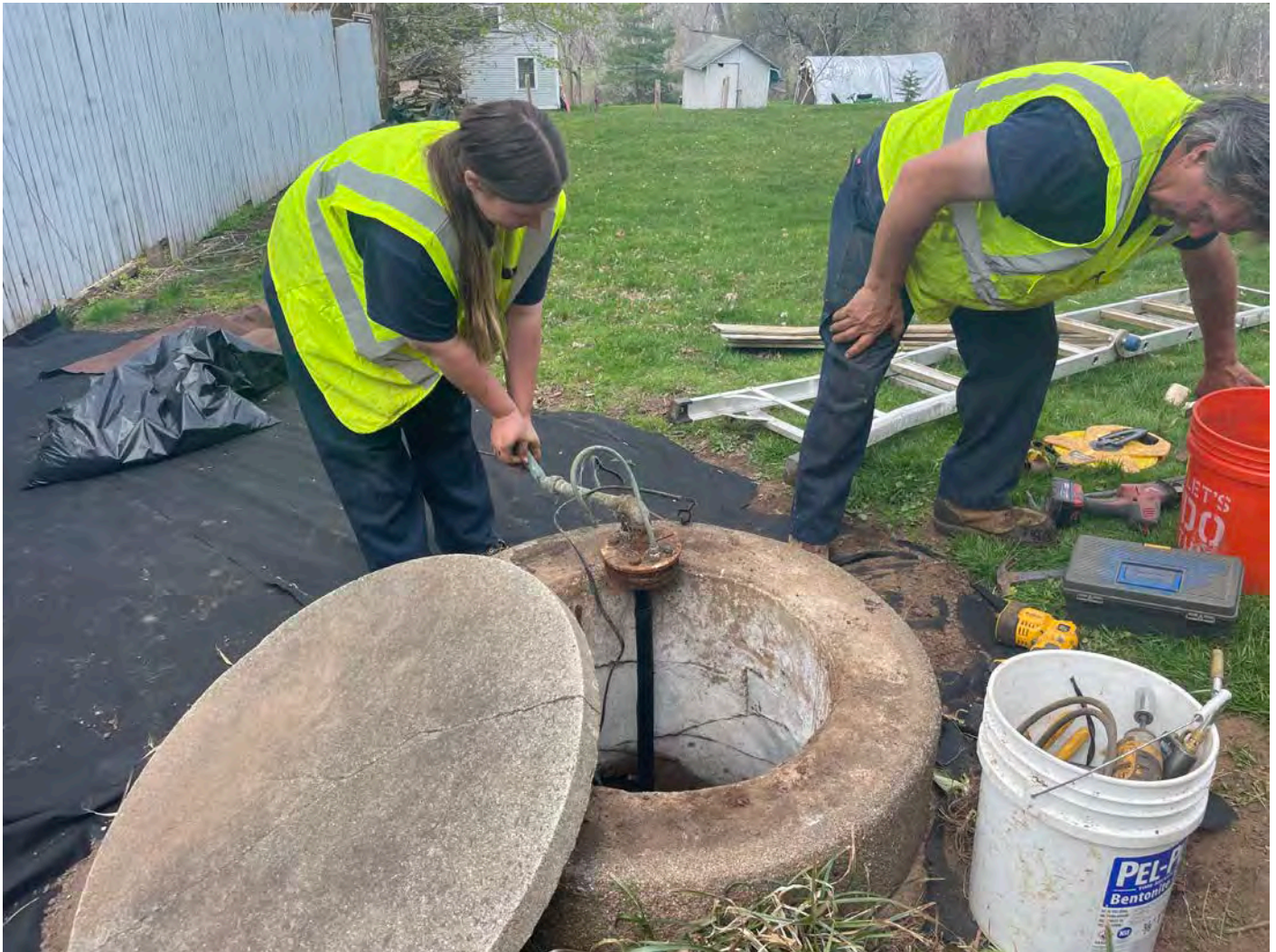
Picture 4: Grela pulling the pump from the well located at the 158 Maple Avenue, Durham, property. View to the west.
