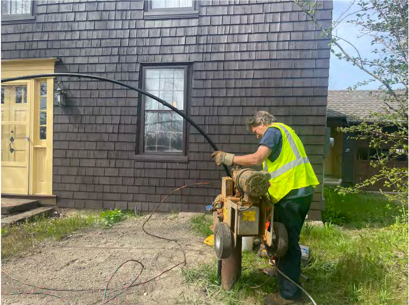
Picture 1: Grela pulling the pump from the well located at the 25 Talcott Lane, Durham, residence. View to the north.
