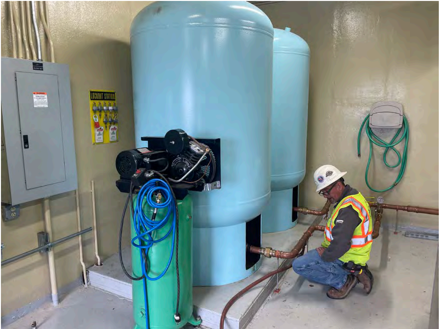
Picture 10: Ludlow assessing how to move the two expansion tanks located at the southeast corner of the Long Hill pump station in Middletown. View to the southeast.
