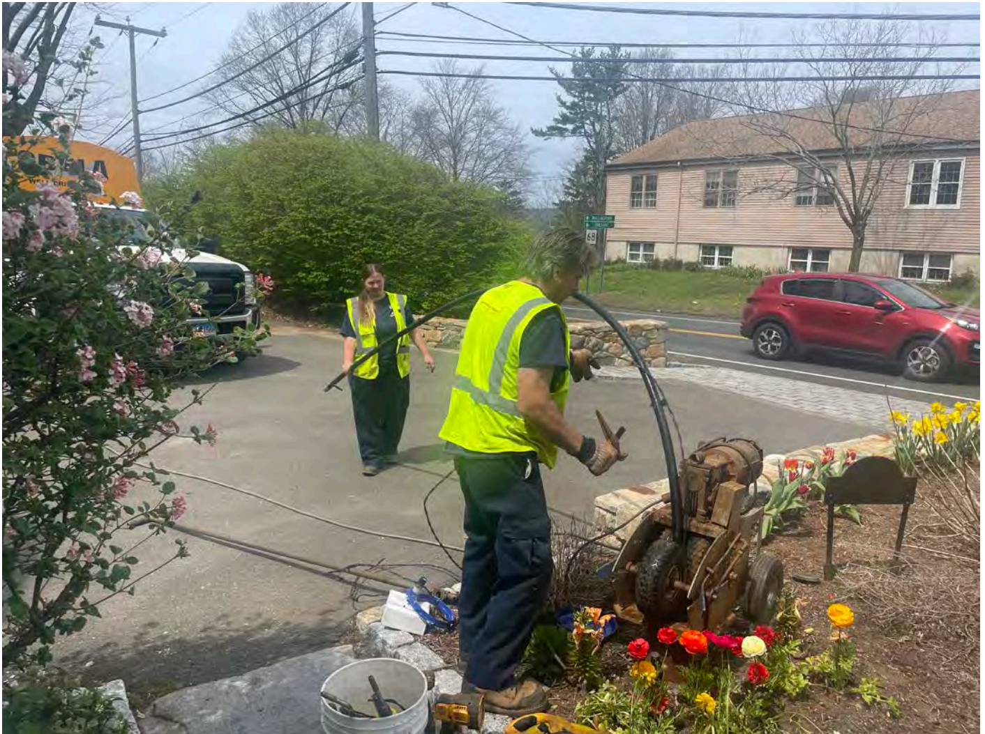
Picture 7: Grela pulling the pump from the well located at the 220 Main Street, Durham, property. View to the northwest.
