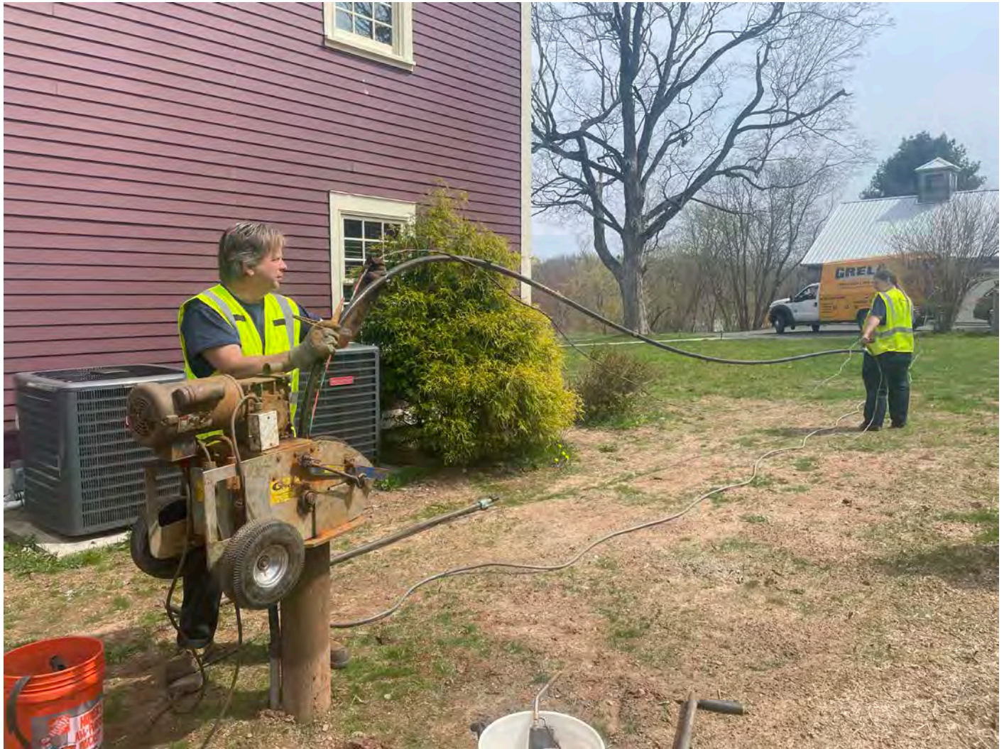
Picture 2: Grela pulling the pump from the well located at the 35 Maiden Lane, Durham, residence. View to the south.
