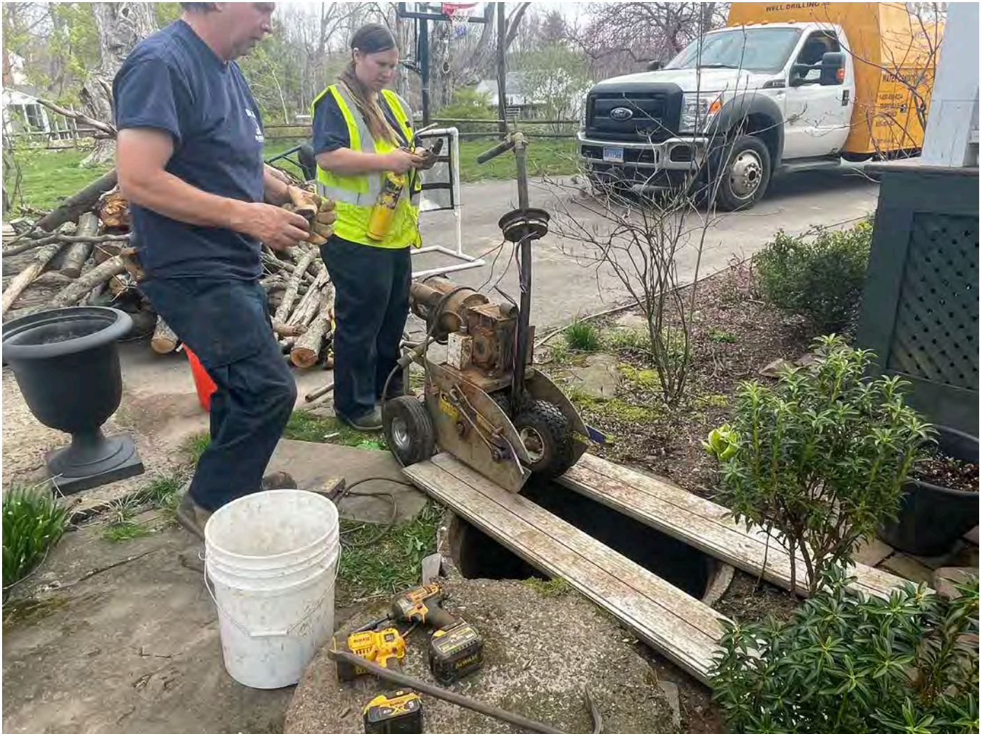
Picture 9: Grela pulling the pump from the well located at the 254 Maple Avenue, Durham, property. View to the northeast.
