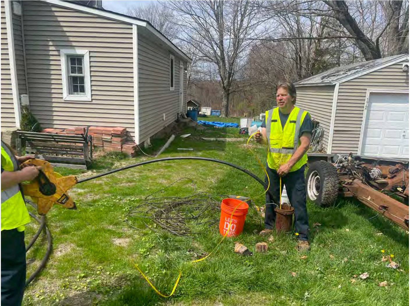
Picture 6: Grela pulling the pump from the well located at the 172 Maple Avenue, Durham, residence. View to the west.
