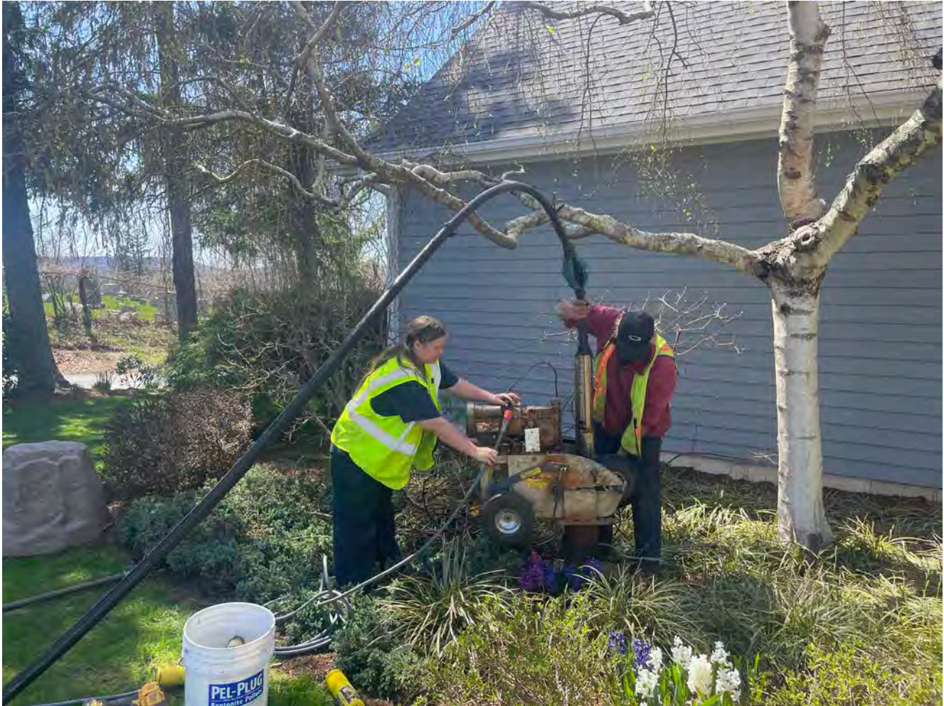
Picture 1: Grela pulling the well pump from the well located at the 29 Maple Avenue, Durham, residence. View to the southwest.
