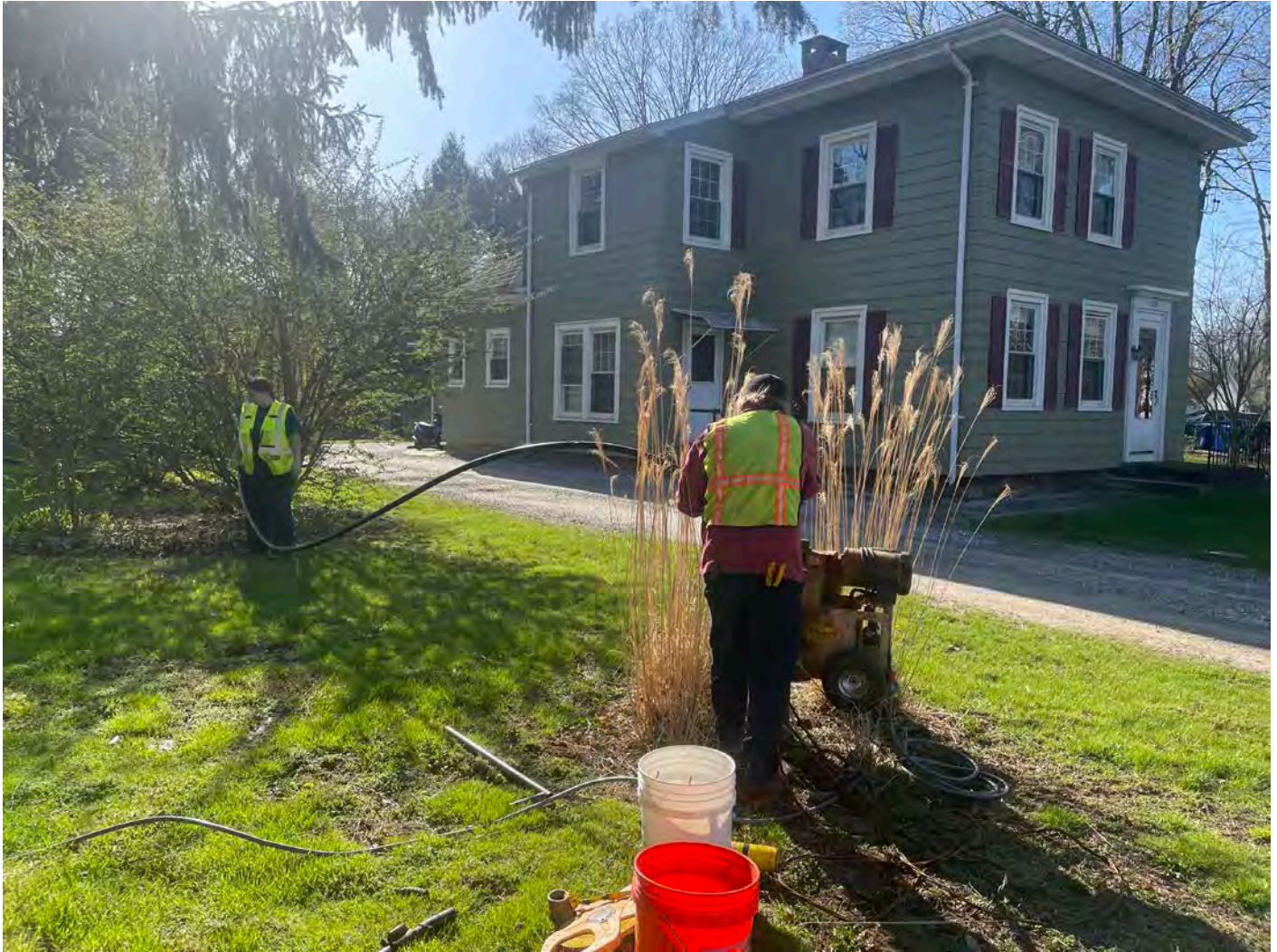
Picture 7: Grela pulling the well pump from the well located at the 307 Main Street, Durham, property. View to the southeast.
