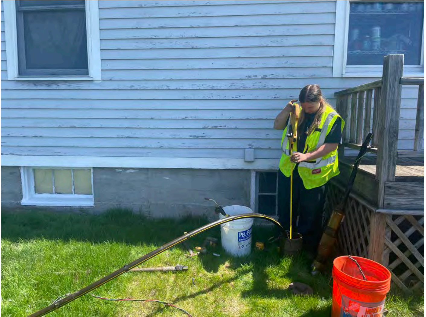
Picture 2: Grela pulling the well pump from the well located at the 47 Wallingford Road, Durham, residence. View to the northwest.
