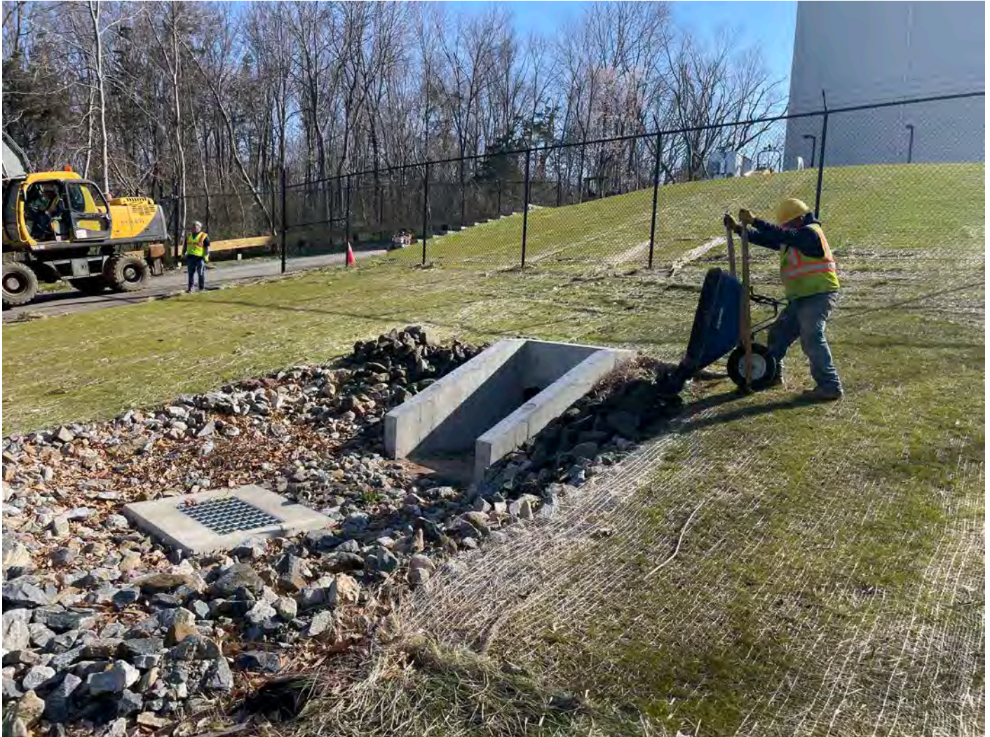
Picture 9: Ludlow in the process of placing additional rock on the east side of the catch basin plunge bowl located at ~Station 11+80 on the Shared Access Driveway, in Middletown. View to the northeast.
