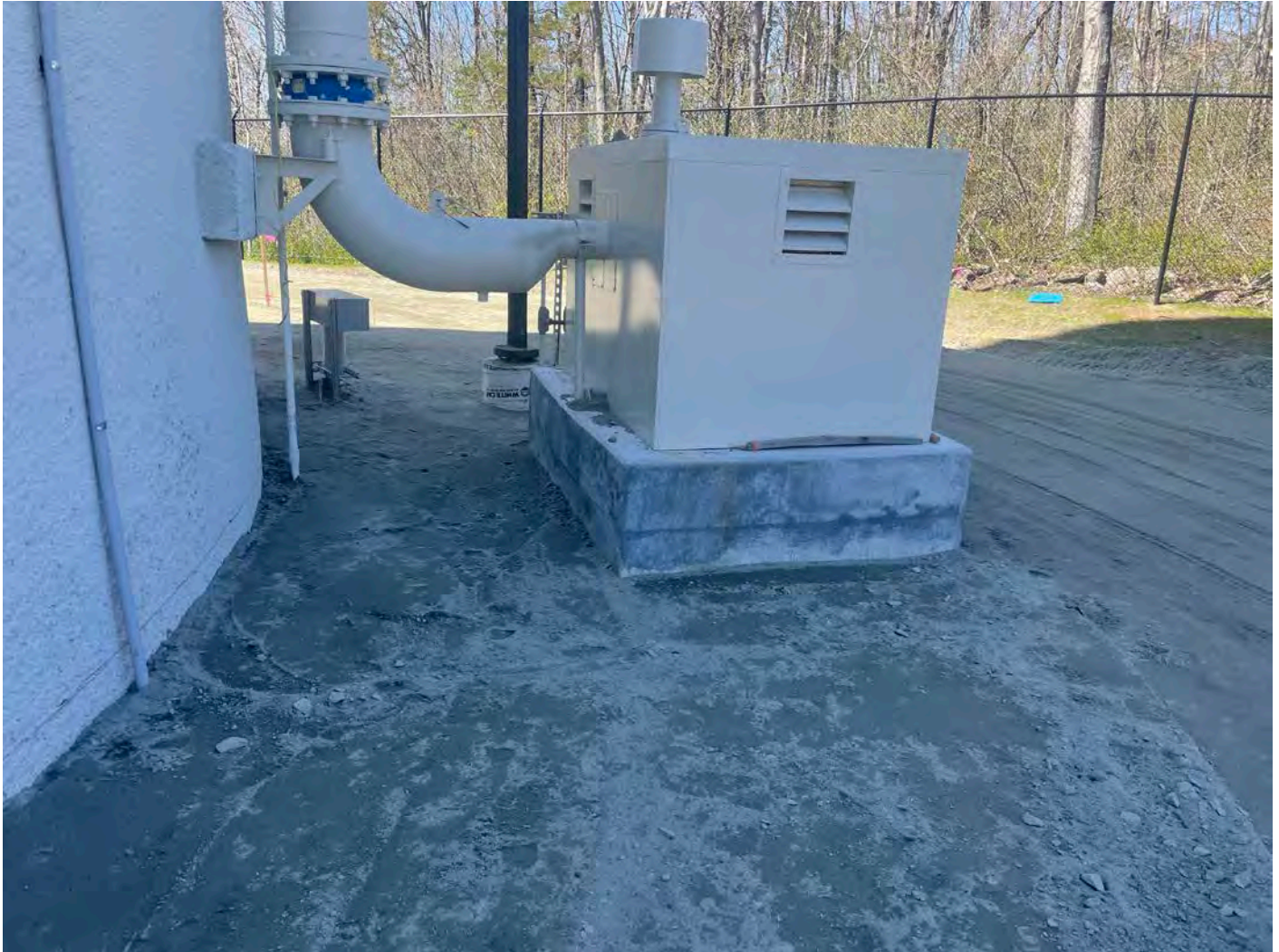
Picture 12: Blower enclosure located on the northeast side of the water tank east of the Shared Access Driveway in Middletown where Ludlow has placed and compacted fill around the blower base. View to the northwest.
