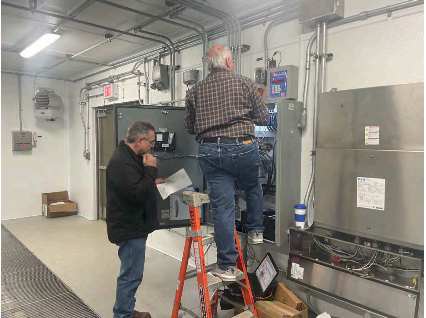
Picture 11: Knapp Engineering working on programming the autodialer at the booster station located at Station 750+43 on S. Main Street in Middletown. View to the northwest.
