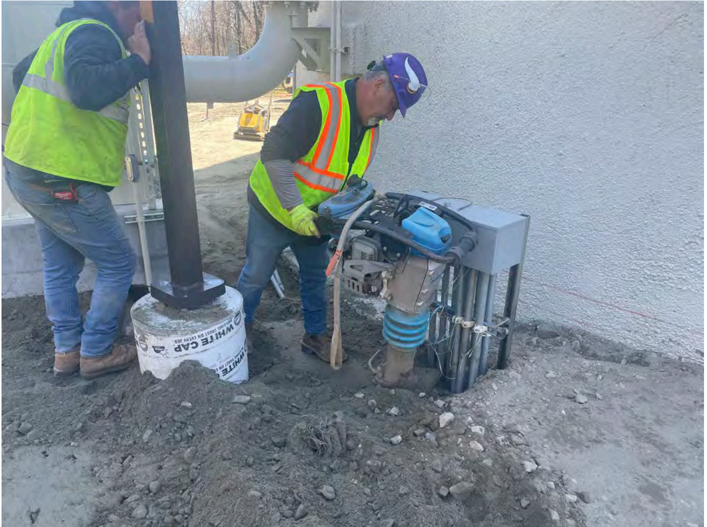
Picture 10: Ludlow using a jumping jack to compact fill on the northeast side of the water tank located to the east of the Shared Access Driveway, in Middletown. View to the southeast.
