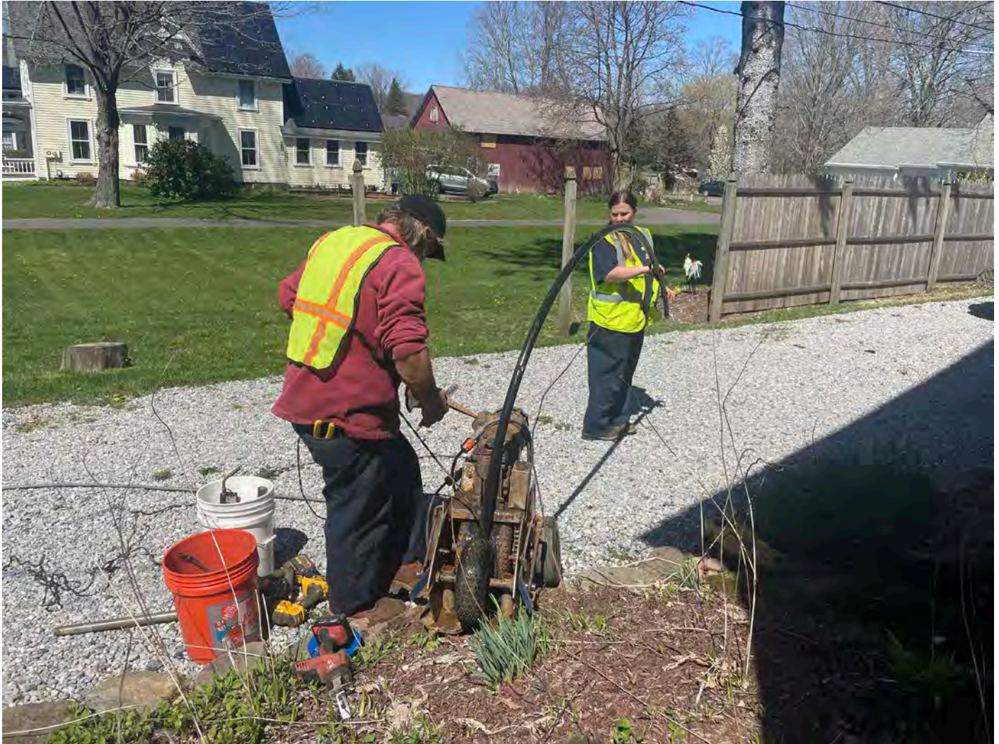
Picture 6: Grela pulling the well pump from the well located at the 257 Main Street, Durham, residence. View to the northeast.
