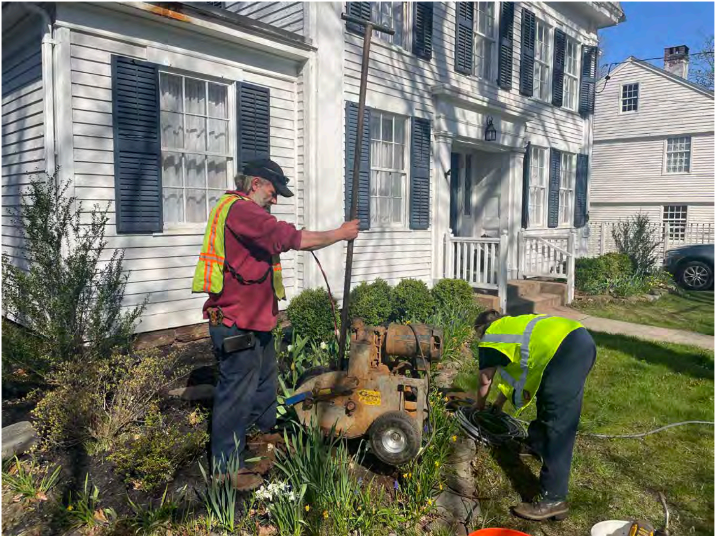
Picture 4: Grela pulling the well pump from the well located at the 246 Main Street, Durham, property. View to the northwest.
