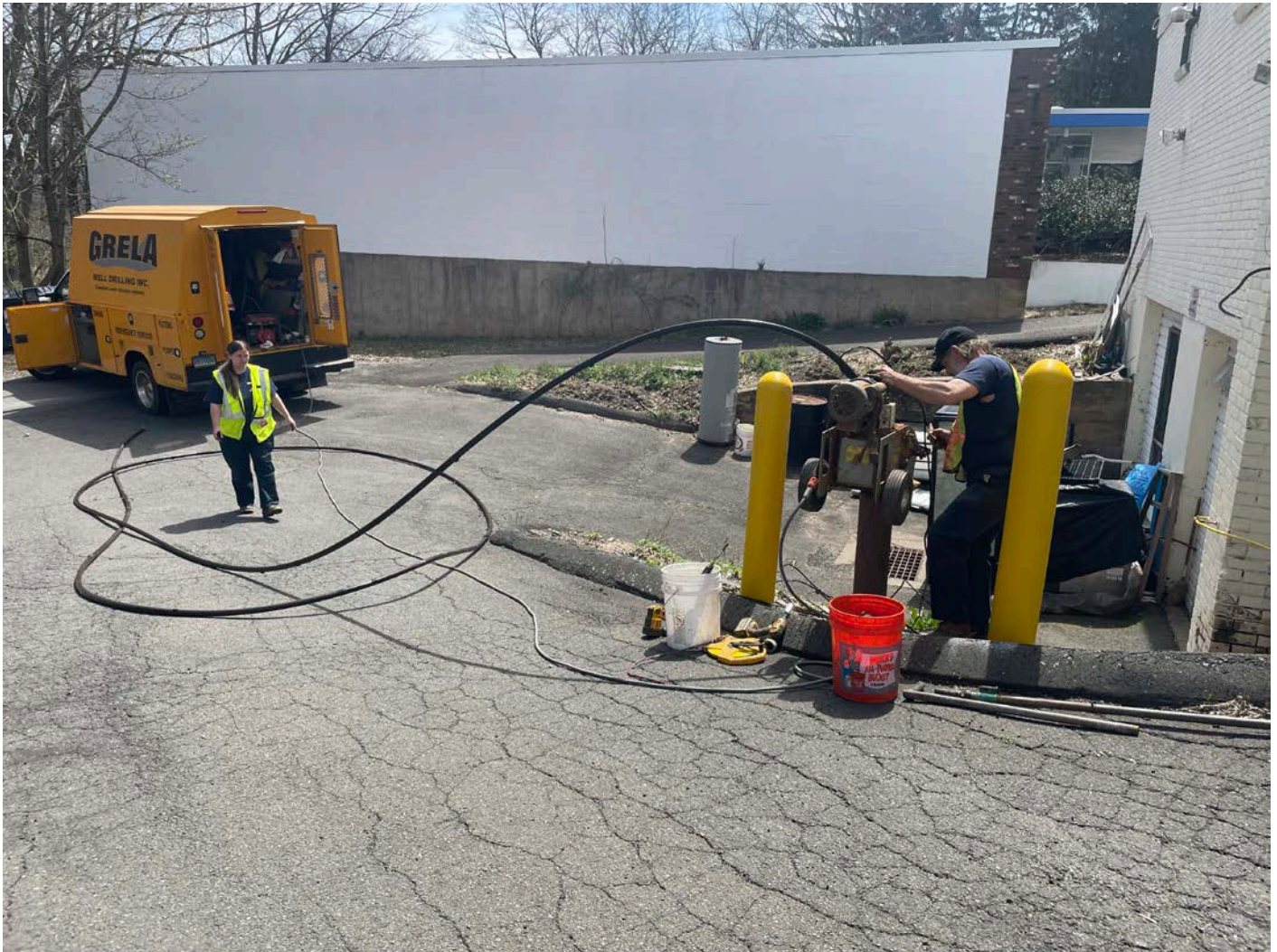
Picture 7: Grela pulling the well pump from the well located at the 325 Main Street, Durham, property. View to the southeast.
