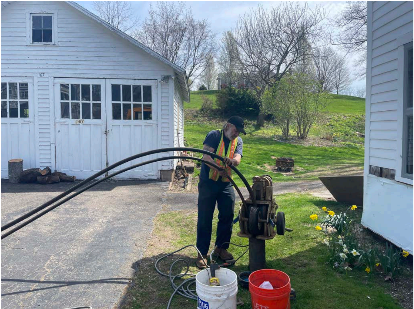
Picture 1: Grela pulling the well pump from the well located at the 167 Main Street, Durham, residence. View to the east.
