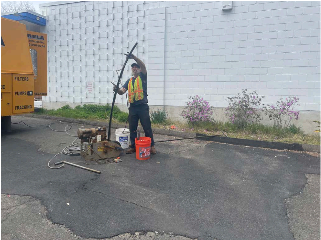
Picture 5: Grela pulling the well pump from the well located at the 321 Main Street, Durham, property. View to the northwest.
