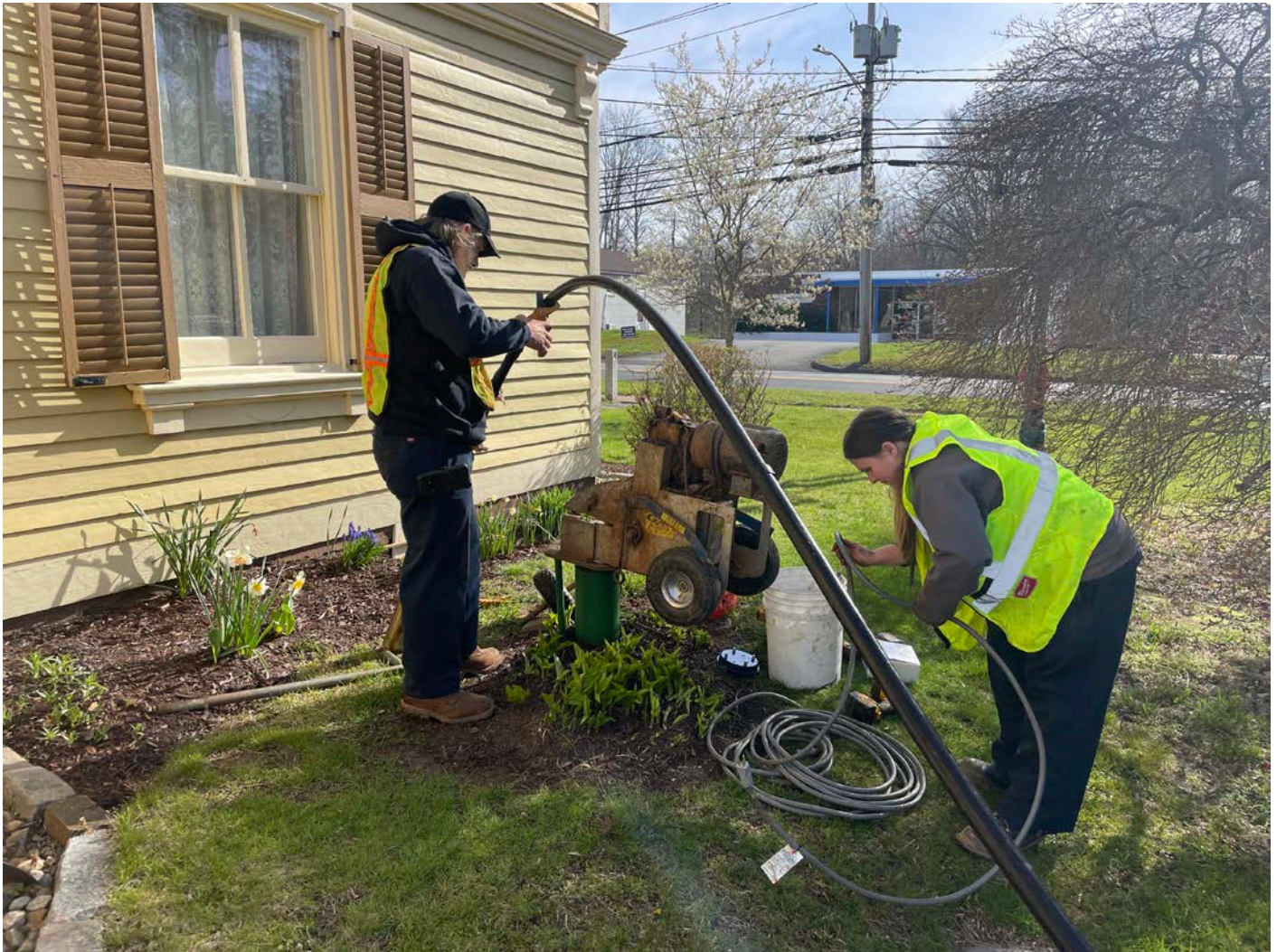
Picture 6: Grela pulling the well pump from the well located at the 322 Main Street, Durham, residence. View to the east.
