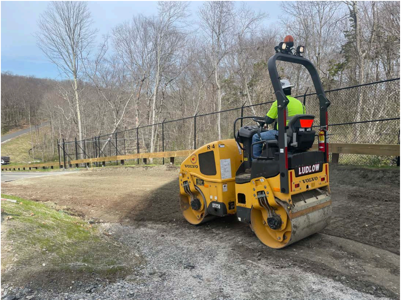
Picture 10: Ludlow using a rolling compactor on fill on the Shared Access Driveway, in Middletown, immediately north of the electrical enclosure. View to the northwest.
