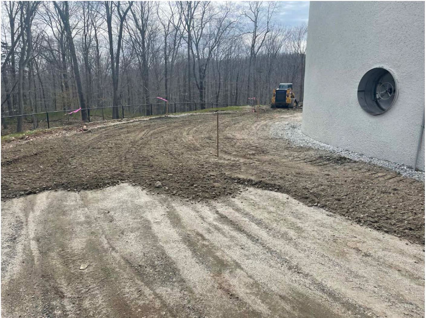
Picture 13: Processed stone that Ludlow placed on the south side of the water tank located east of the Shared Access Driveway in Middletown. View to the west/southwest.
