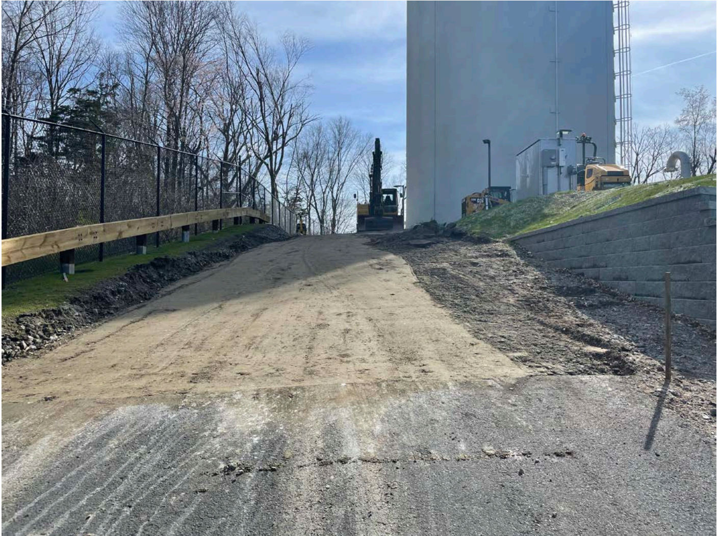
Picture 9: Ludlow in the process of compacting the fill where they removed pavement from Station 11+15 eastwards on the Shared Access Driveway, in Middletown. View to the east.
