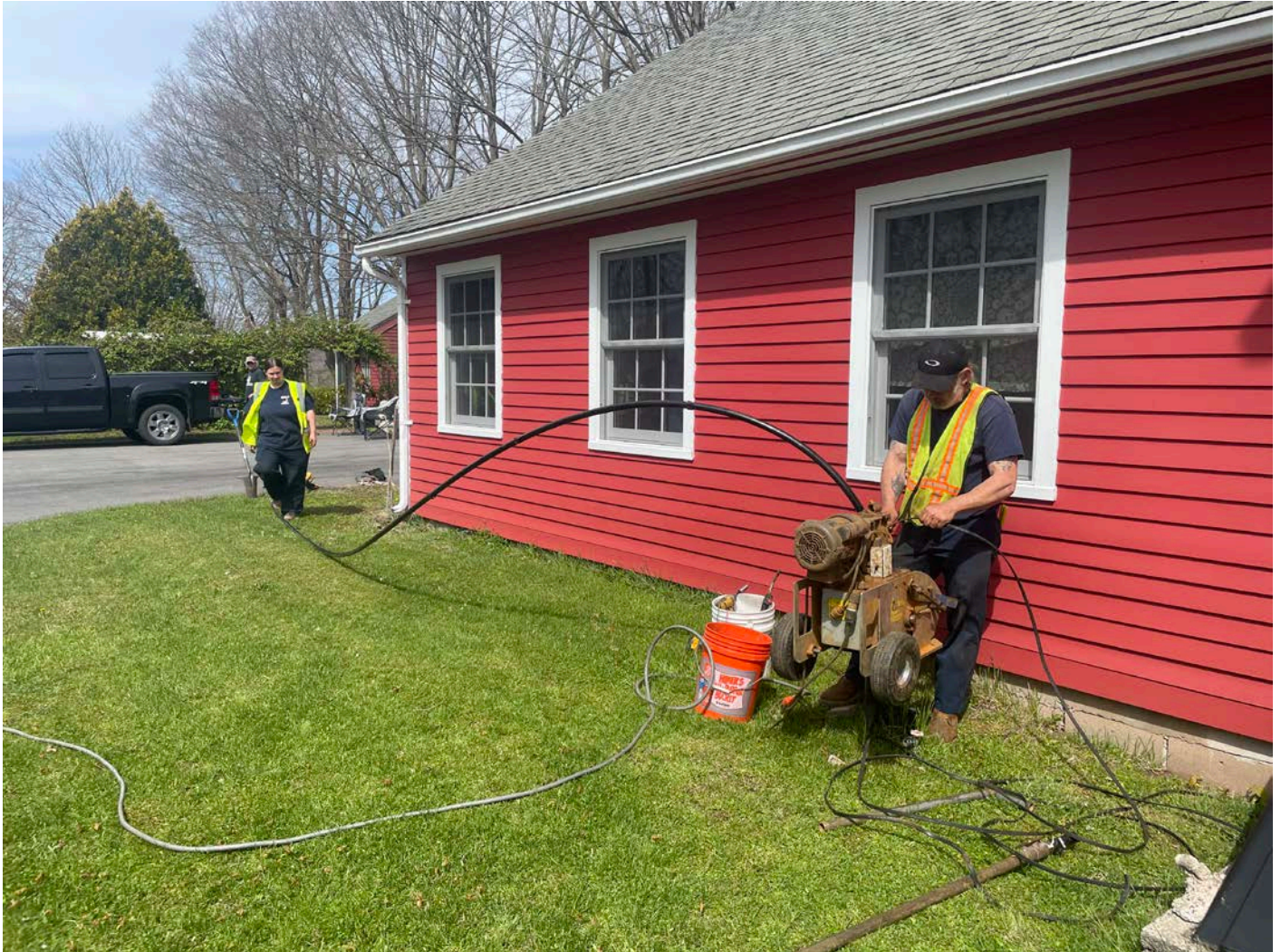
Picture 2: Grela pulling the well pump from the well located at the 216 Main Street, Durham, residence. View to the northwest.
