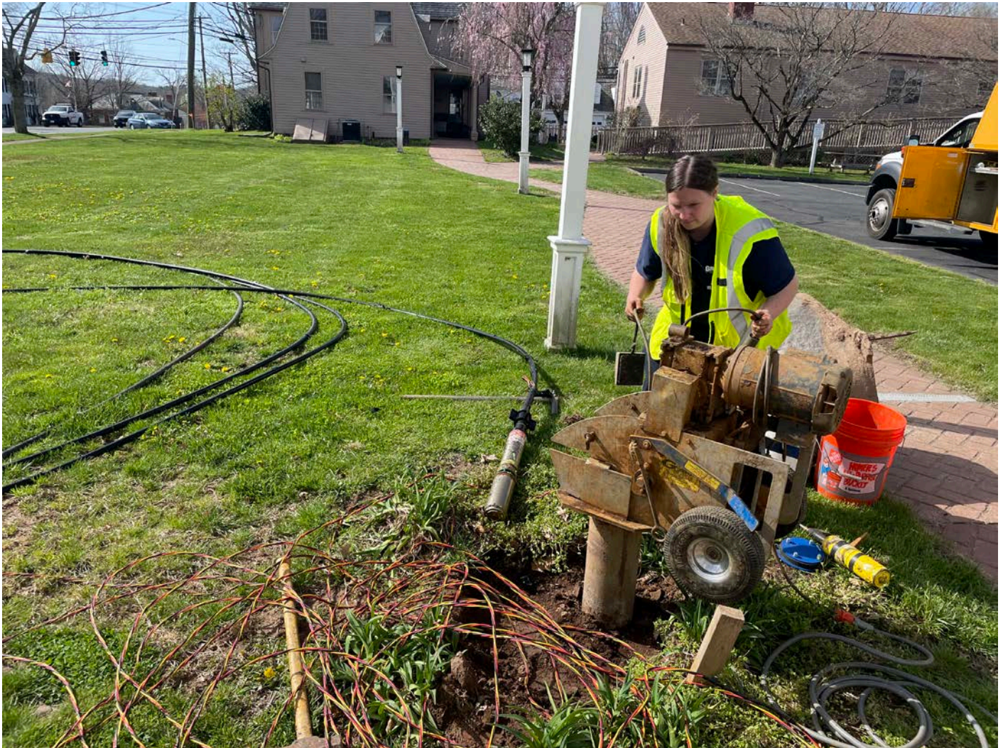
Picture 4: Grela pulling the well pump from the well located at the 236 Main Street, Durham, property. View to the south.
