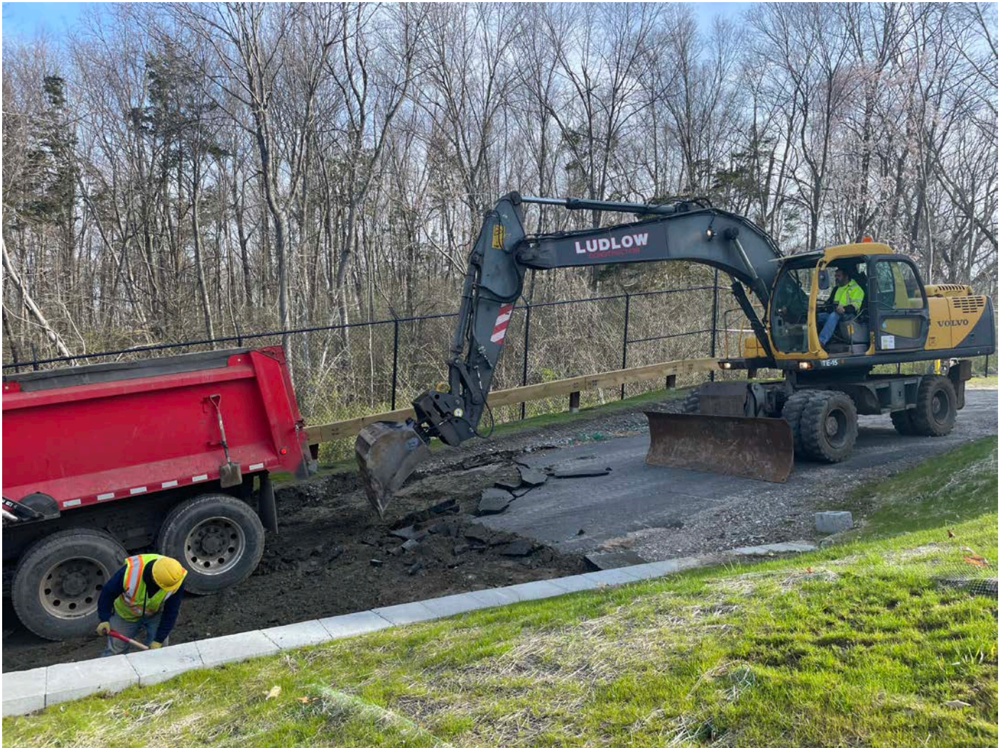
Picture 8: Ludlow removing asphalt from the tank driveway, east of Station 11+15 on the Shared Access Driveway in Middletown. View to the southeast.
