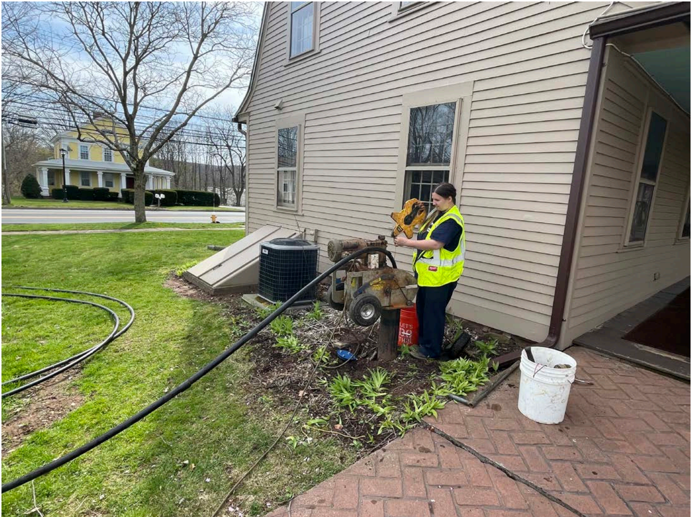
Picture 3: Grela pulling the well pump from the well that services the buildings located at 228 and 228R Main Street, Durham. View to the southeast.
