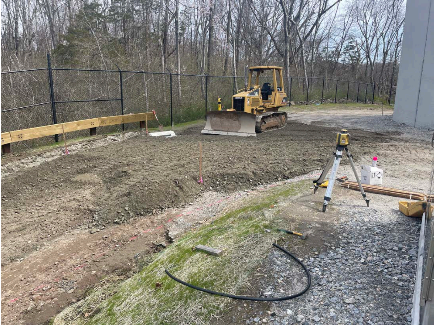
Picture 11: Ludlow grading processed stone they just placed on the northwest side of the water tank located east of the Shared Access Driveway in Middletown. View to the east.
