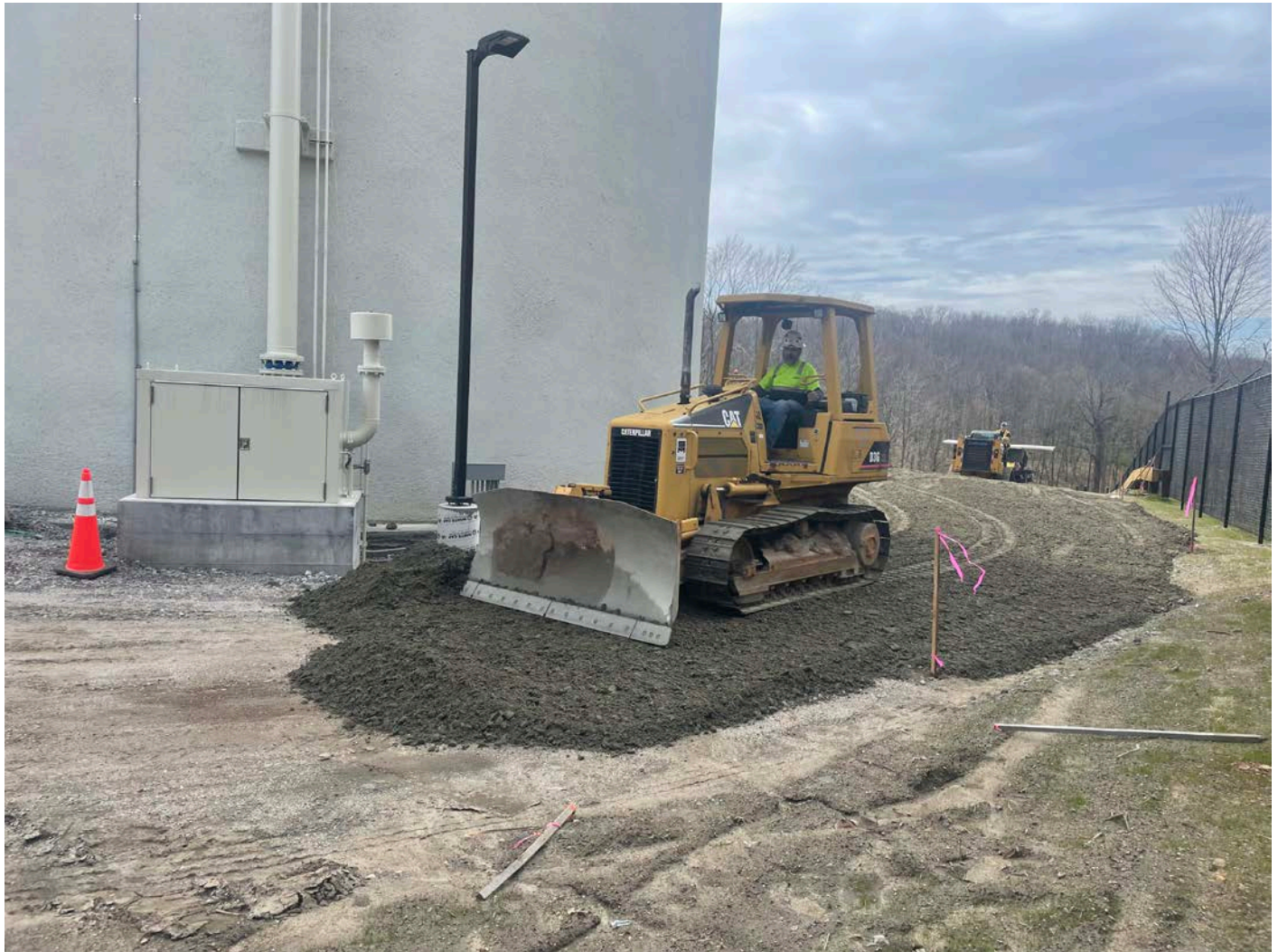
Picture 12: Ludlow grading processed stone they just placed on the northeast side of the water tank located east of the Shared Access Driveway in Middletown. View to the west.
