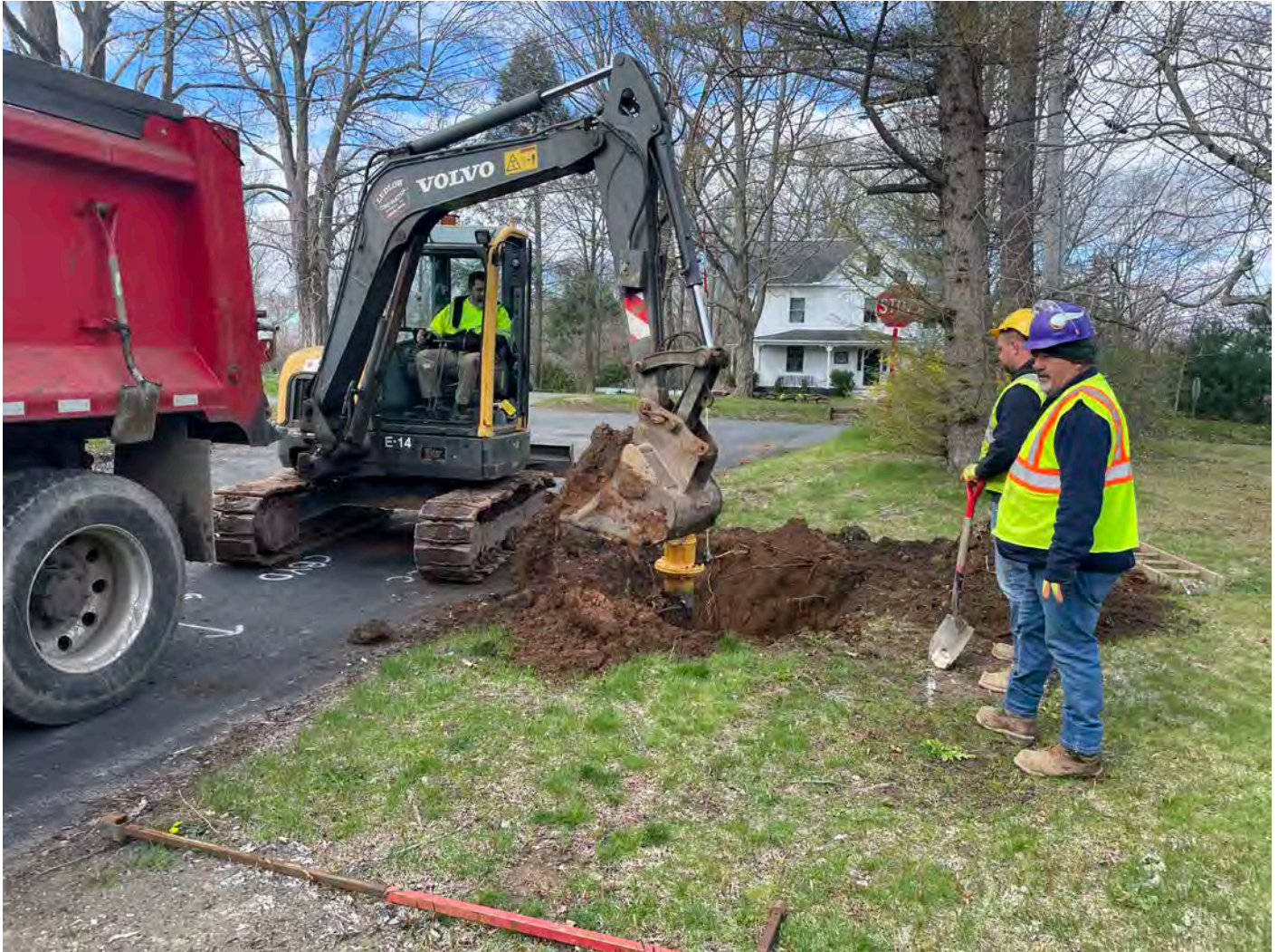
Picture 11: Ludlow excavating around the stem of the hydrant located at Station 305+41 on Talcott Lane, Durham. View to the west.
