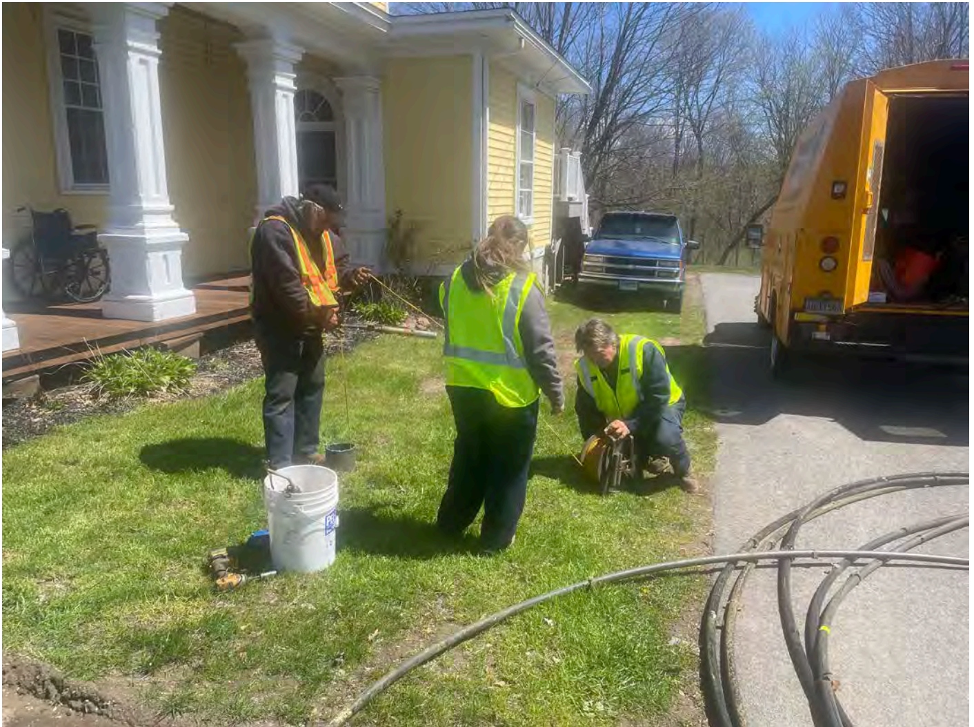
Picture 2: Grela pulling the well pump from the well located at the 227 Main Street, Durham, residence. View to the east.
