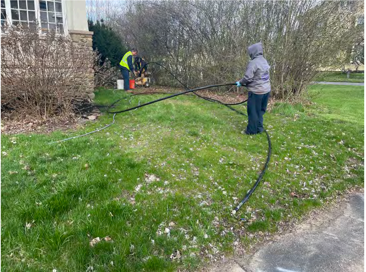
Picture 7: Grela pulling the well pump from the well located at the 316 Main Street, Durham, residence. View to the northwest.
