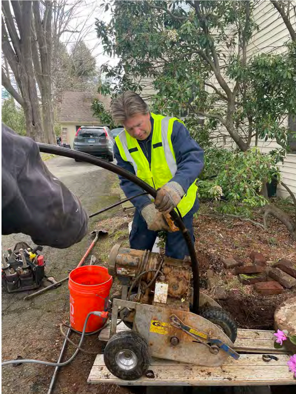
Picture 5: Grela pulling the well pump from the well located at the 297 Main Street, Durham, residence. View to the southeast.
