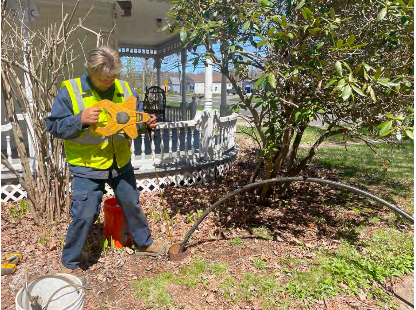
Picture 6: Grela pulling the well pump from the well located at the 312 Main Street, Durham, residence. View to the northeast.
