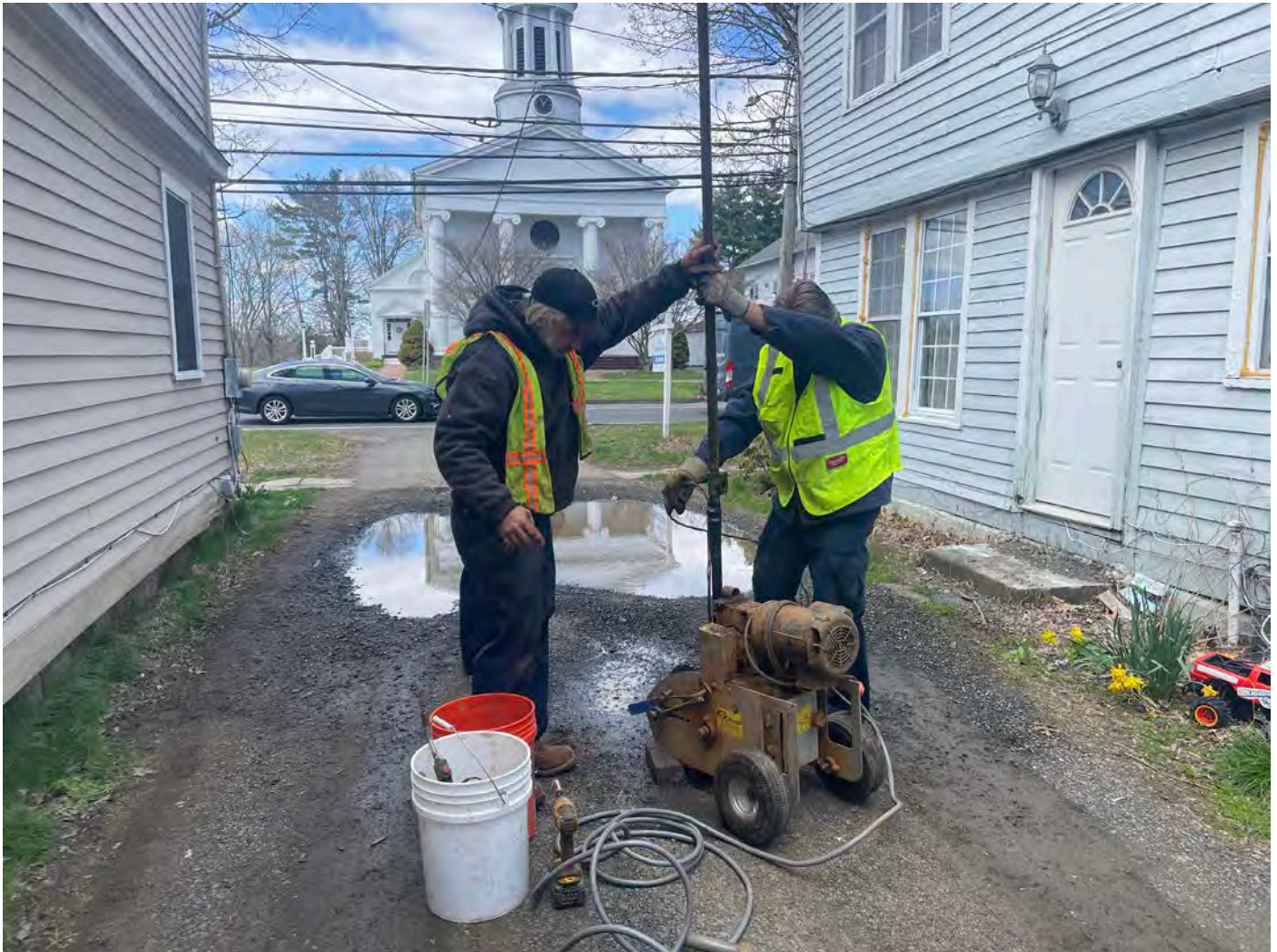
Picture 3: Grela pulling the well pump from the well located between the 233 and 235 Main Street, Durham, residences (which both share the same well). View to the west.
