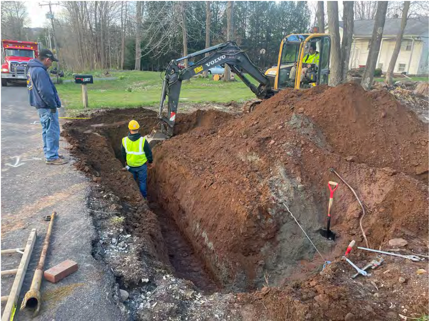
Picture 8: Ludlow excavating a trench as they work to move an existing curb stop located at Station 936+88 to Station 936+67 on Maple Avenue. View to the south.
