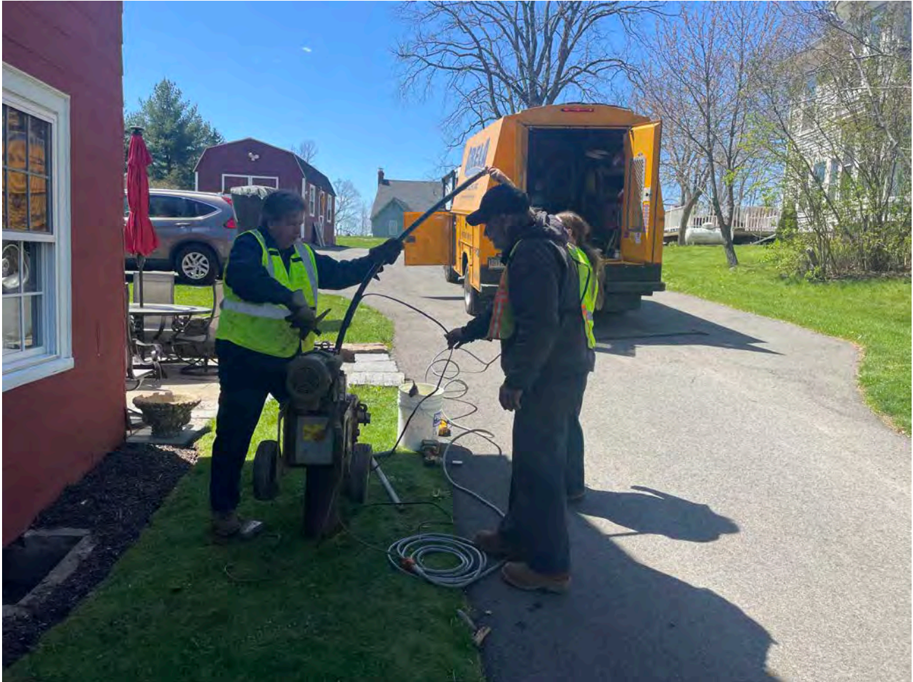
Picture 1: Grela pulling the well pump from the well located at the 186 Main Street, Durham, residence. View to the west.
