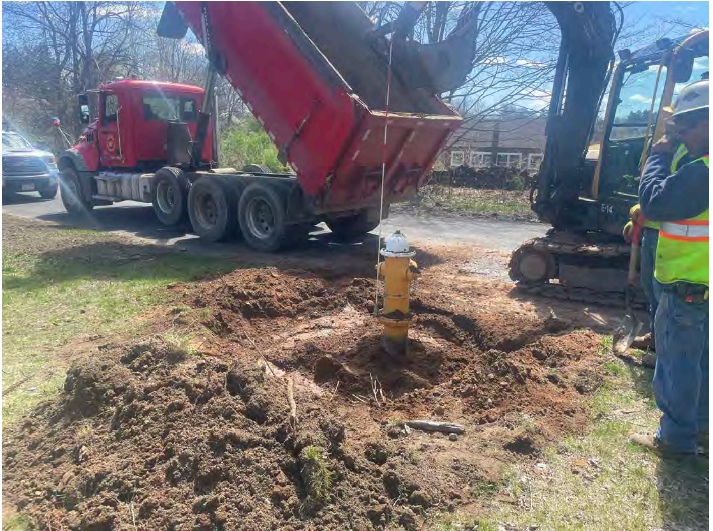
Picture 13: Ludlow has partially backfilled around the hydrant located at Station 305+41 on Talcott Lane, Durham. View to the west.
