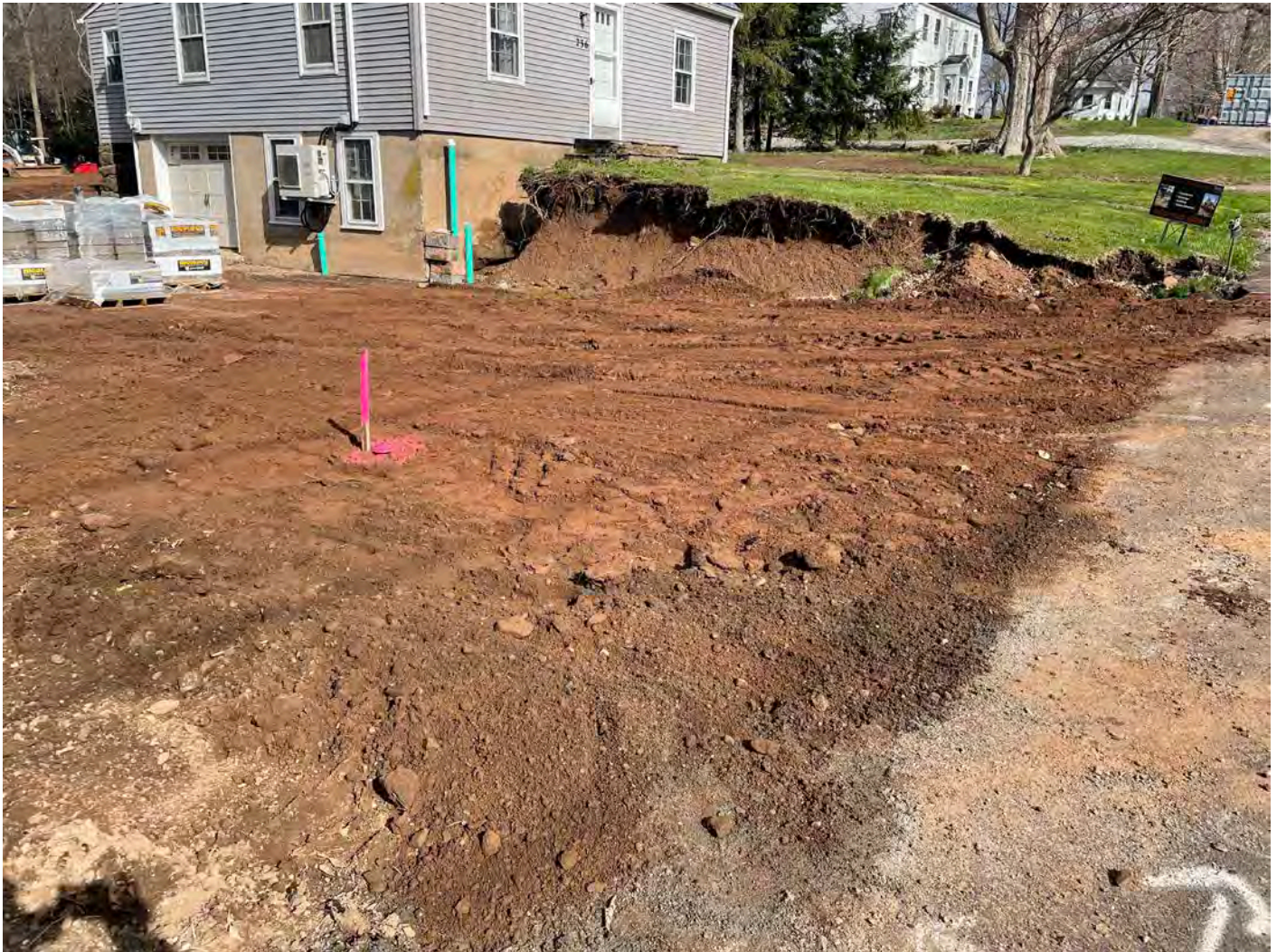
Picture 10: The area located on the west side of Maple Avenue after Ludlow moved a curb stop from Station 936+67 to Station 936+88. View to the northwest.
