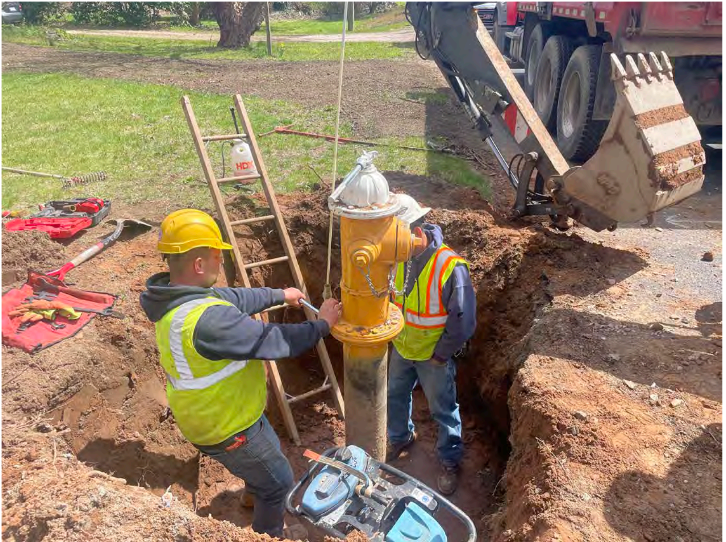
Picture 12: Ludlow working to straighten the stem of the hydrant located at Station 305+41 on Talcott Lane, Durham. View to the east.
