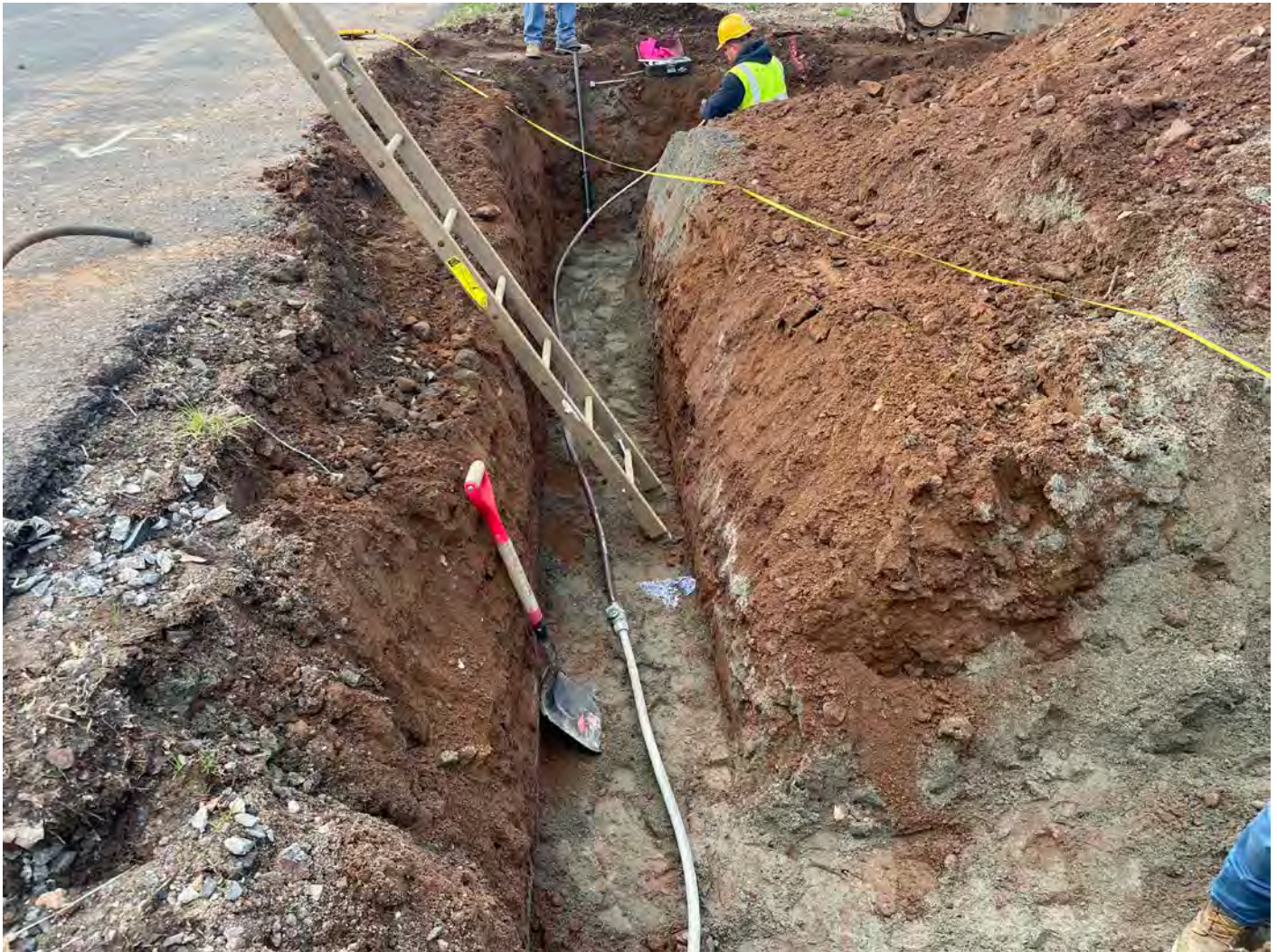
Picture 9: Ludlow in the process of moving the curb stop formerly located at Station 936+88 to Station 936+67 on Maple Avenue, Durham. Ludlow has laid out 1" copper water line over 6" of sand. View to the south.
