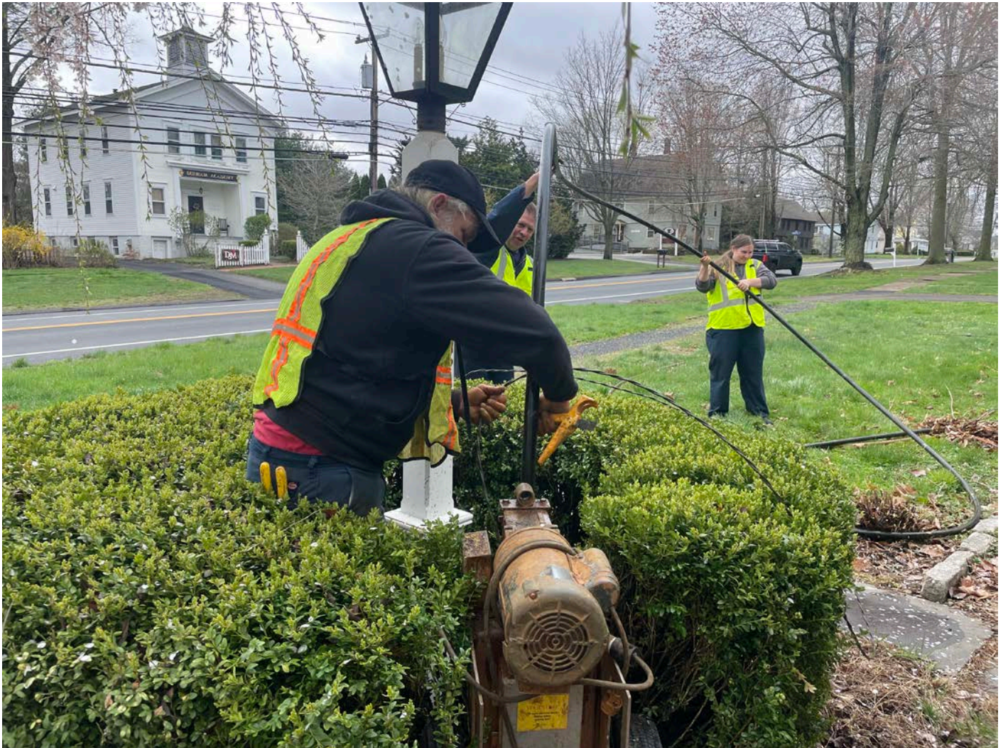
Picture 3: Grela pulling the well line and well pump from the well located at the 256 Main Street, Durham, residence. View to the southeast.
