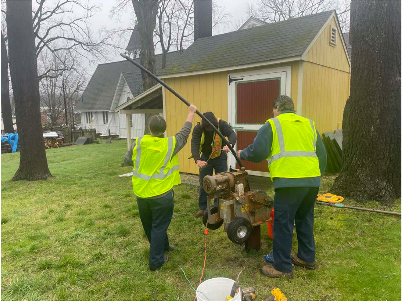
Picture 1: Grela pulling the well pump from the well located at the 202 Main Street, Durham, residence. View to the southeast.
