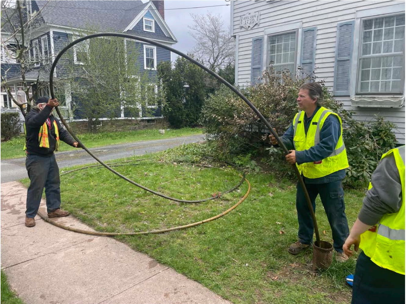
Picture 5: Grela pulling the well pump from the well located at the 267 Main Street, Durham, residence. View to the southeast.
