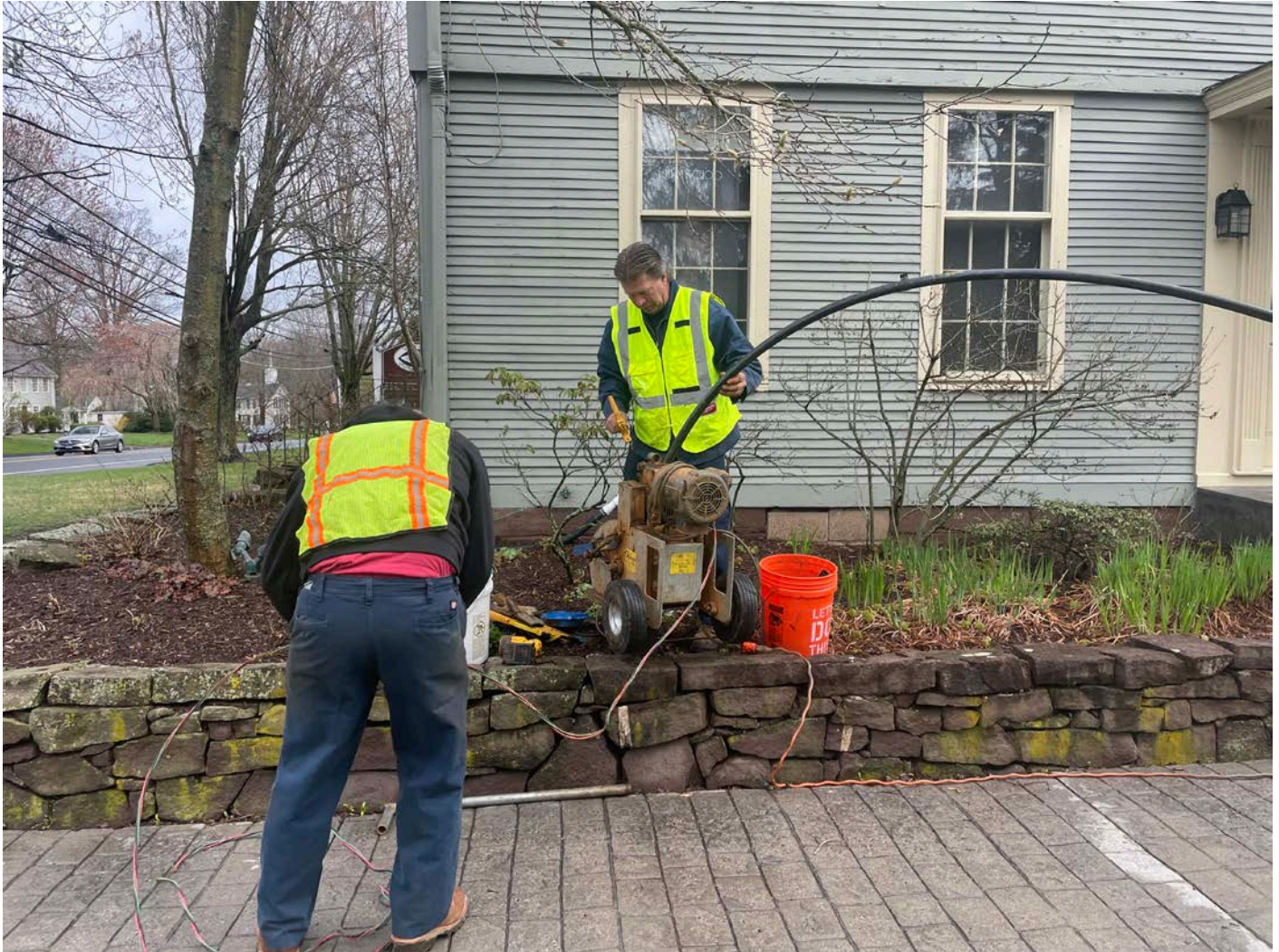
Picture 2: Grela pulling the well line and well pump from the well located at the 243 Main Street, Durham, residence. View to the north.
