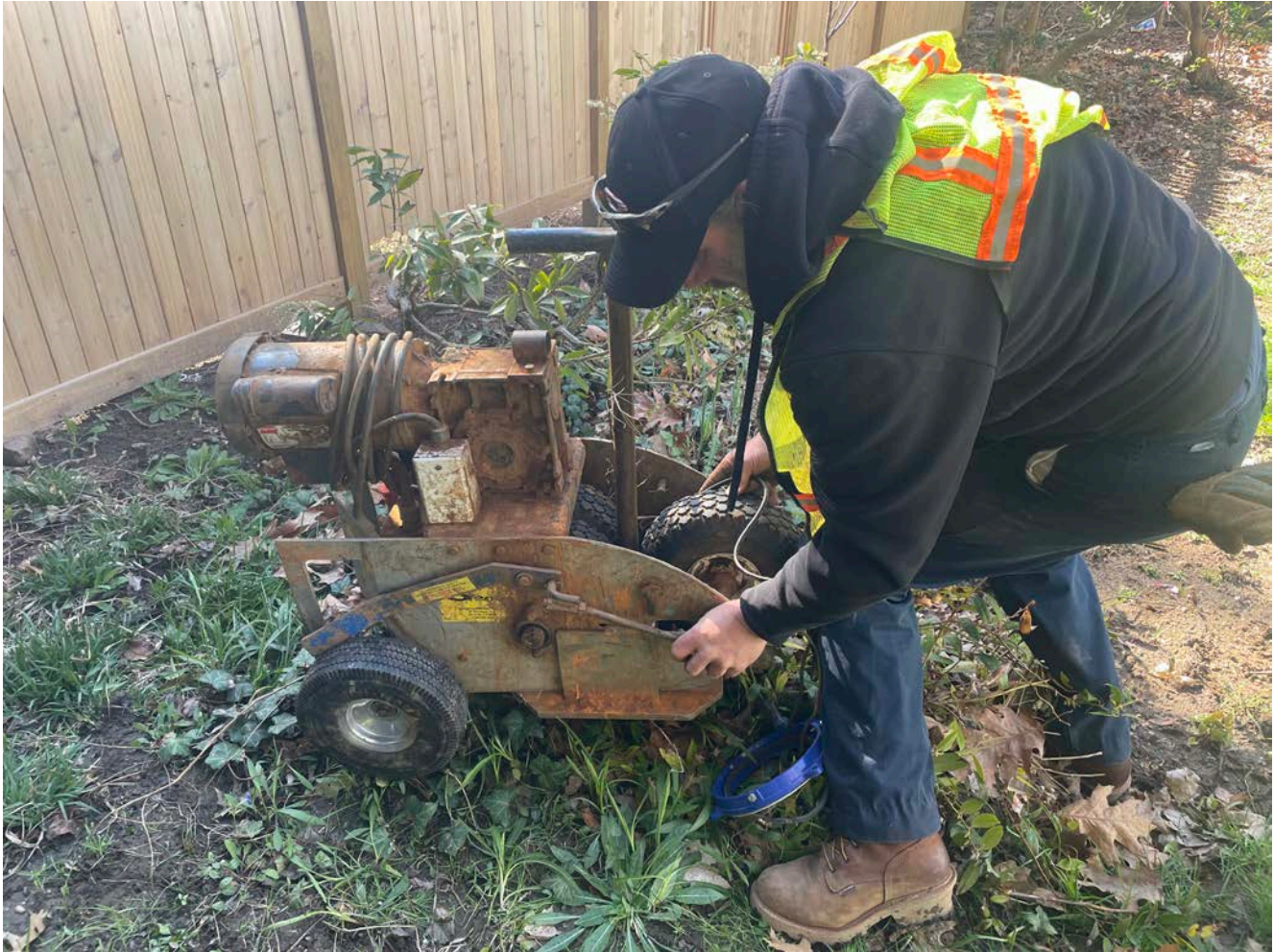
Picture 1: Grela setting up a machine that will pull the well line and well pump from the well located at the 239 Main Street, Durham, residence. View to the southeast.
