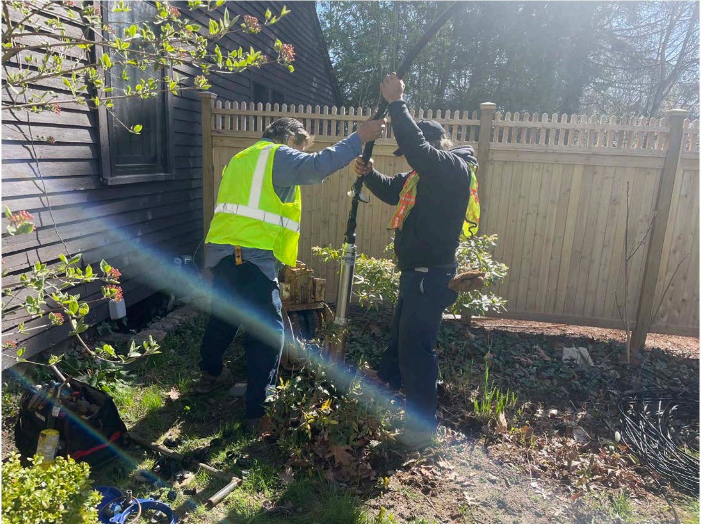
Picture 2: Grela pulling the well line and well pump from the well located at the 239 Main Street, Durham, residence. View to the east.
