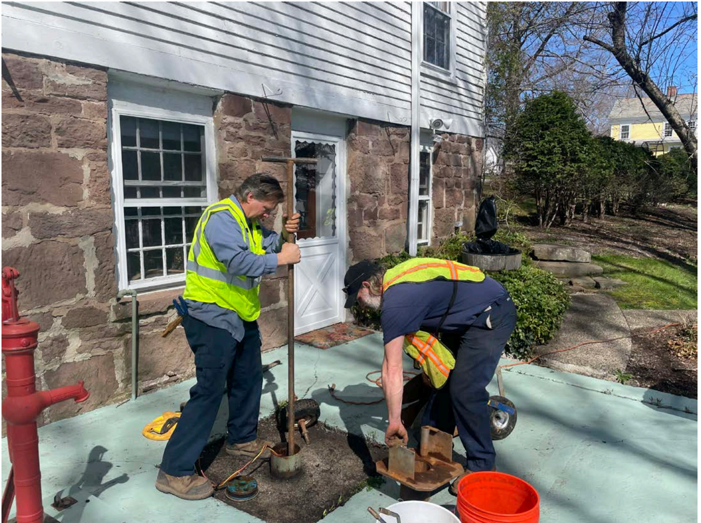
Picture 4: Grela setting up to pull the well line and well pump from the well located on the east side of the 215 Main Street, Durham, residence. View to the north.
