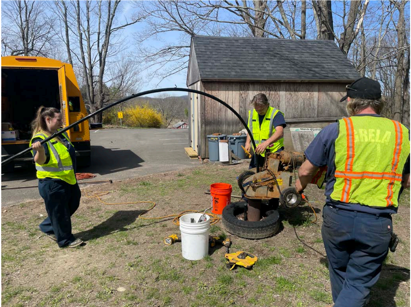
Picture 5: Grela pulling the well line and well pump from the well located at the 176 Main Street, Durham, residence. View to the west.
