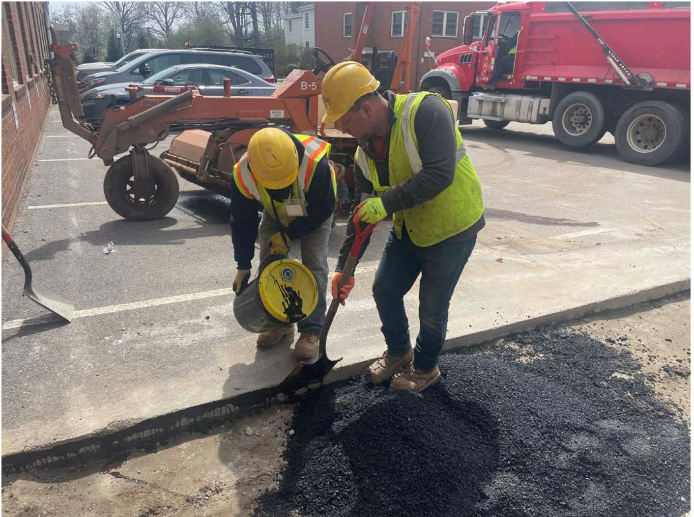
Picture 10: Ludlow placing tack coat on the cut edges of pavement on the trench footprint at the Durham Manufacturing property as they prepare to pave the trench. View to the south.
