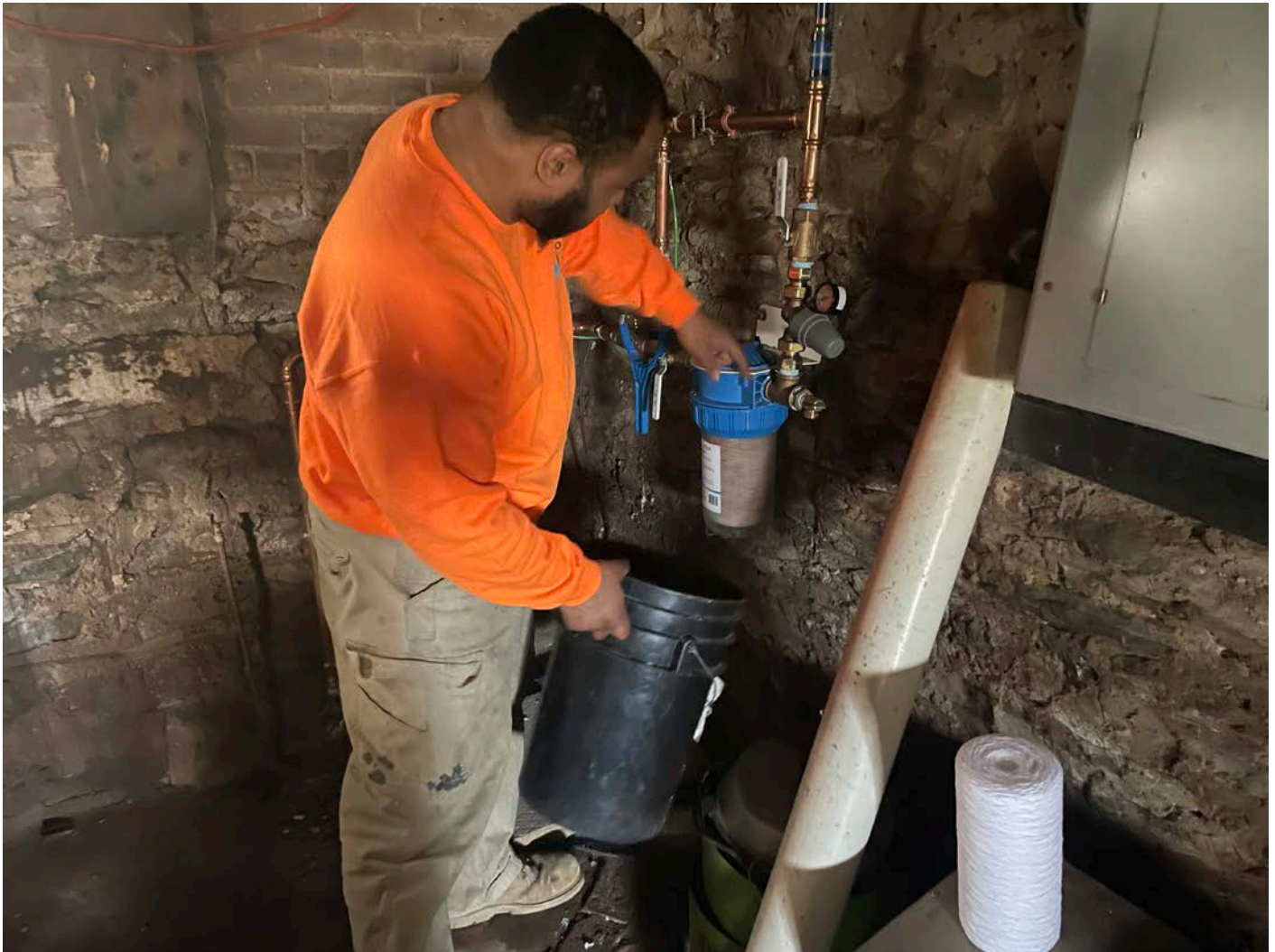
Picture 9: Fazzino changing out the water filter on the water system they recently installed at the 29 Maiden Lane, Durham, residence.
