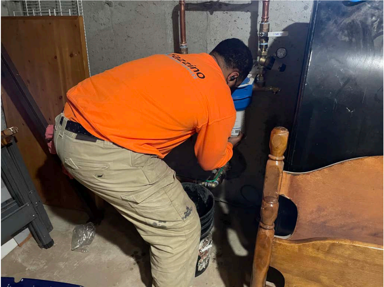
Picture 1: Fazzino changing out the water filter on the water system they recently installed at the 10 John's Way, Durham, residence.
