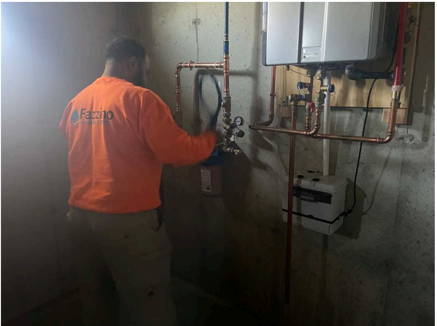
Picture 4: Fazzino changing out the water filter on the water system they recently installed at the 109 Maple Avenue, Durham, residence.
