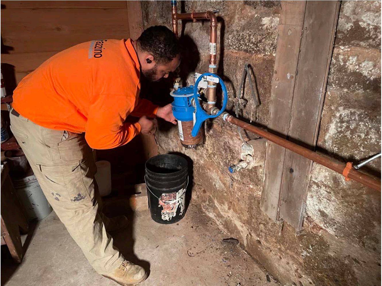
Picture 5: Fazzino changing out the water filter on the water system they recently installed at the 308 Main Street, Durham, residence.
