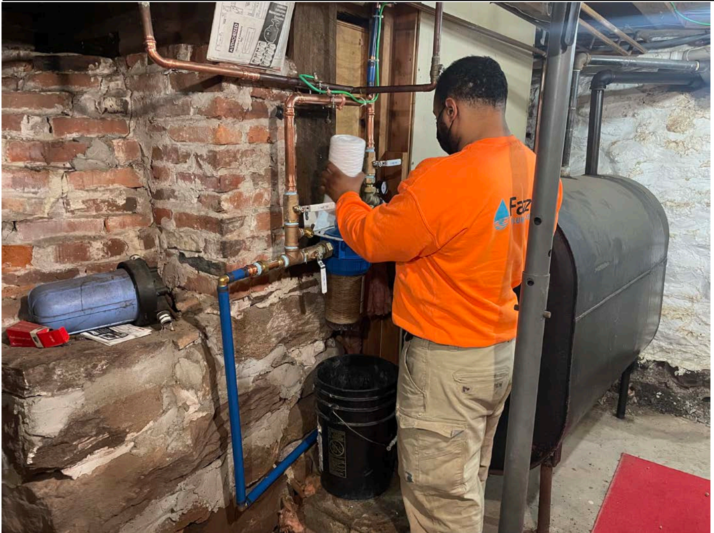
Picture 2: Fazzino changing out the water filter on the water system they recently installed at the 22 Wallingford Road, Durham, residence.
