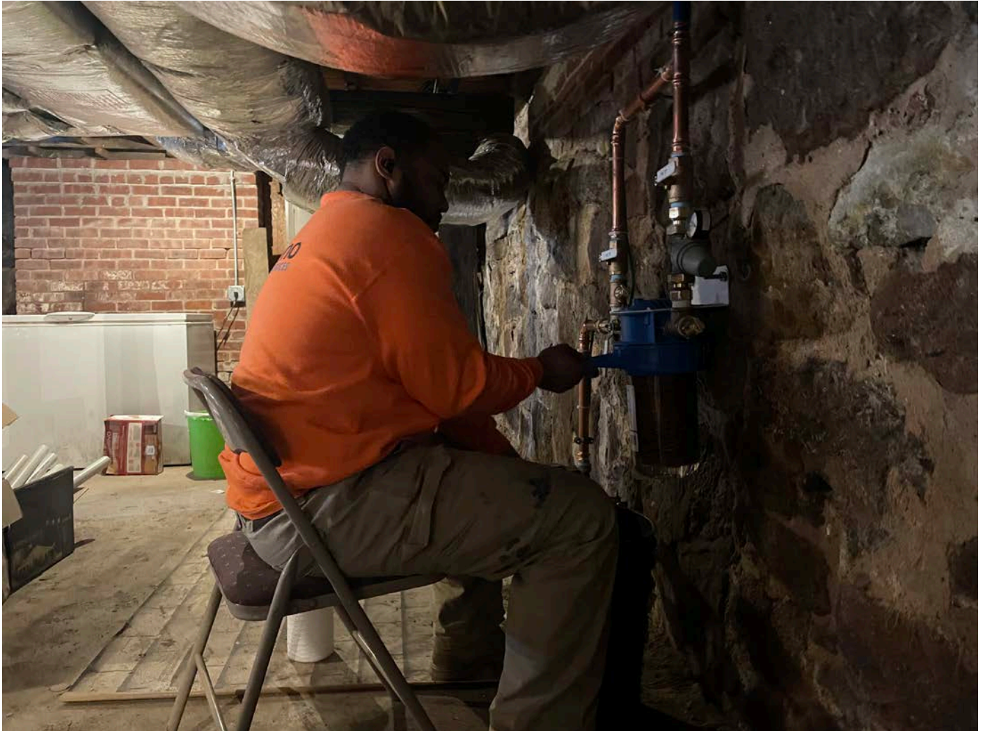
Picture 6: Fazzino changing out the water filter on the water system they recently installed at the 293 Main Street, Durham, residence.
