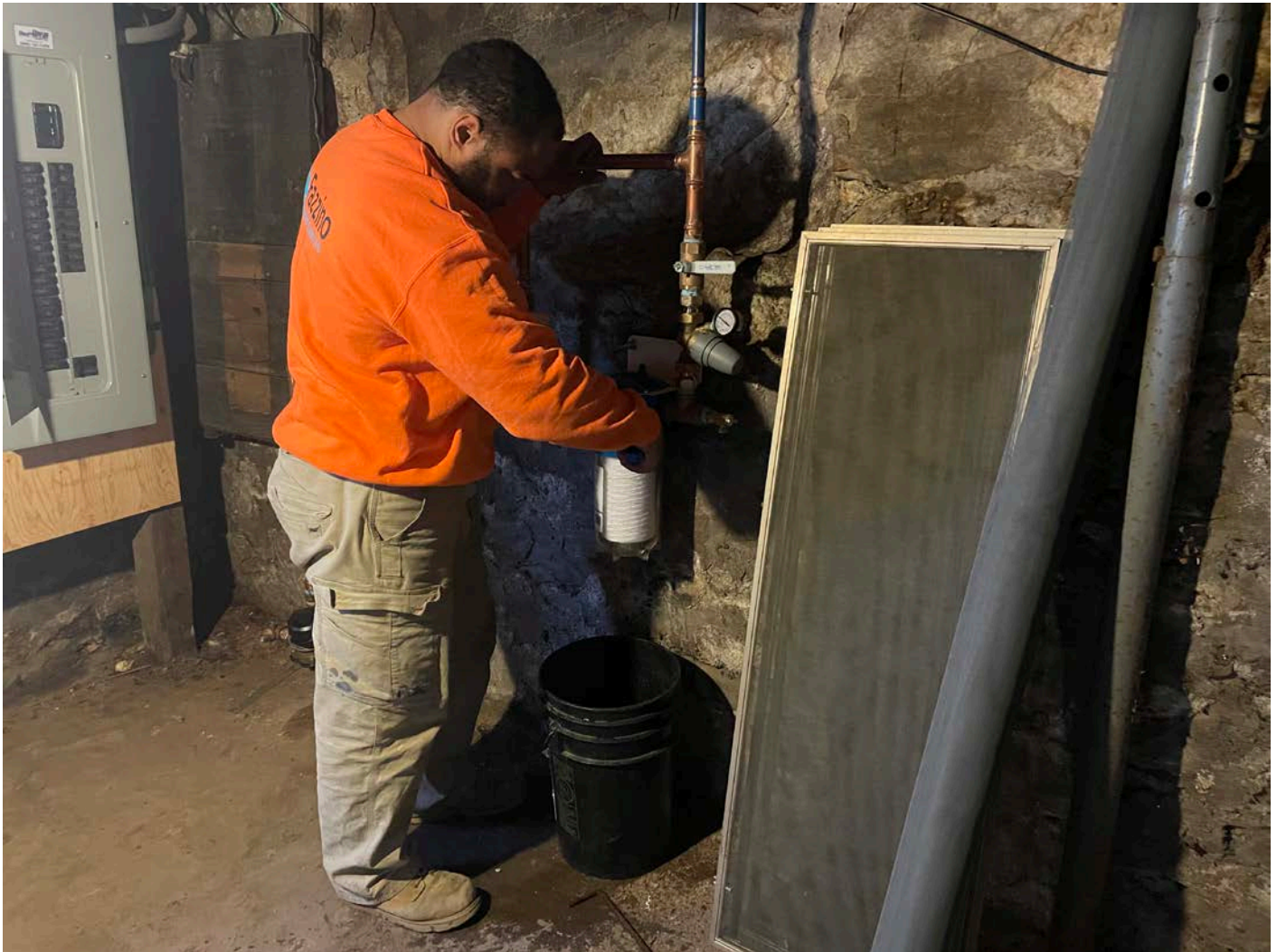
Picture 7: Fazzino changing out the water filter on the water system they recently installed at the 246 Main Street, Durham, residence.
