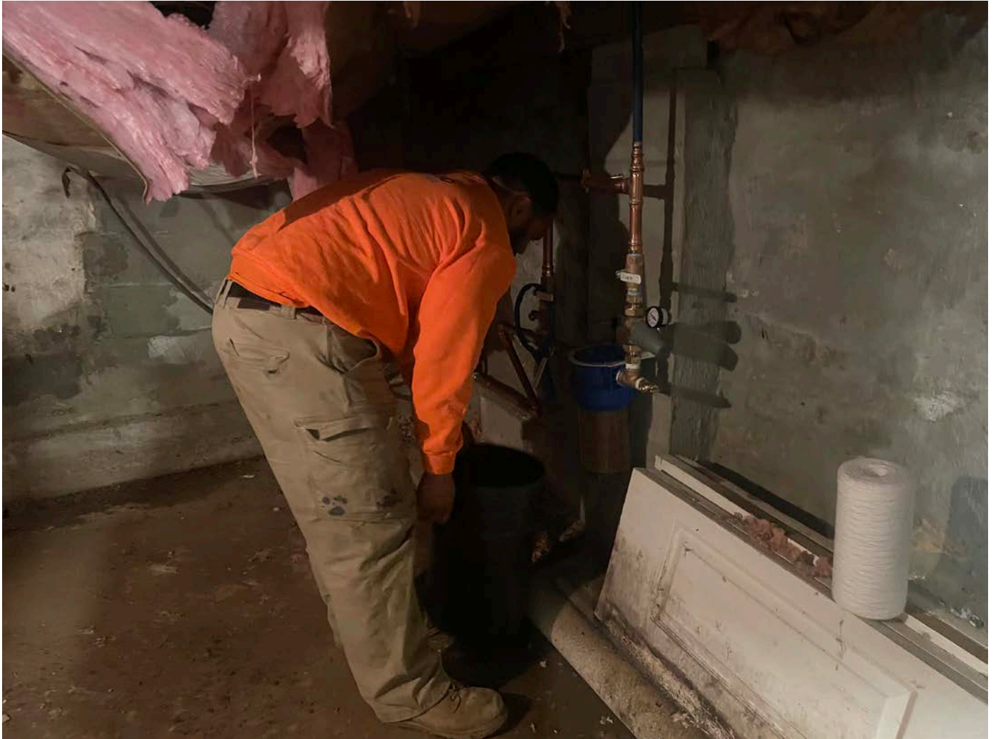
Picture 8: Fazzino changing out the water filter on the water system they recently installed at the 233 Main Street, Durham, residence.
