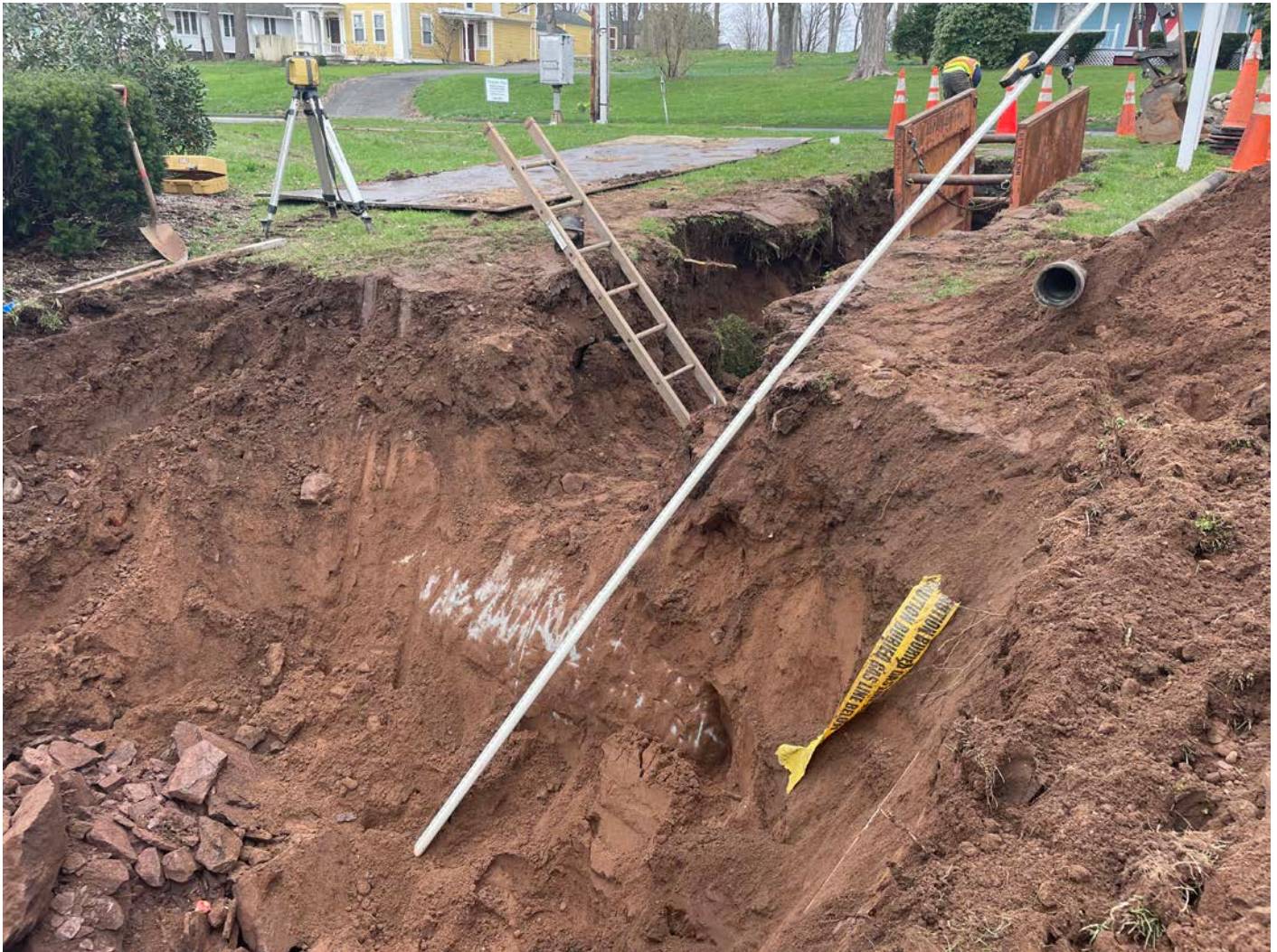
Picture 1: Pit that Ludlow is excavating for the placement of a water meter vault on 4-14-22. The east side of one of two underground water tanks can be seen approximately 4' below surface grade. View to the west/southwest.
