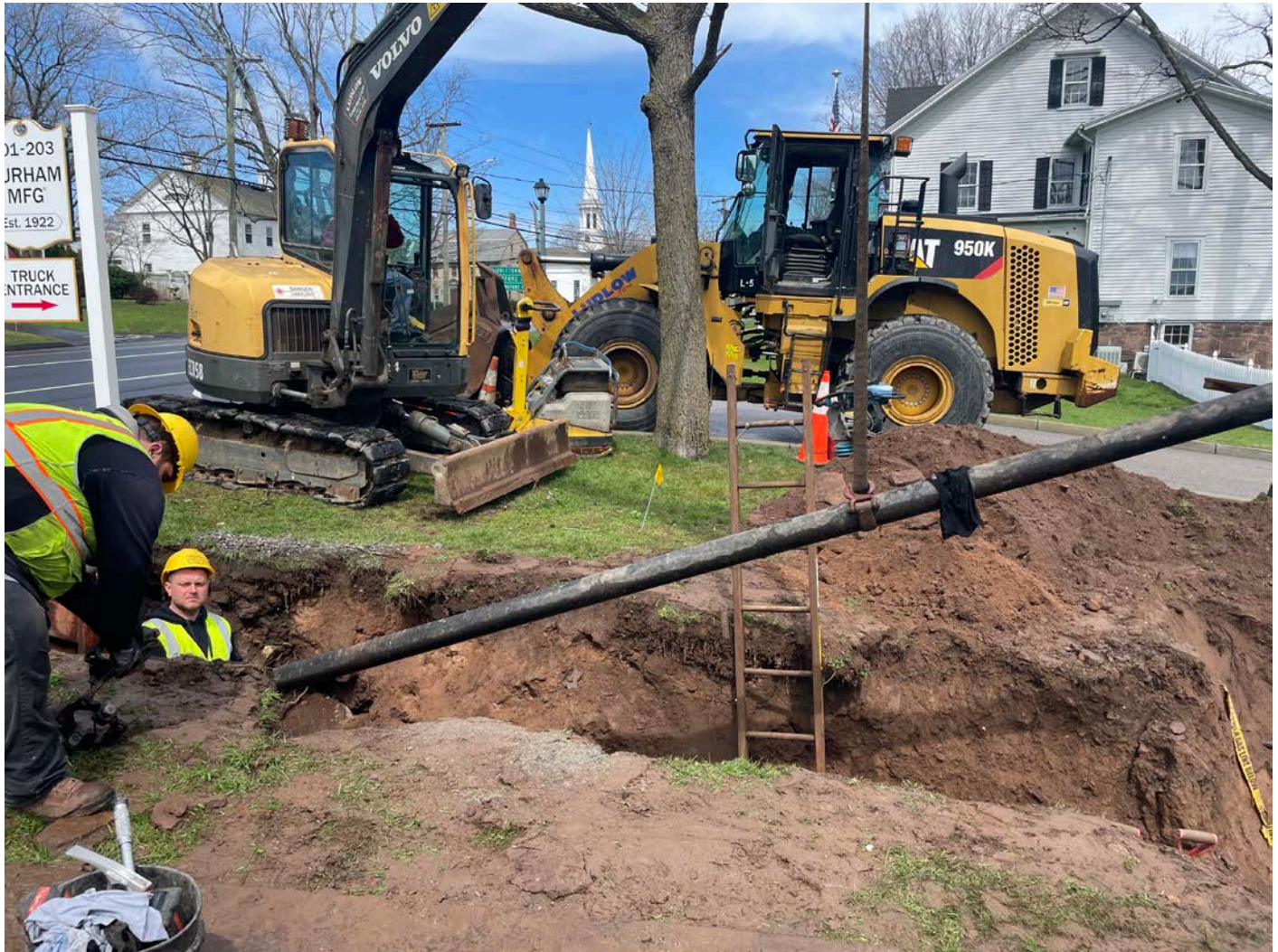
Picture 4: Ludlow in the process of installing 4" DIP water service line at the Durham Manufacturing property. View to the north.
