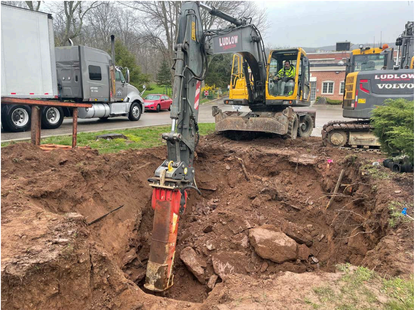
Picture 2: Ludlow using a pneumatic hammer to break up rock as they excavate a pit for the placement of a water meter vault on 4-14-22. View to the west.
