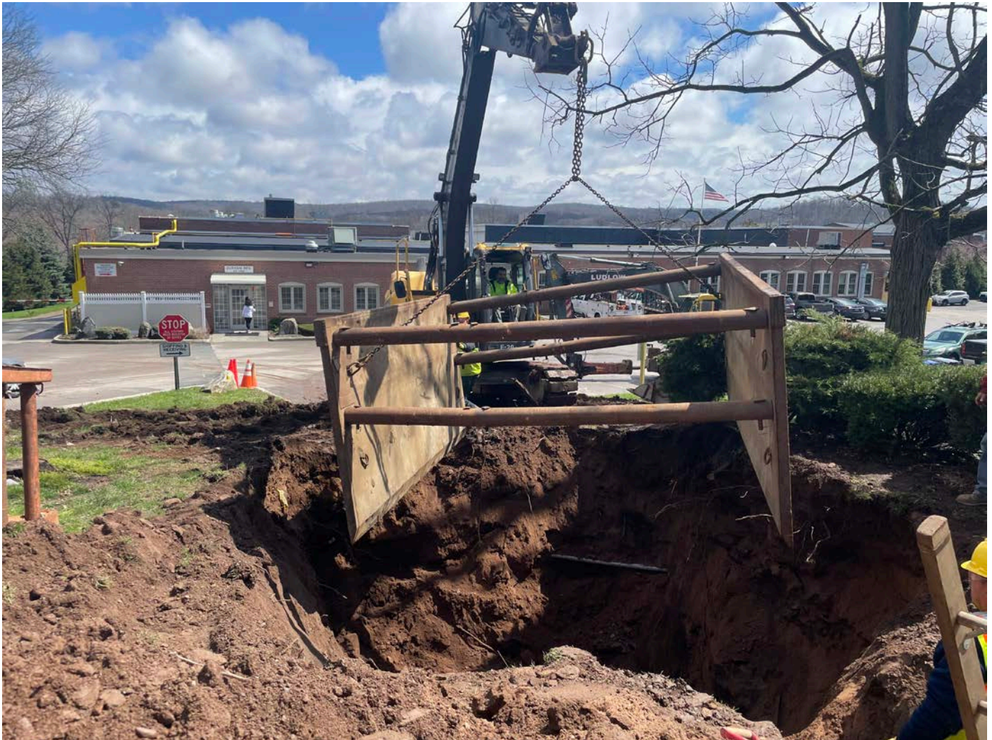
Picture 6: Ludlow setting a trench box inside of the pit they excavated for the installation of a water meter pit at the Durham Manufacturing property. View to the east.
