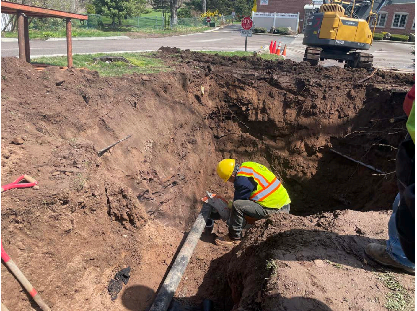
Picture 5: Ludlow saw cutting excess 4" DIP they just installed on the west side of where the water meter vault will be installed tomorrow. View to the east.
