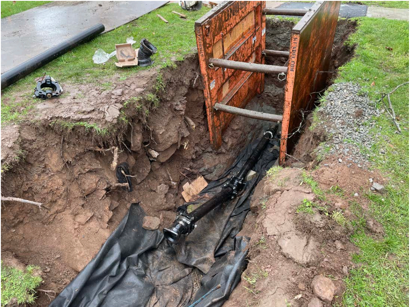
Picture 3: 4" DIP water service line that Ludlow has begun to install at the Durham Manufacturing property. View to the west.
