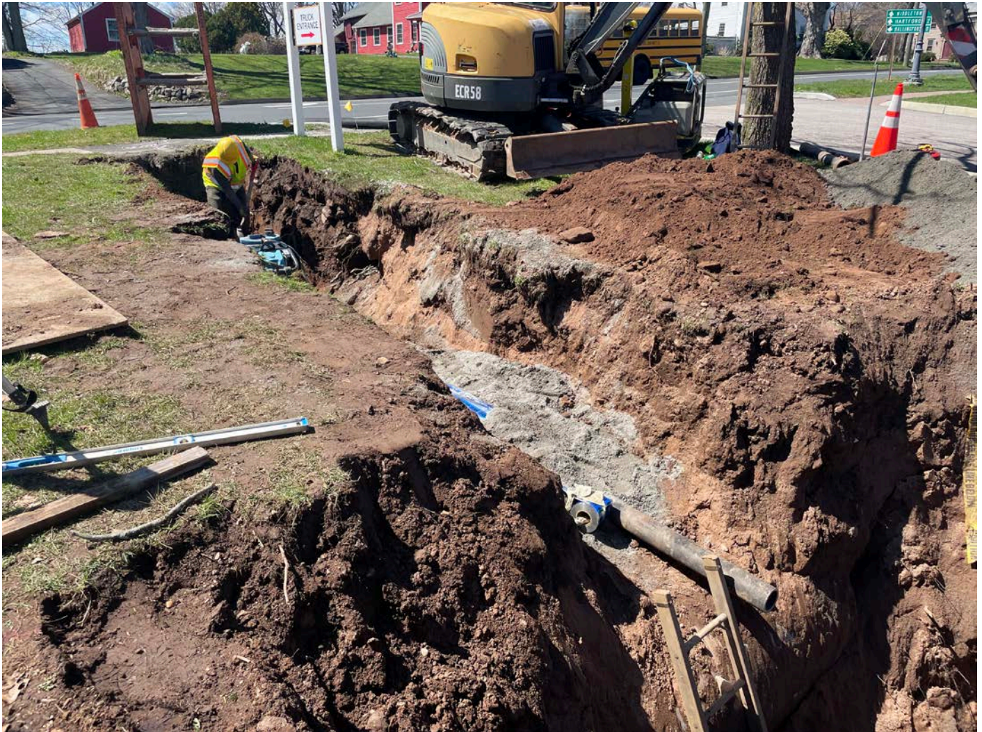
Picture 9: View of partially-backfilled 4" DIP that Ludlow installed to the west of the pit they excavated for the installation of a water meter pit at the Durham Manufacturing property. View to the northwest.
