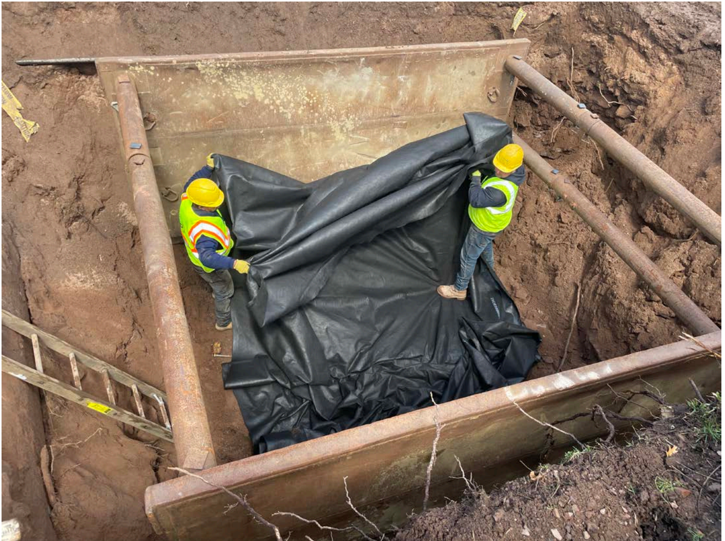
Picture 7: Ludlow placing geofabric inside of the pit they excavated for the installation of a water meter pit at the Durham Manufacturing property. View to the northeast.
