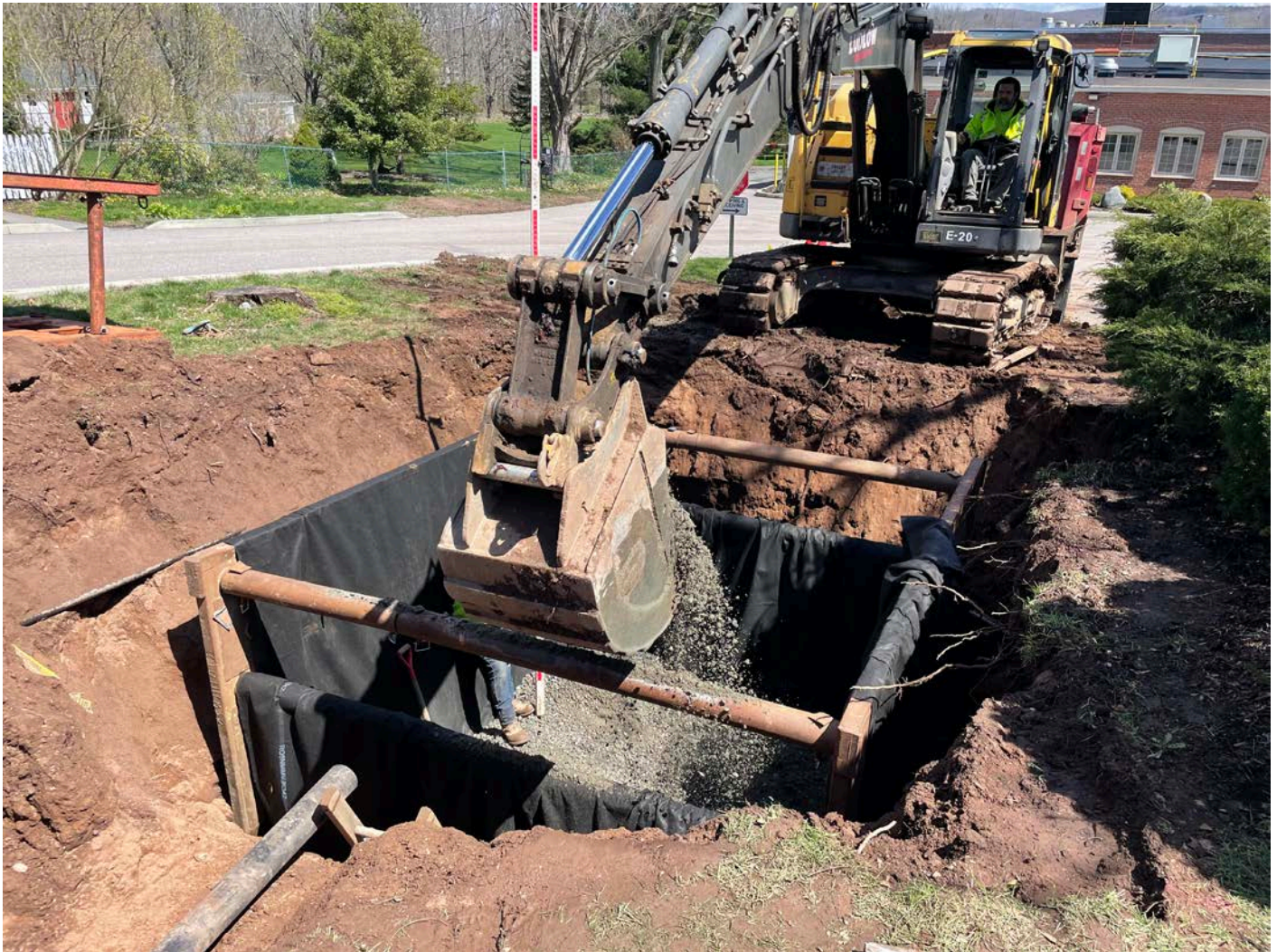
Picture 8: Ludlow placing ¾" gravel on top of the geofabric they placed inside of the pit they excavated for the installation of a water meter pit at the Durham Manufacturing property. View to the east.
