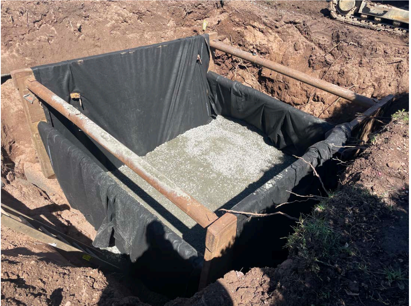
Picture 10: Pit that Ludlow excavated for the installation of a water meter pit at the Durham Manufacturing property, after having placed \frac{3}{4} " gravel. View to the northeast.
