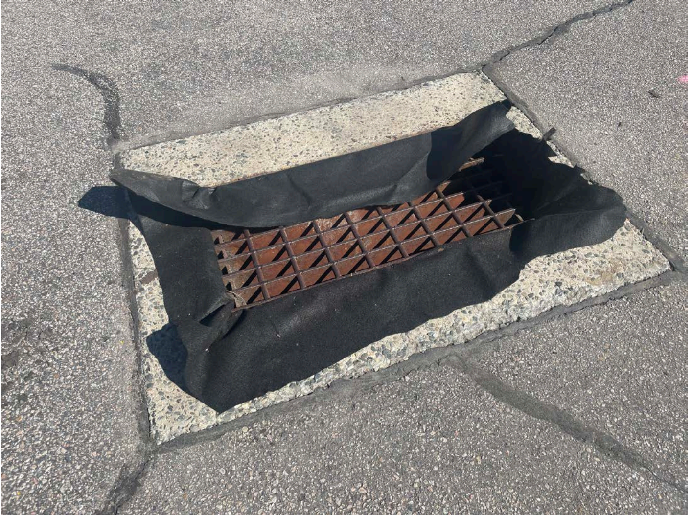
Picture 3: One of two catch basins where Ludlow placed filter fabric beneath the grate to capture sediment while they install a 4" DIP water line at the Durham Manufacturing property. View to the northwest.
