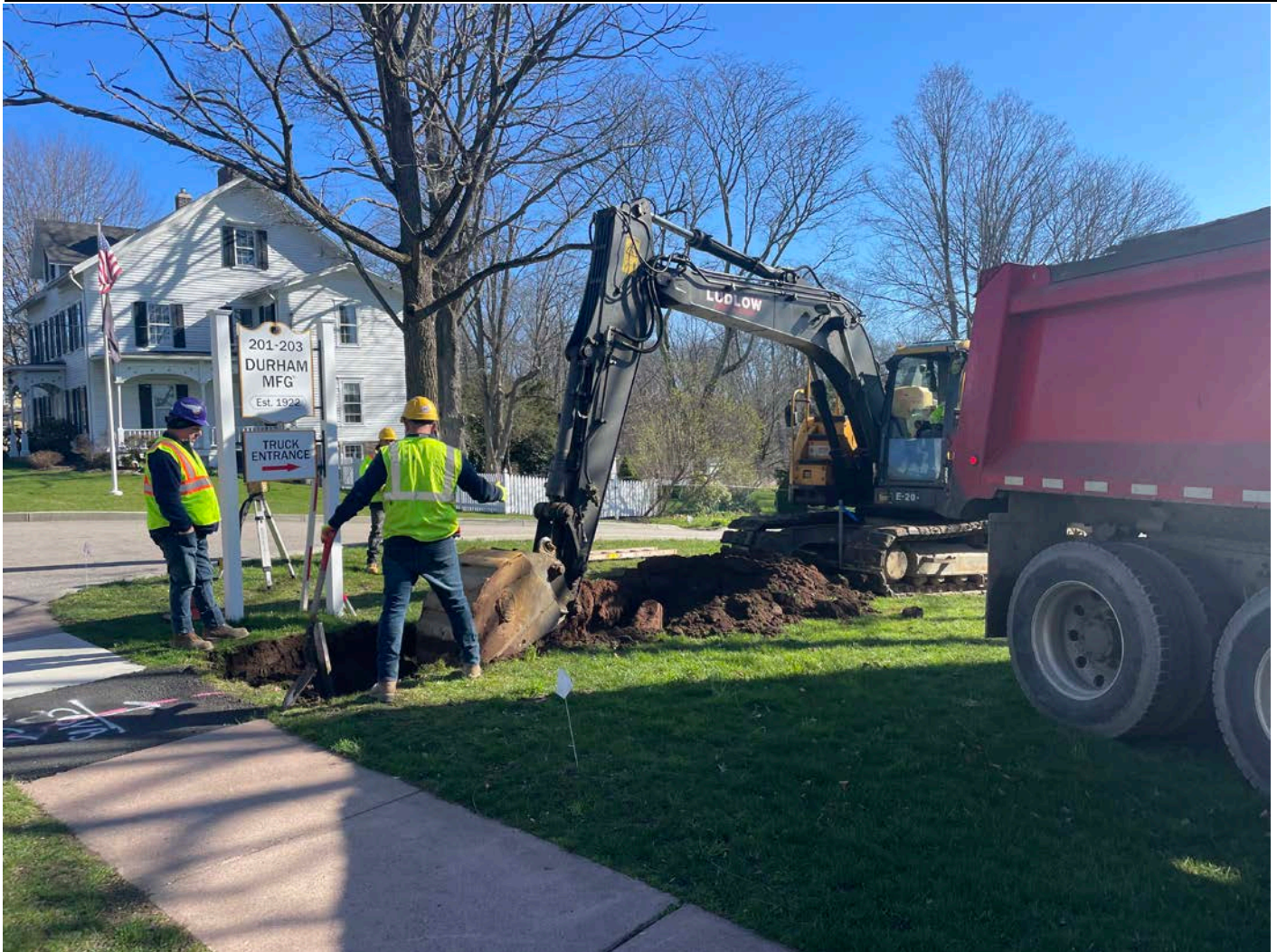
Picture 1: Ludlow beginning to excavate a trench at the Durham Manufacturing property for the installation of a 4" DIP water service line. View to the northeast.
