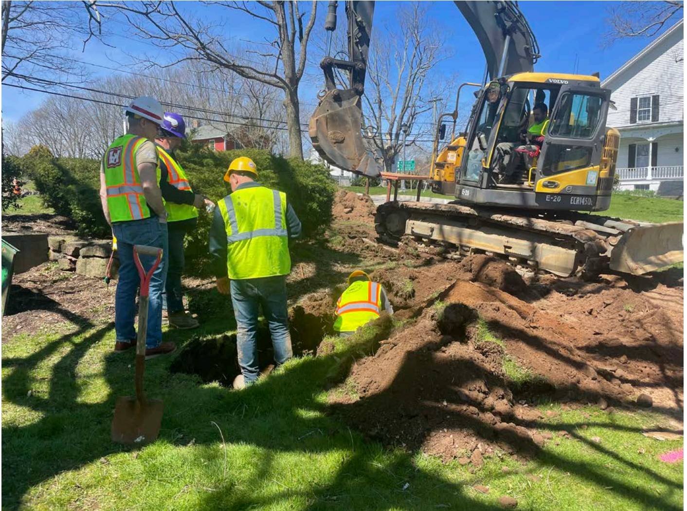
Picture 6: Ludlow excavating a test pit south of the existing well vault as they work to daylight the well line and its associated power line. View to the northwest.
