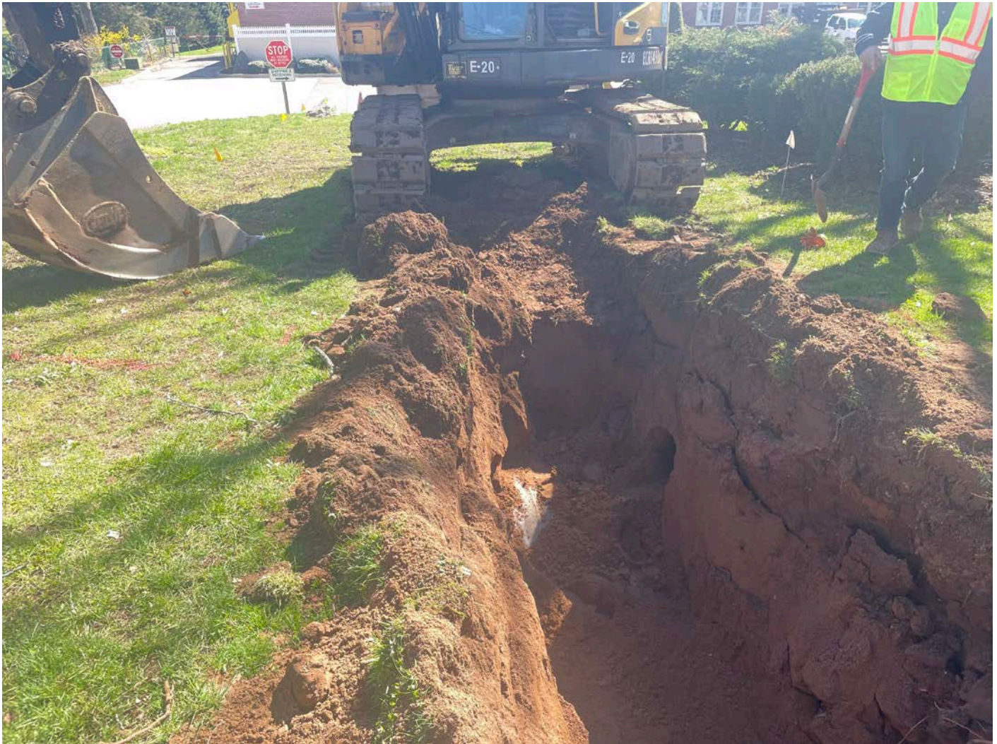
Picture 4: Top of the first water storage tank that Ludlow daylighted while excavating a trench for the installation of a 4" DIP water service line at the Durham Manufacturing property. View to the east.
