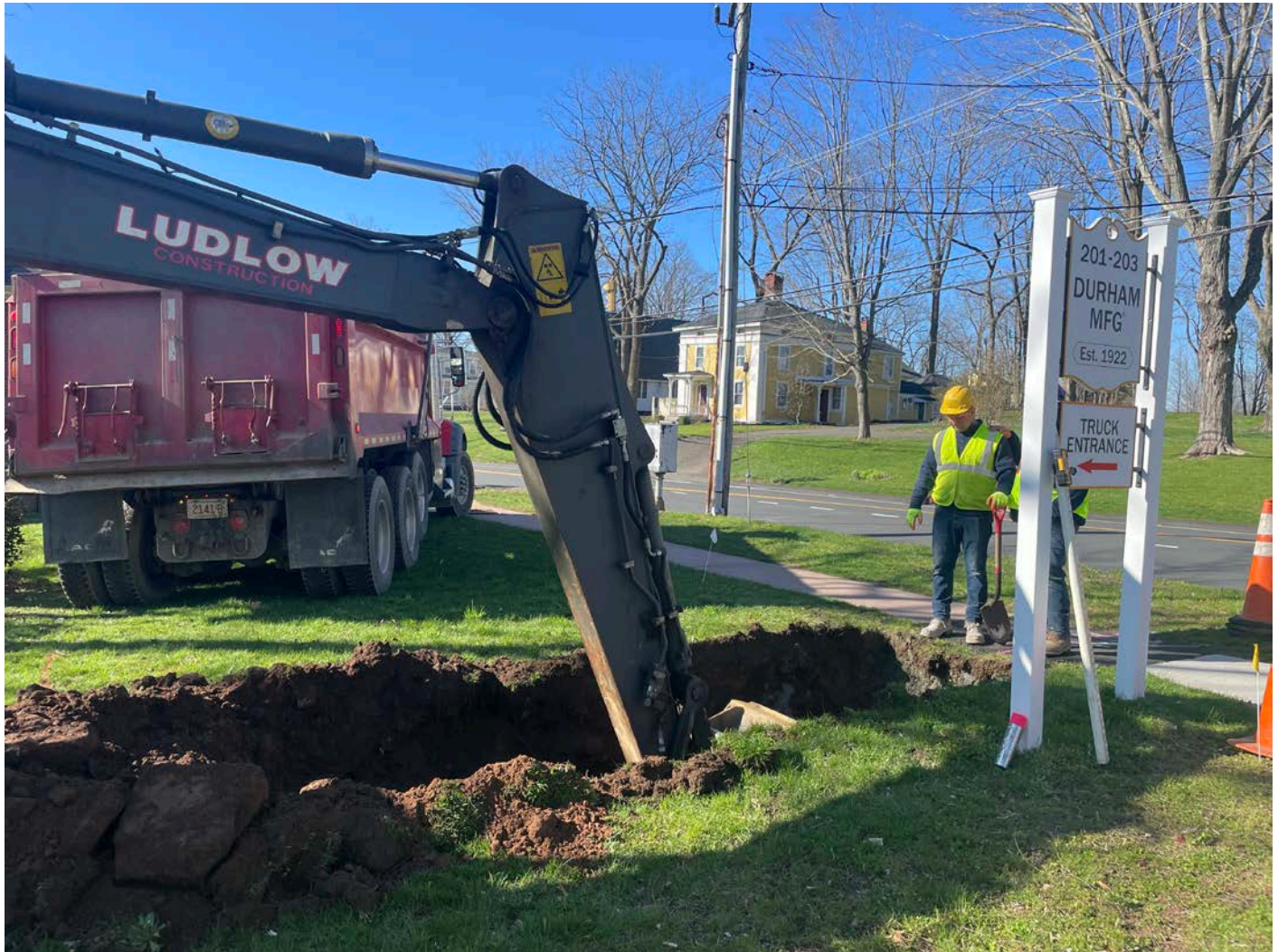
Picture 2: Ludlow beginning to excavate a trench at the Durham Manufacturing property for the installation of a 4" DIP water service line. View to the southwest.
