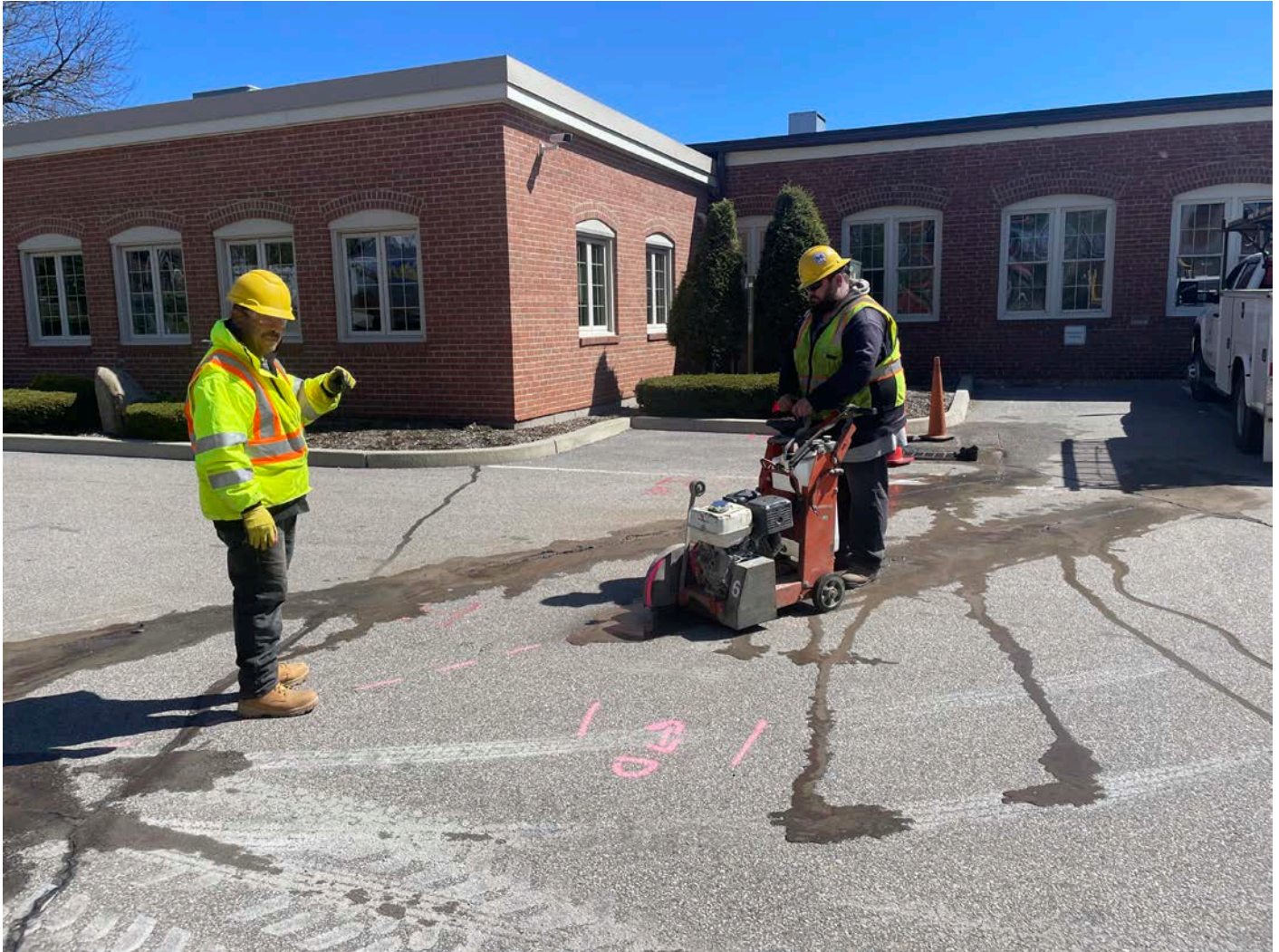
Picture 5: Ludlow saw cutting the footprint of trench through the driveway of the Durham manufacturing facility for the installation of the 4" DIP waterline. View to the east.
