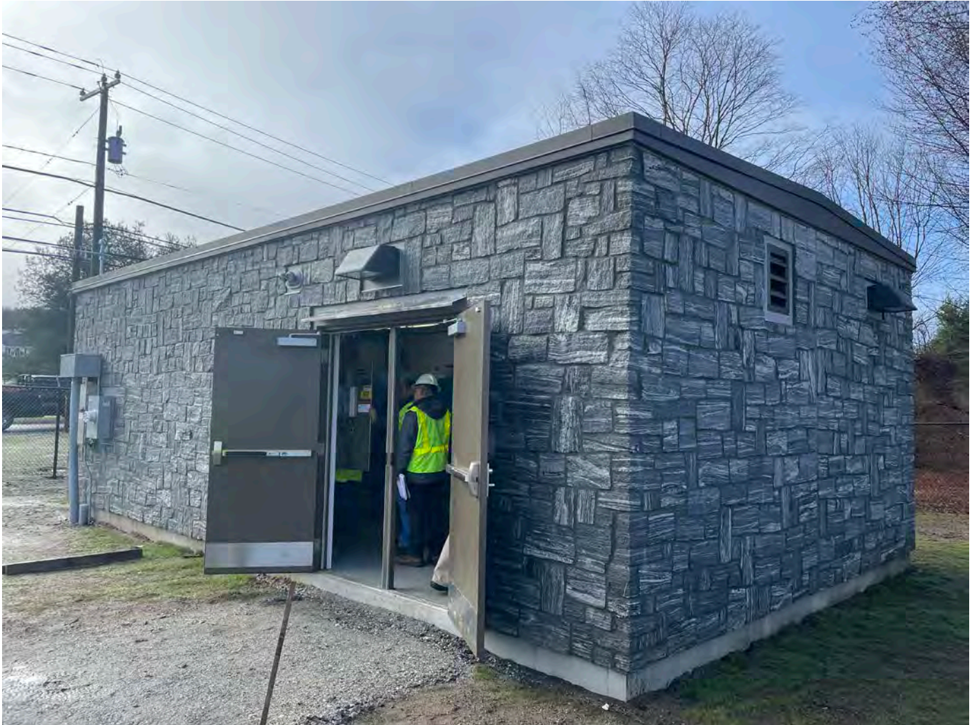
Picture 4: Exterior view of the booster station located on S. Main Street in Middletown. View to the southeast.
