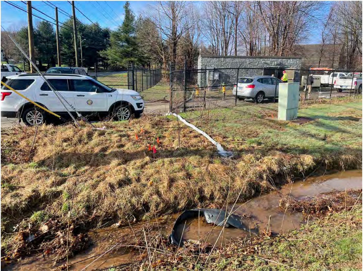
Picture 5: Potable water generated from start-up activities being discharged to a swale located to the north/northeast of the booster station located on S. Main Street in Middletown. View to the south.
