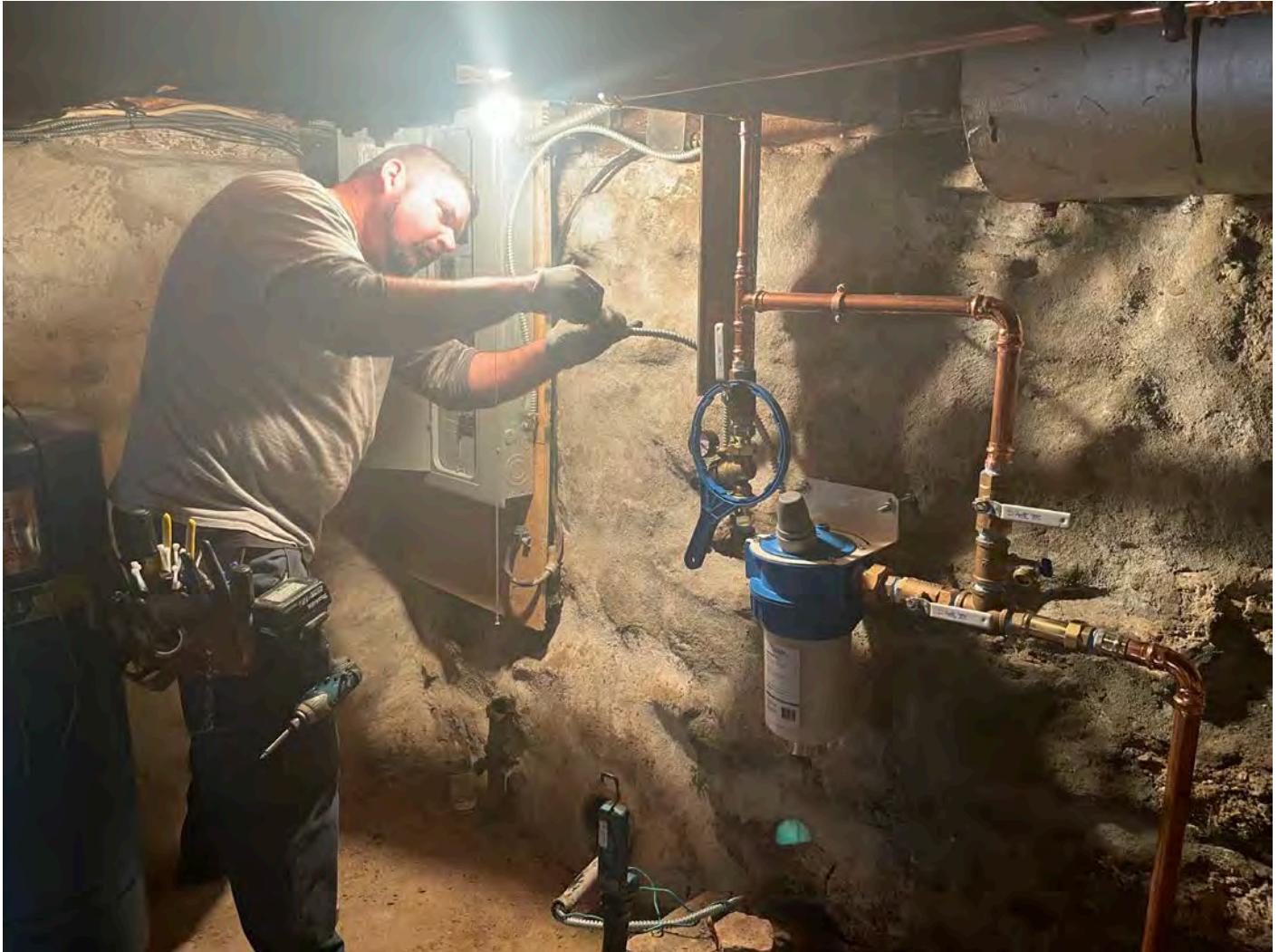
Picture 2: Apuzzo Electric installing a ground line to the final water service components at the 25 Talcott Lane, Durham, residence.
