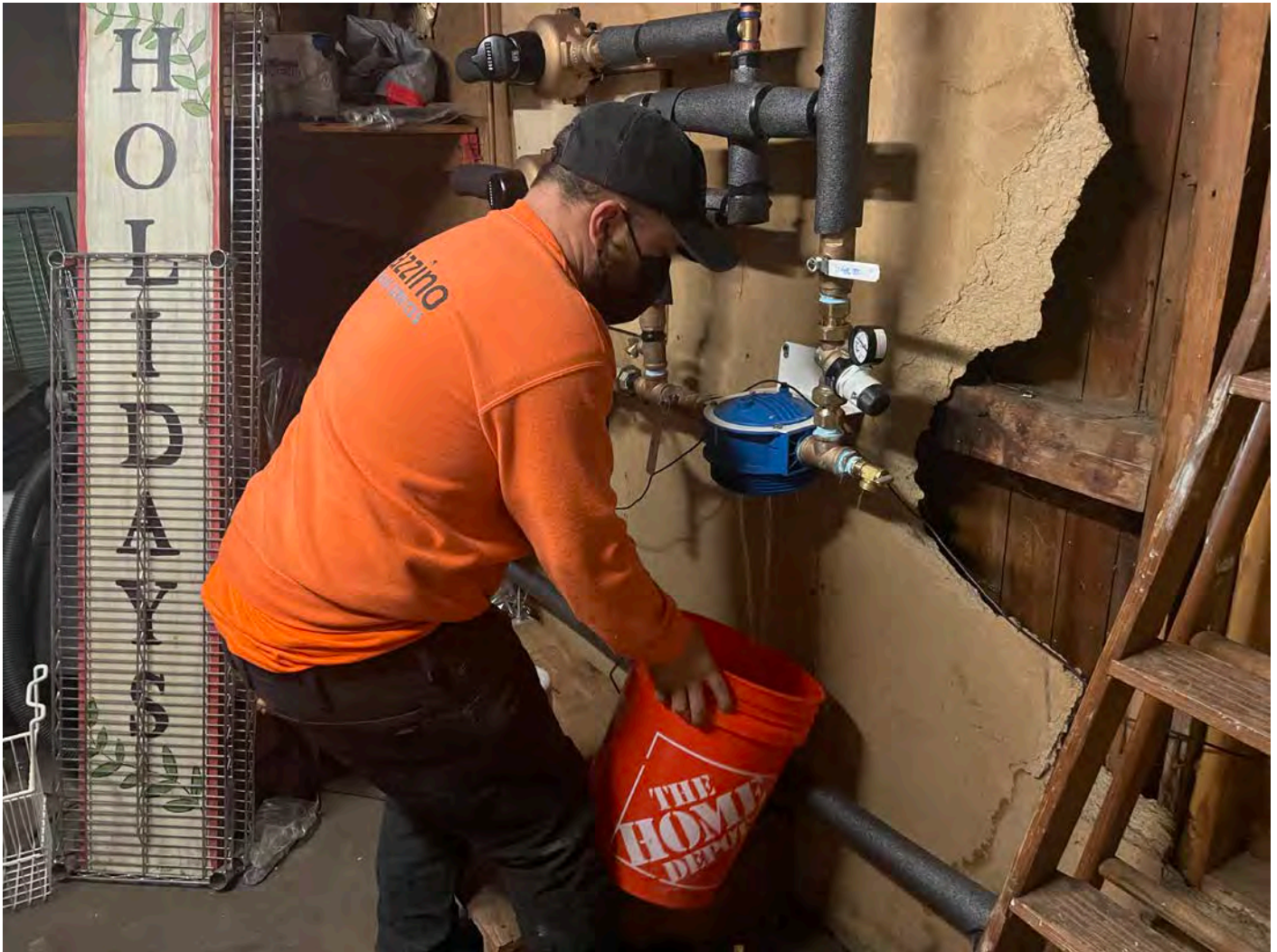
Picture 14: Fazzino Plumbing changing out the filter on the recently installed final water system at the 238 Main Street, Durham, building.
