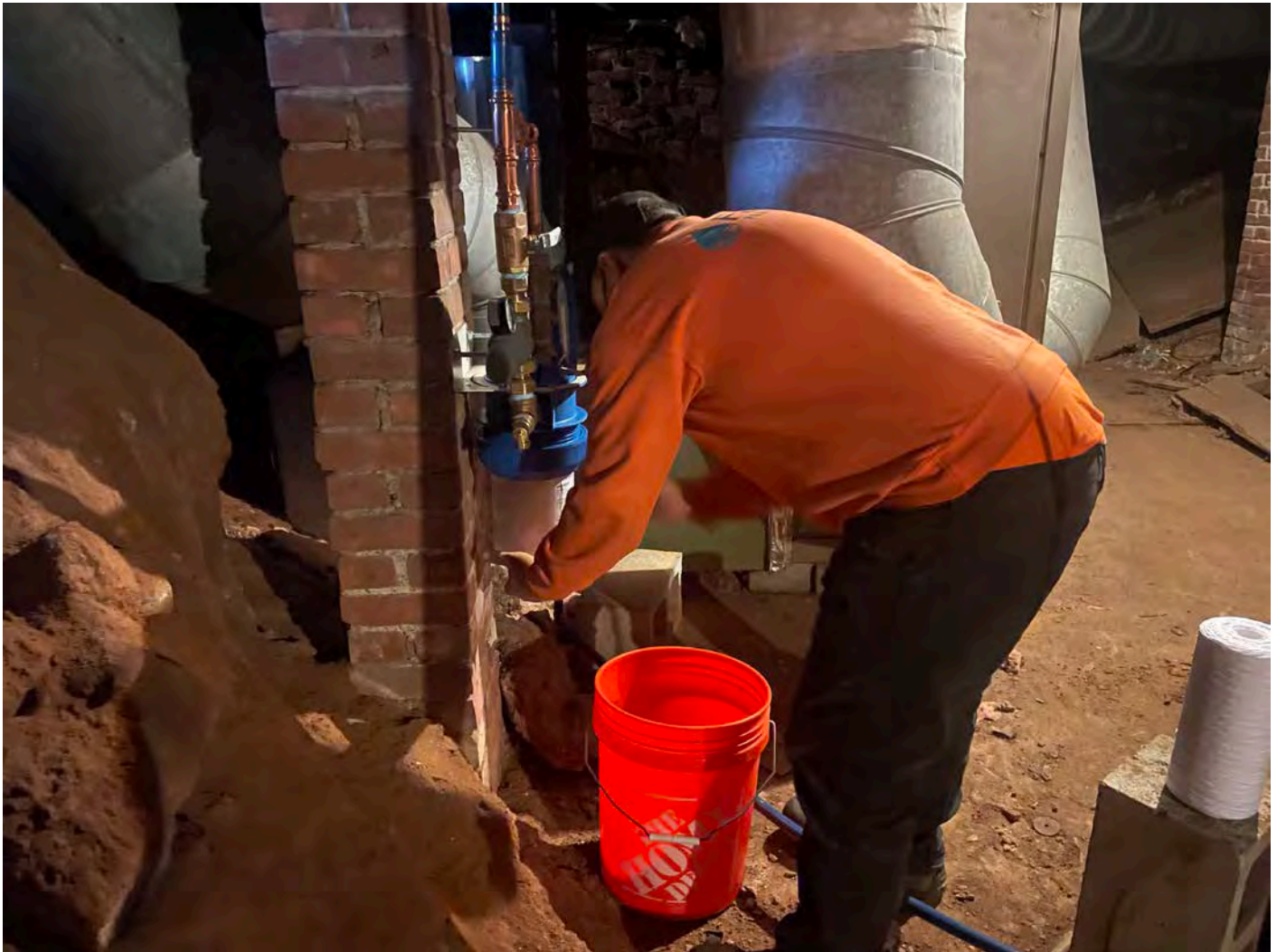
Picture 13: Fazzino Plumbing changing out the filter on the recently installed final water system at the 236 Main Street, Durham, building.
