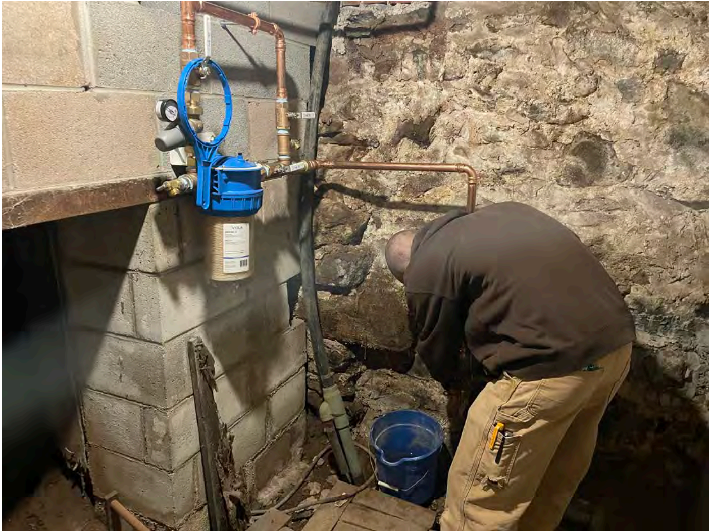
Picture 5: Apuzzo Electric installing a ground line to the final water service components at the 162 Maple Avenue, Durham, residence.
