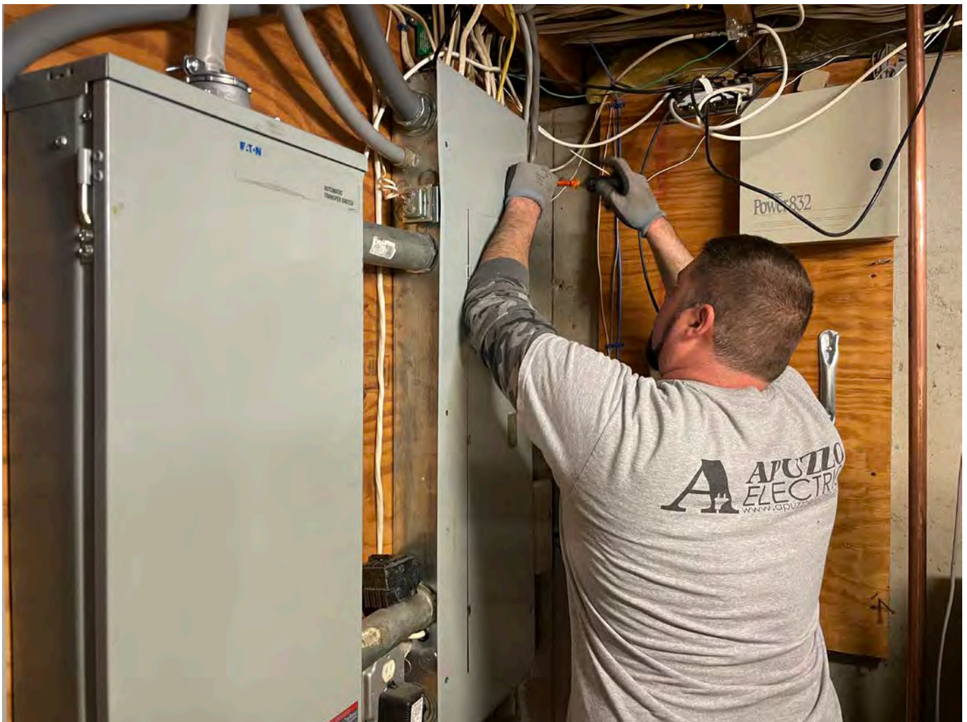
Picture 8: Apuzzo Electric installing a ground line to the final water service components at the 212R Maple Avenue, Durham, residence.
