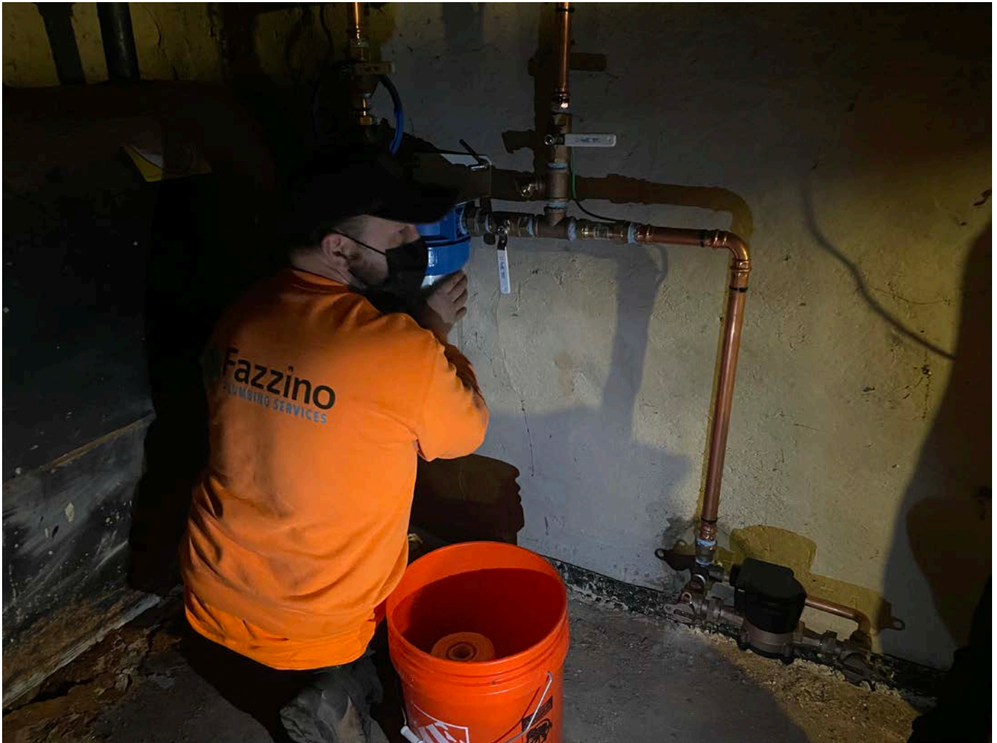
Picture 1: Fazzino Plumbing changing out the filter on the recently-installed final water system at the 19 Maiden Lane, Durham, residence.
