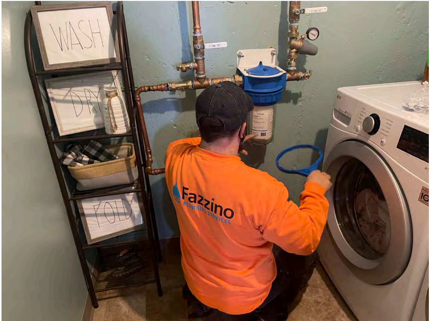
Picture 4: Fazzino Plumbing changing out the filter on the recently-installed final water system at the 129 Maple Avenue, Durham, residence.
