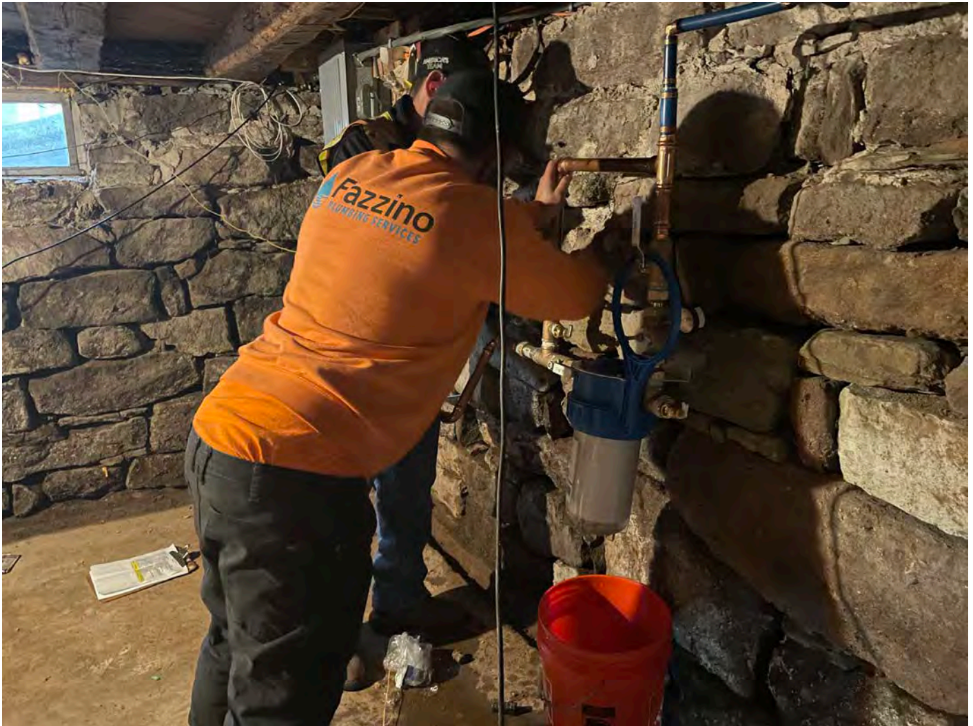
Picture 16: Fazzino Plumbing changing out the filter on the recently installed final water system at the 248 Main Street, Durham, residence.
