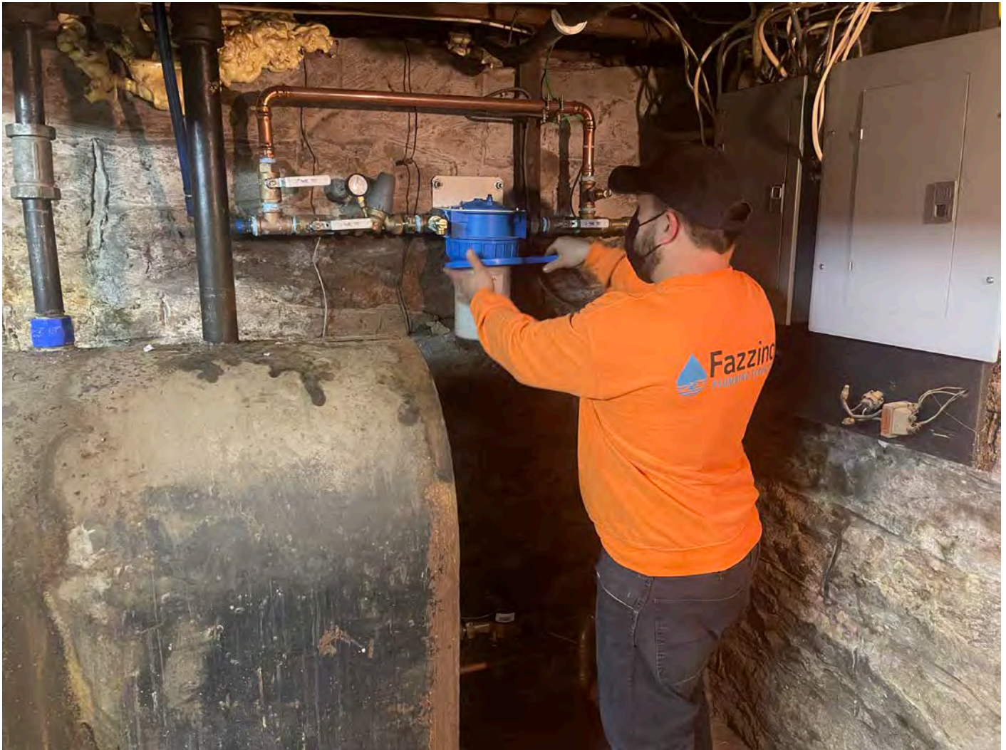
Picture 3: Fazzino Plumbing changing out the filter on the recently installed final water system at the 120 Main Street, Durham, residence.
