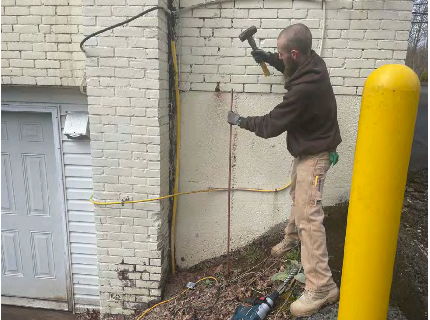
Picture 11: Apuzzo Electric installing a ground line to the final water service components at the 235 Main Street, Durham, building.
