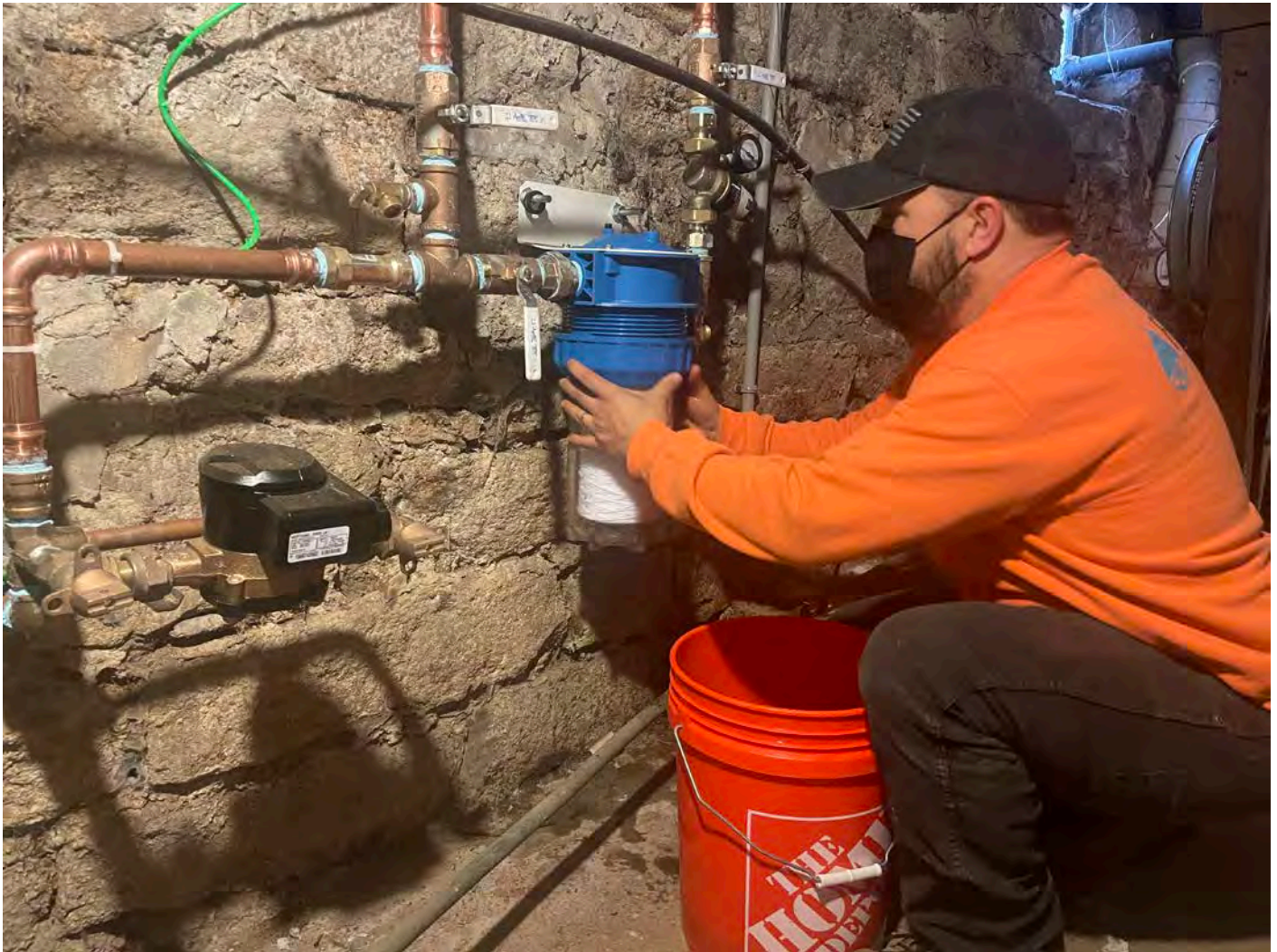
Picture 17: Fazzino Plumbing changing out the filter on the recently installed final water system at the 257 Main Street, Durham, residence.
