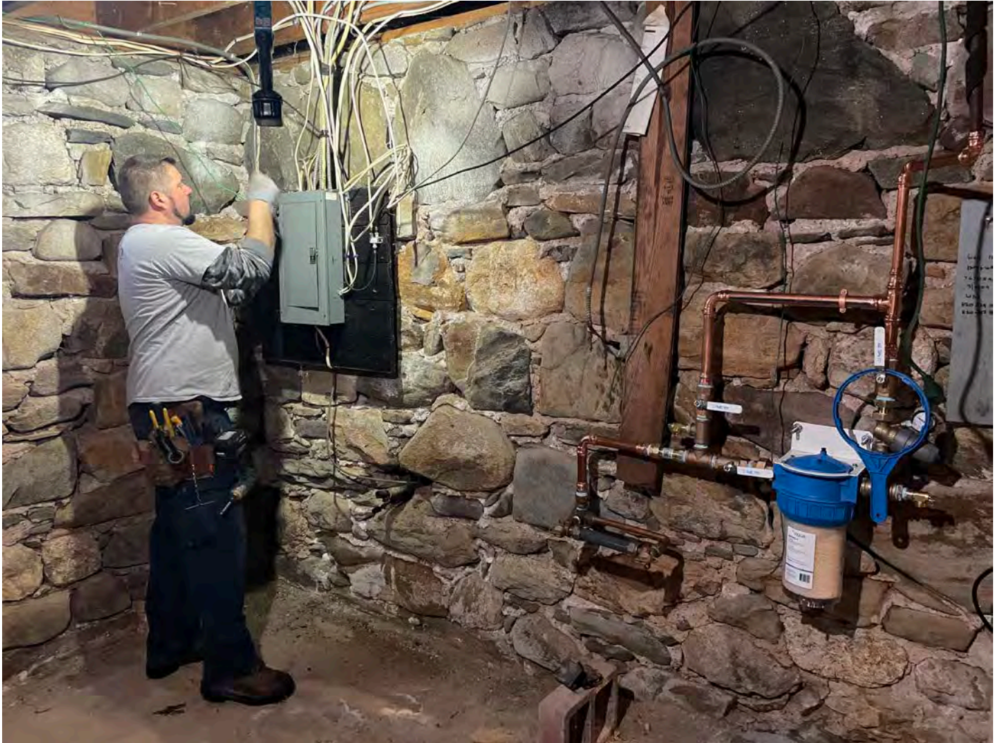
Picture 12: Apuzzo Electric installing a ground line to the final water service components at the 235 Maple Avenue, Durham, residence.
