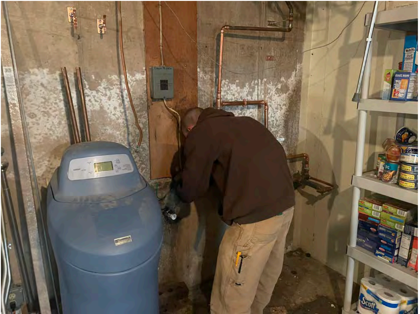
Picture 7: Apuzzo Electric installing a ground line to the final water service components at the 206 Maple Avenue, Durham, residence.
