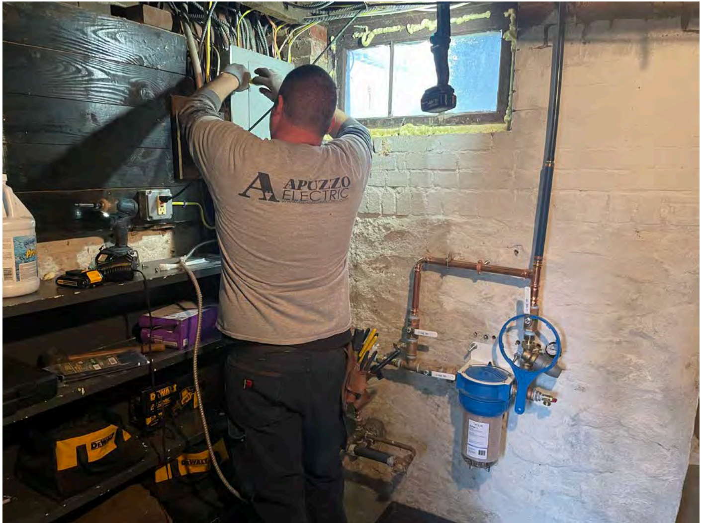
Picture 15: Apuzzo Electric installing a ground line to the final water service components at the 105 Maiden Lane, Durham, residence.
