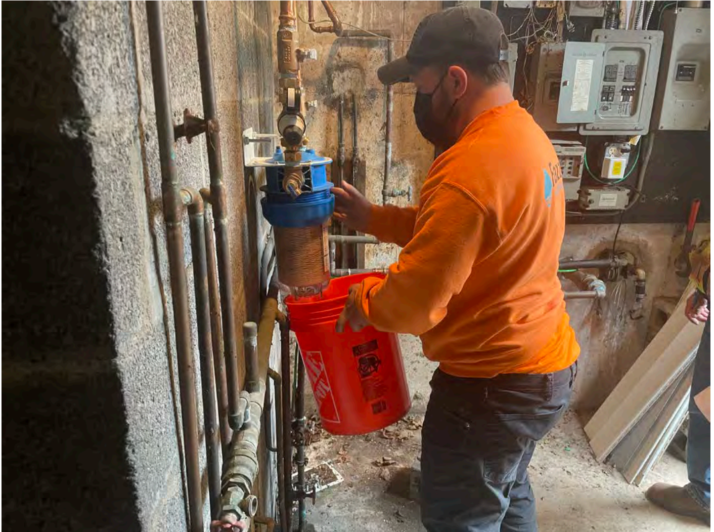
Picture 6: Fazzino Plumbing changing out the filter on the recently installed final water system at the 196 Main Street, Durham, building.
