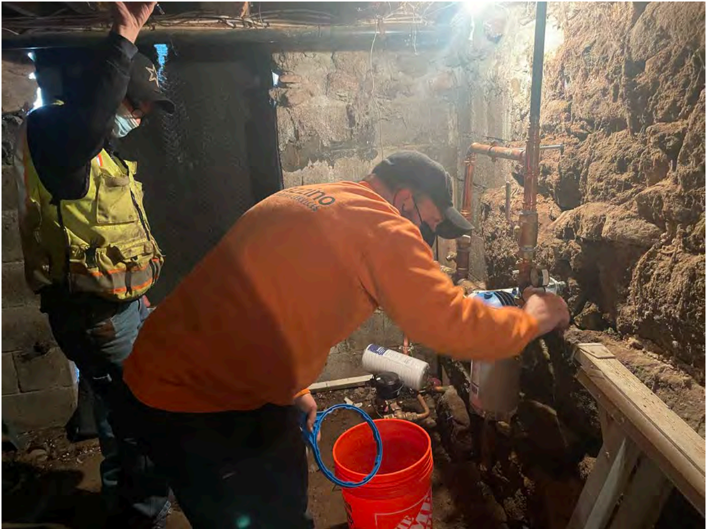
Picture 9: Fazzino Plumbing changing out the filter on the recently installed final water system at the 228 Main Street, Durham, residence.
