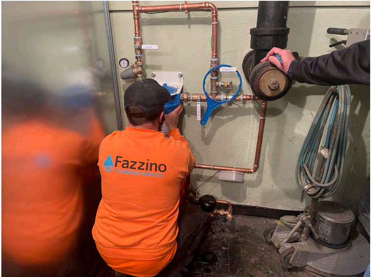
Picture 10: Fazzino Plumbing changing out the filter on the recently installed final water system at the 228R Main Street, Durham, residence.
