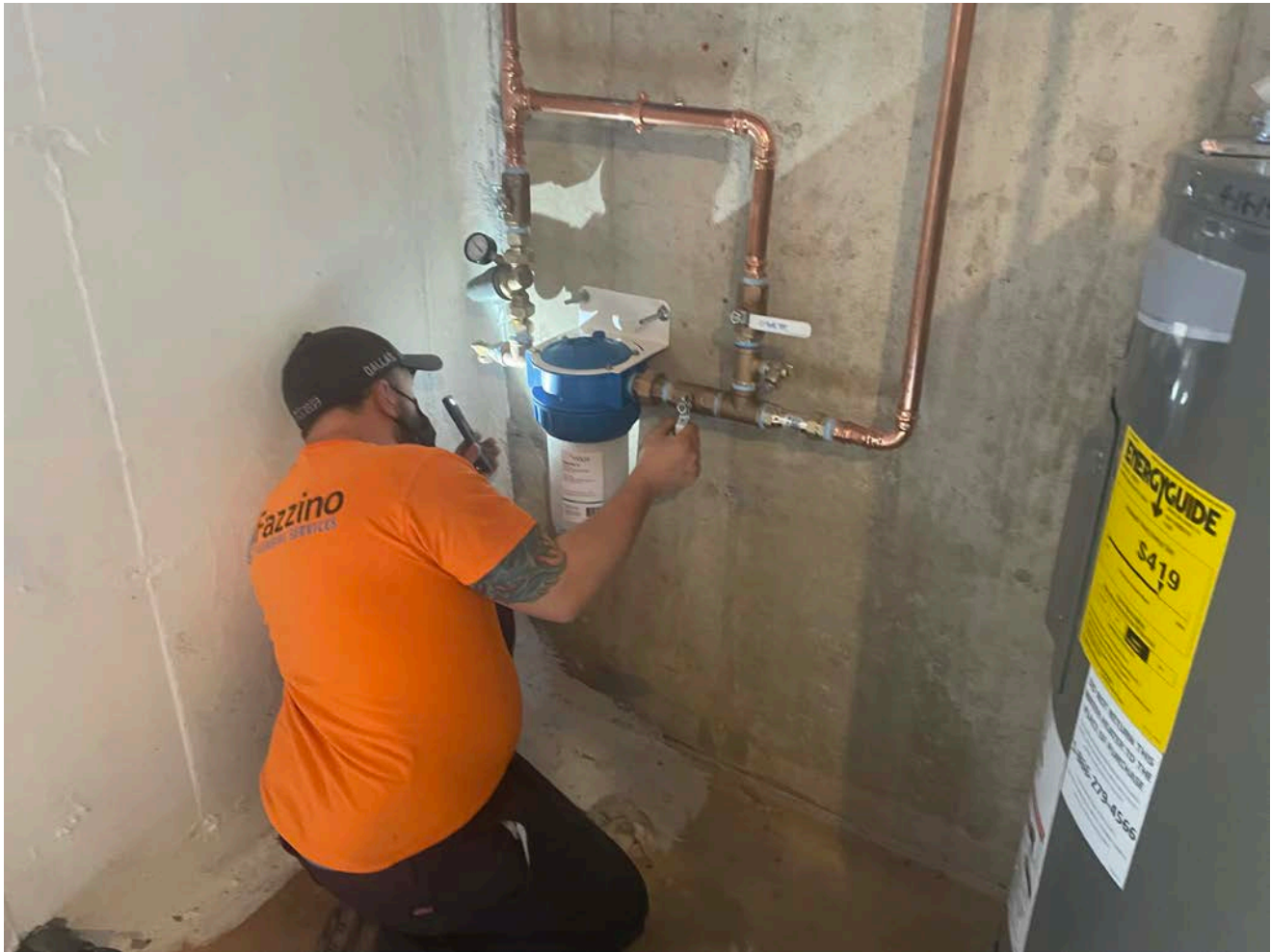
Picture 3: Fazzino Plumbing inspecting the final water system components they installed today at the 166 Maple Avenue residence in Durham.
