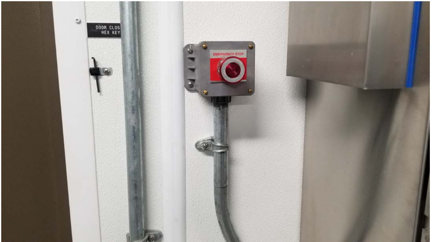
Picture 4: Emergency Generator Stop Button installed at the Water Booster Station.
