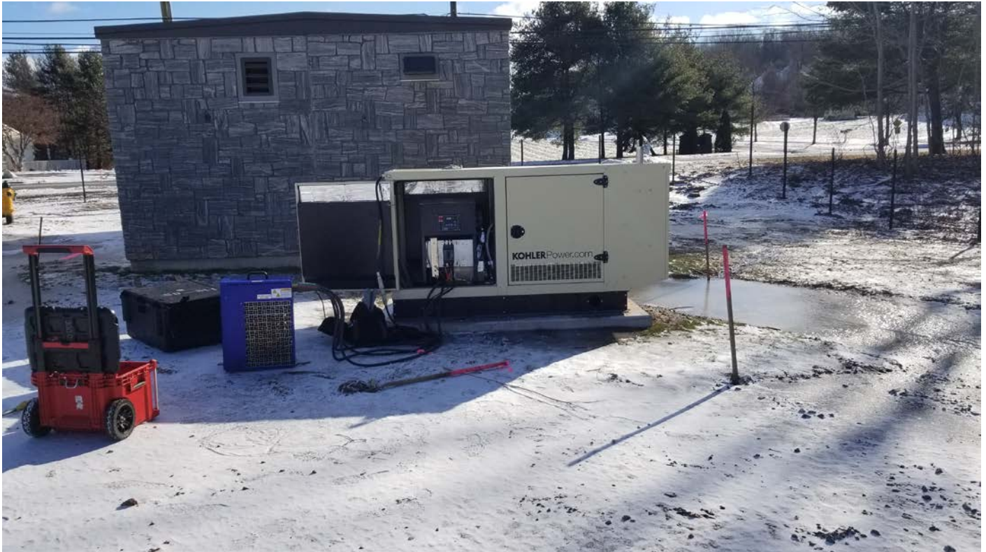
Picture 7: Load bank connected to the generator set at the Booster Station.
