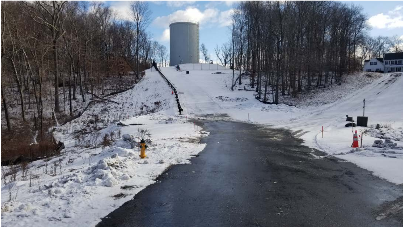
Picture 2: Water Tank Driveway – Fence gates have not yet been installed.
