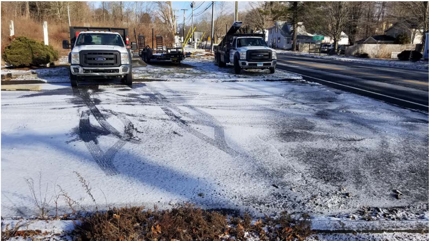
Picture 1: Atlas Fence installing fence posts at the PRV Vault, Main Street, Durham.
