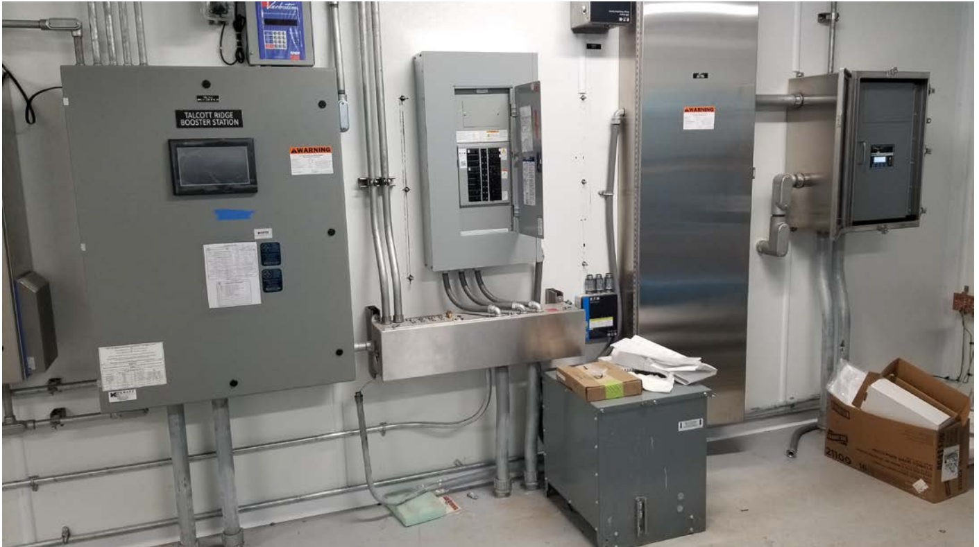
Picture 3: Temporary Loadcenter and transformer installed at the Water Booster Station.
