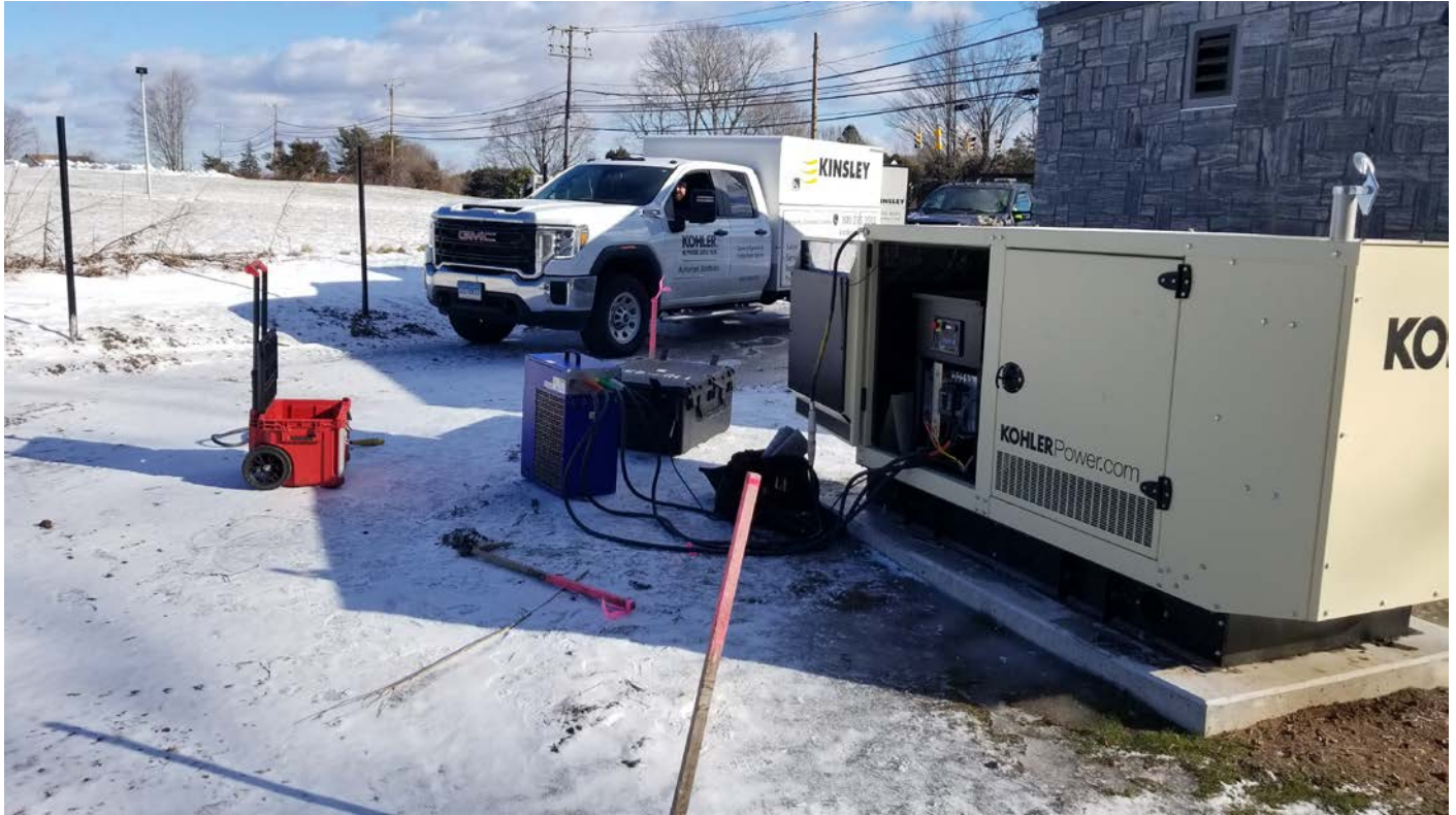
Picture 5: Load bank connected to the generator set at the Booster Station.
