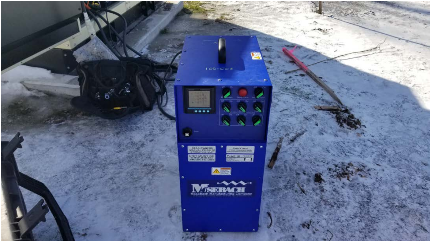
Picture 6: Load bank connected to the generator set at the Booster Station.
