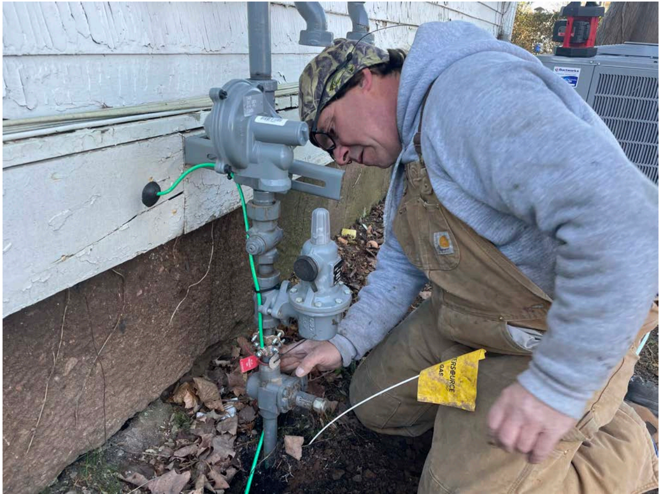
Picture 7: Apuzzo Electric installing new bonding wires on the north side of the 313 Main Street, Durham, residence.
