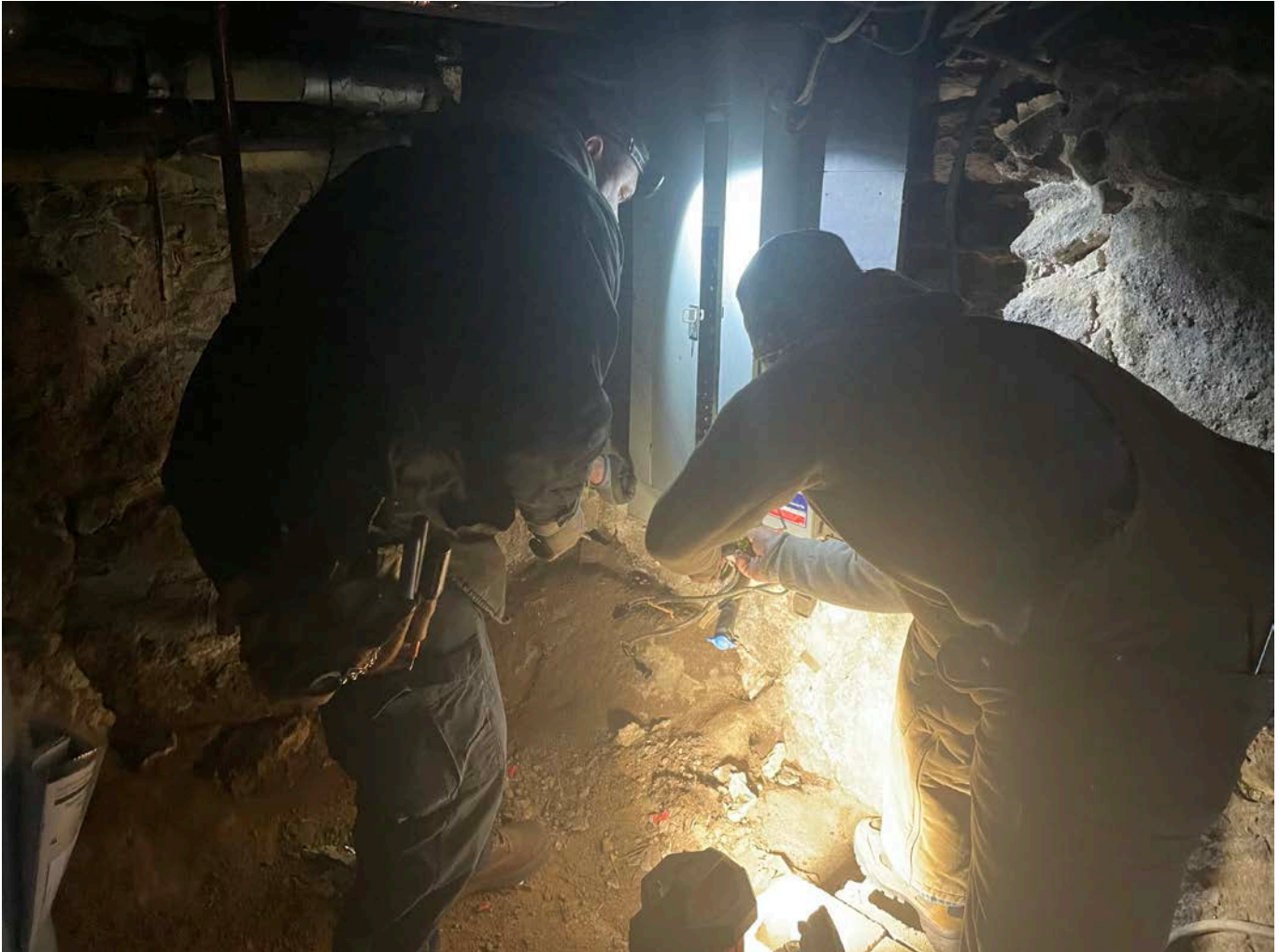
Picture 8: Apuzzo Electric installing new bonding wires to the recently installed water system components at the 297 Main Street, Durham, residence.
