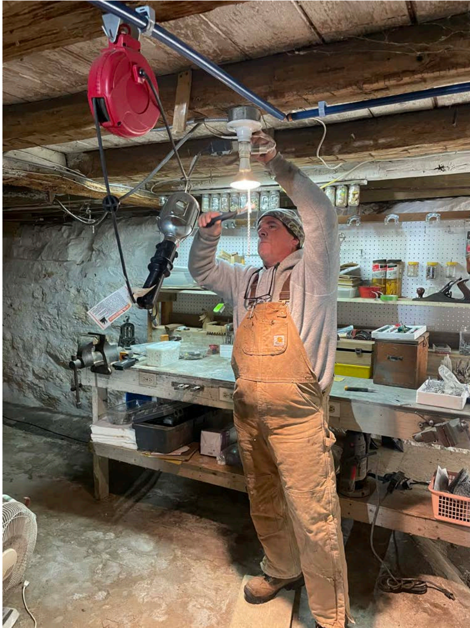
Picture 4: Apuzzo Electric installing new bonding wires to the recently installed water system components at the 322 Main Street, Durham, residence.
