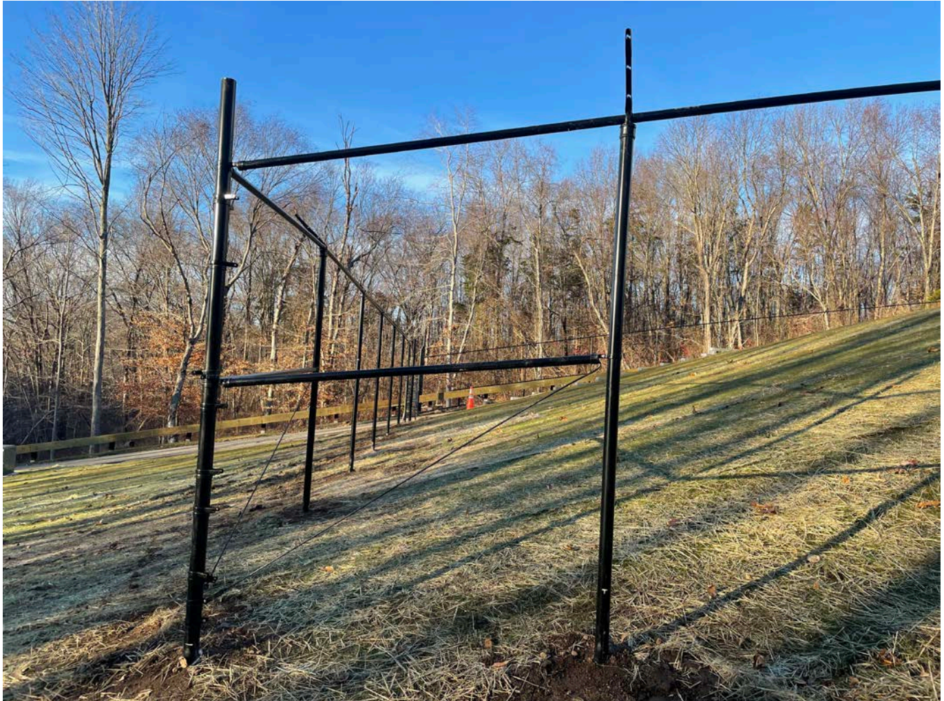
Picture 11: View of progress that Eagle Fence and Guardrail has made at the southwest corner of the water tank work zone. View to the north.
