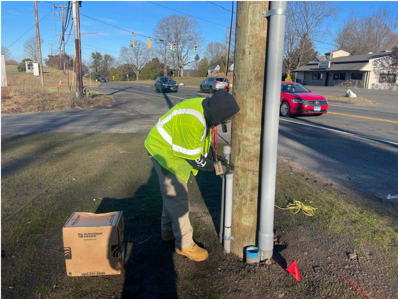
Picture 9: Frontier in the process of running communication lines from pole #9845 located on the west side of S. Main Street, Middletown, to the booster station located at Station 750+63. View to the northeast.
