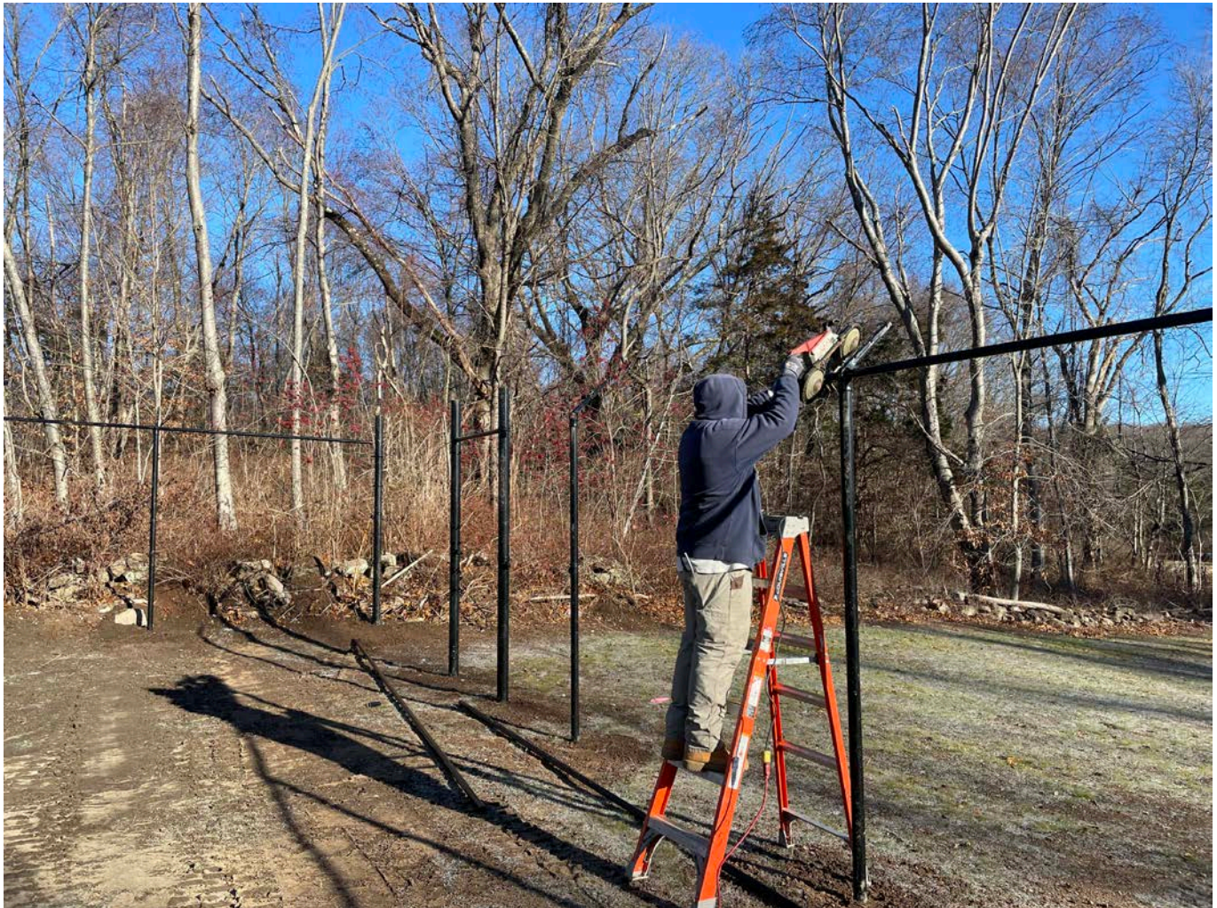
Picture 5: Eagle Fence and Guardrail cutting a section of top rail to size as they install a permanent fence around the water tank work zone located east of the Shared Access Driveway in Middletown. View to the northeast.
