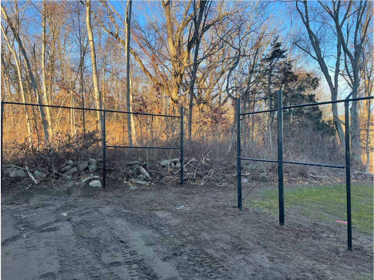
Picture 10: View of progress that Eagle Fence and Guardrail has made at the northeast corner of the water tank work zone. View to the northeast.
