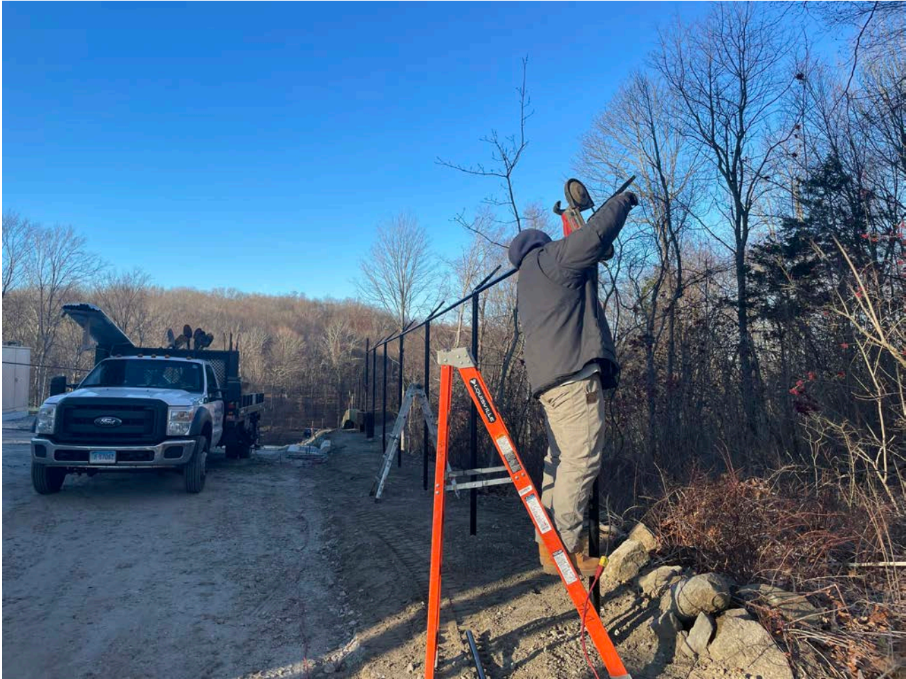
Picture 3: Eagle Fence and Guardrail cutting a section of top rail to size as they install a permanent fence around the water tank work zone located east of the Shared Access Driveway in Middletown. View to the west.
