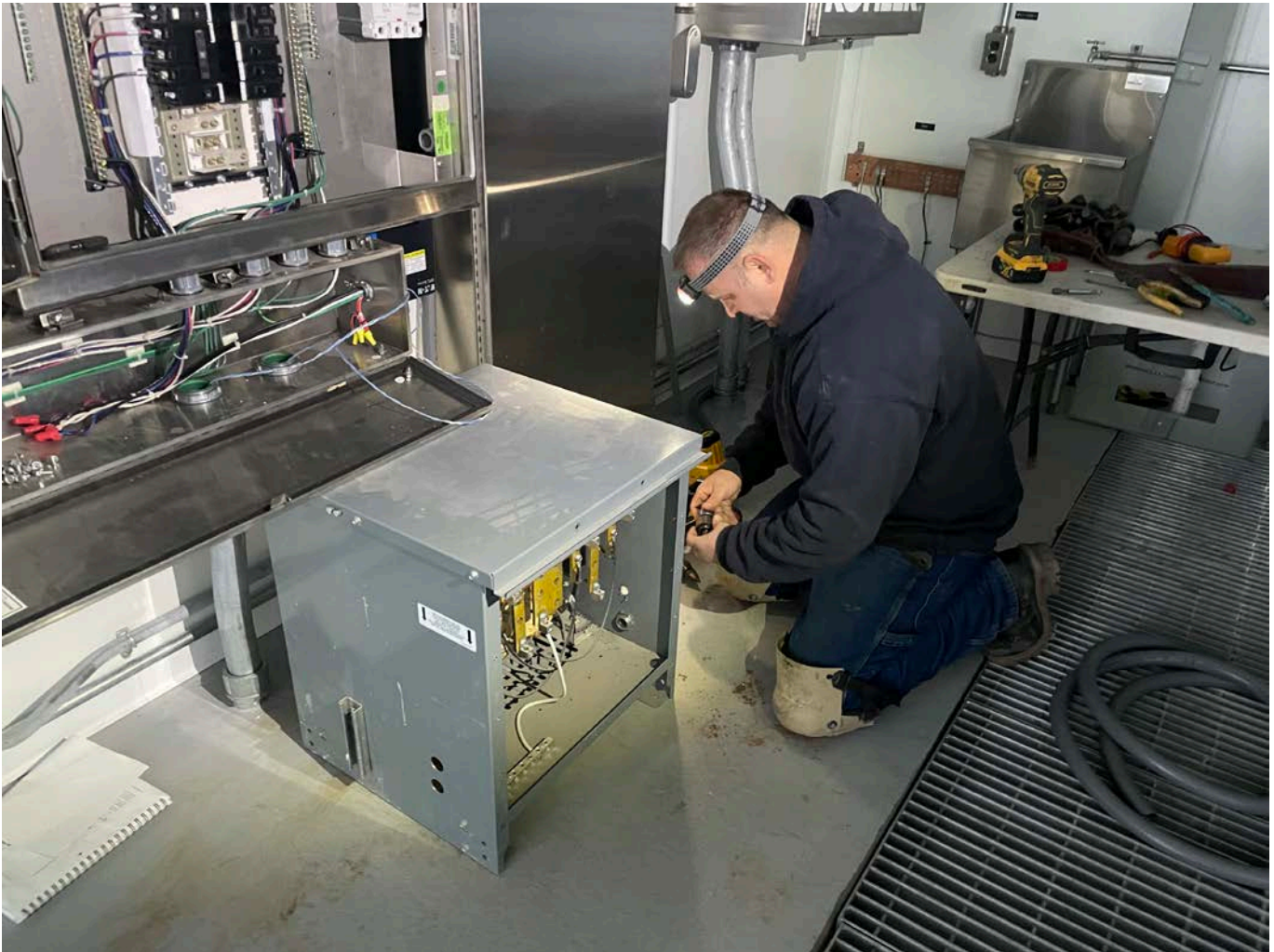
Picture 2: United Concrete wiring a temporary transformer to the booster station located at Station 750+63 on S. Main Street, Middletown. View to the northeast.
