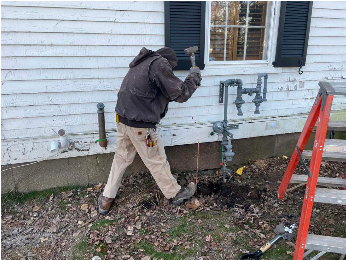
Picture 6: Apuzzo Electric in the process of installing one of two grounding rods they installed on the north side of the 313 Main Street, Durham, residence. View to the southwest.
