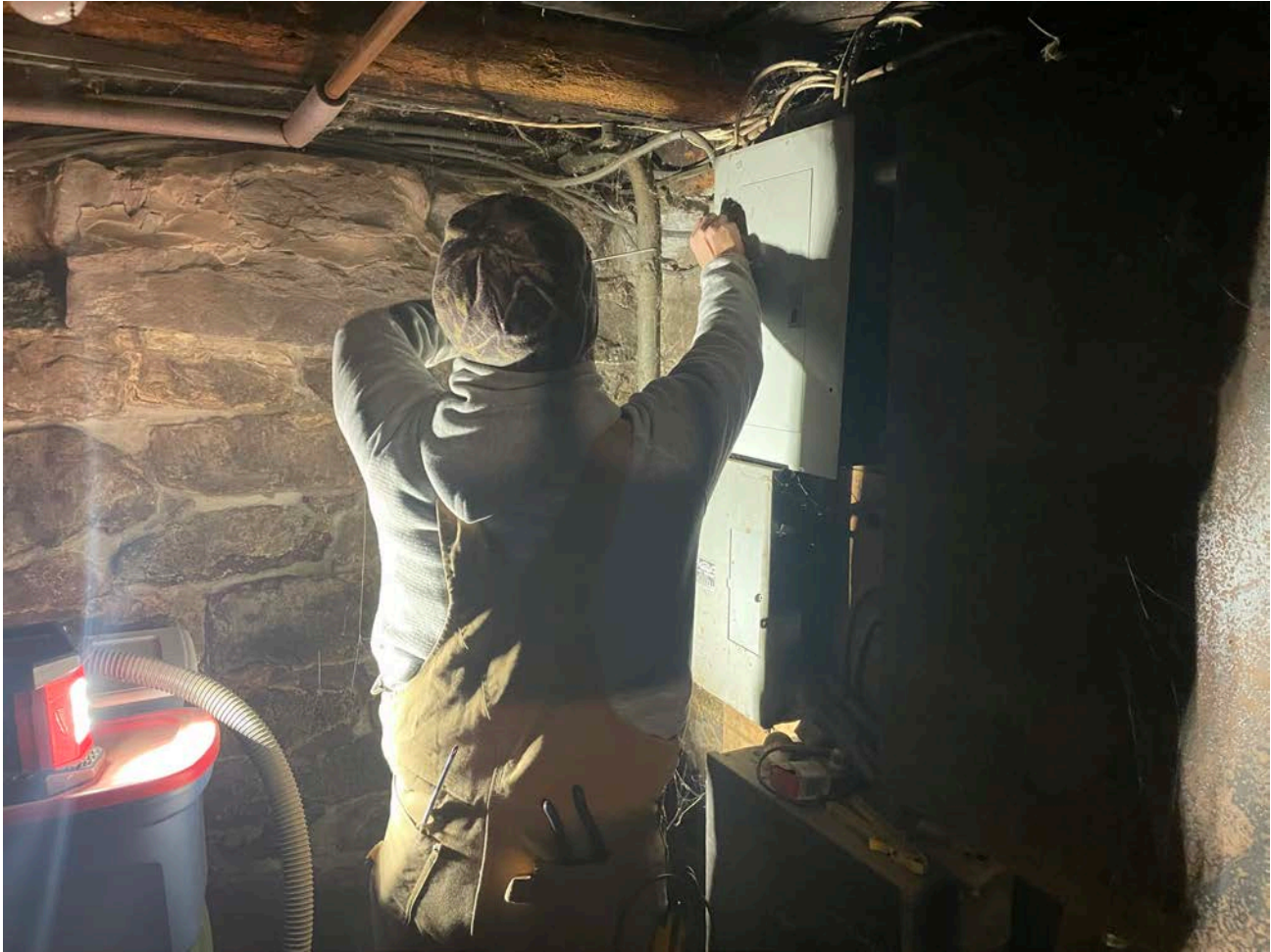
Picture 1: Apuzzo Electric installing new bonding wires to the recently installed water system components at the 110 Maple Avenue, Durham, residence.
