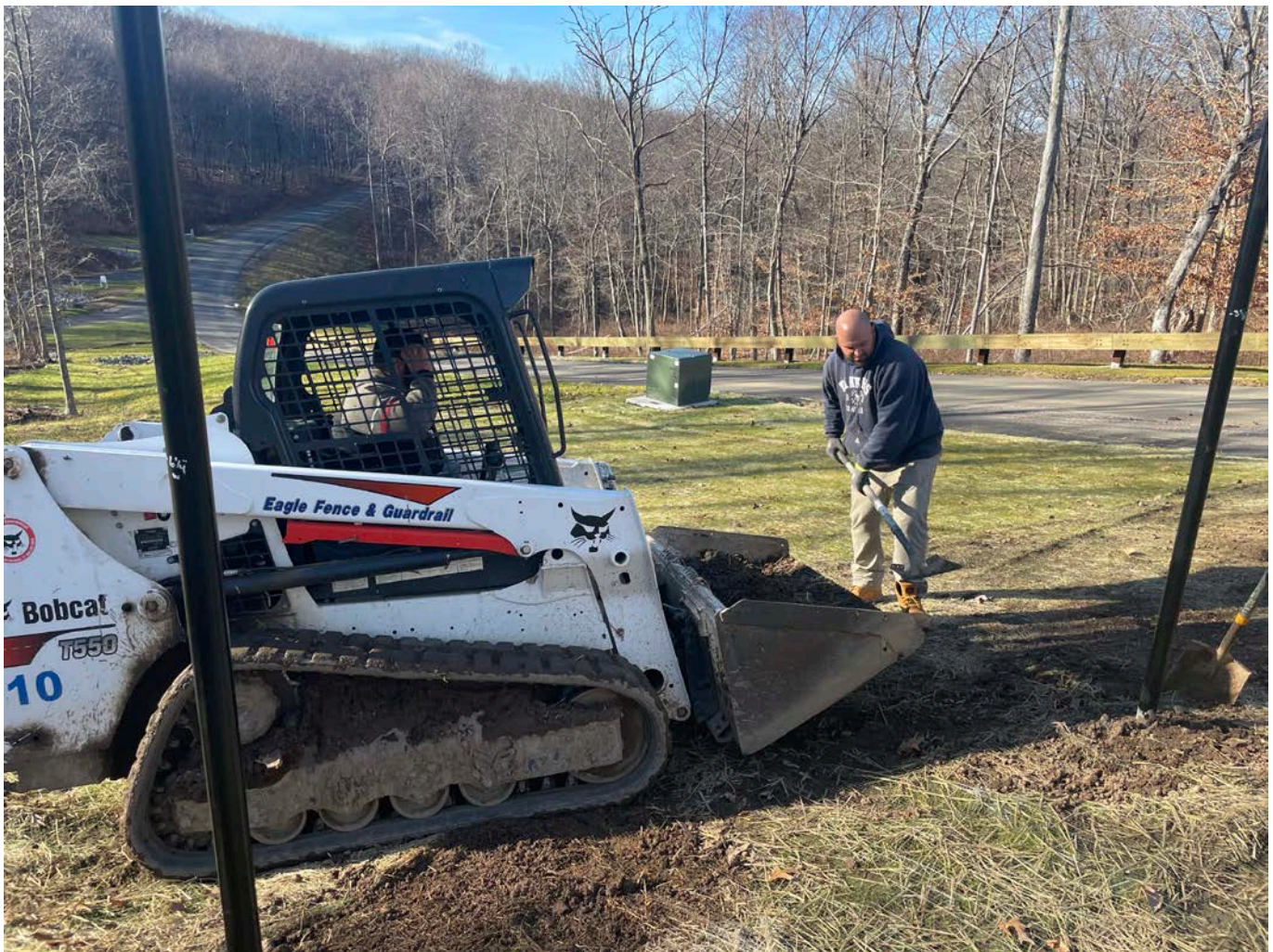
Picture 2: Eagle Fence and Guardrail placing soil that was displaced during the installation of the fence posts into the bucket of a bobcat to be moved elsewhere. View to the northwest.
