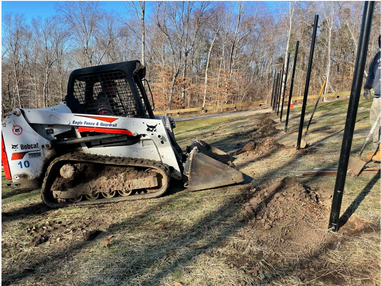
Picture 1: Eagle Fence and Guardrail grading soil around the fence posts they installed at the water tank work zone on December 16, 2021. View to the north.
