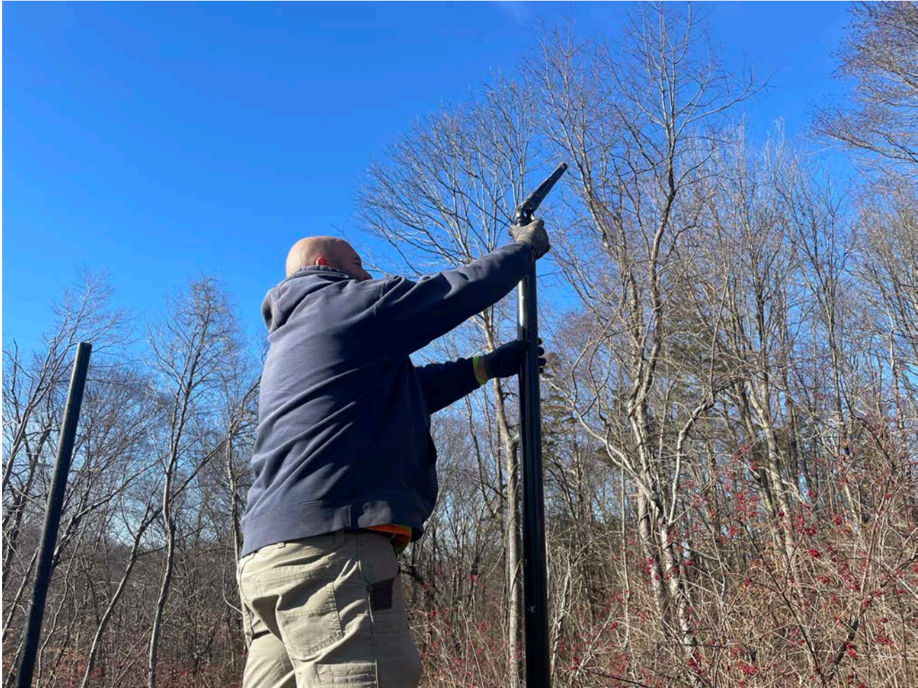
Picture 3: Eagle Fence and Guardrail placing a wire bracket on top of a fence post at the water tank work zone. View to the northwest.
