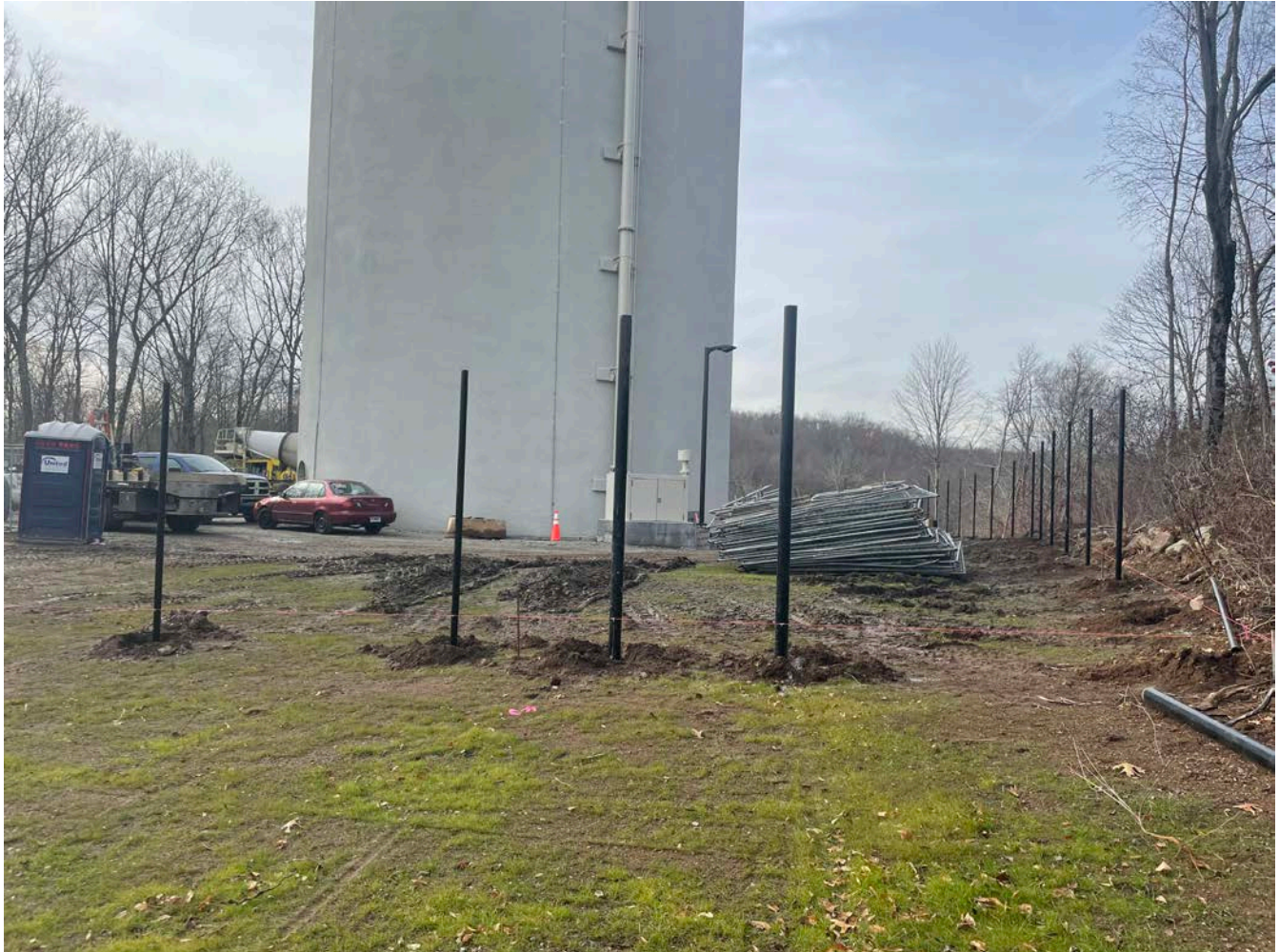
Picture 10: View of the fence posts that Eagle Fence and Guardrail have set into place on the east and north side of the water tank located east of the Shared Access Road in Middletown. View to the west.
