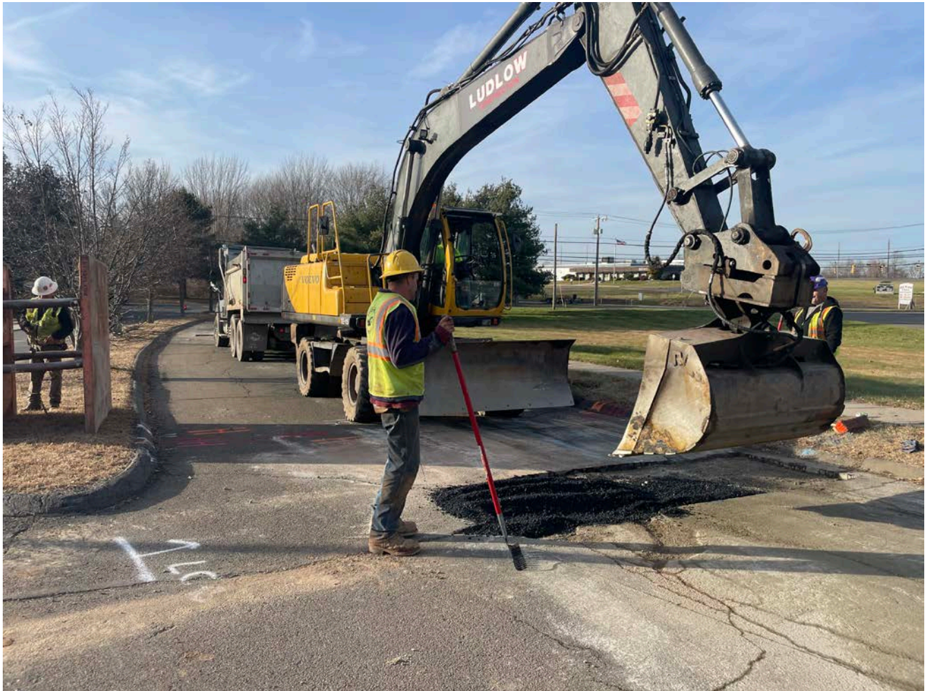
Picture 14: Ludlow placing asphalt over the backfilled trench they excavated at Station 754+13 on the westbound lane of Talcott Ridge Drive. View to the northwest.
