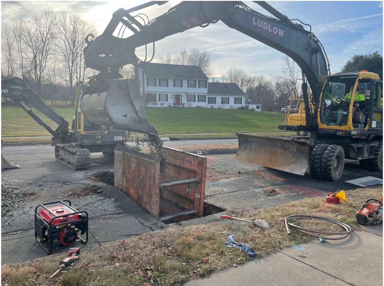
Picture 12: Ludlow placing sand over the 1" copper line they used to connect the curb stop at Station 754+13 to the 8" DIP water line that Ludlow previously installed on Talcott Ridge Drive.
