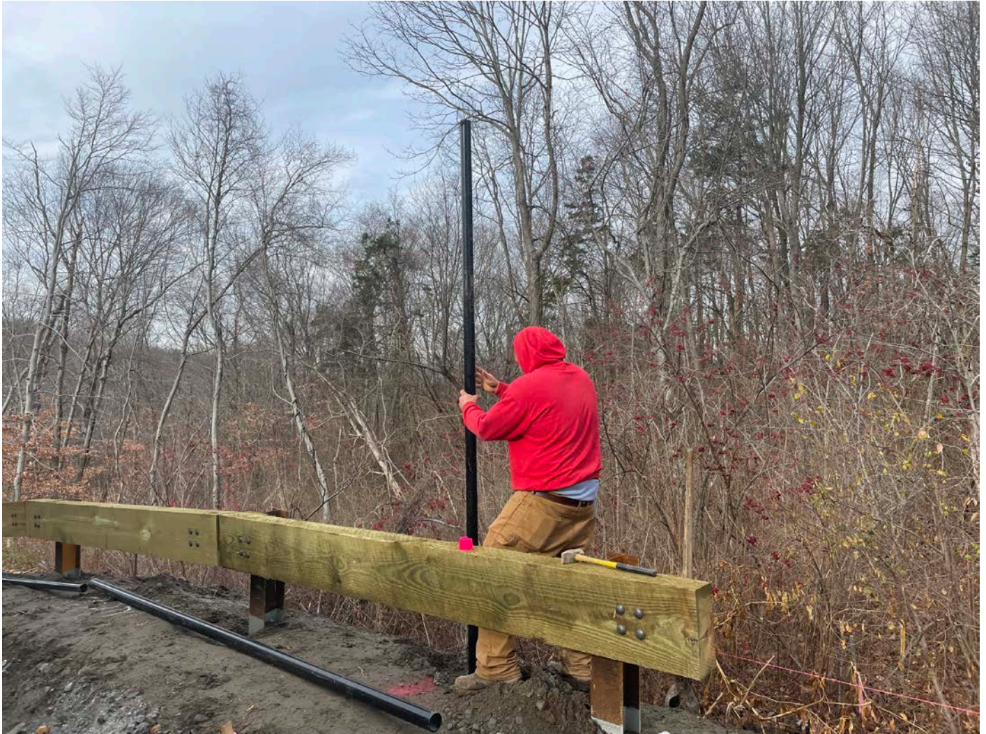
Picture 6: Eagle Fence and Guardrail installing a fence post at Station 10+50 on the north side of the Shared Access Driveway in Middletown.
