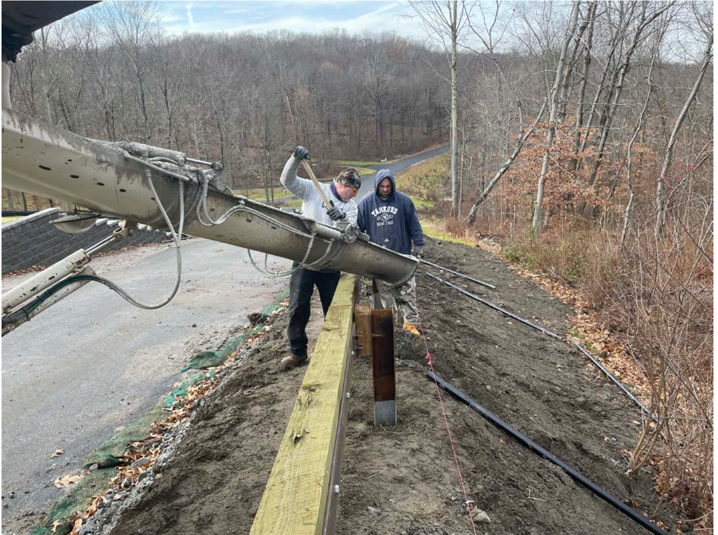
Picture 7: Eagle Fence and Guardrail guiding a Tilcon concrete truck as it places concrete into the holes that Eagle made for the installation of fence posts around the water tank and altitude valve vault located east of the Shared Access Driveway in Middletown.
