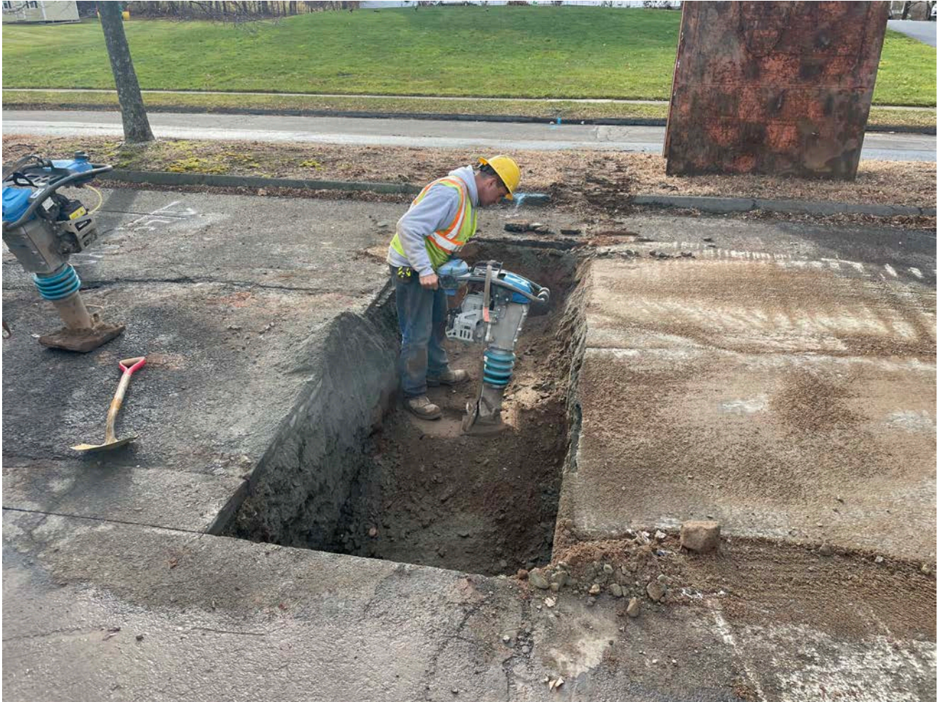
Picture 8: Ludlow compacting backfill they placed in 1' lifts at Station 753+68 on the westbound lane of Talcott Ridge Drive in Middletown. View to the south.
