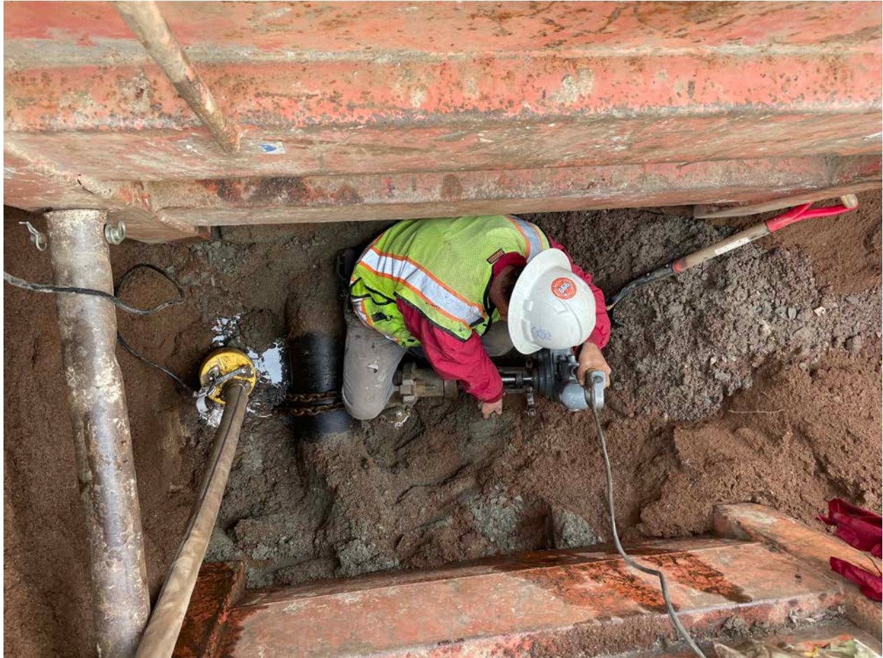
Picture 4: Ludlow tapping the new 8" DIP line that Ludlow previously installed on the westbound lane of Talcott Ridge Drive for the installation of a corporation stop.
