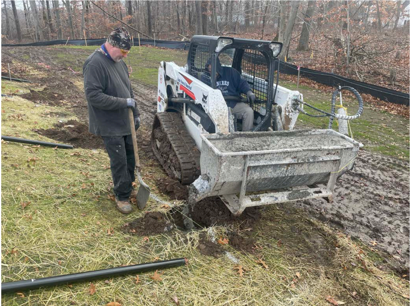
Picture 9: Eagle Fence and Guardrail placing concrete into the holes they made for the installation of fence posts at the water tank work zone. View to the southeast.
