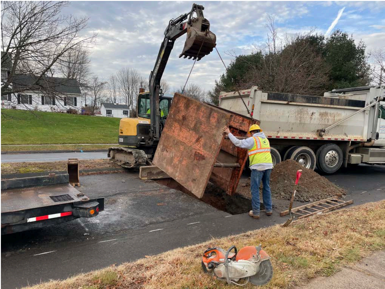
Picture 3: Ludlow placing a trench box in the excavation they made at Station 753+68 as they prepare to migrate water service for the 9 Talcott Ridge Drive residence from the old City waterline to the new 8" DIP line that Ludlow installed. View to the southwest.
