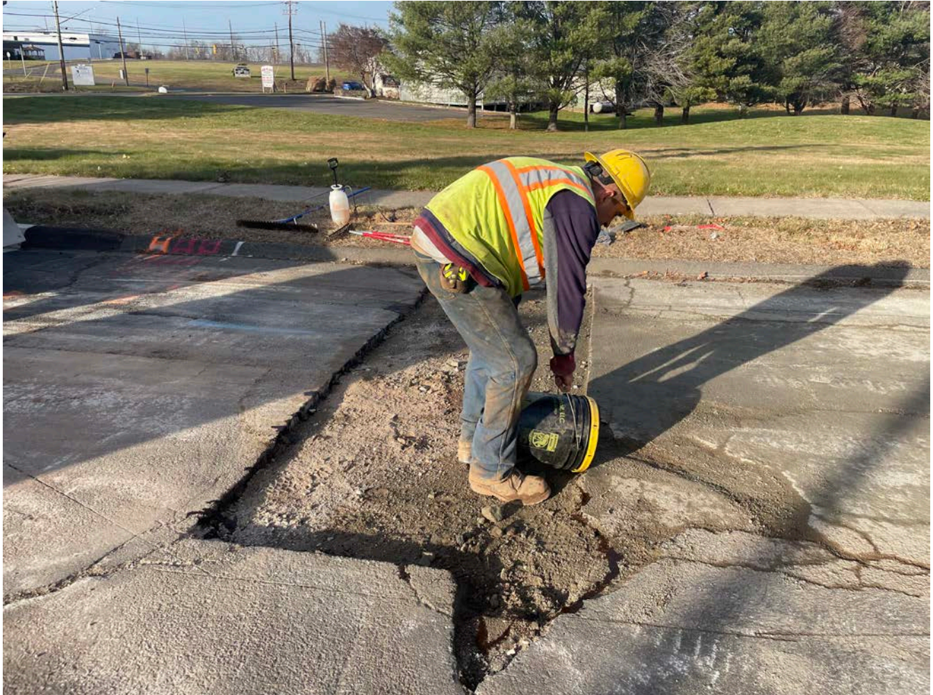
Picture 13: Ludlow placing tack coat on the cut edges of pavement where they excavated at Station 754+13 on the westbound lane of Talcott Ridge Drive. View to the northwest.
