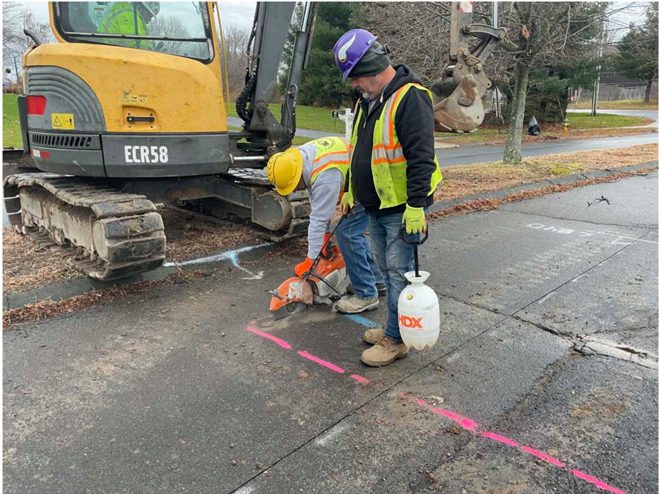
Picture 1: Ludlow saw-cutting pavement at Station 753+68 as they prepare to migrate water service for the 9 Talcott Ridge Drive residence from the old City waterline to the new 8" DIP line that Ludlow installed. View to the southwest.
