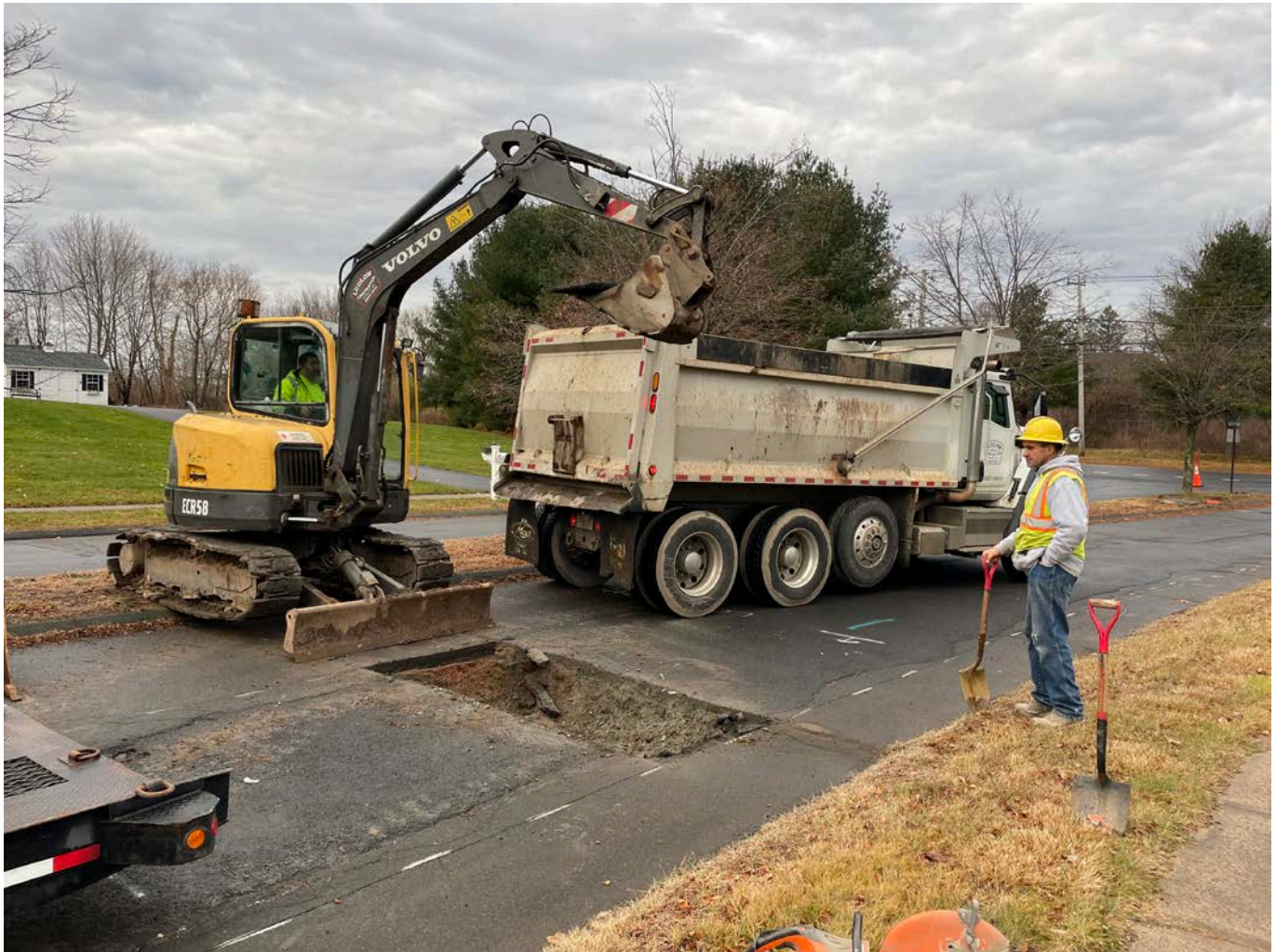
Picture 2: Ludlow excavating at Station 753+68 as they prepare to migrate water service for the 9 Talcott Ridge Drive residence from the old City waterline to the new 8" DIP line that Ludlow installed. View to the southwest.
