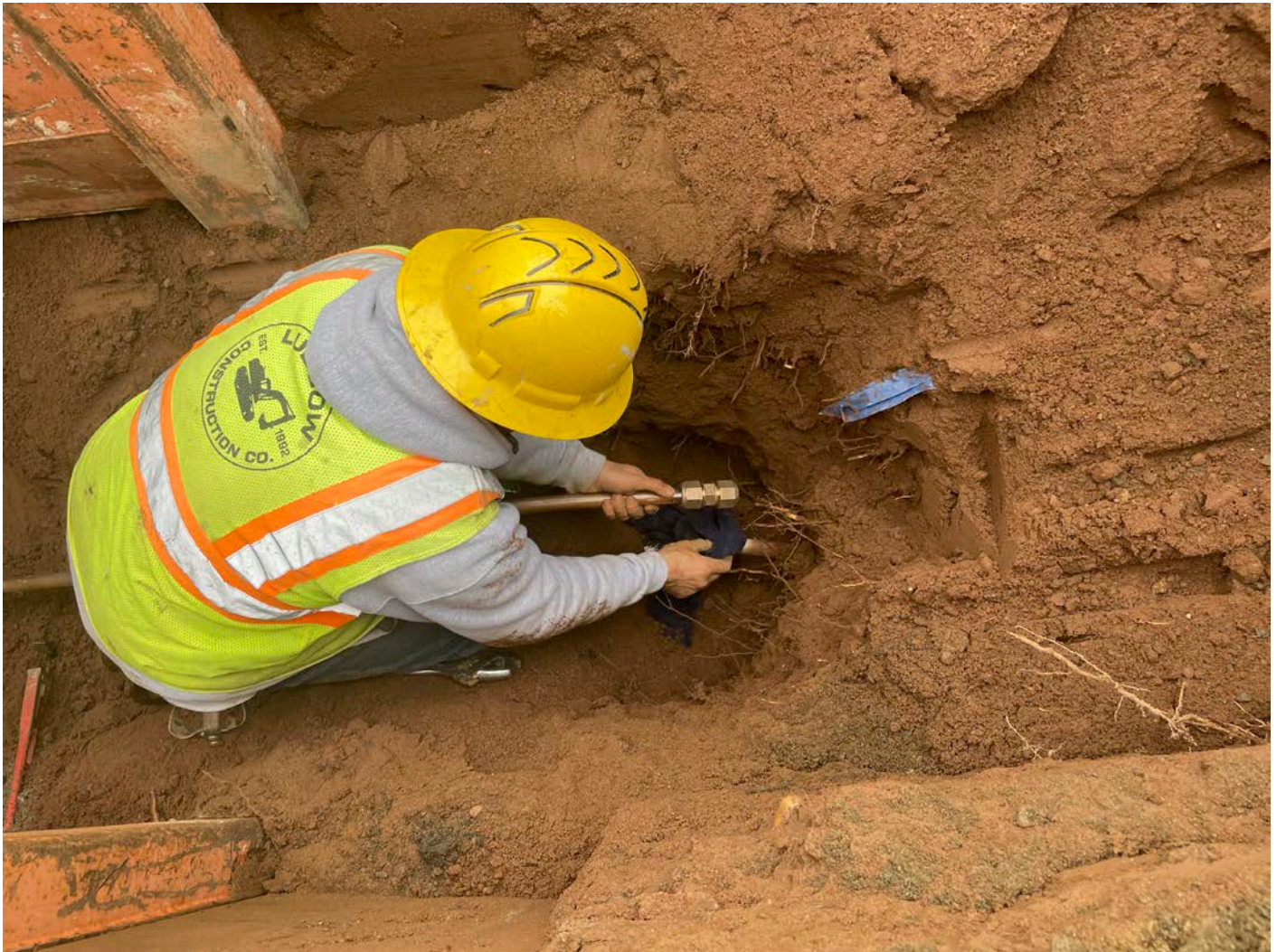
Picture 5: Ludlow connecting a 1" copper water service line they just attached to the 8" DIP line that Ludlow previously installed on the westbound lane of Talcott Ridge Drive to the 9 Talcott Ridge Drive residence service line.
