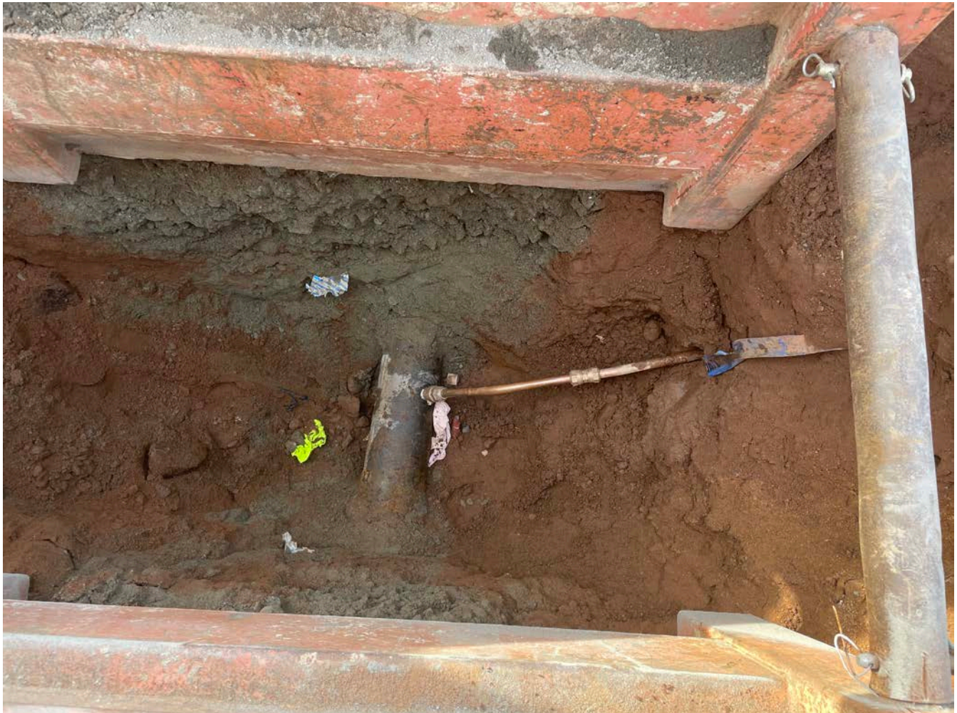
Picture 11: Connection that Ludlow made between the curb stop at Station 754+13 and the 8" DIP water line that Ludlow previously installed on Talcott Ridge Drive.
