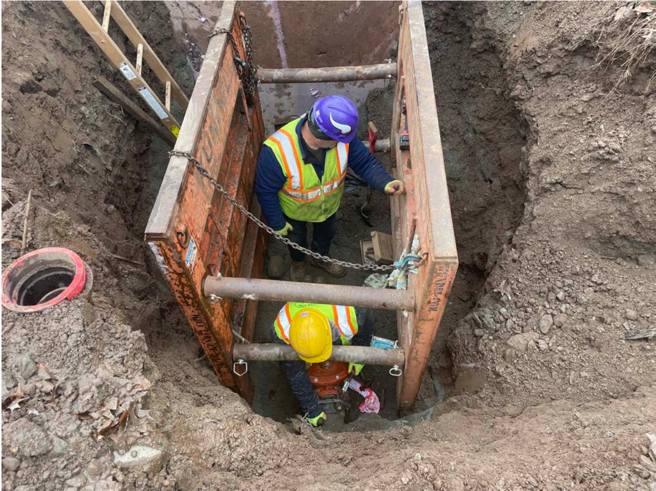
Picture 3: Ludlow removing the 6" gate valve located approximately 8' south of the altitude valve vault after having broken one of the bolts on the valve, necessitating its replacement. View to the north.
