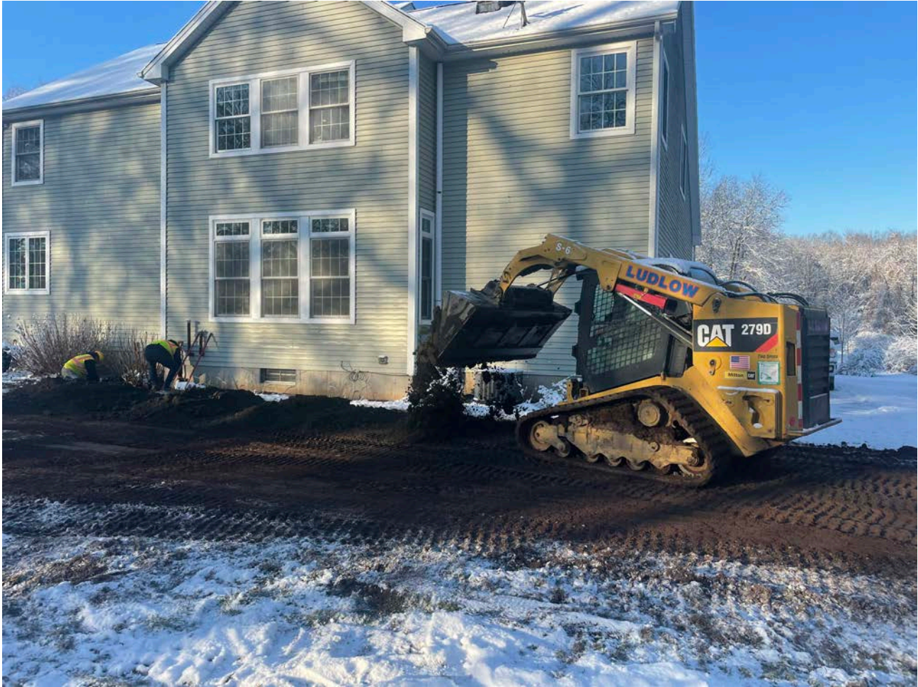
Picture 1: Ludlow placing loam on the east side of the 93R Maiden Lane property as they work to restore those portions of the property that were disturbed during the installation of a 1" copper water service line. View to the southwest.
