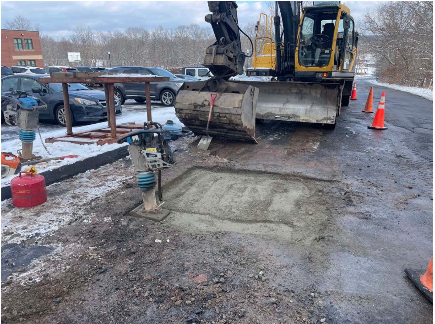
Picture 7: Ludlow has just finished backfilling the excavation they made on the westbound lane of Pickett Lane at Station 503+90 after removing a 1" copper blow-off line that they no longer need. View to the east.
