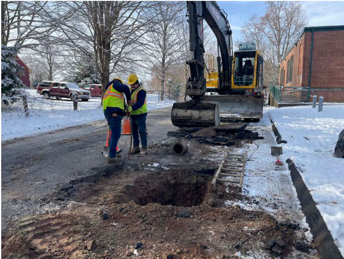
Picture 4: Ludlow opening up the westbound lane of Pickett Lane at Station 503+90 to access and remove a 1" copper blow-off line that they no longer have a need for. View to the west.
