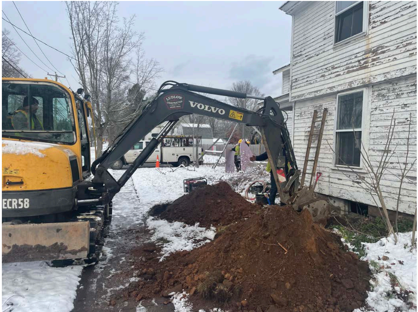
Picture 9: Ludlow excavating on the west side of the 275 Main Street residence for the 1" copper water service line. View to the northeast.
