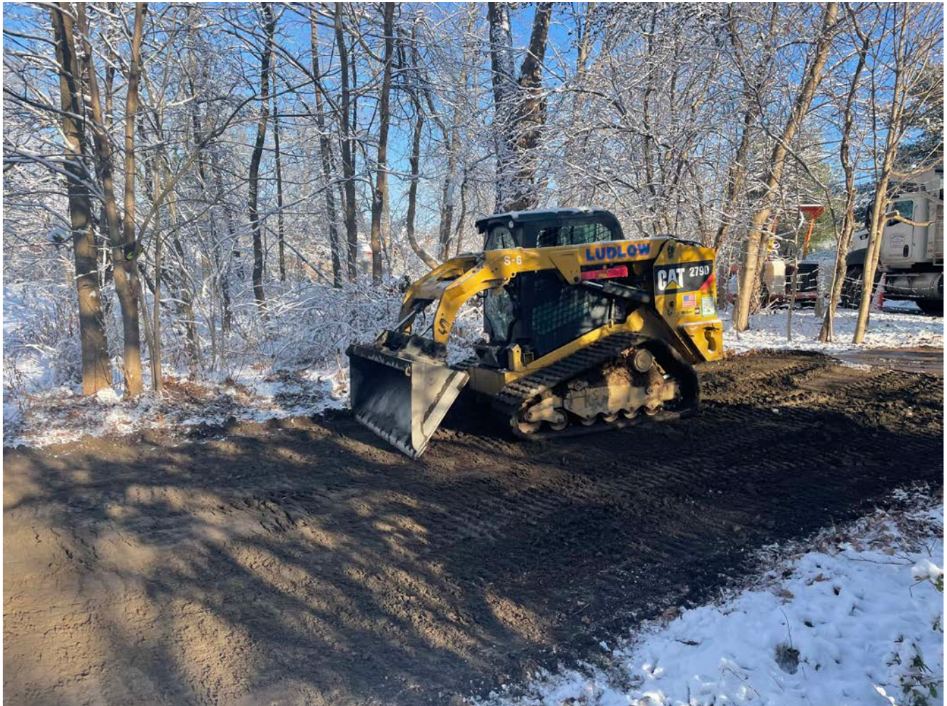
Picture 2: Ludlow grading loam at the 93R Maiden Lane property as they work to restore those portions of the property that were disturbed during the installation of a 1" copper water service line. View to the northeast.
