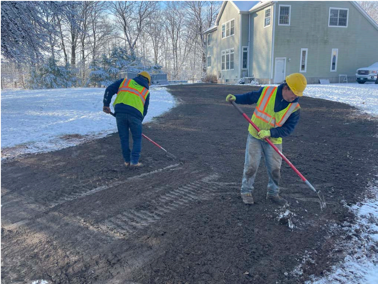
Picture 3: Ludlow raking out loam on the 93R Maiden Lane property as they work to restore those portions of the property that were disturbed during the installation of a 1" copper water service line. View to the southwest.
