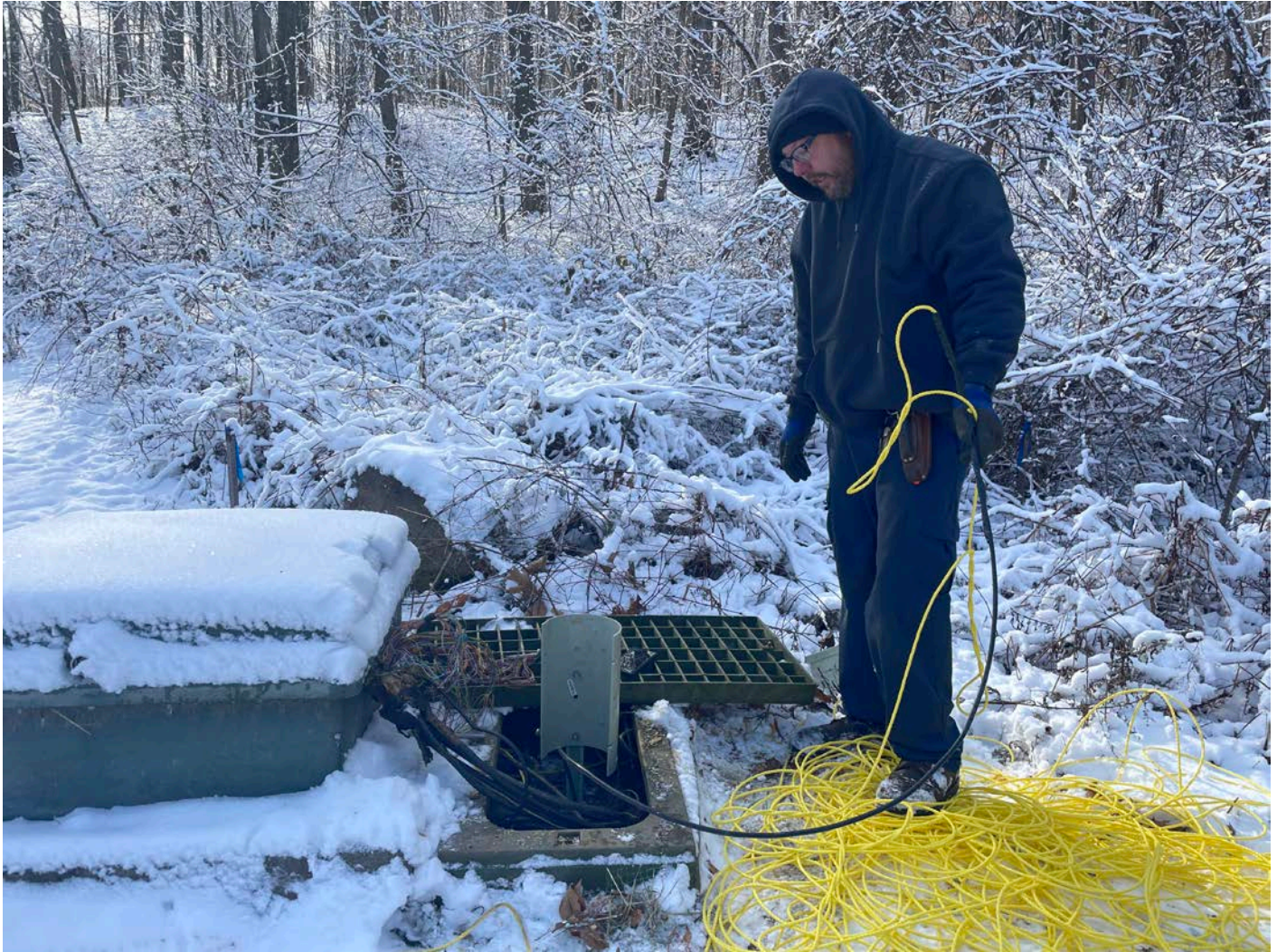
Picture 5: Frontier after having pulled communication lines from the electrical enclosure located on the north side of the altitude valve vault to the RPC located on the west side of the driveway for 224 Talcott Ridge Drive and the south side of the Shared Access Driveway. View to the south.
