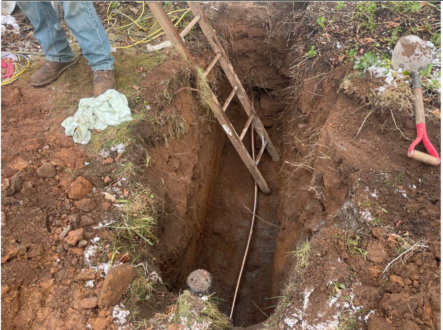
Picture 10: Trench that Ludlow excavating on the west side of the 275 Main Street residence for the 1” copper water service line. View to the east.
