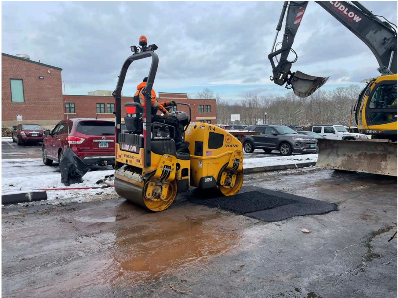
Picture 8: Ludlow compacting asphalt they just placed on the eastbound lane of Pickett Lane at Station 503+90 after removing a 1" copper blow-off line. View to the northeast.
