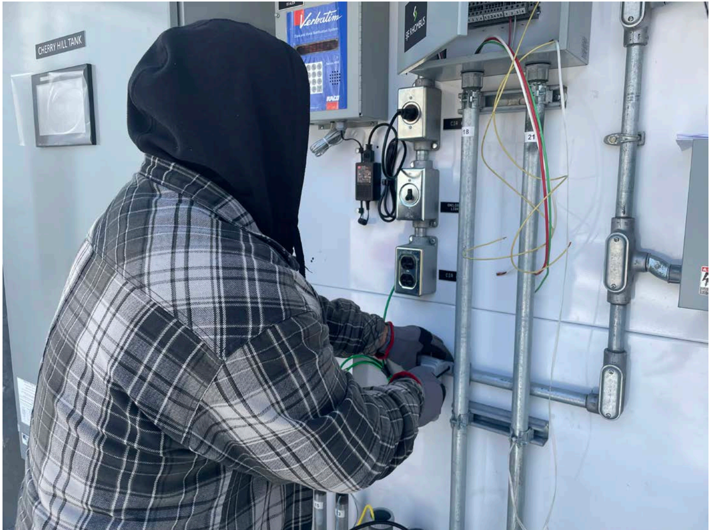
Picture 6: Frontier connecting communication lines to the electrical enclosure located on the north side of the altitude vault. View to the south.
