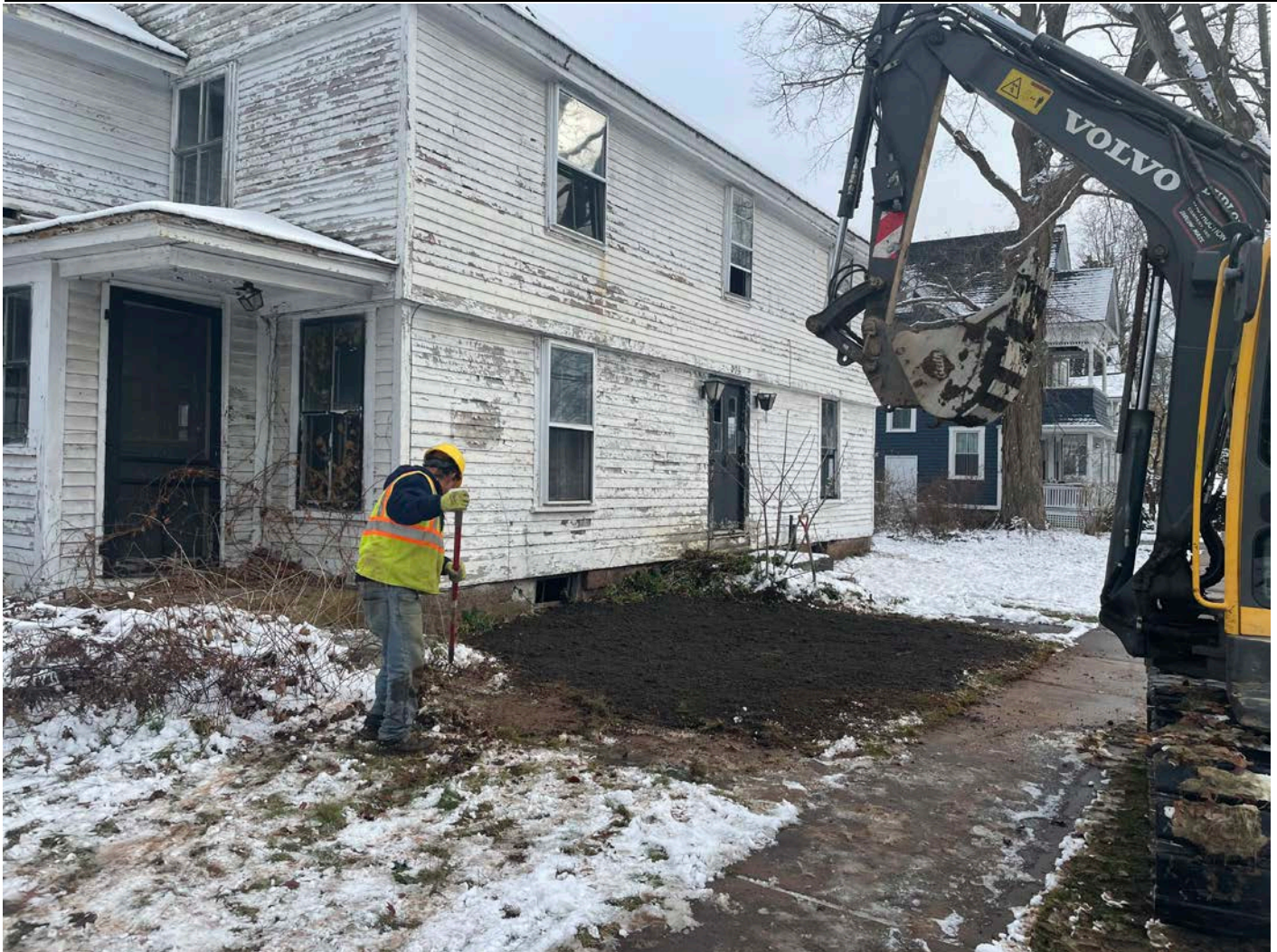
Picture 12: Ludlow raking out loam over the area that was disturbed during the installation of a 1" copper water service line they installed at the 275 Main Street property. View to the southeast.
