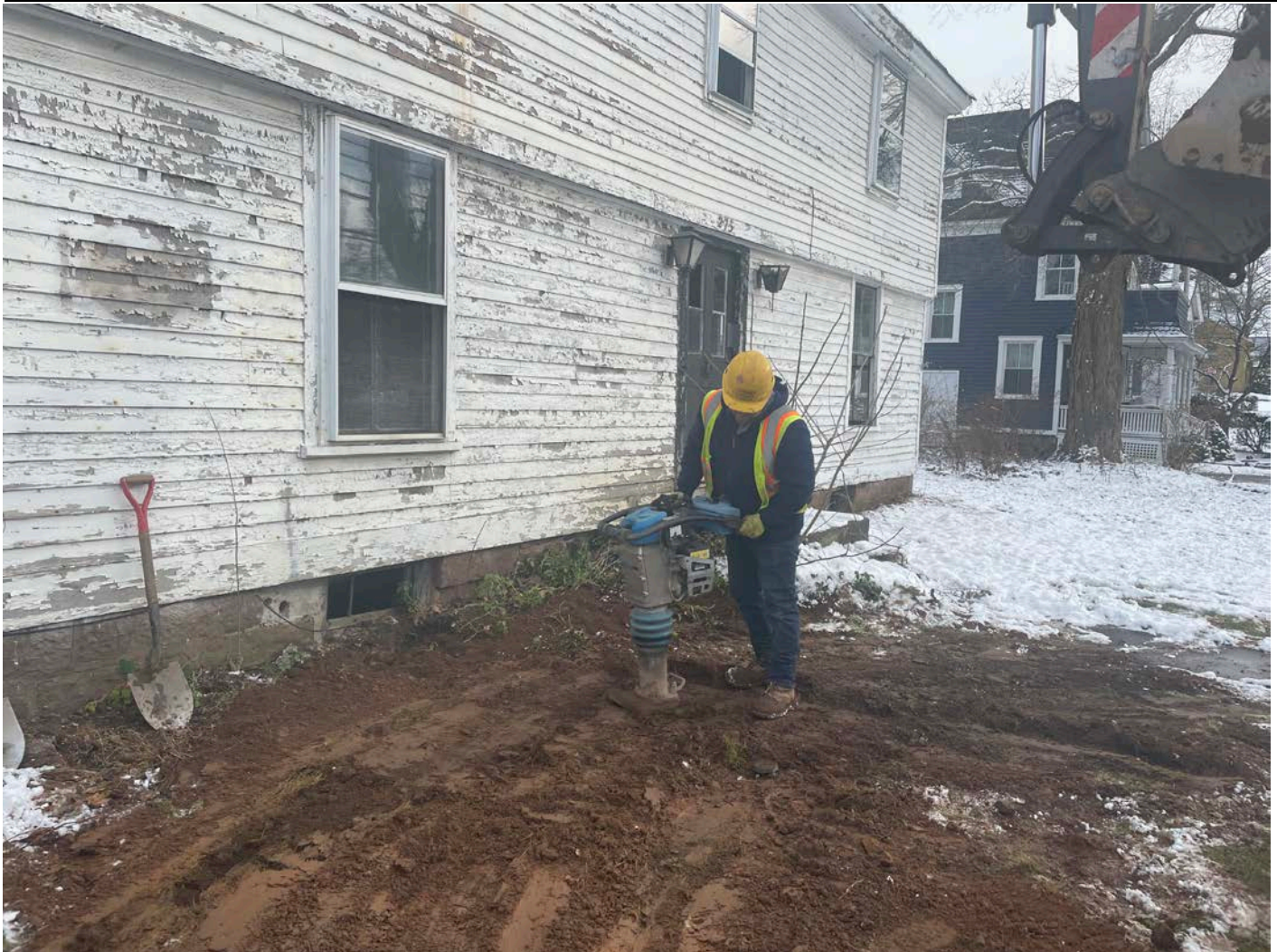
Picture 11: Ludlow compacting fill they placed over the 1" copper water service line they installed at the 275 Main Street property. View to the southwest.
