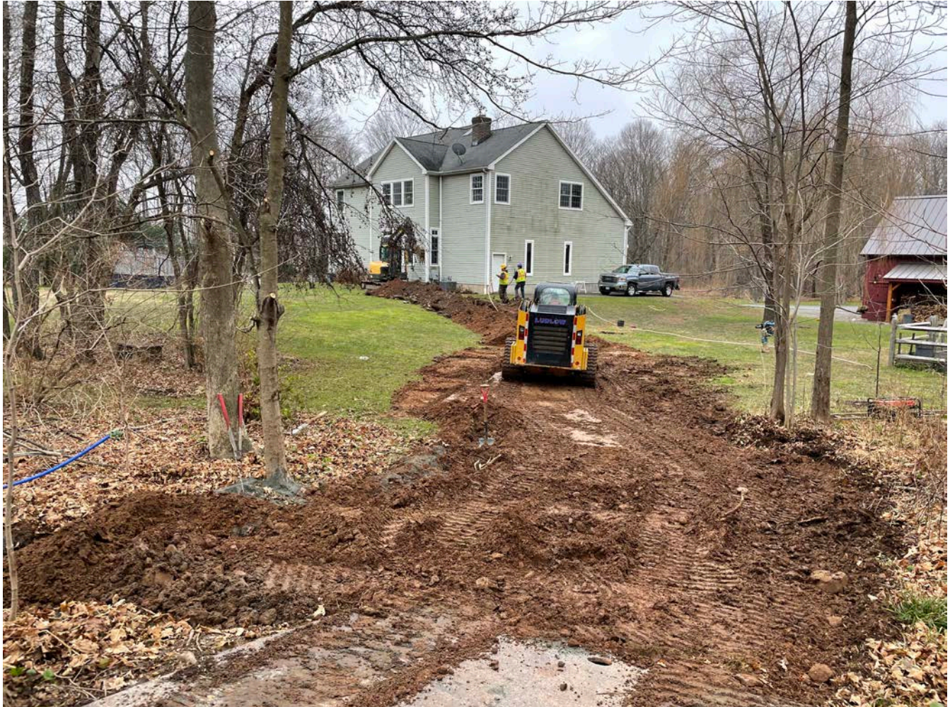
Picture 9: Ludlow backfilling over the of the 1” copper water service line that they are installing at the 93R Maiden Lane residence. View to the southwest.
