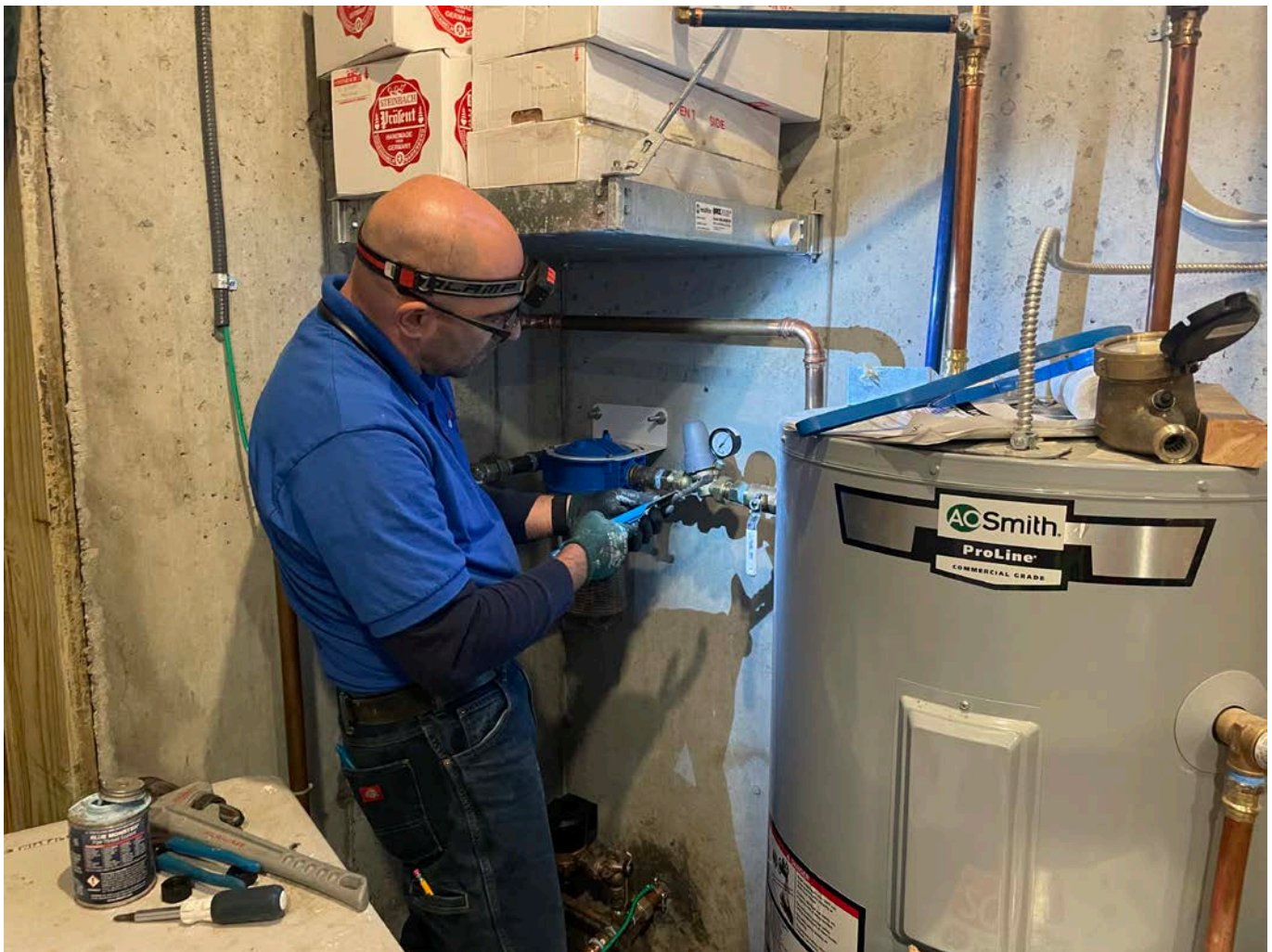
Picture 2: Fazzino Plumbing replacing brass tees that were part of the final water service components that were previously installed at the 174 Main Street residence.
