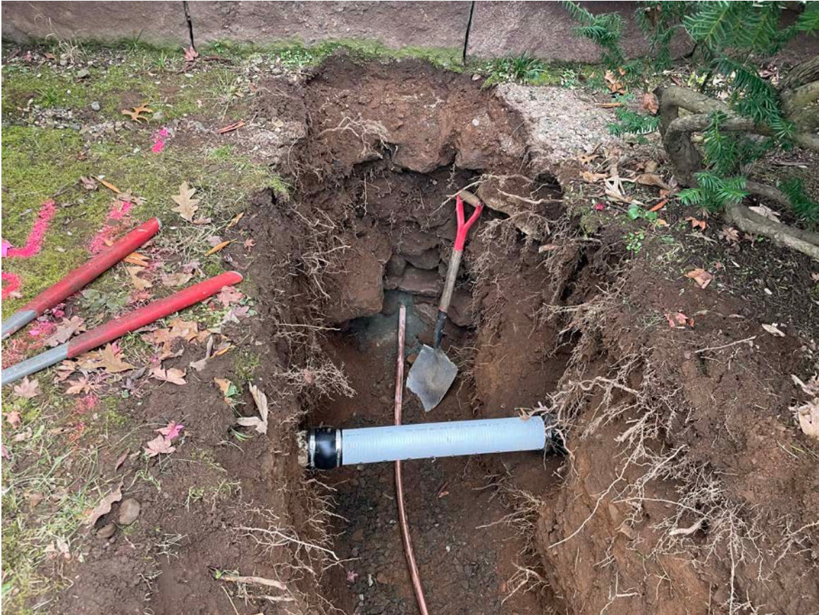
Picture 4: Ludlow has also repaired a 4" perforated PVC drain pipe on the east side of the 123 Maiden Lane residence's foundation with a new piece of perforated PVC and two Fernco boots. View to the west.
