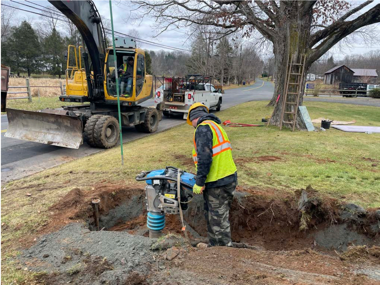
Picture 3: Ludlow compacting native fill in the trench they are backfilling at the 123 Maiden Lane property after the installation of a 1" copper water service line. View to the east.
