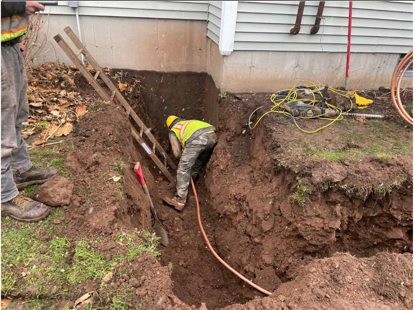
Picture 10: Ludlow inserting 1" copper water service line through a hole they drilled on the east side of the foundation for the 93R Maiden Lane residence. View to the west.
