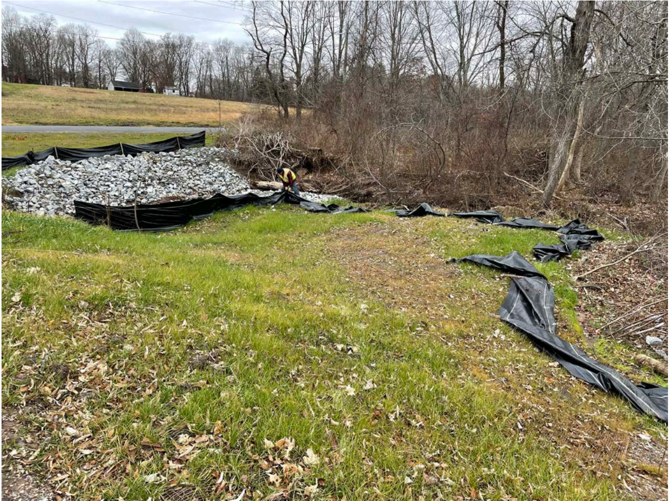
Picture 8: Ludlow removing the silt fence they previously placed on either side of Ball Brook on the north side of Maiden Lane during the Maiden Lane stream crossing.
