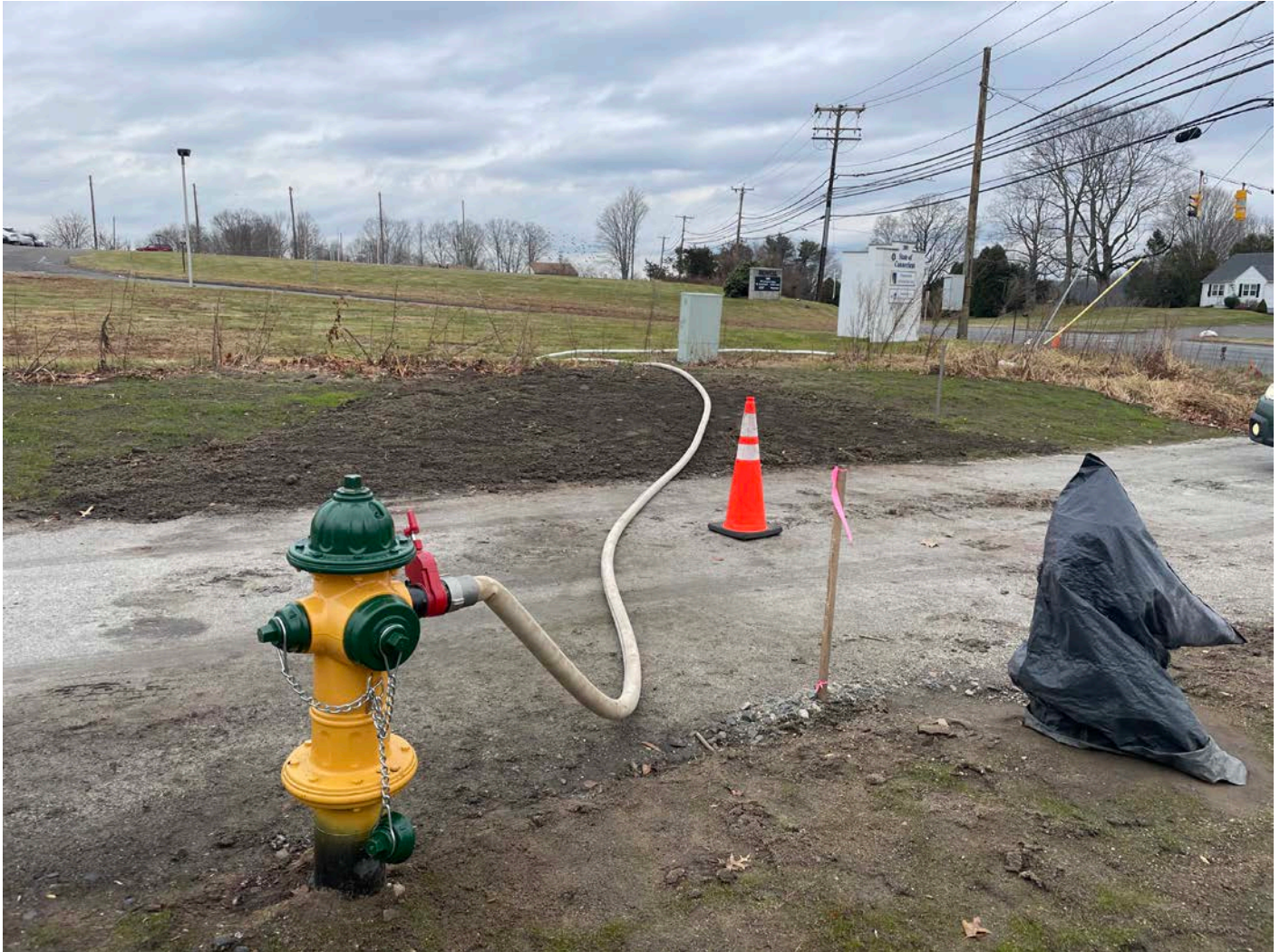
Picture 5: Ludlow purging the 8" DIP waterlines located on the east side of the booster station. The purged water is being directed into a storm drain located on the north side of the booster station driveway. View to the northeast.
