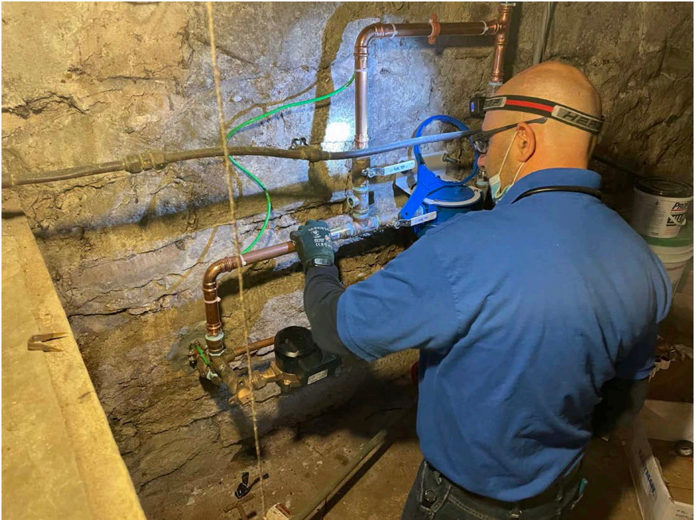
Picture 6: Fazzino Plumbing replacing brass tees that were part of the final water service components that were previously installed at the 265 Main Street residence.
