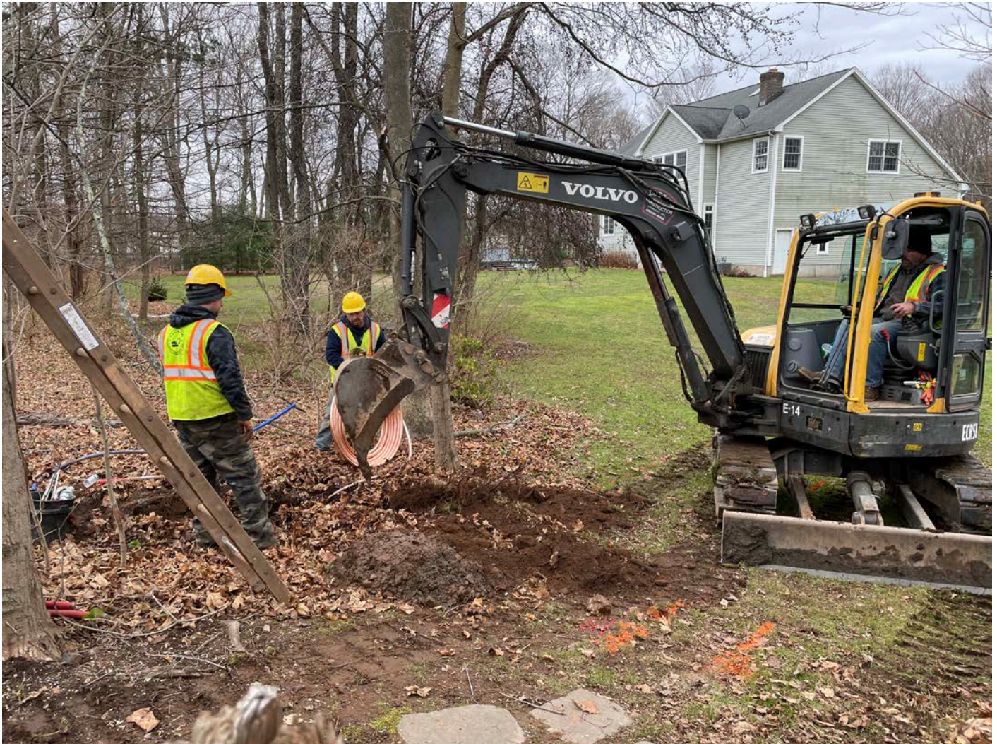
Picture 7: Ludlow beginning to excavate on the west side of the curb stop of the 93R Maiden Lane residence for the installation of a 1" copper water service line. View to the southwest.
