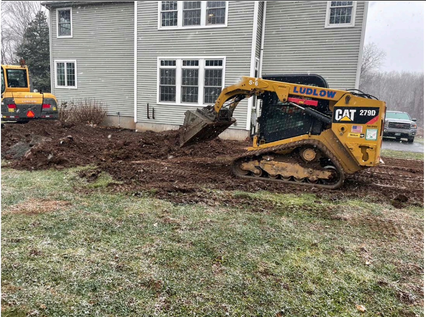
Picture 11: Ludlow grading fill they placed over the 1" copper water service line they installed at the 93R Maiden Lane property. View to the southwest.
