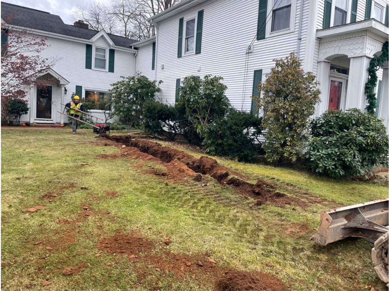
Picture 1: Ludlow excavating a trench for the installation of a 1" copper water service line on the east side of the 123 Maiden Lane residence. View to the southwest.
