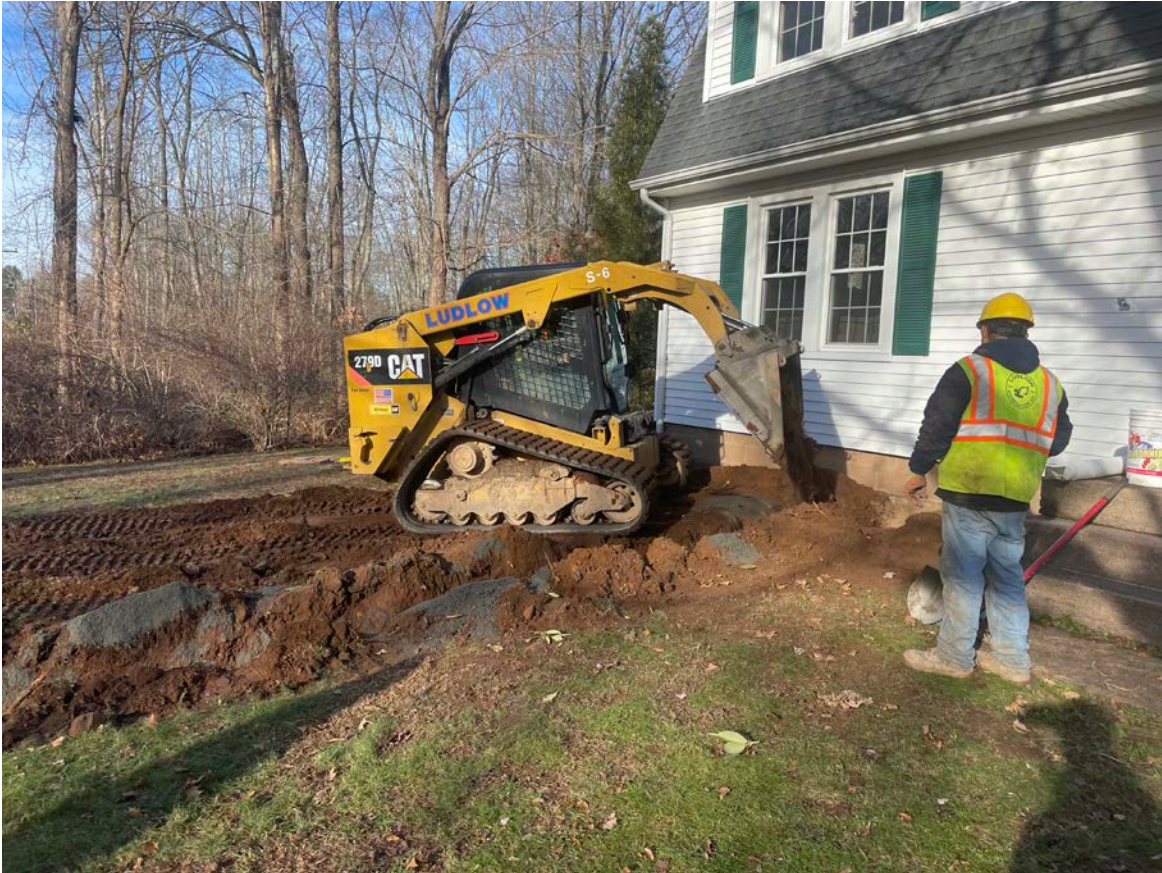
Picture 4: Ludlow placing sand over the 1" copper water service line they installed at the 110 Maiden Lane property. View to the west.
