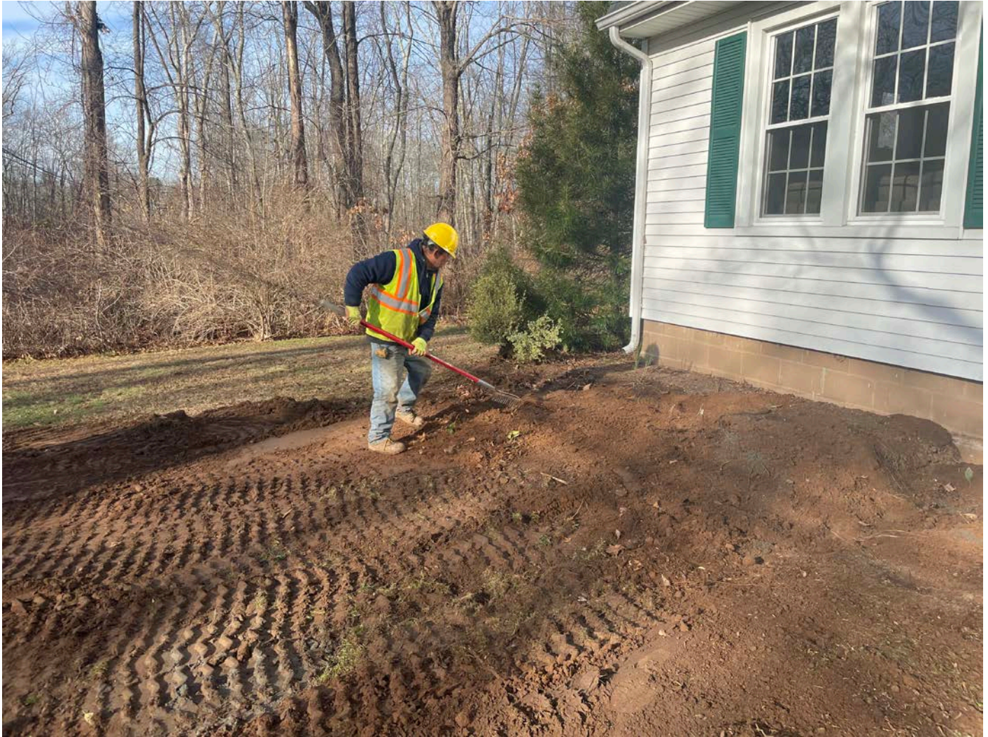
Picture 5: Ludlow raking out loam that they placed on the southside of the 110 Maiden Lane residence to restore those areas that were disturbed by the installation of a 1" copper water service line. View to the west.
