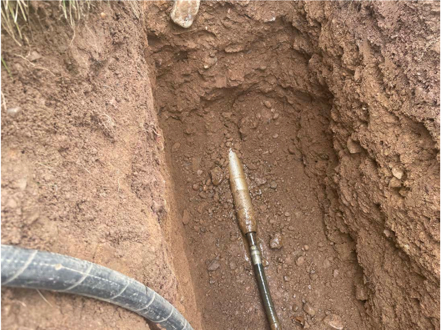
Picture 7: Pneumatic mole that Ludlow is using to make a hole beneath the sidewalk of the 105 Maiden Lane residence for the installation of a 1" copper water service line. View to the north.
