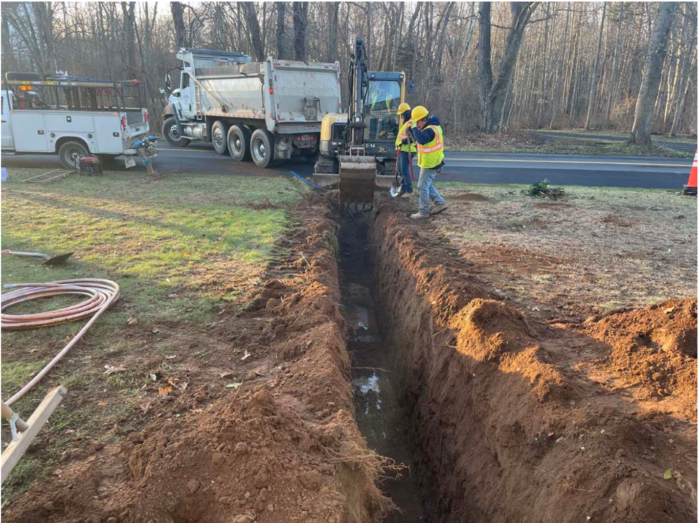
Picture 2: Ludlow excavating a trench for the installation of a 1" copper water service line on the south side of the 110 Maiden Lane residence. View to the south.
