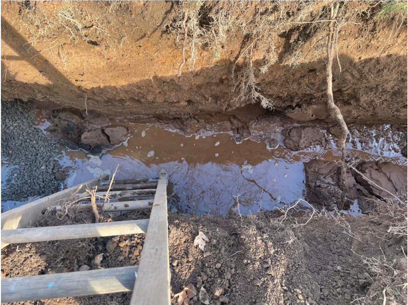
Picture 8: Water that was observed in the bottom of the trench that Ludlow is excavating at the 105 Maiden Lane property for the installation of a 1" copper water service line.
