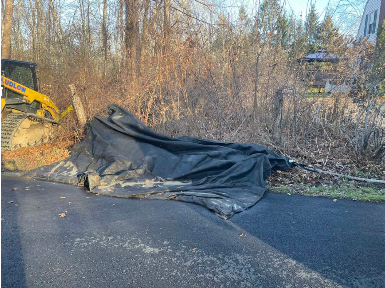
Picture 3: Silt bag that Ludlow placed on the north side of Maiden Lane to discharge water being pumped from the trench they are excavating at the 110 Maiden Lane property for the installation of a 1" copper water service line. View to the north.
