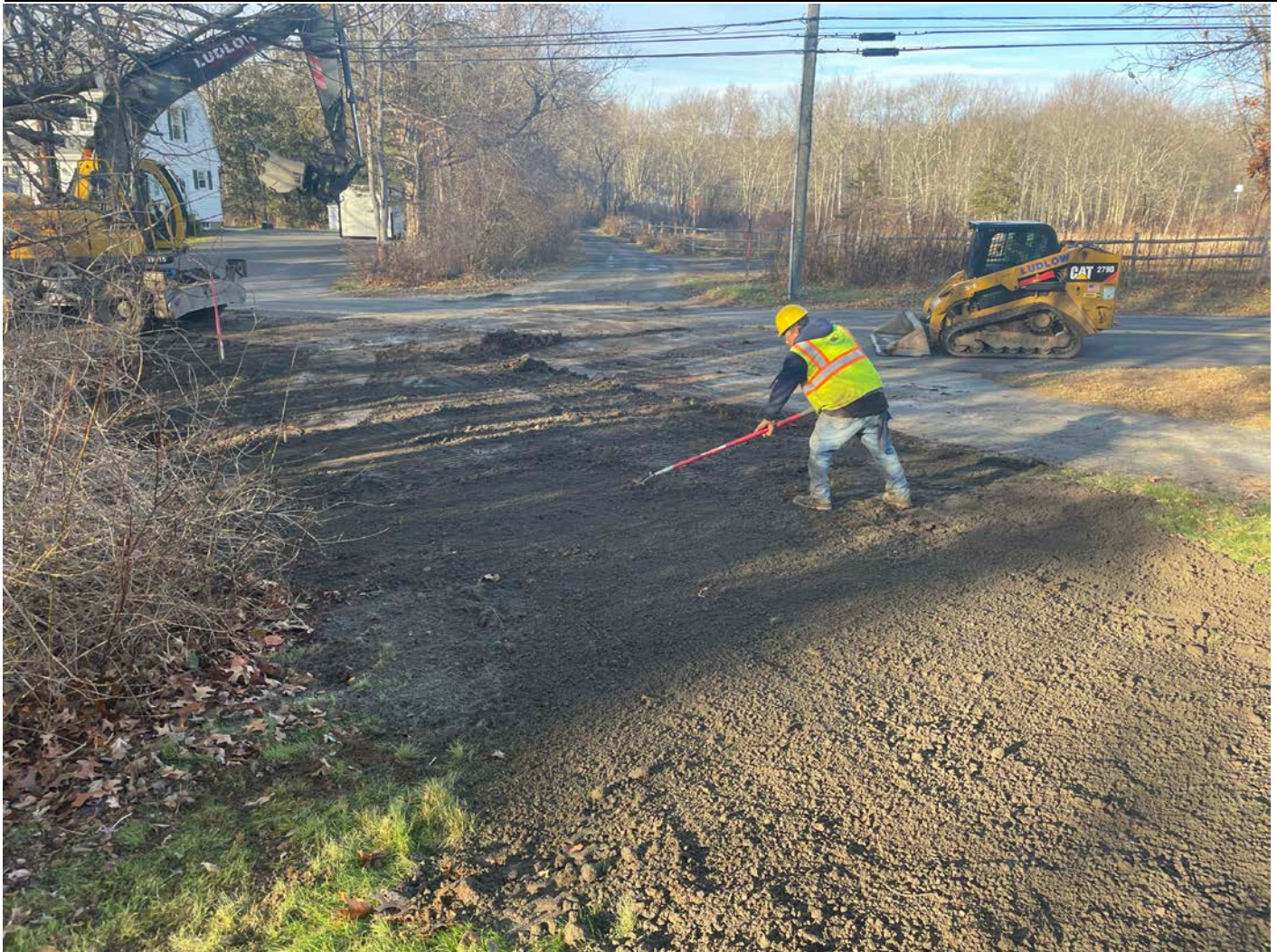
Picture 11: Ludlow raking loam at the 105 Maiden Lane property as they work to restore those portions of the property that were disturbed by the installation of a 1" copper water service line. View to the north.
