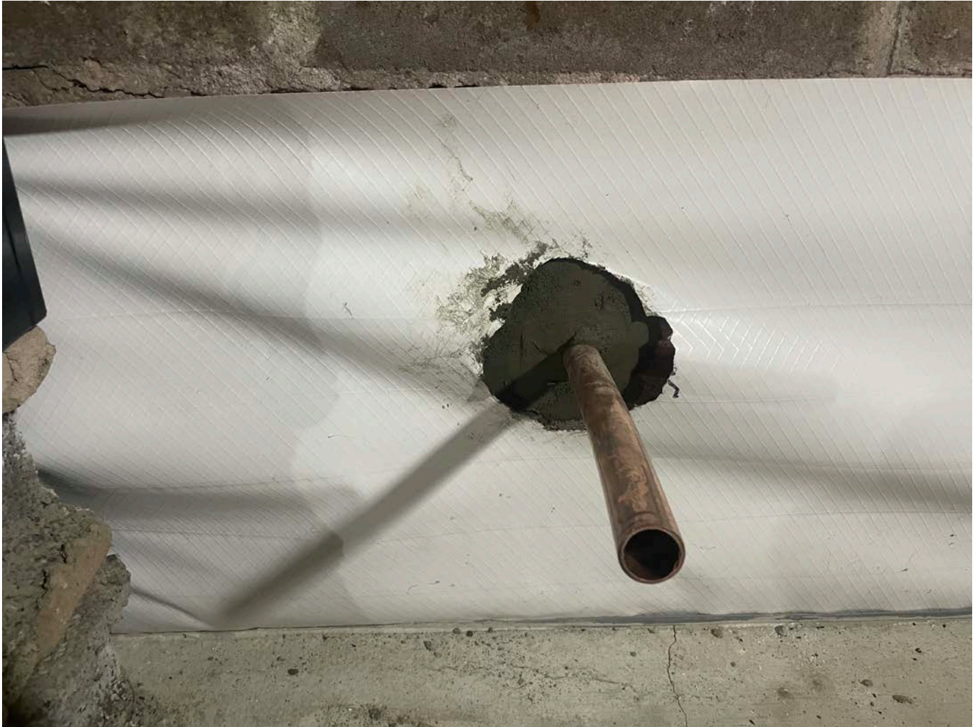
Picture 6: 1" copper water service line that Ludlow inserted through the southern foundation of the 110 Maiden Lane residence and secured in place with non-shrink grout. View to the south.
