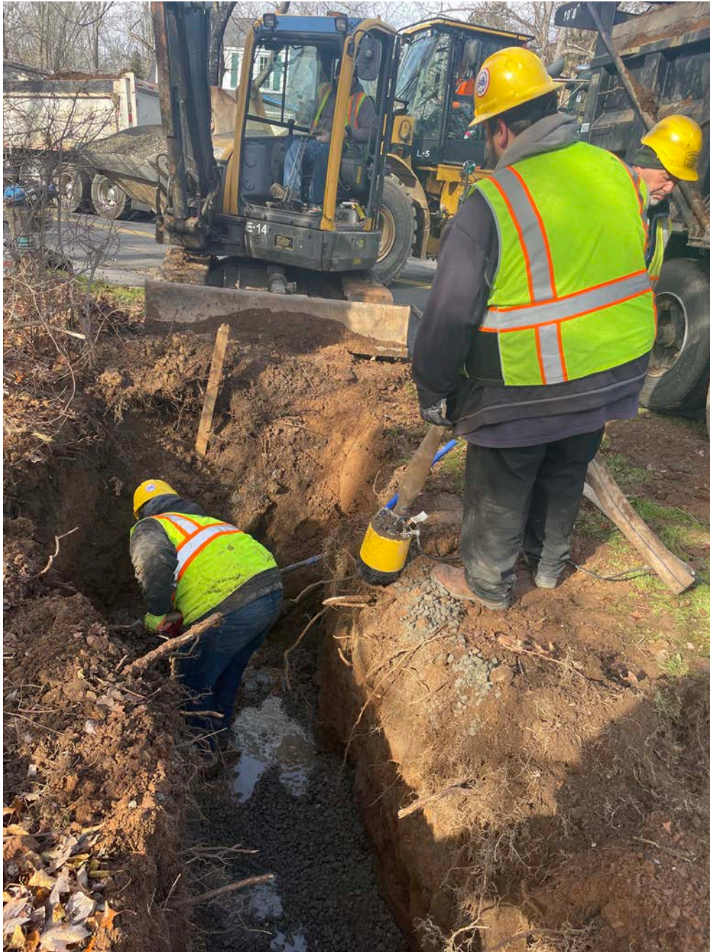
Picture 9: Ludlow preparing to set a pump in the trench they excavated at the 105 Maiden Lane property for the installation of a 1" copper water service line. View to the southwest.
