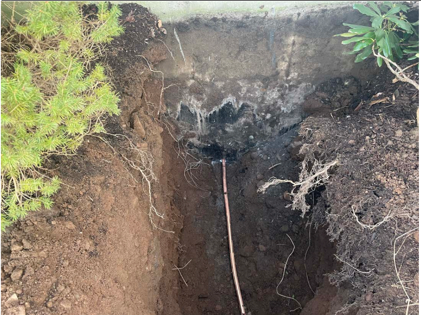
Picture 10: 1" copper water service line that Ludlow has passed through the penetration they made on the northern foundation of the 105 Maiden Lane residence and secured in place with non-shrink grout. View to the north.
