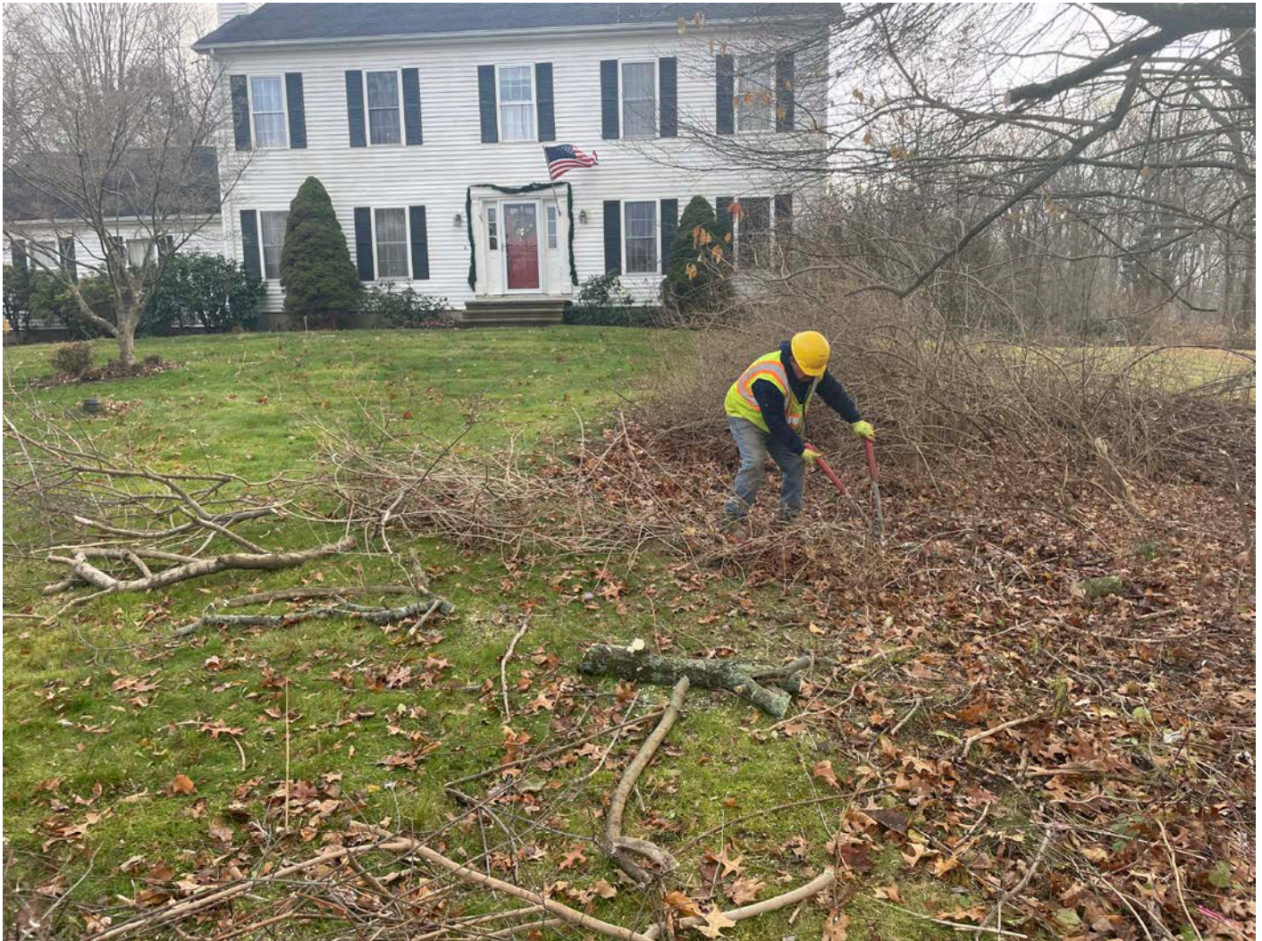
Picture 10: Ludlow clearing brush at the 105 Maiden Lane property as they begin to clear a path for the installation of a copper water service line. View to the south.
