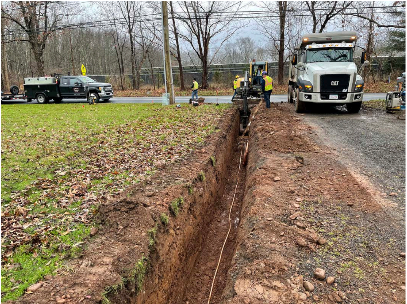
Picture 2: Ludlow excavating a trench for the installation of the 1" copper water line shown in the foreground. View to the south.
