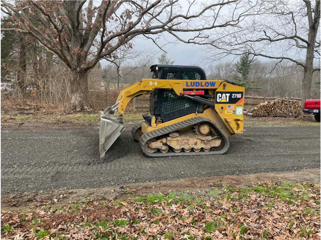
Picture 8: Ludlow grading the \frac{3}{4} " processed gravel they used to restore the driveway at the 78 Maiden Lane property after they installed a 1" copper water service line. View to the west.
