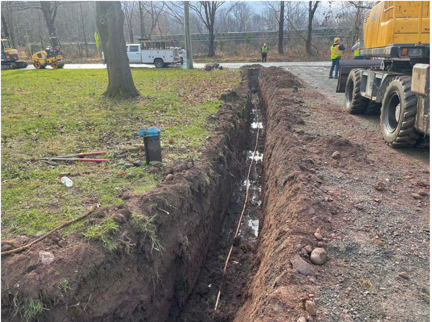
Picture 6: 1" copper water service line that Ludlow has connected to the curb stop at the south end of the trench at the 78 Maiden Lane property. View to the south.
