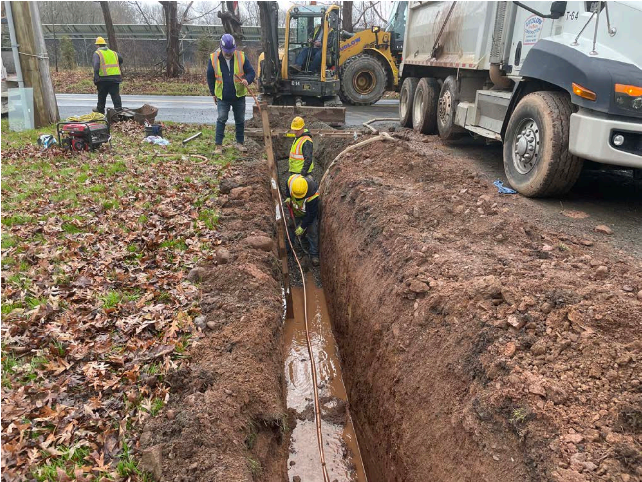
Picture 3: Ludlow placing a pump that has been set in \frac{3}{4} " gravel in the trench they are working in at the 78 Maiden Lane property as they install a 1" copper water service line. View to the south.
