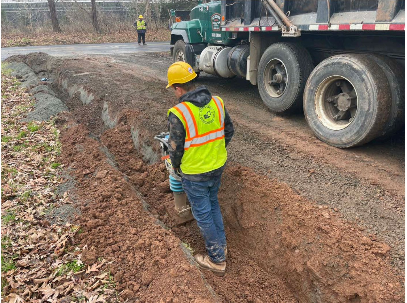
Picture 7: Ludlow using a jumping jack to compact the native fill being used to backfill the trench that Ludlow excavated at the 78 Maiden Lane property. View to the south.
