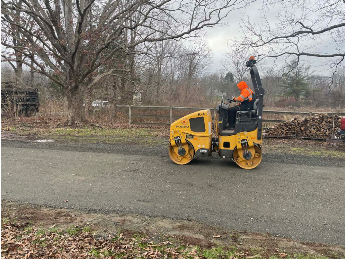
Picture 9: Ludlow compacting the ¾" processed gravel they used to restore the driveway at the 78 Maiden Lane property after they installed a 1" copper water service line. View to the southwest.
