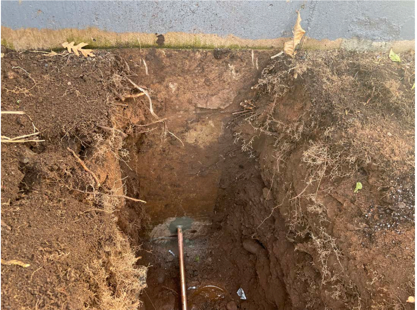
Picture 5: 1" copper water service line that Ludlow has secured in place as it passes through the western foundation of the 78 Maiden Lane residence. View to the east.
