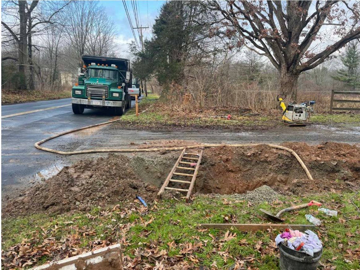
Picture 4: Ludlow pumping water from the trench they excavated at 78 Maiden Lane into a silt bag placed west of the driveway and north of Maiden Lane. View to the west.
