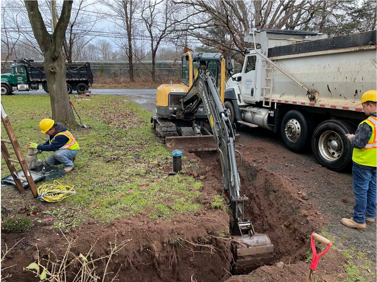
Picture 1: Ludlow excavating a trench for the installation of a 1" copper water service line at the 78 Maiden Lane property. View to the south.
