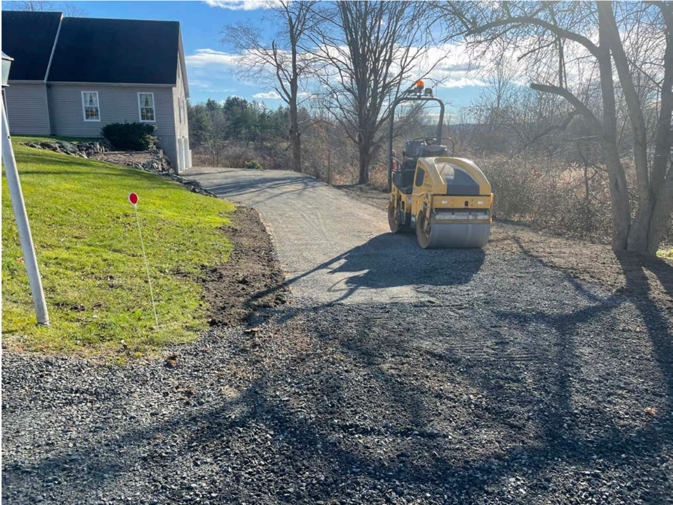
Picture 3: A portion of the driveway at the 14 Talcott Lane property where Ludlow has placed and rolled \frac{3}{4} " gravel as they work to restore those portions of the property that were disturbed during the installation of a 2" copper water service line. View to the south.
