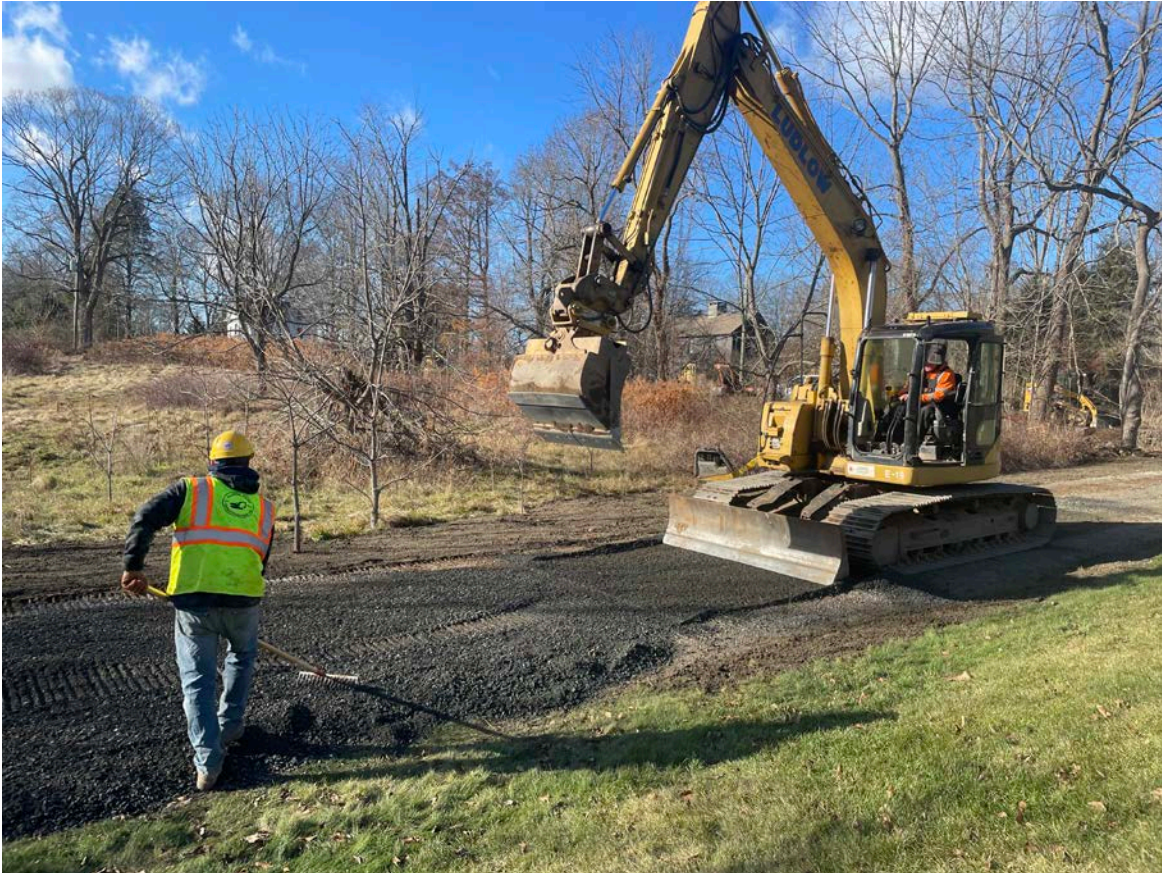
Picture 4: Ludlow placing and raking out \frac{3}{4} " gravel on the driveway of the 14 Talcott Lane property where they are working to restore those portions of the property that were disturbed during the installation of a 2" copper water service line. View to the northwest.
