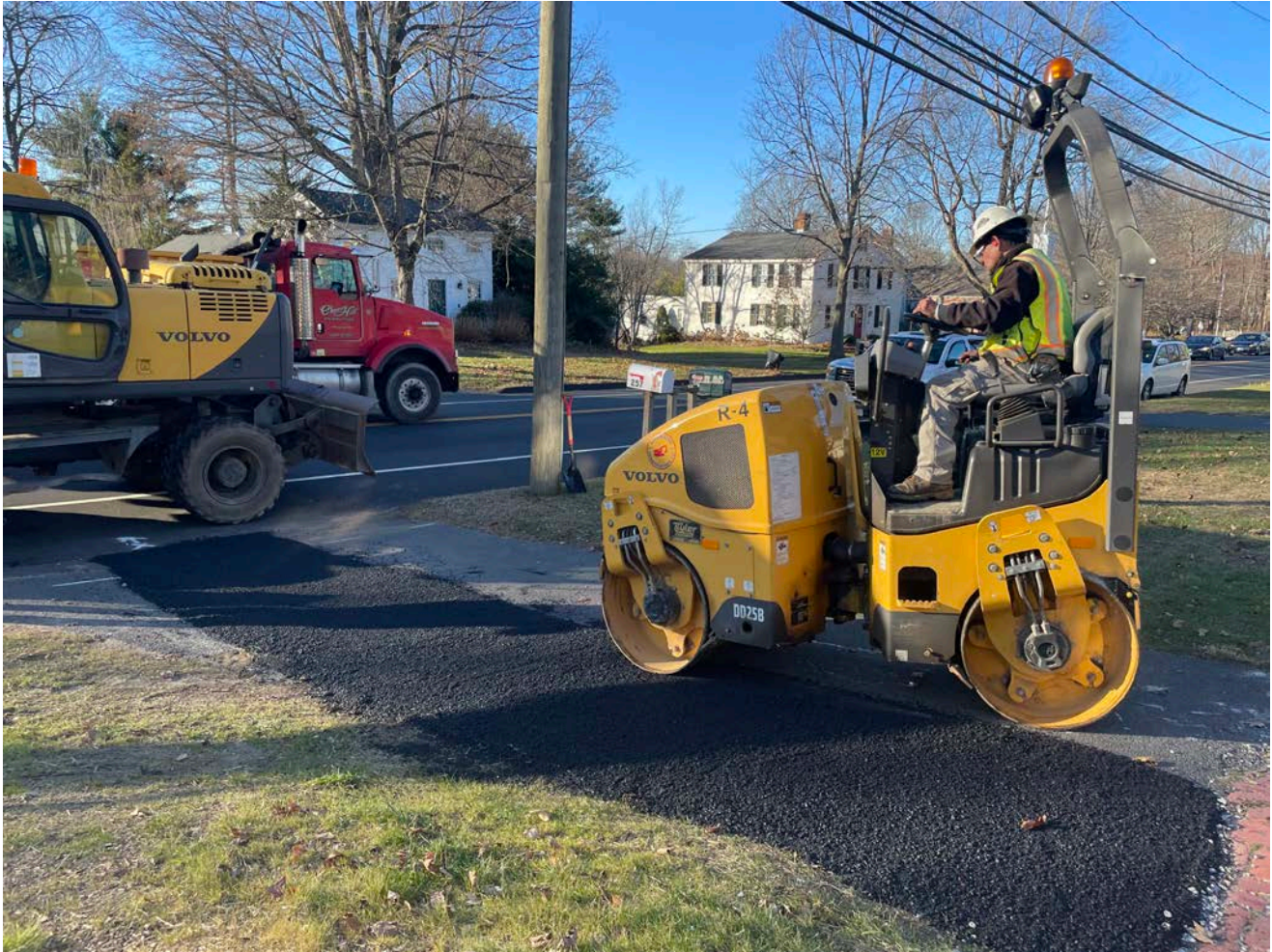
Picture 8: Ludlow compacting asphalt they placed over the curb stop trench patch on the driveway apron for the 257 Main Street, Durham, to address some settling that occurred there. View to the northwest.
