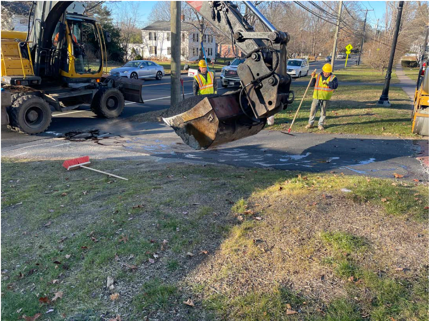
Picture 6: Ludlow placing asphalt over the curb stop trench patch on the driveway apron for the 257 Main Street, Durham, to address some settling that occurred there. View to the northwest.
