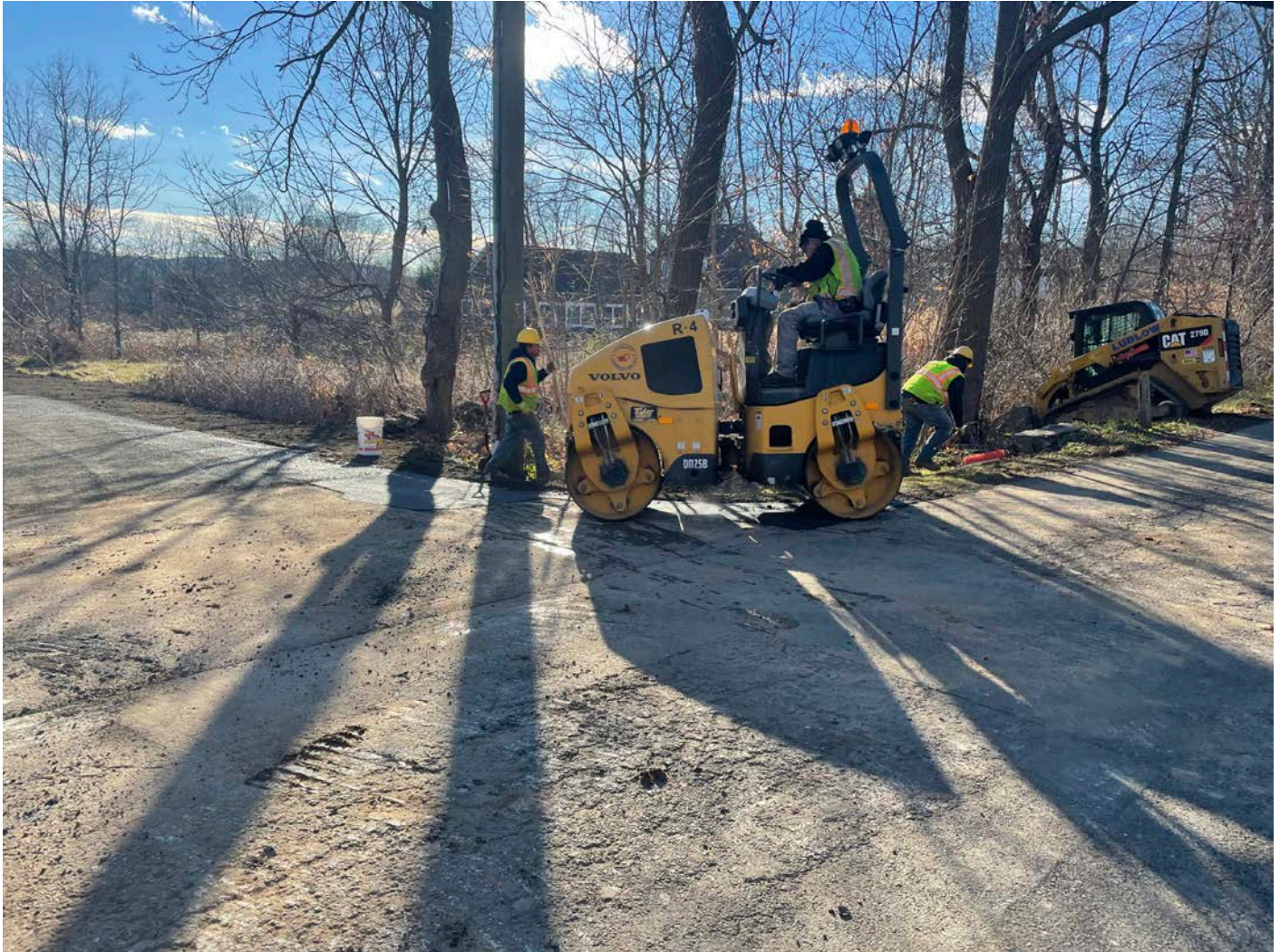
Picture 5: Ludlow compacting asphalt they just placed at the northwest corner of the driveway apron for the 14 Talcott Lane property. View to the southwest.
