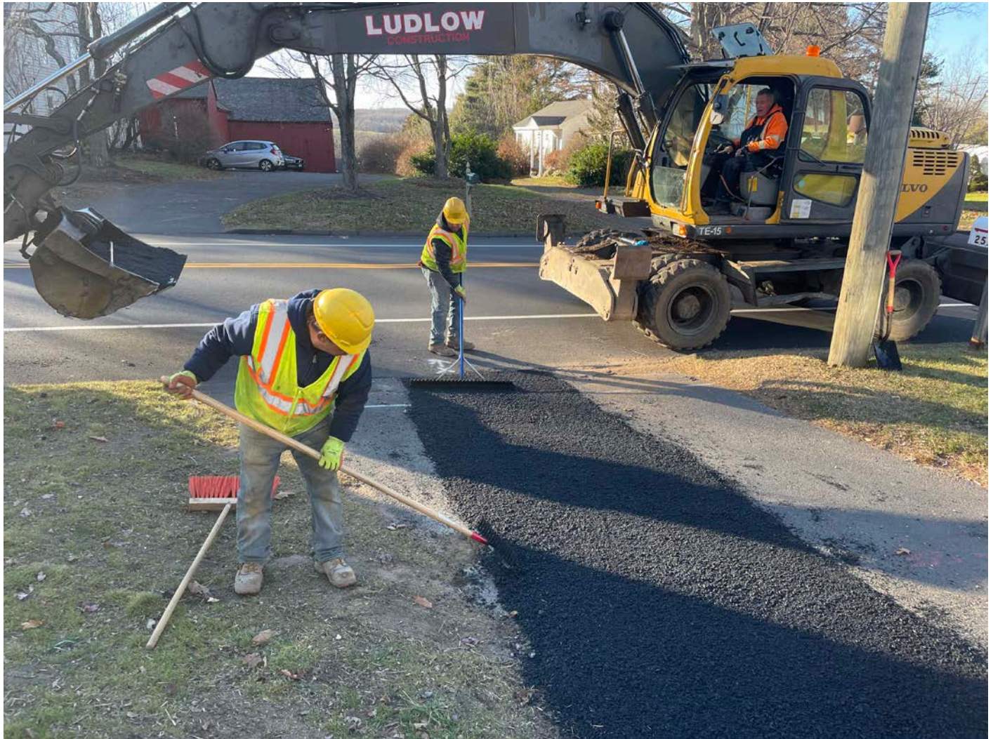
Picture 7: Ludlow raking asphalt that they just placed over the curb stop trench patch on the driveway apron for the 257 Main Street, Durham, to address some settling that occurred there. View to the west.
