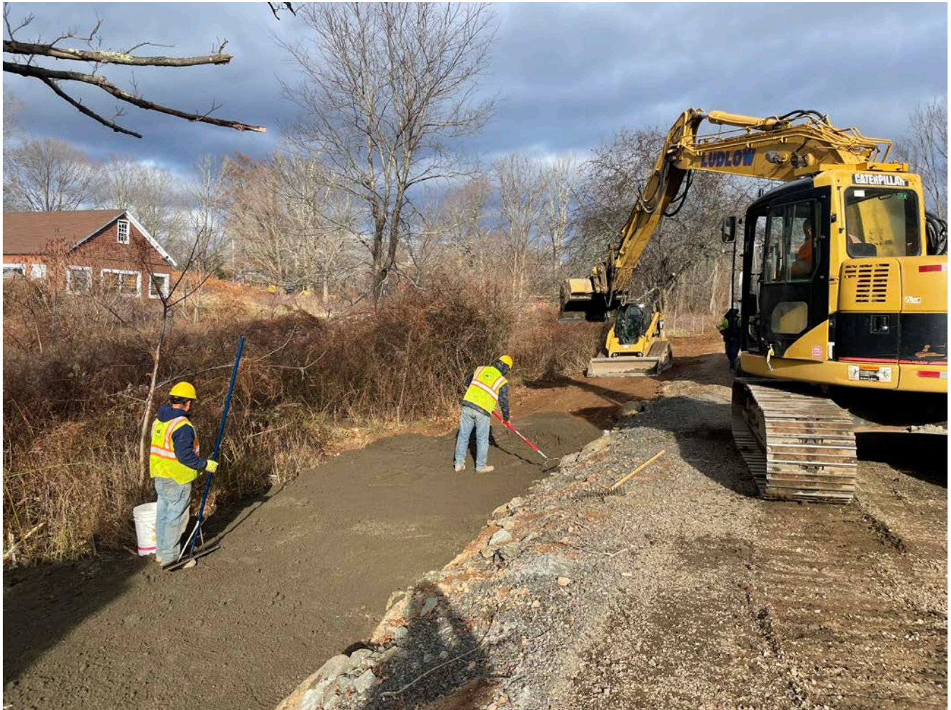
Picture 2: Ludlow placing, grading, and raking out loam on the west side of the driveway of the 14 Talcott Lane property as they finish the installation of a 2" copper water service line. View to the north.
