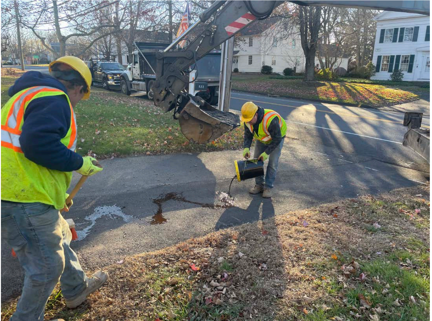
Picture 9: Ludlow placing tack coat over the curb stop trench patch on the driveway apron for the 253 Main Street, Durham, to address some settling that occurred there. View to the wouthwest.
