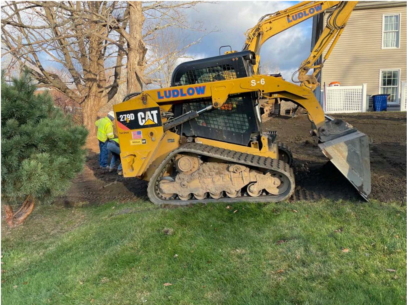
Picture 1: Ludlow grading loam to the southwest of the 14 Talcott Lane property as they finish up the installation of a 2" copper water service line. View to the north.
