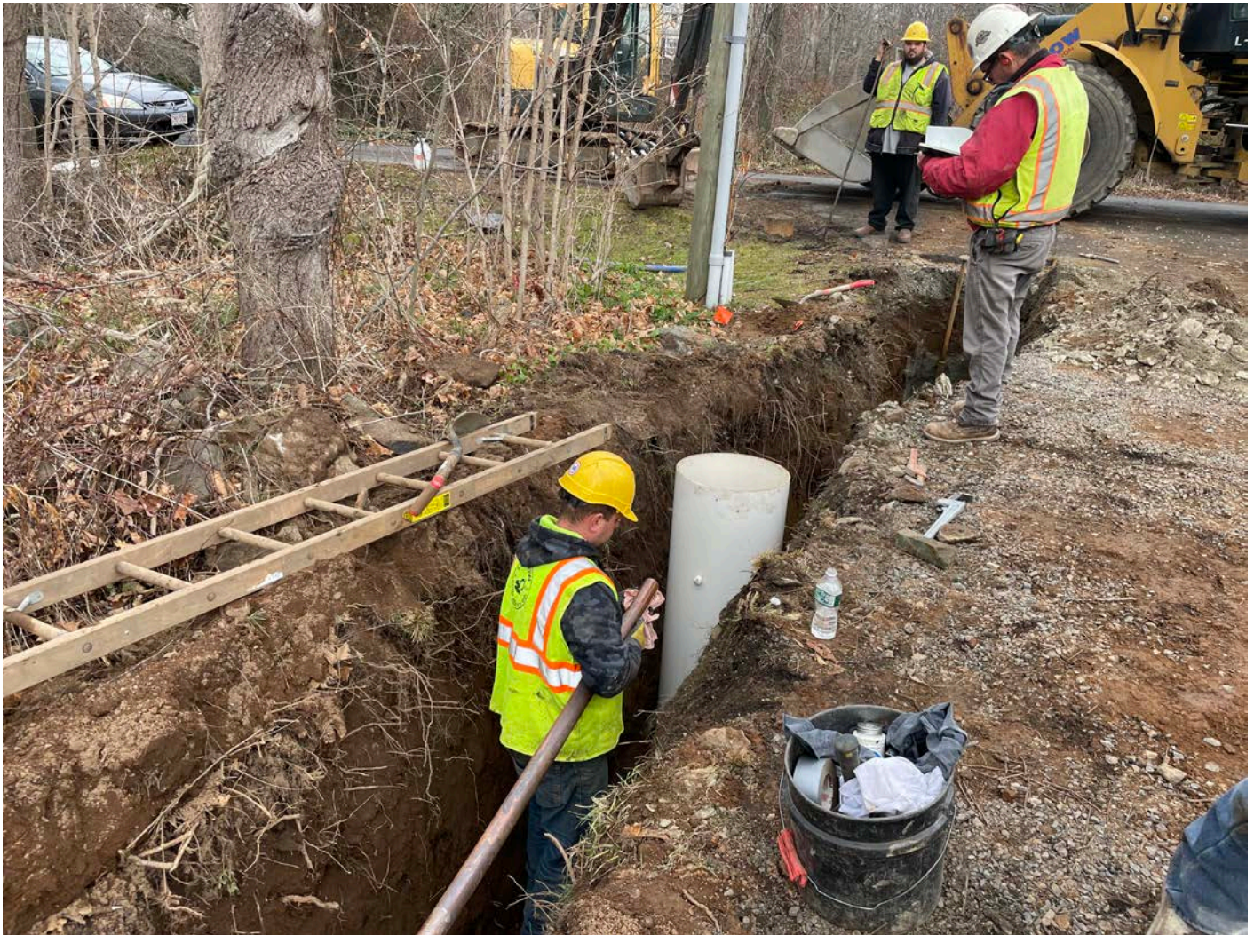
Picture 5: Ludlow preparing to connect 2" copper water line to a meter pit at the 14 Talcott Lane property. View to the south.
