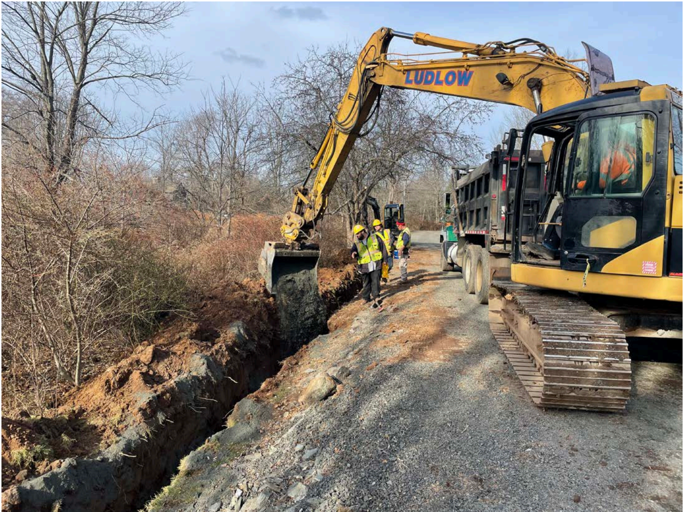
Picture 7: Ludlow placing sand over the 2" copper water service line they have installed on the west side of the driveway for the 14 Talcott Lane property. View to the north.
