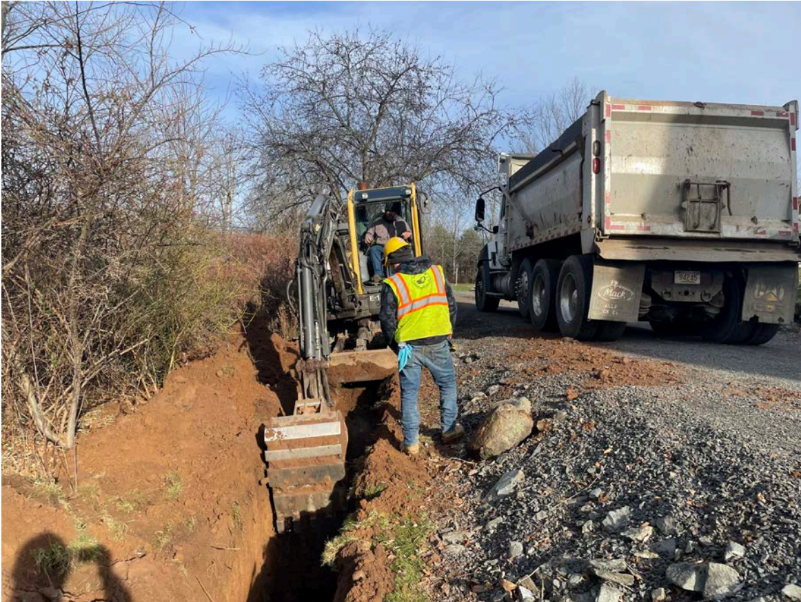
Picture 4: Ludlow excavating on the west side of the driveway for the 14 Talcott Lane property for the installation of a 2" copper water service line. View to the north.
