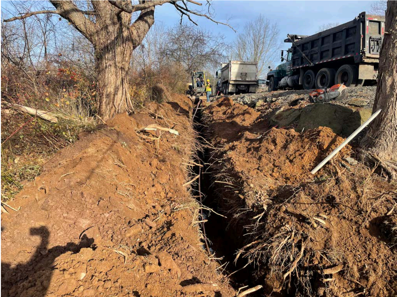
Picture 3: Trench that Ludlow has excavated on the west side of the 14 Talcott Lane property for the installation of a 2" copper water service line. View to the north.
