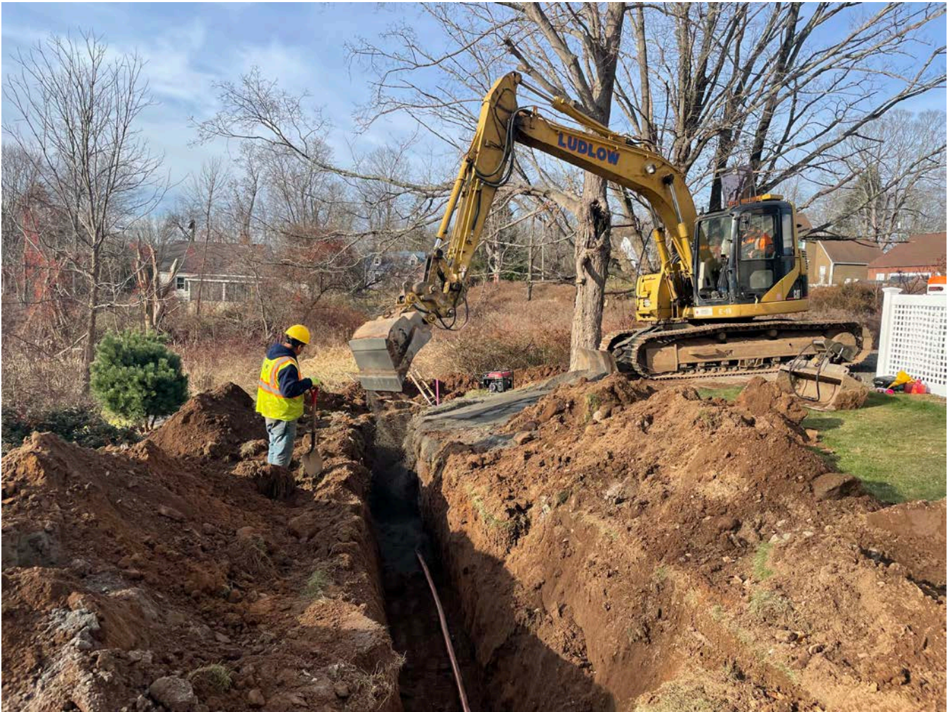
Picture 2: Ludlow placing sand above and below the 2" copper water service line on the west side of the driveway for the 14 Talcott Lane property. View to the south.
