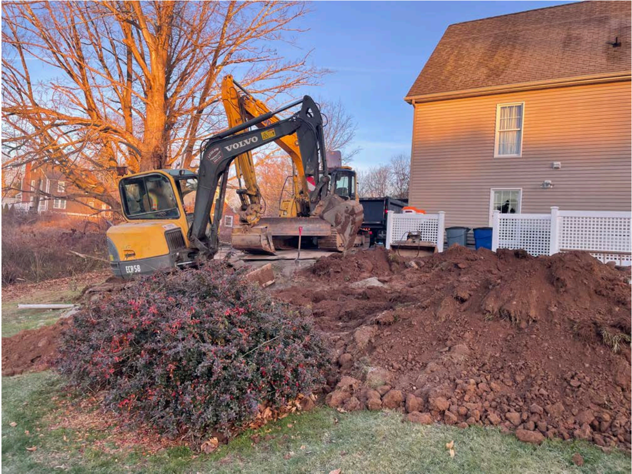
Picture 1: Ludlow excavating a trench on the south side of the 14 Talcott Lane residence for the installation of a 2" copper water service line. View to the northwest.
