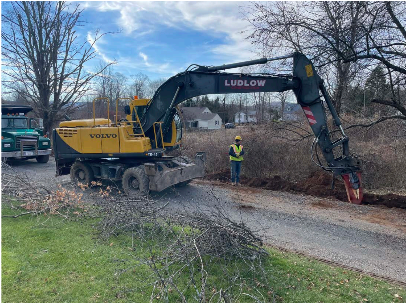
Picture 5: Ludlow hammering rock on the west side of the driveway at 14 Talcott Lane as they continue the installation of a 2" copper water service line. View to the southwest.
