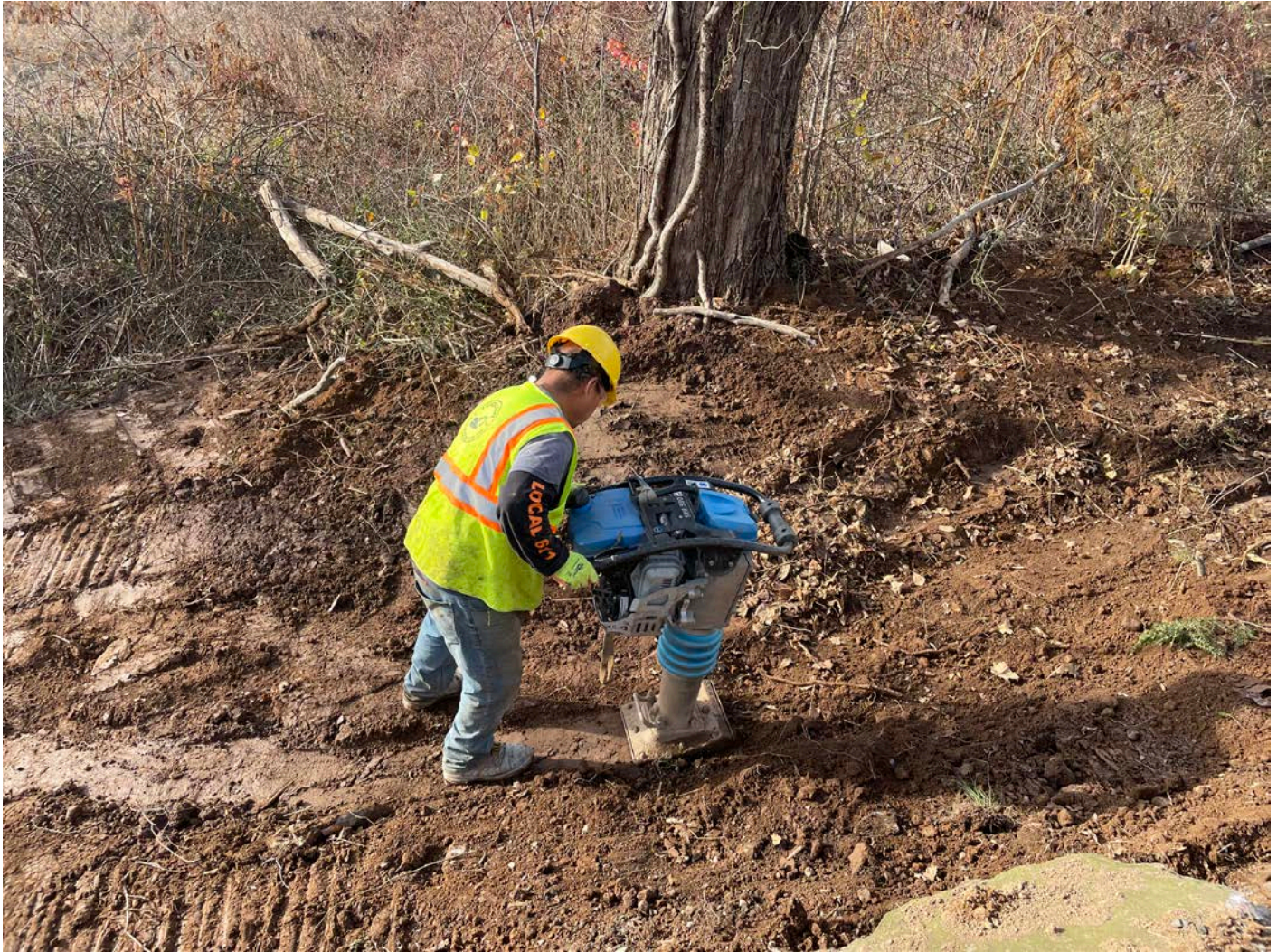
Picture 6: Ludlow using a jumping jack to compact native fill that they are backfilling the trench at the 14 Talcott Lane property with in 1' lifts View to the west.
