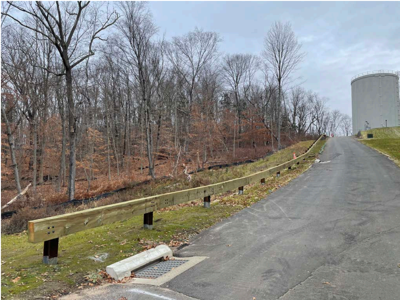
Picture 3: Guardrail that Eagle Fence and Guardrail installed between Stations 10+50 and 13+70 on the north side of the Shared Access Driveway in Middletown.
