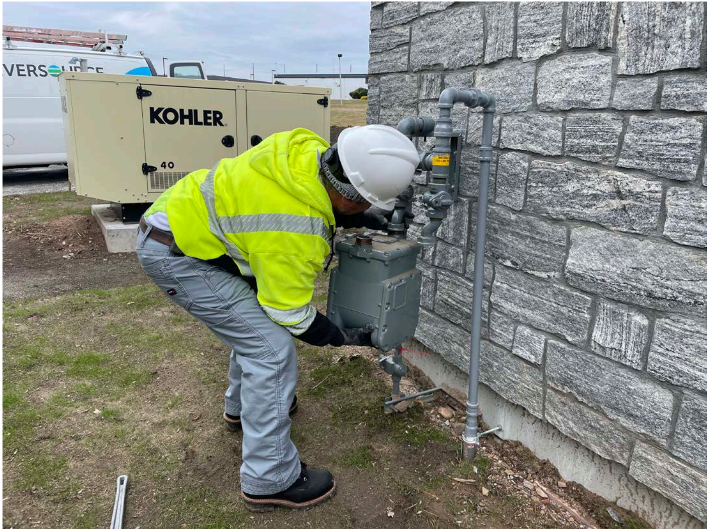
Picture 5: Eversource installing a gas meter on the south side of the booster station next to the southwest corner.
