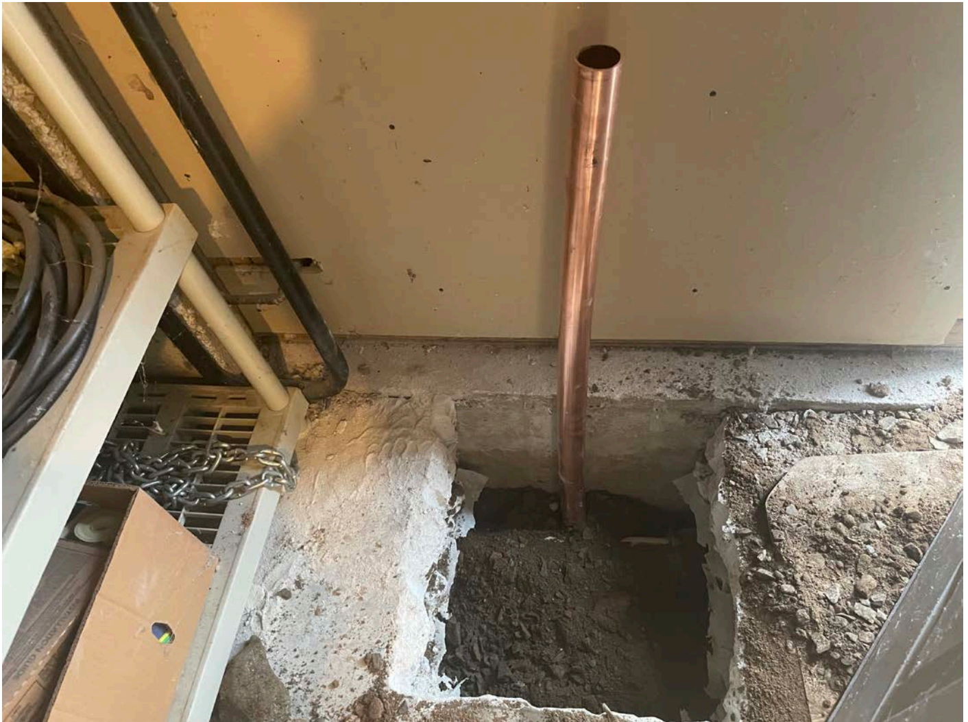
Picture 8: 2" copper water line that Ludlow has brought to the inside of the 14 Talcott Lane residence. View to the south.
