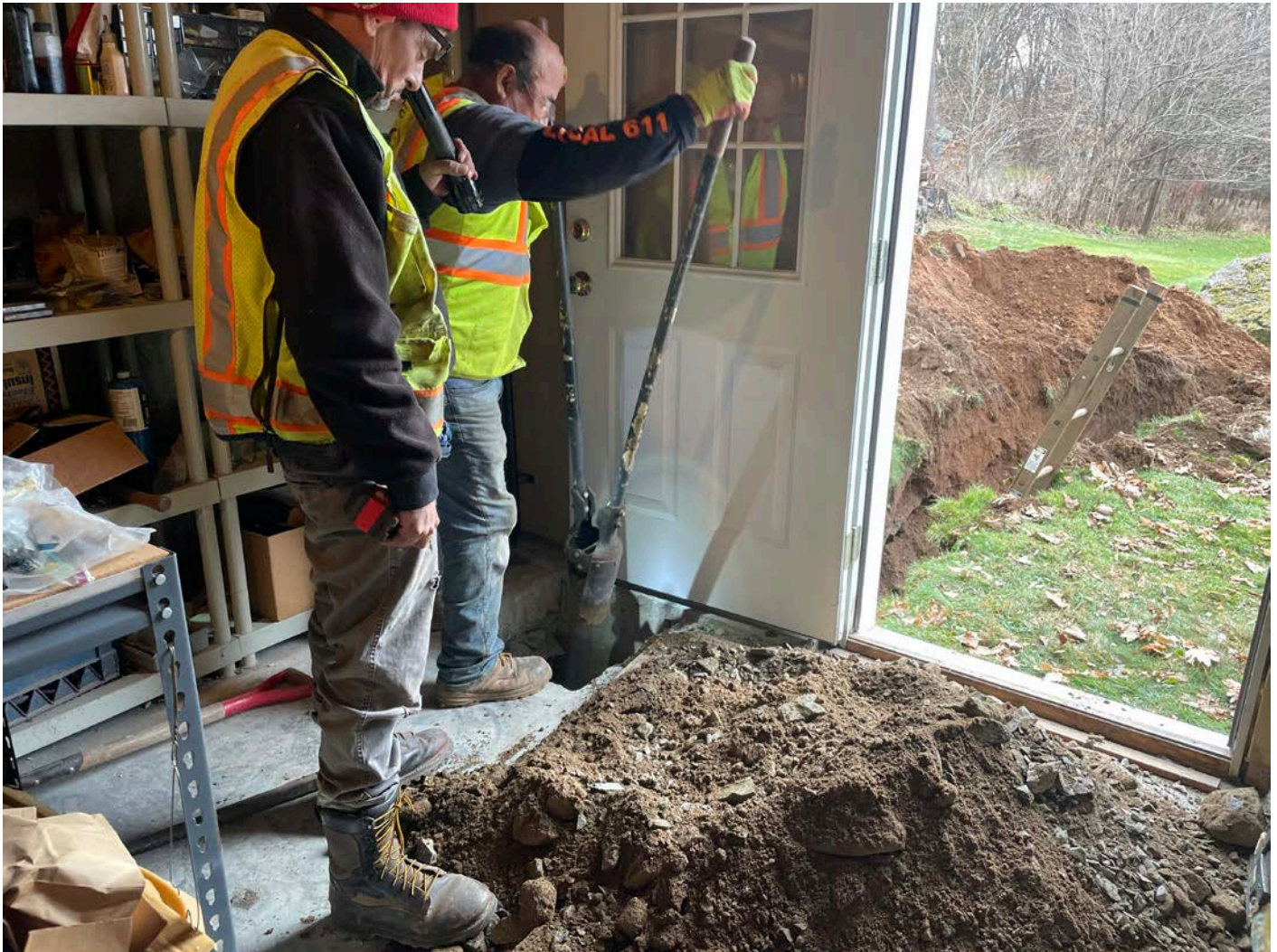
Picture 6: Ludlow using a post hole digger to remove soil down to where they cored a 2” hole through the southern foundation wall of the 14 Talcott Lane residence. View to the south.
