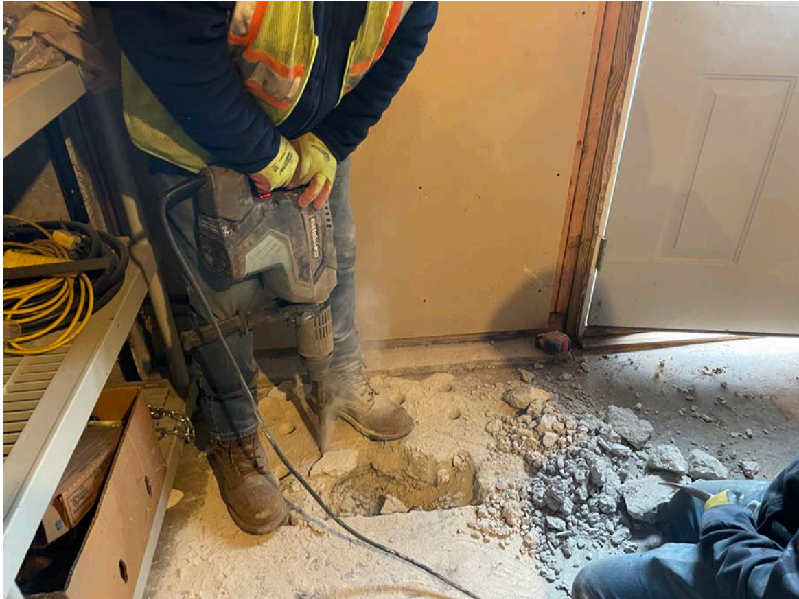
Picture 4: Ludlow penetrating the concrete floor of the 14 Talcott Lane residence to bring a 2" copper water service line inside the home. View to the south.
