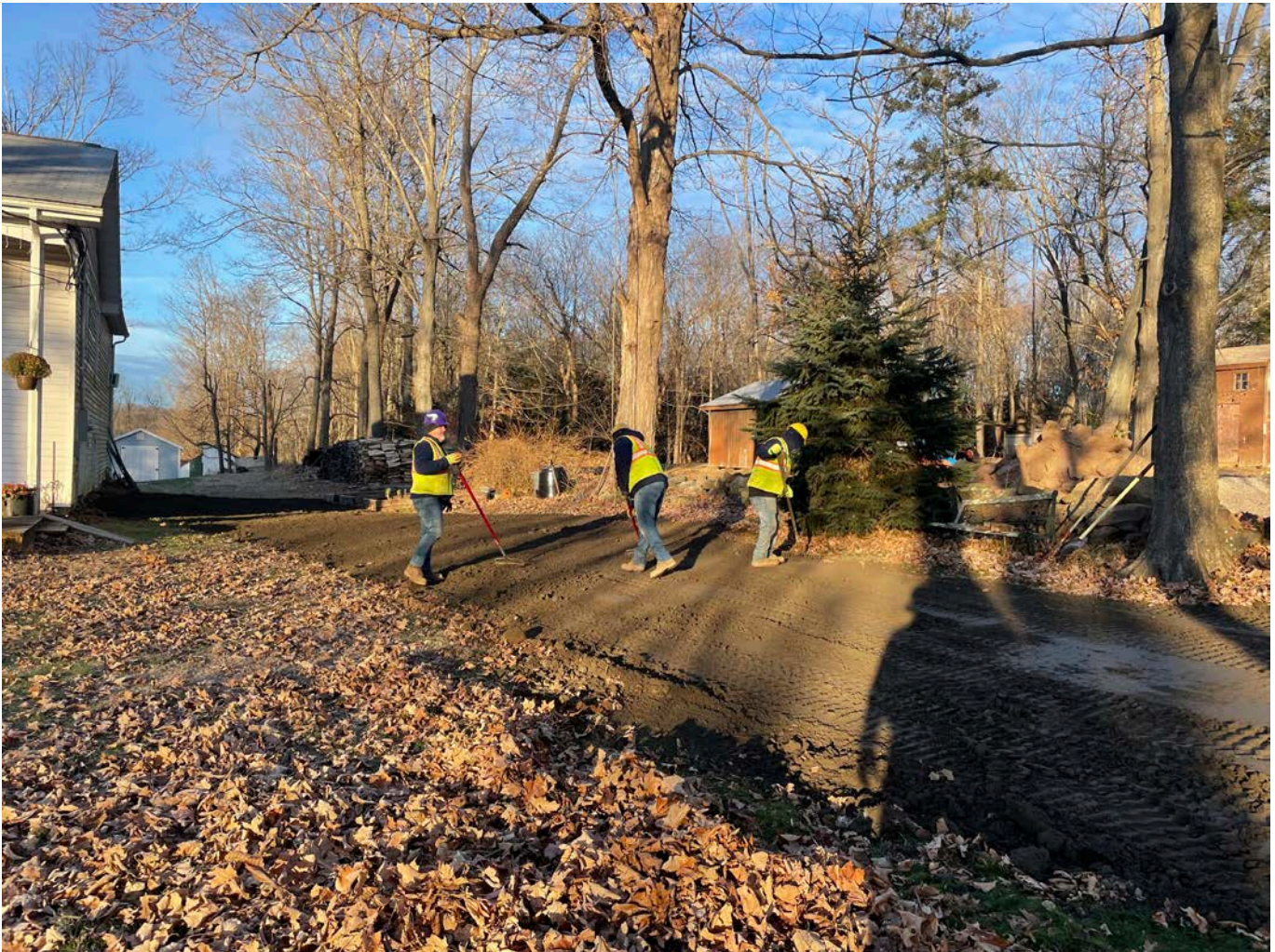
Picture 2: Ludlow raking out the loam they placed at the 230 Maple Avenue property to restore those areas that were disturbed during the installation of a 1" copper water service line. View to the northwest.
