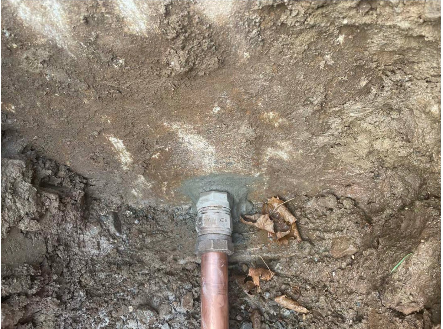
Picture 7: 2" copper water service line that Ludlow inserted through the southern foundation of the 14 Talcott Lane residence and secured in place with non-shrink grout. View to the north.
