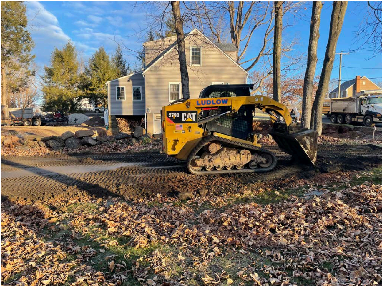
Picture 1: Ludlow grading loam that they placed at the 230 Maple Avenue property to restore those areas that were disturbed during the installation of a 1" copper water service line. View to the north.
