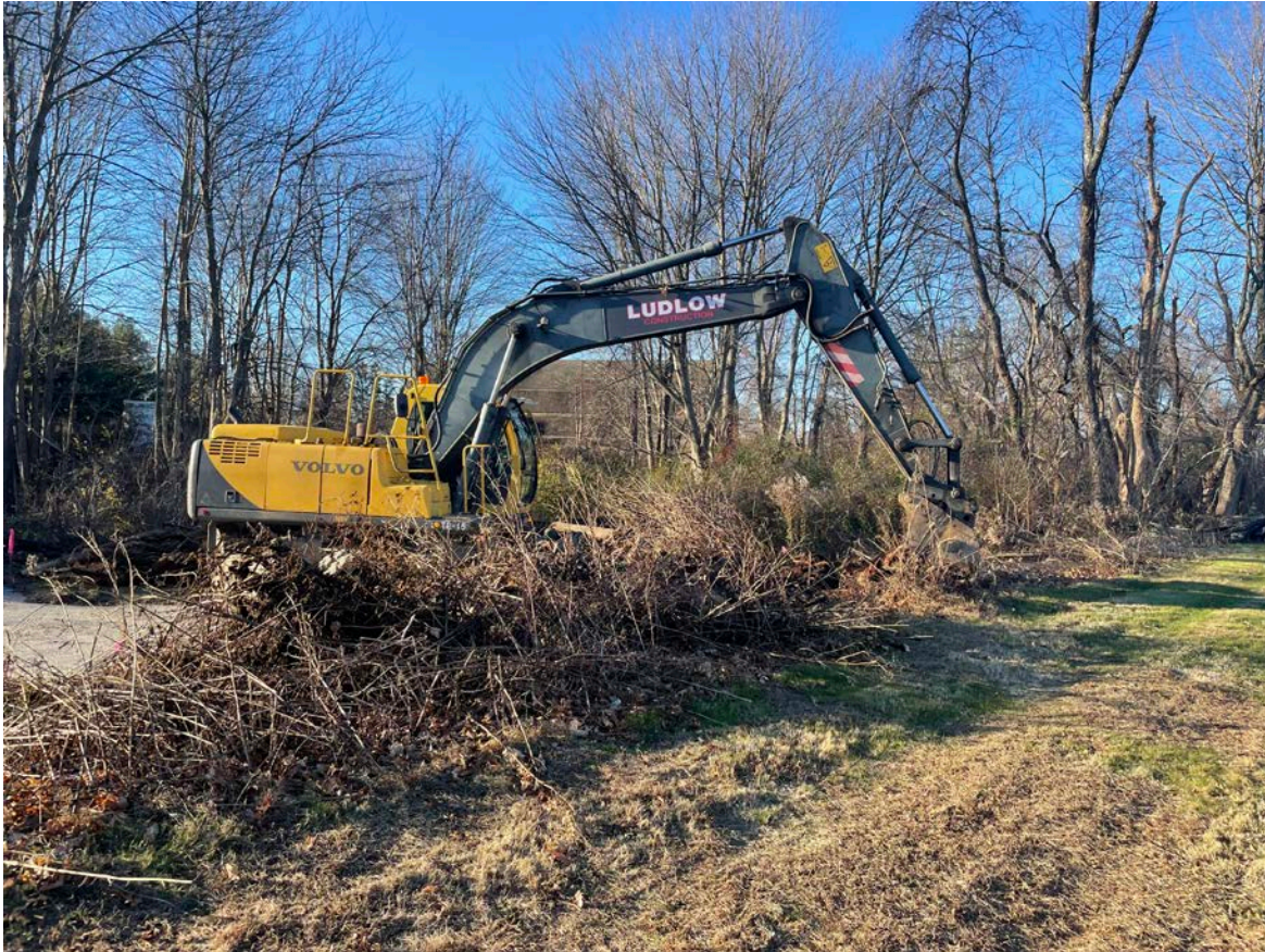
Picture 3: Ludlow excavating brush and tree stumps at the northwest corner of the booster station work zone located at Station 750+63 in Middletown. View to the west.
