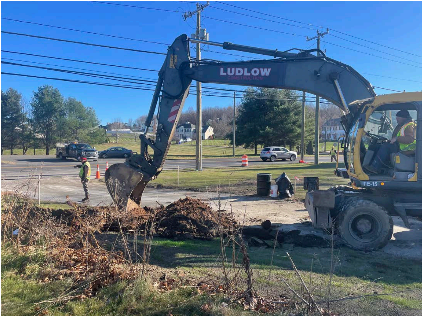
Picture 8: Ludlow excavating a tree stump from the north side of the booster station work zone located at Station 750+63 in Middletown. View to the southeast.
