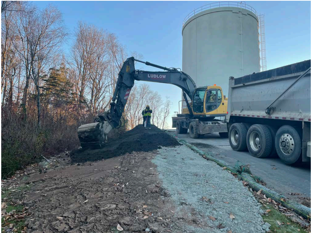
Picture 1: Ludlow placing loam on top of the 1.25"-minus gravel they placed and compacted yesterday on the north side of the water tank located east of the Shared Access Driveway in Middletown. View to the east.
