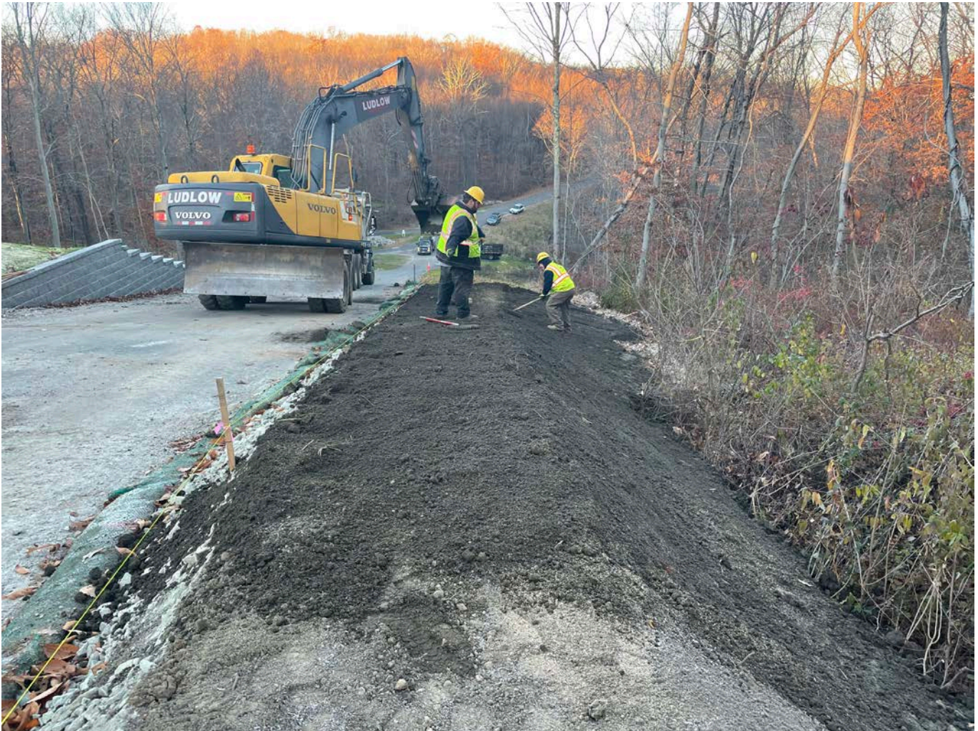
Picture 2: Ludlow placing grass seed on top of the loam they placed between Stations 10+50 and 11+75 on the north side of the Shared Access Driveway in Middletown. View to the west.
