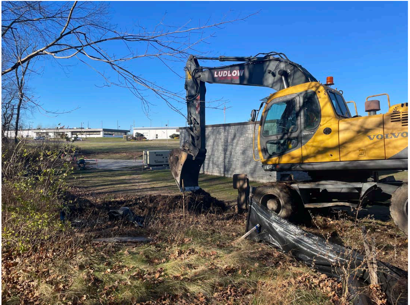
Picture 9: Ludlow excavating brush at the southeast corner of the booster station work zone located at Station 750+63 in Middletown. View to the northwest.
