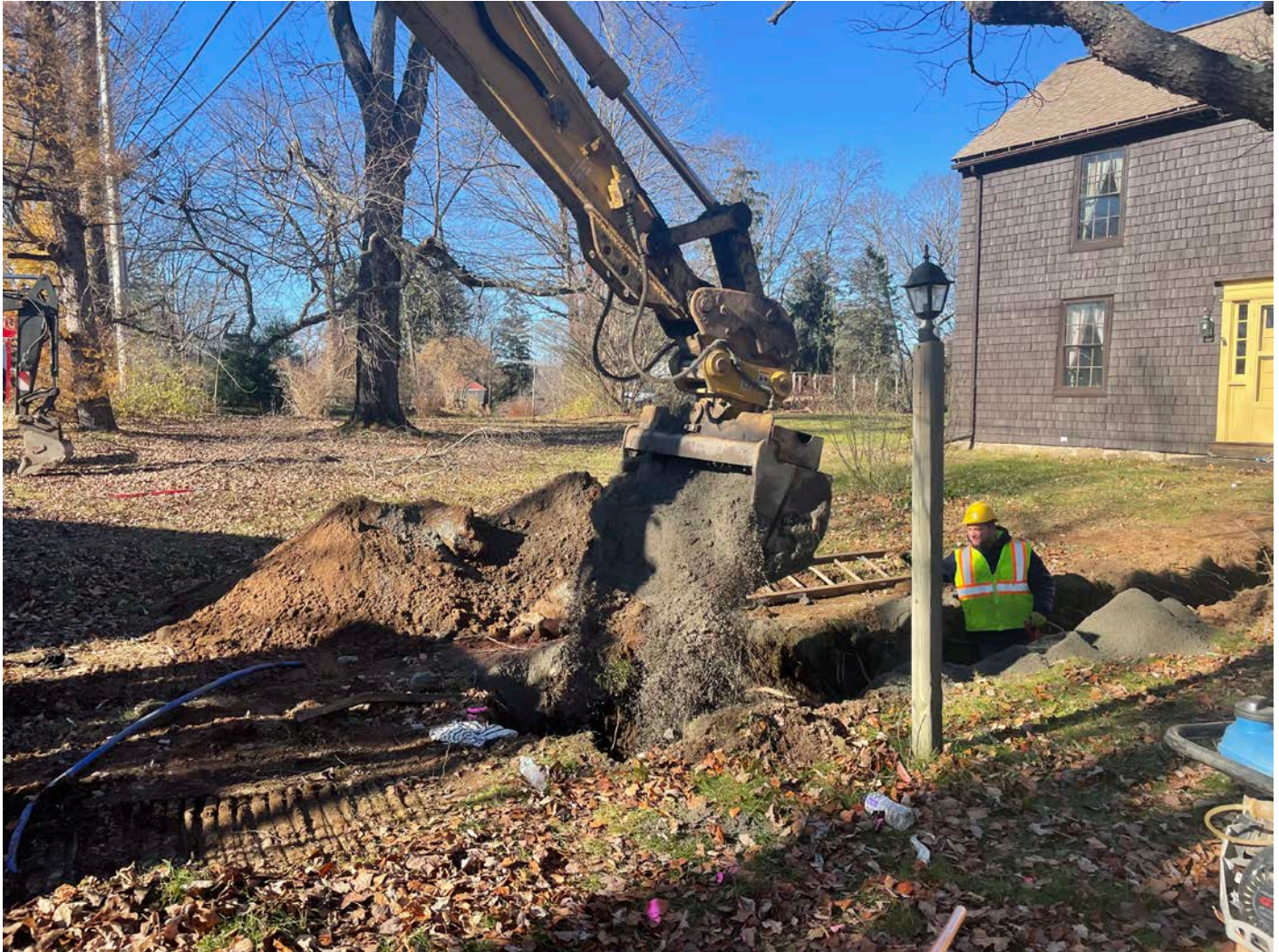
Picture 6: Ludlow placing sand over the 1” copper water service line they just installed at the 25 Talcott Lane property. View to the northwest.
