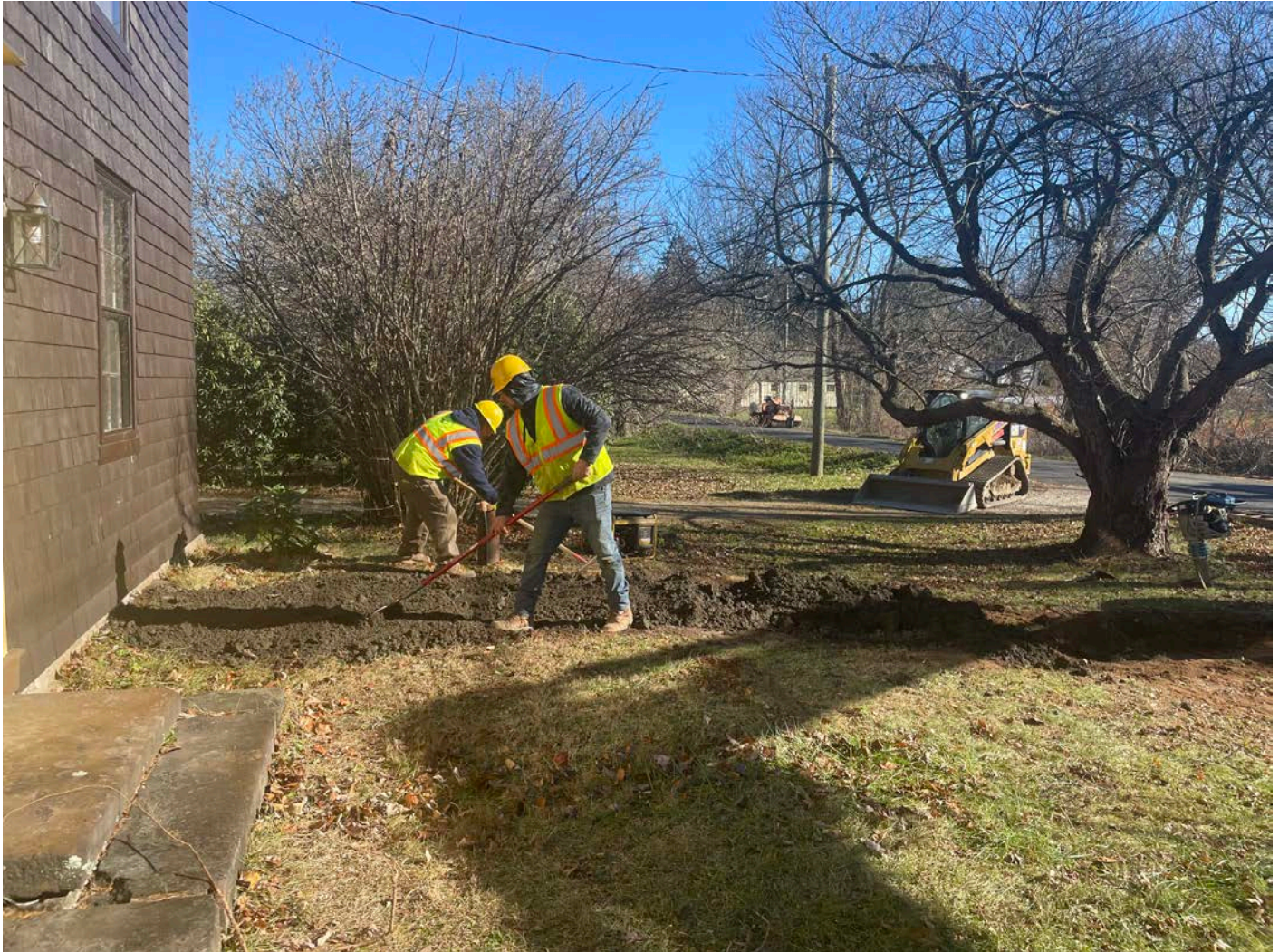
Picture 7: Ludlow raking out loam that was placed to restore those areas of the 25 Talcott Lane property that were disturbed during the installation of a 1" copper water service line. View to the east.
