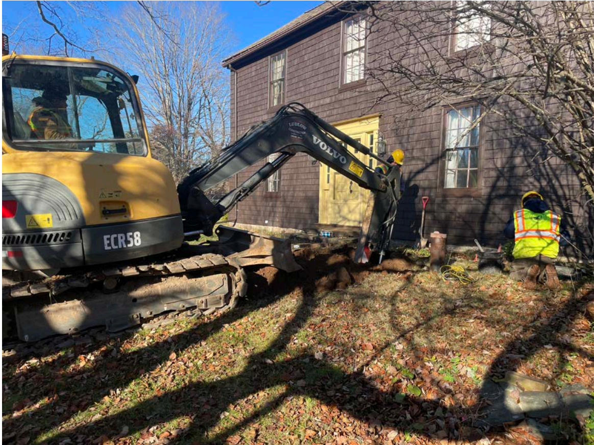
Picture 4: Ludlow excavating a trench on the south side of the 25 Talcott Lane residence for the installation of a 1" copper water service line. View to the northwest.
