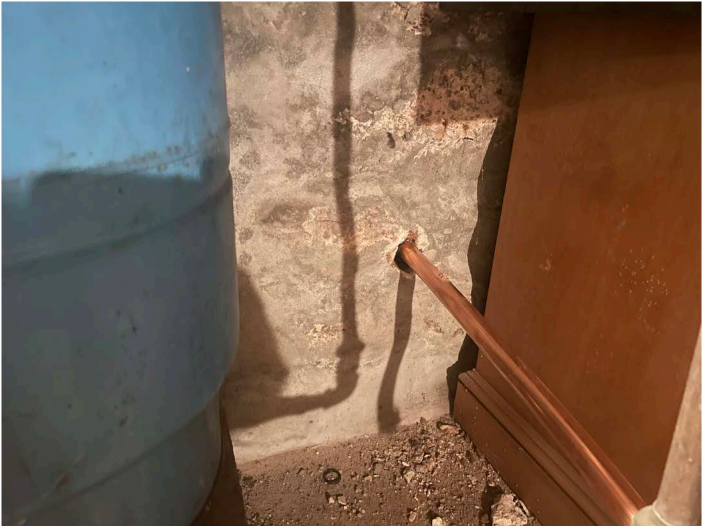
Picture 5: 1" copper water service line that Ludlow installed through the southern foundation of the 25 Talcott Lane residence. View to the south.
