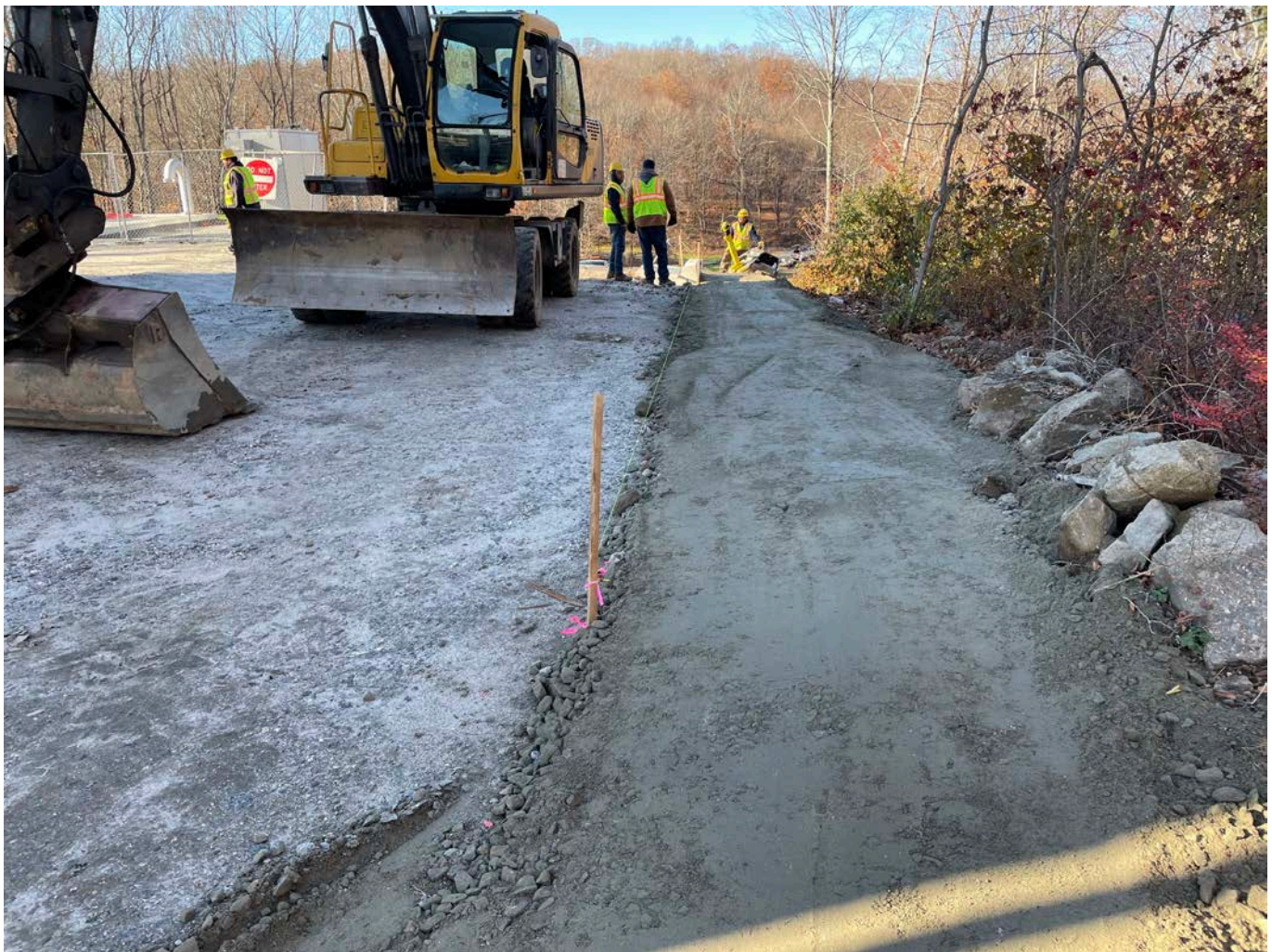
Picture 2: 1.25"-minus gravel that Ludlow has placed and compacted on the north side of the water tank located east of the Shared Access Driveway in Middletown. View to the west.
