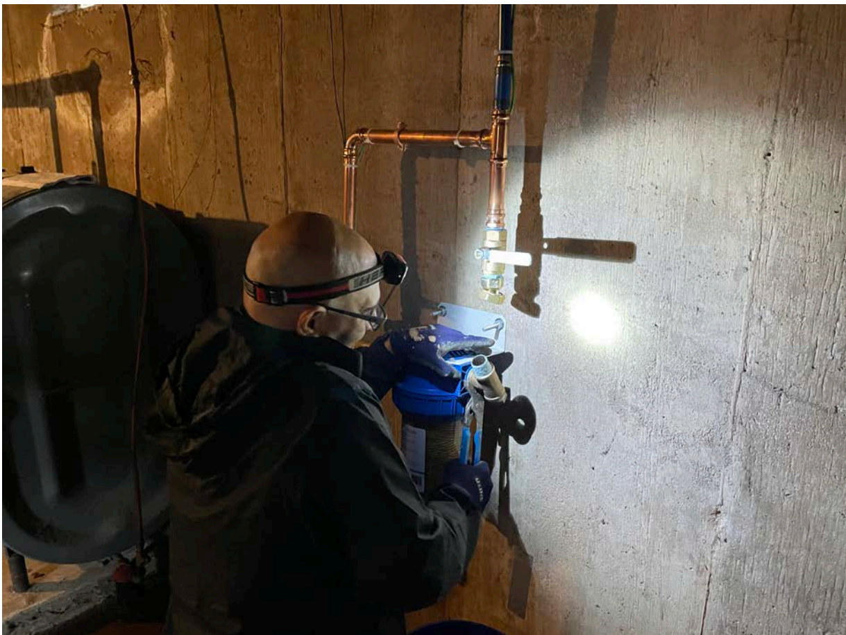
Picture 5: Fazzino Plumbing replacing a brass TEE at the 17 Wallingford Road, residence.
