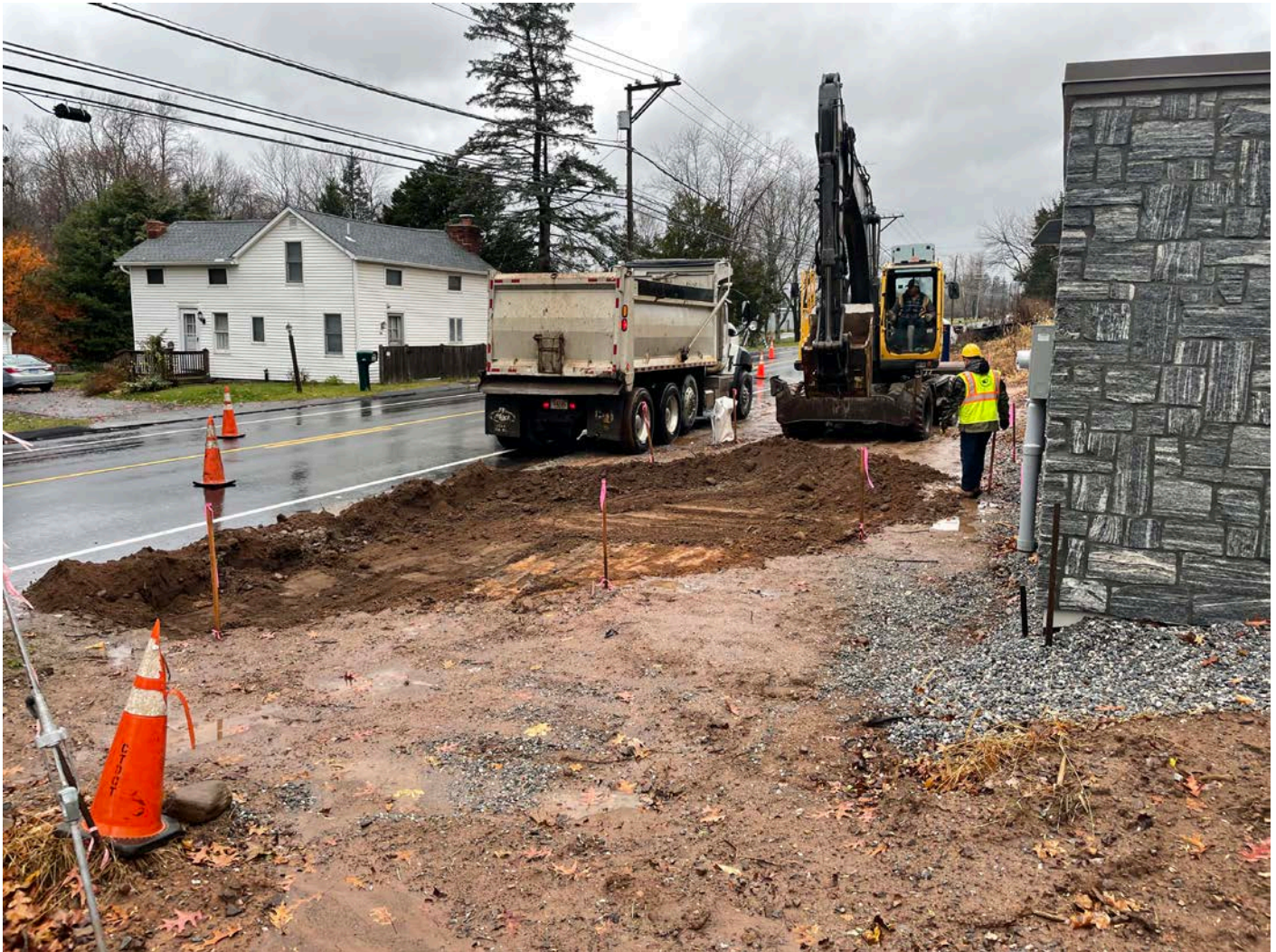
Picture 7: Ludlow removing 12" of fill within the footprint of the driveway for the water meter building located at Station 124+60. View to the northwest.
