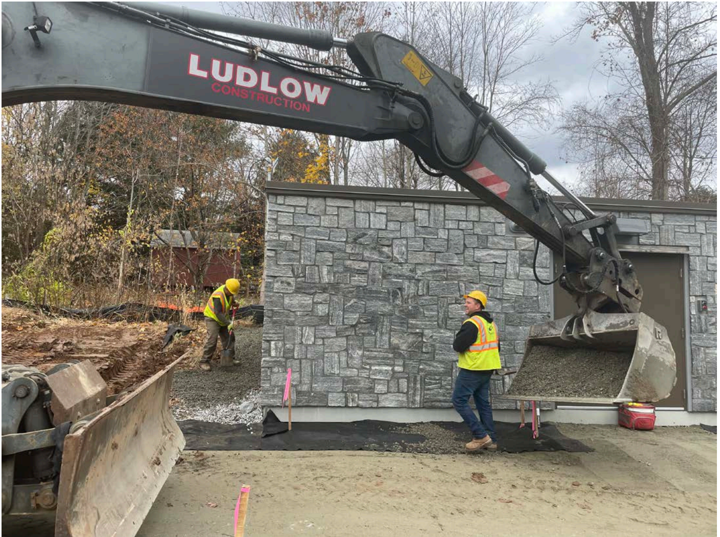
Picture 11: Ludlow placing ¾" gravel over filter fabric on the west side of the water meter building. View to the east.
