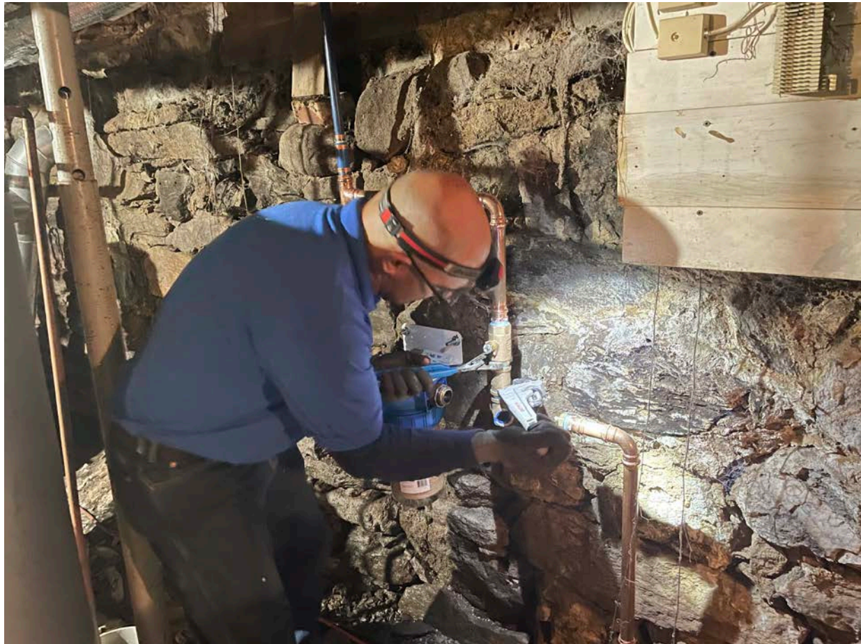
Picture 6: Fazzino Plumbing replacing a brass tee at the 208 Main Street, Durham, residence.
