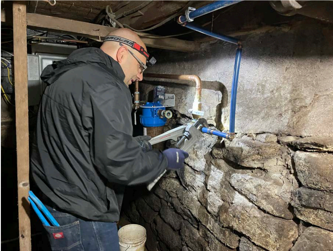
Picture 3: Fazzino Plumbing replacing a brass tee at the 168 Main Street, Durham, residence.
