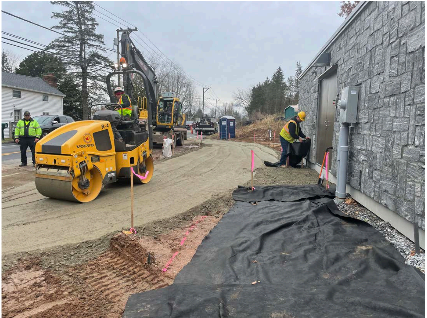
Picture 10: Ludlow using a rolling compactor on 1.25"-minus gravel that they placed on the footprint of the driveway at the water meter building located at Station 124+60. View to the north.
