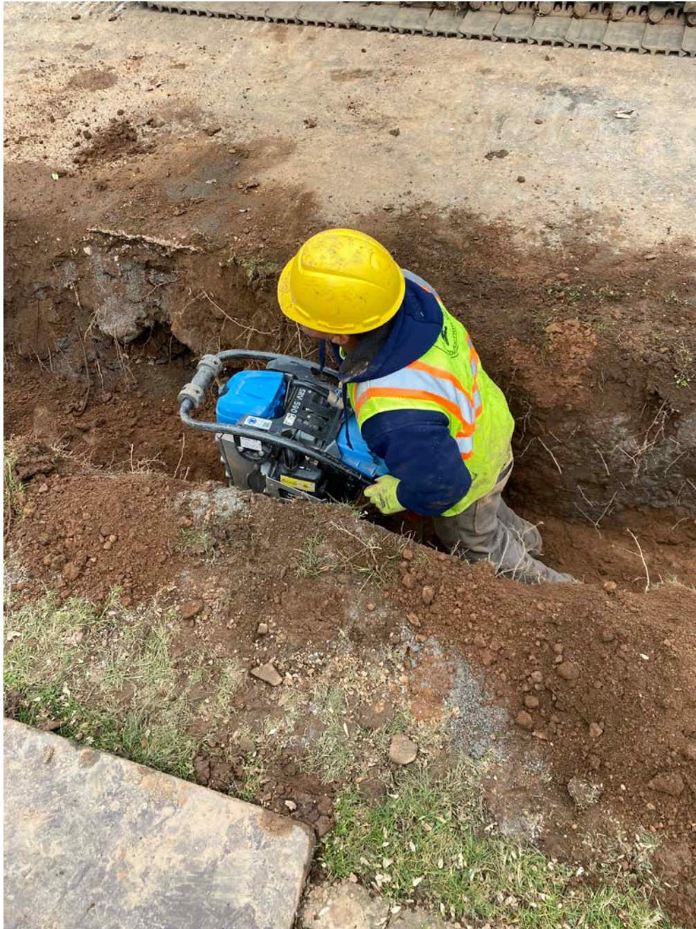
Picture 8: Ludlow compacts the backfill in the trench of the 1" copper water service line to 254 Maple Ave residence with a jumping jack compactor.
