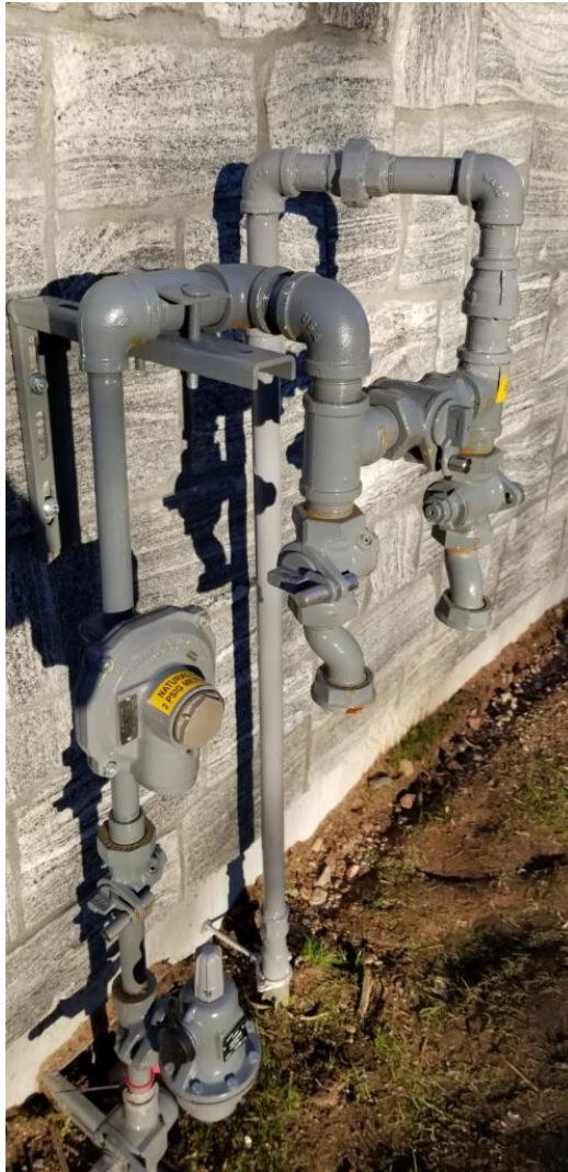
Picture 11: Fazino Plumbing returned to the Booster station and replaced all fittings with new fittings from Ward MFG.
