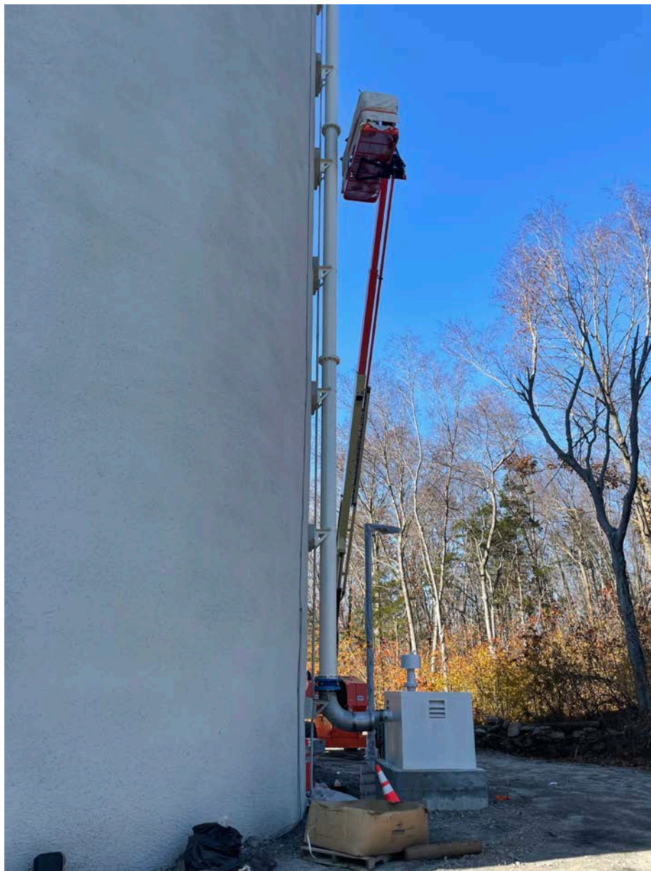
Picture 5: Keltic Painting in the process of painting the 12" air duct located on the northeast side of the water tank located east of the Shared Access Driveway in Middletown. View to the northwest.
