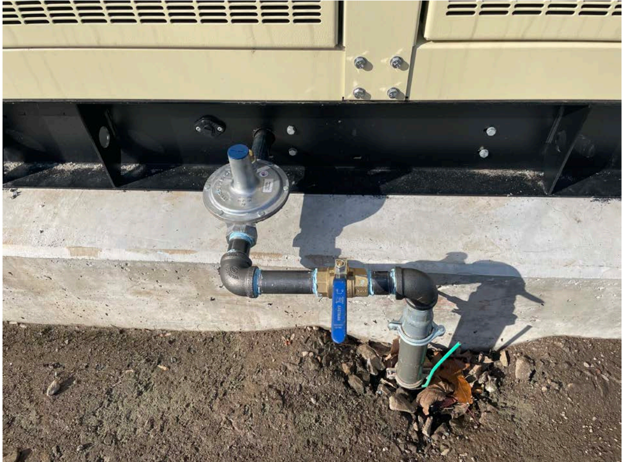
Picture 4: Natural gas line and regulator that Fazzino Plumbing installed on the east side of the generator at the booster station. View to the west.
