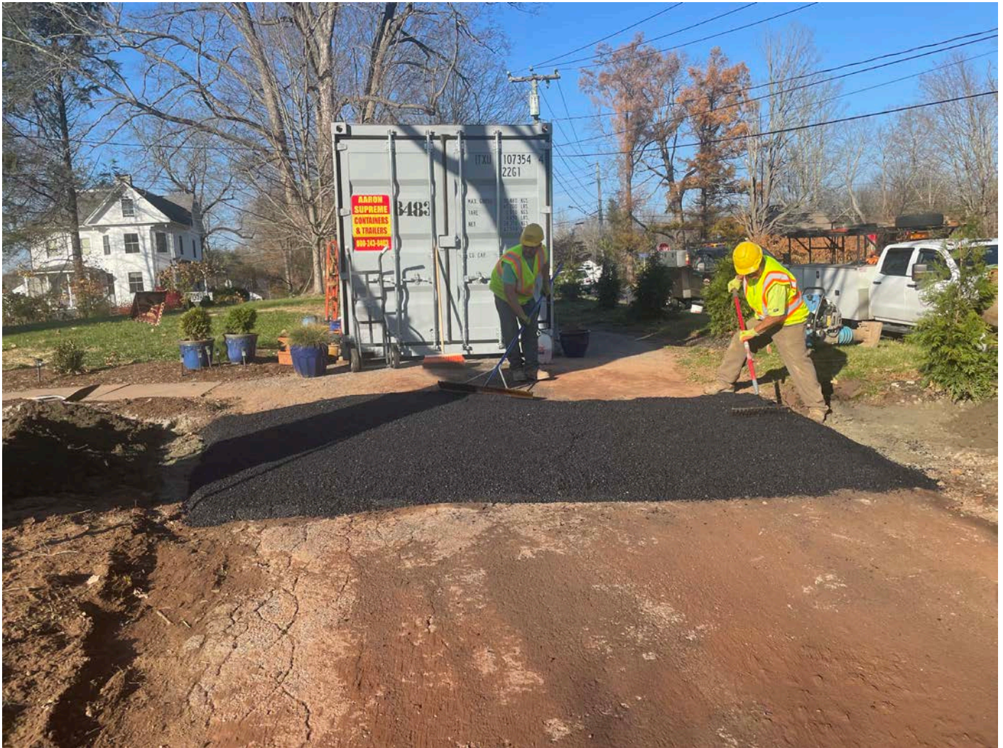
Picture 7: Ludlow placing asphalt over the trench footprint at the 244 Maple Avenue property. View to the north.
