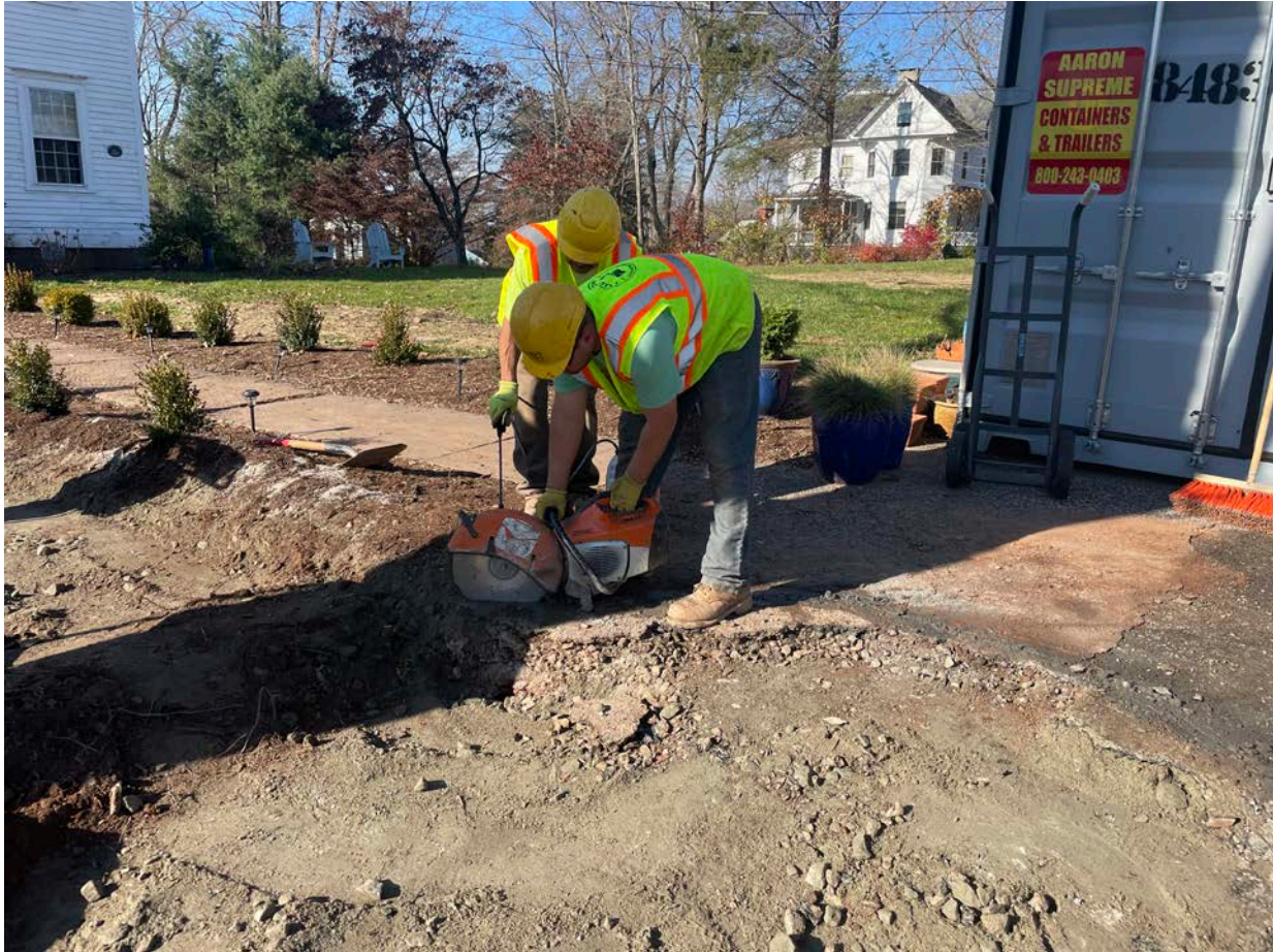
Picture 6: Ludlow saw cutting the edge of the asphalt driveway that they excavated a trench across in the process of installing a 1" copper water service line at the 244 Maple Avenue property. View to the northwest.
