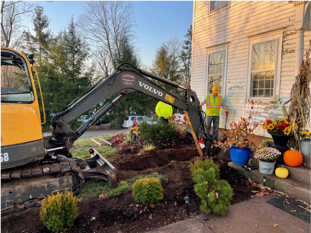
Picture 1: Ludlow excavating on the east side of the 244 Maple Avenue property for the installation of a 1" copper water service line. View to the southwest.
