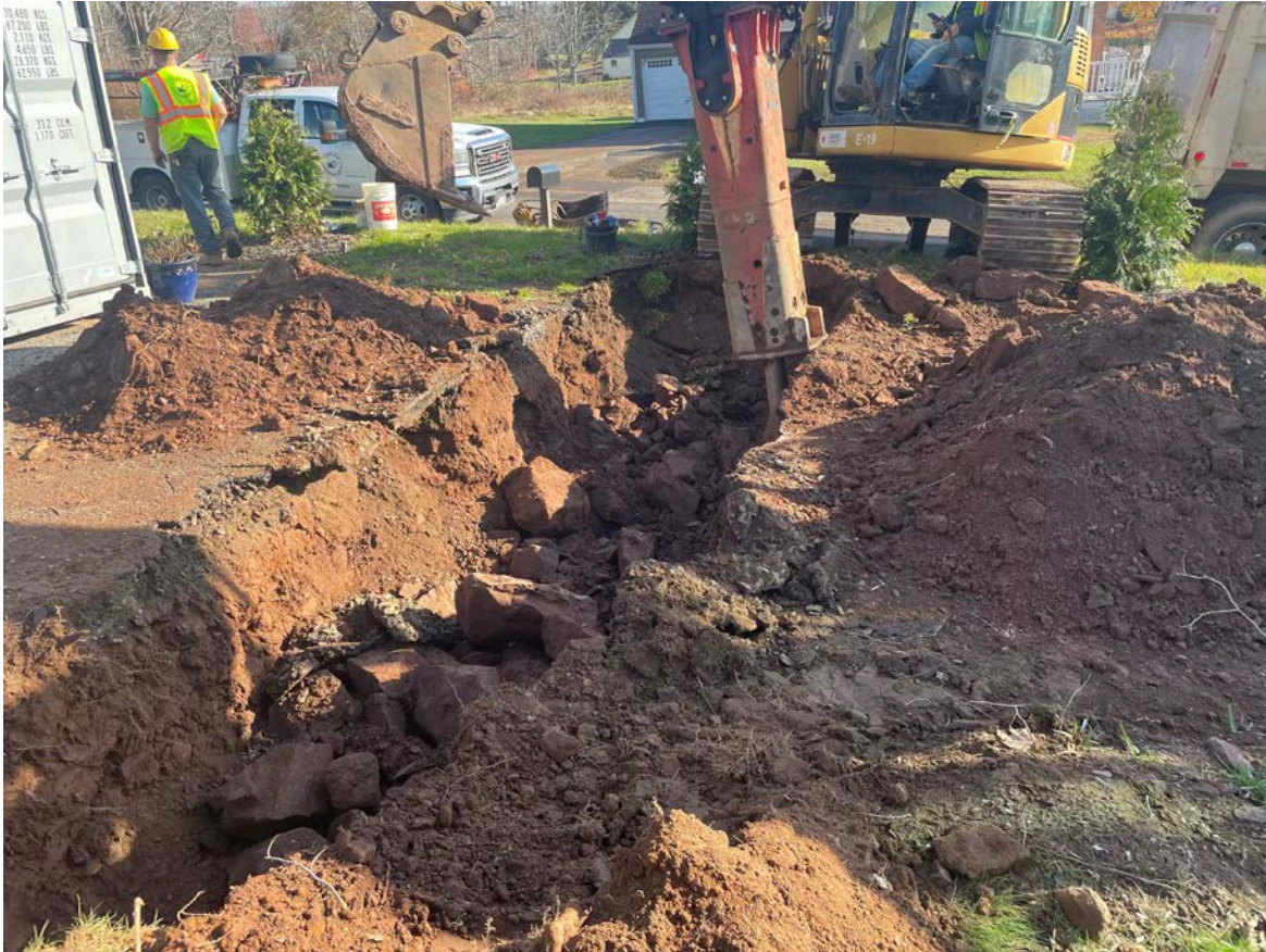
Picture 3: Ludlow hammering rock in the trench they are excavating at the 244 Maple Avenue property. View to the east.
