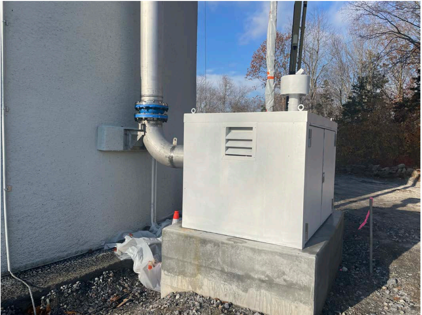
Picture 2: Blower enclosure that Keltic Painting has applied the first of two coats of paint. Water tank work zone located east of the Shared Access Driveway, Middletown. View to the northwest.
