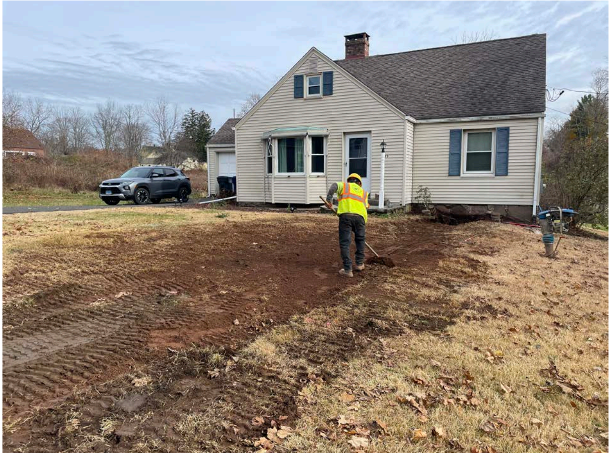
Picture 4: Ludlow raking out loam that they placed at the 235 Maple Avenue property to restore those areas of the lawn that were disturbed during the installation of a 1" copper water service line. View to the east.
