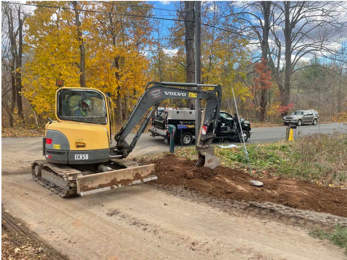
Picture 5: Ludlow placing loam next to the meter pit for the 228R Maple Avenue property. View to the southeast.
