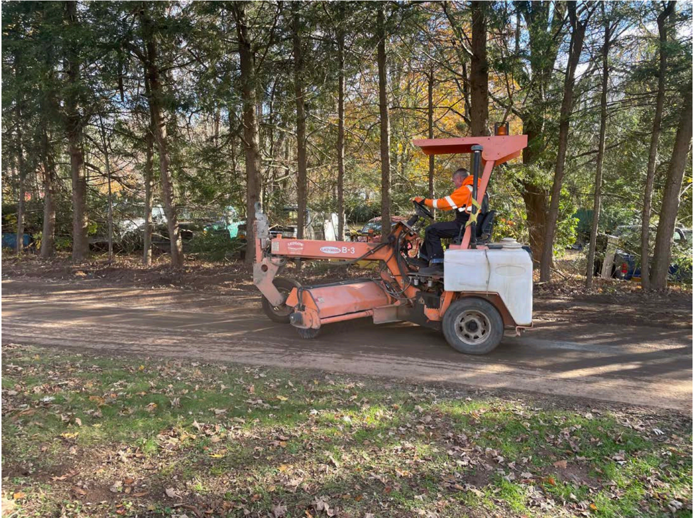
Picture 10: Ludlow cleaning the driveway at the 228R Maple Avenue property with a Broce Broom. View to the south.
