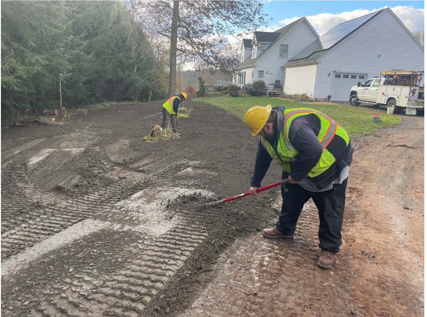
Picture 8: Ludlow raking out freshly placed loam to the west of the driveway for the 228R Maple Avenue property. View to the west.
