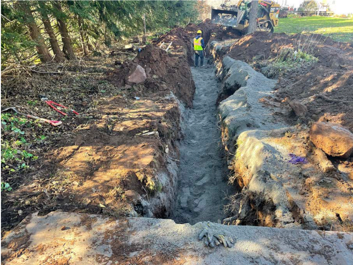
Picture 3: Ludlow placing sand over 1.5" copper water pipe that they installed at the 228R Maple Avenue property. View to the west.
