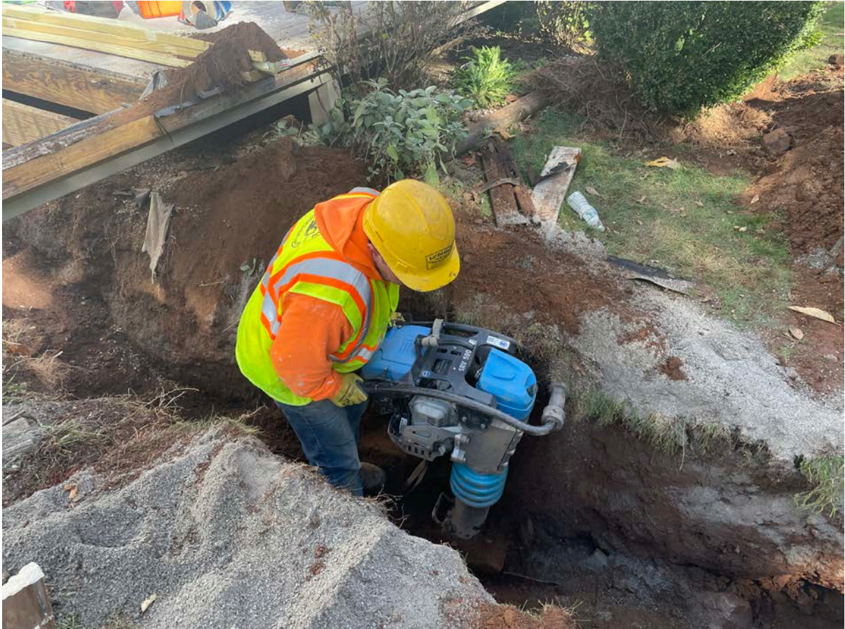
Picture 4: Ludlow compacting native fill that they placed over the 1.5" copper water service line they installed on the south side of the 228R Maple Avenue residence. View to the northeast.
