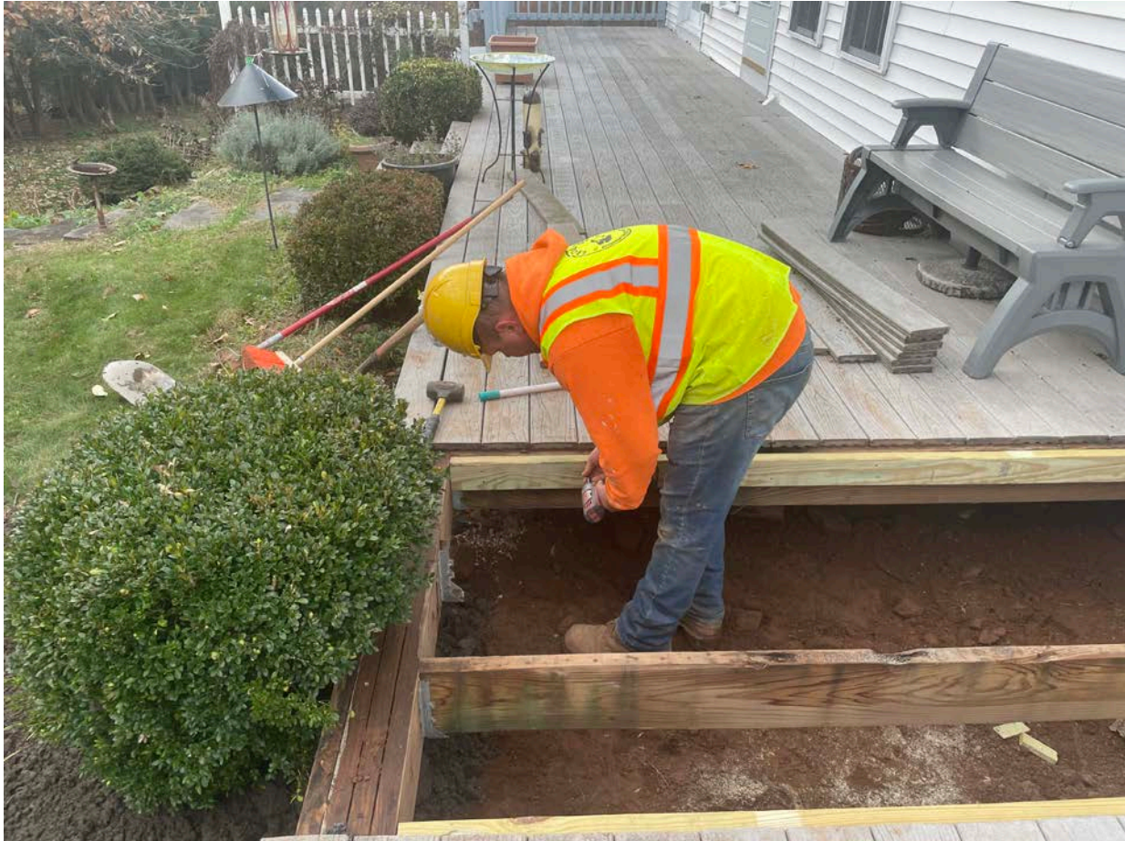
Picture 6: Ludlow attaching a 2x4 to one of the joists of the deck located on the south side of the 228R Maple Avenue residence to provide additional support when the deck slats are replaced. View to the west.
