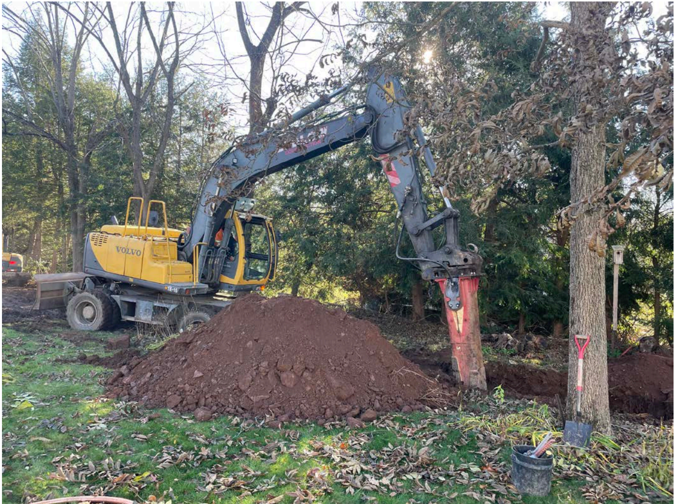
Picture 2: Ludlow hammering rock in the trench they are excavating for the installation of a 1.5" copper water service line at the 228 Maple Avenue property in Durham. View to the southeast.
