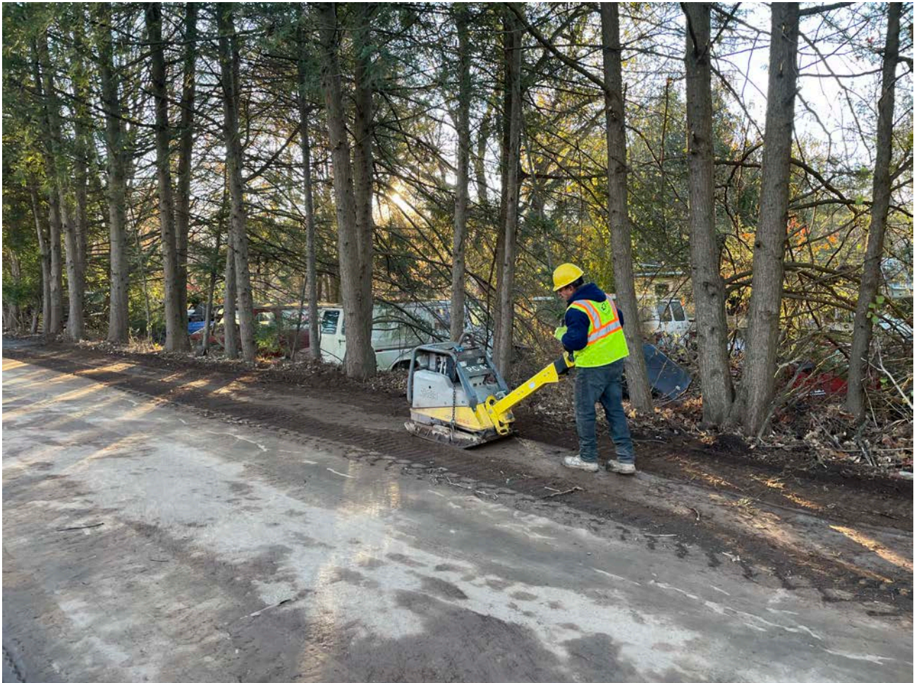
Picture 1: Ludlow compacting native fill that was backfilled over the 1.5" copper water service line that they installed on the south side of the driveway at the 228 Maple Avenue property. View to the southeast.
