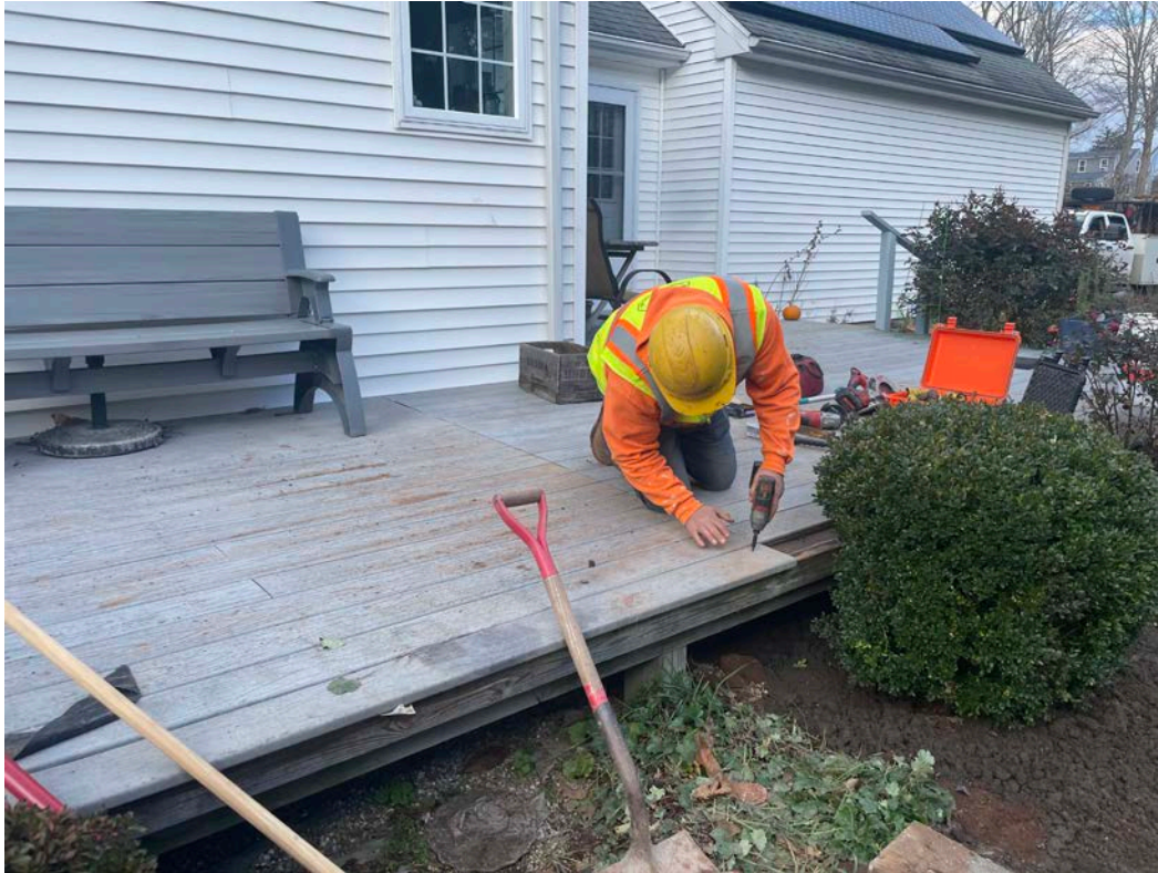
Picture 9: Ludlow replacing deck slats on the south side of the 228R Maple Avenue residence after they installed a 1.5" copper water service line. View to the east.
