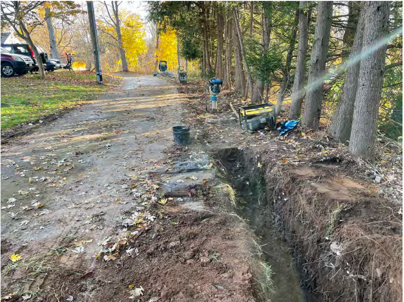
Picture 2: Trench that Ludlow has begun to backfill over a 1.5" copper water service line at the 228 Maple Avenue property in Durham. View to the east.
