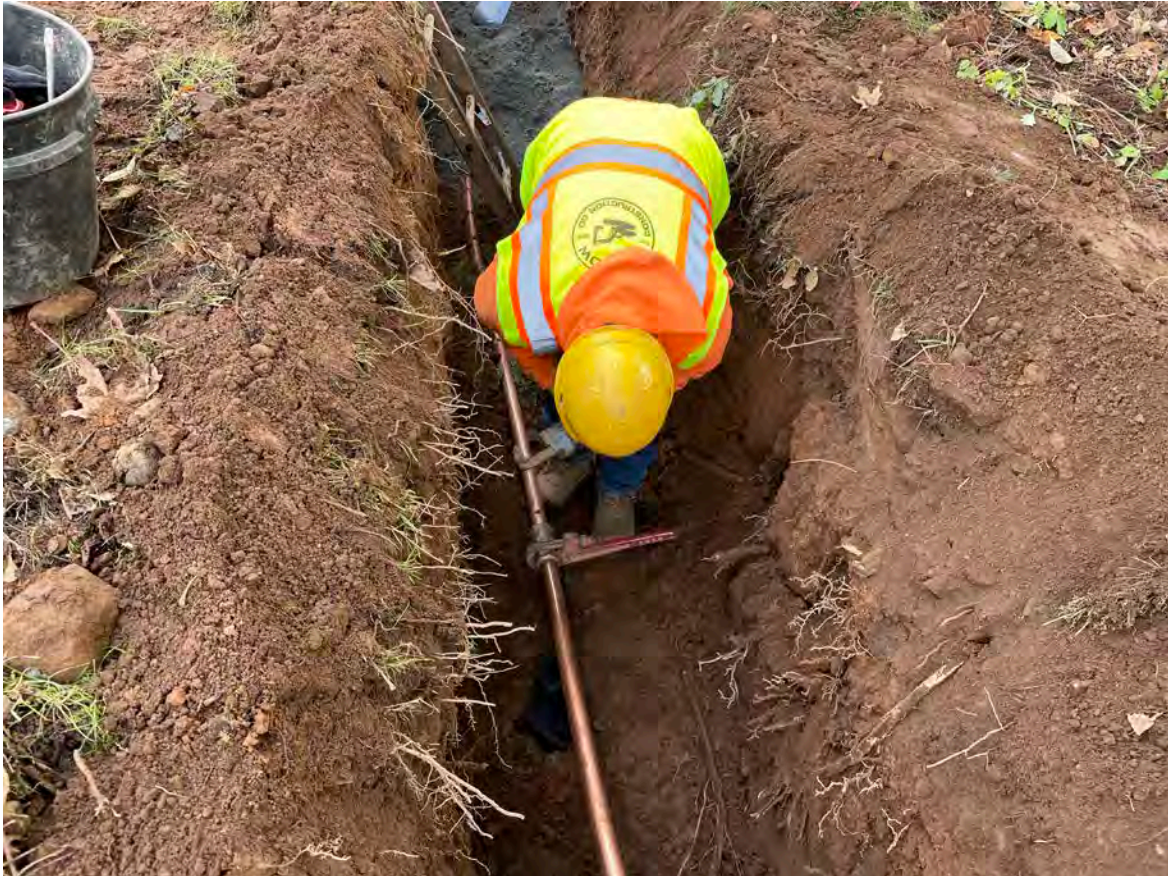
Picture 3: Ludlow joining two sections of 1.5" copper water pipe together at the 228R Maple Avenue property. View to the east.
