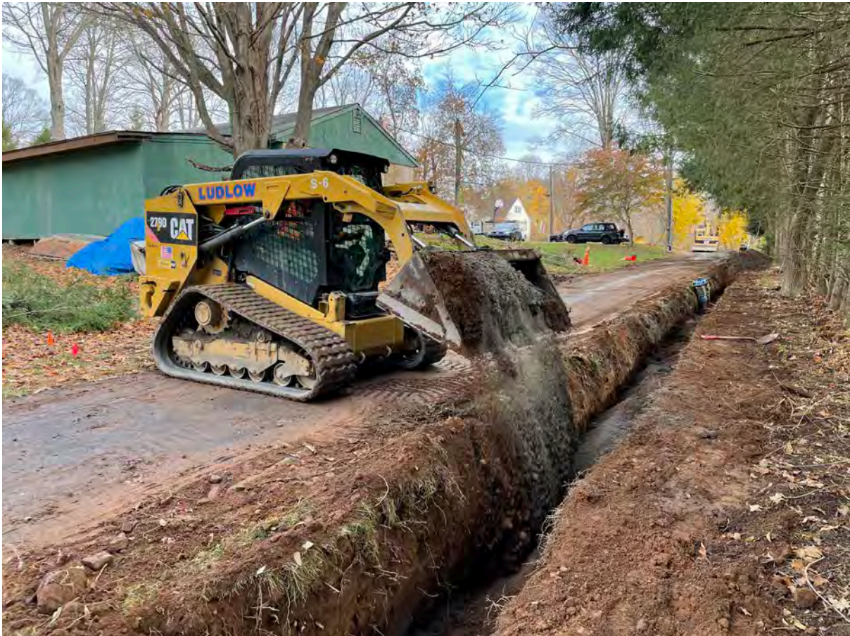
Picture 5: Ludlow placing sand over the 1.5" copper water service line they are installing at the 228R Maple Avenue property. View to the east.
