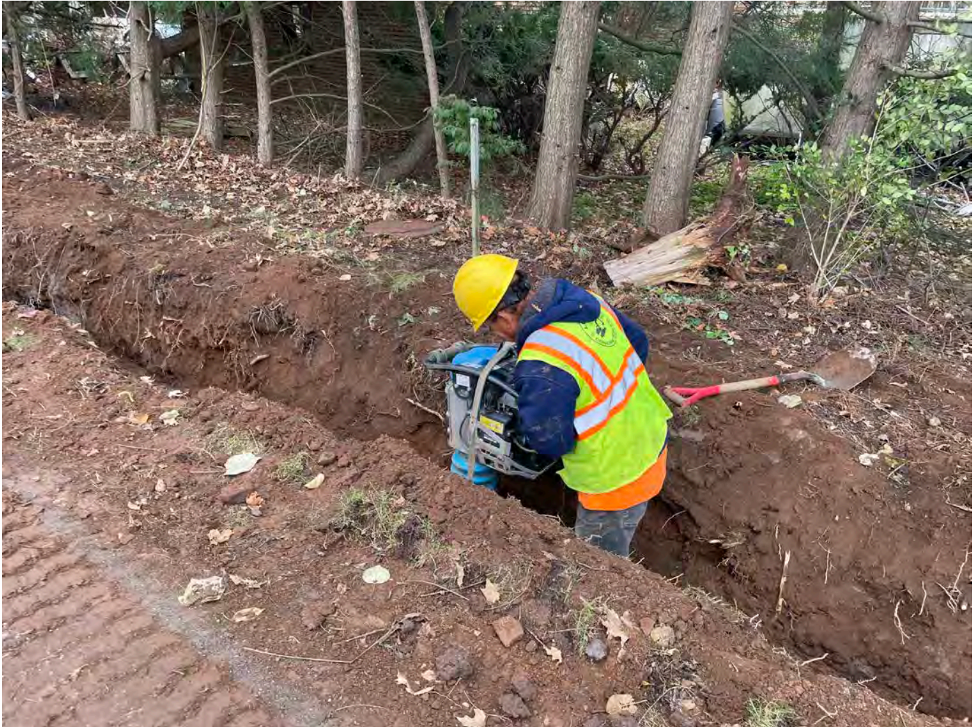
Picture 8: Ludlow compacting native fill that has been placed in a 1' lift over they sand and caution tape that was placed over the 1.5" copper water service line they installed at the 228R Maple Avenue property. View to the southeast.
