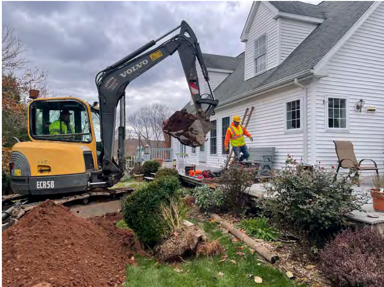
Picture 6: Ludlow excavating a trench on the south side of the 228R Maple Avenue residence for the installation of a 1.5" copper water service line. View to the west.
