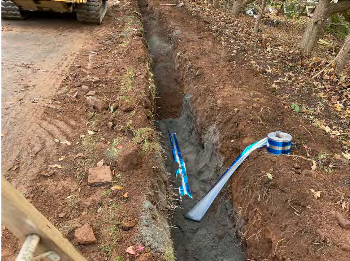
Picture 4: Sand, caution tape, and native fill that Ludlow has placed over the 1.5" copper water service line they installed at the 228R Maple Avenue property. View to the east.
