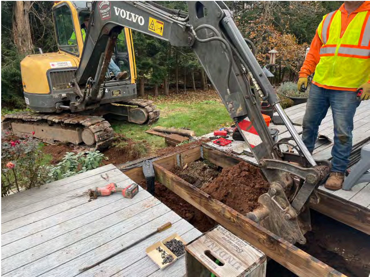
Picture 7: Ludlow excavating a trench on the south side of the 228R Maple Avenue residence for the installation of a 1.5" copper water service line. View to the southwest
