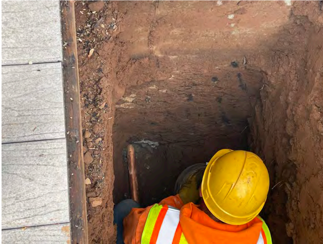
Picture 9: Ludlow using non-shrink grout to secure a 1.5" copper water service line where it penetrates the southern foundation of the 228R Maple Avenue residence. View to the north
