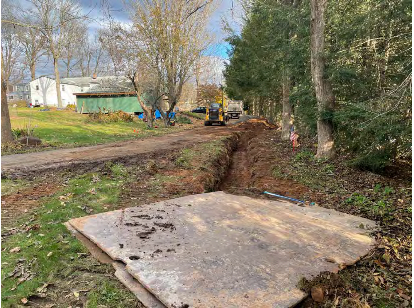
Picture 10: View of the trench that Ludlow has partially backfilled over 1.5" copper water service line that they installed on the south side of the driveway at the 228R Maple Avenue property. View to the east.
