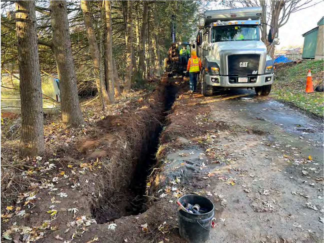
Picture 1: Trench that Ludlow is excavating on the south side of the driveway at the 228 Maple Avenue property for the installation of a 1.5" copper water service line. View to the west.
